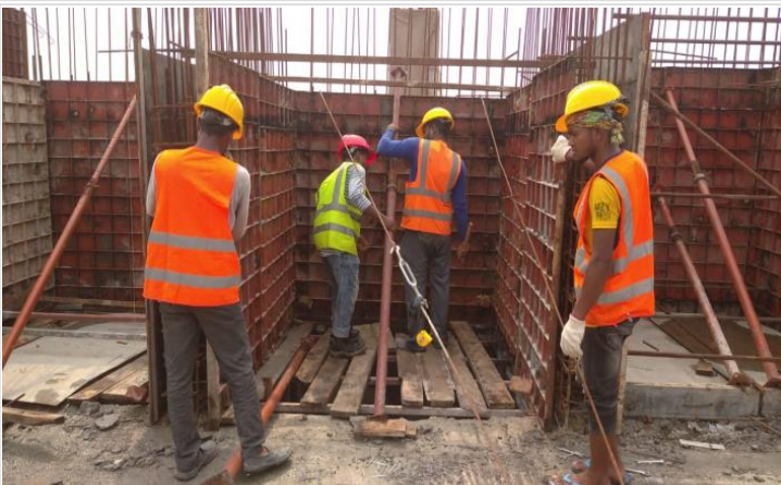
Ground floor Lift Core Shuttering on 07-06-21
