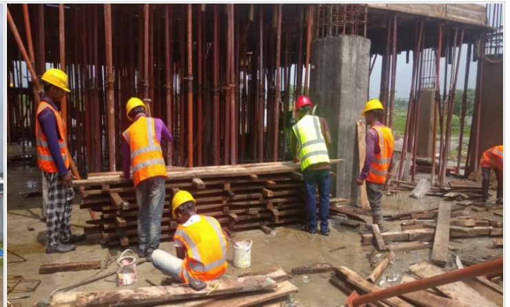
1st floor Slab Shuttering on 15-06-21
