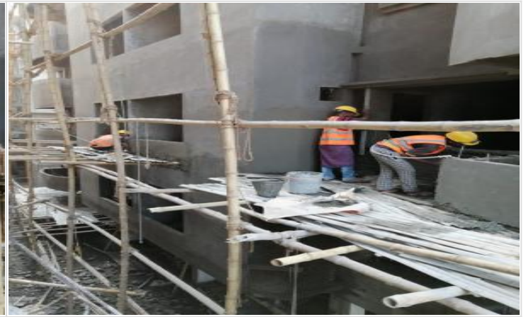
Bulding-Q-Out-side Plastering on 09-05-21
