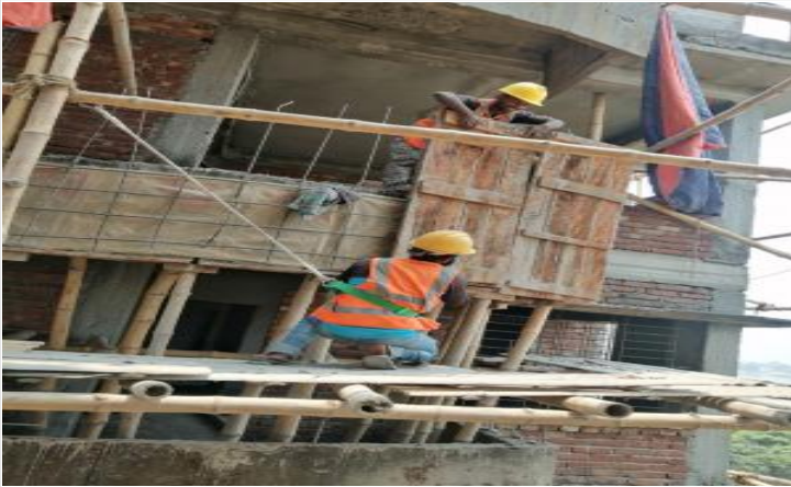
Drop Wall Shuttering on 01-05-21
