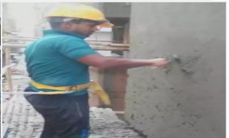
Out-side Plaster Work on 04-05-21
