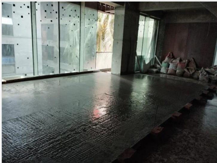
4th Flr-Floor Raining Concreting Complet
