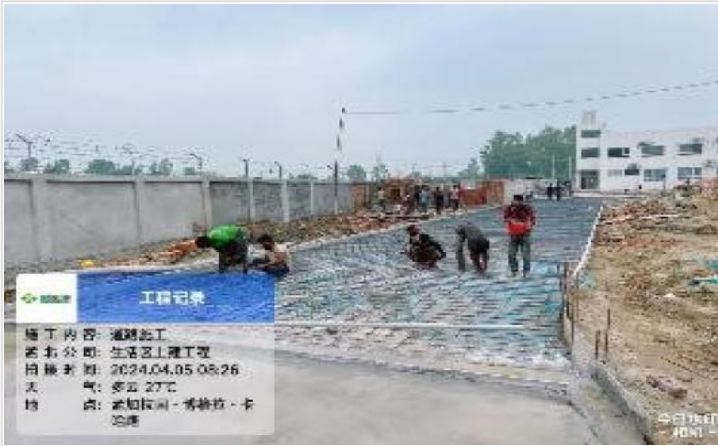
Road-Re-bar work on 05-04-24
