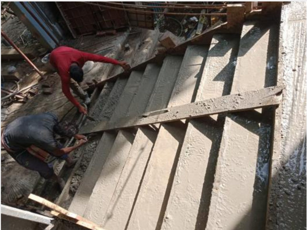
1st Floor Stair Concreting on 27-06-21
