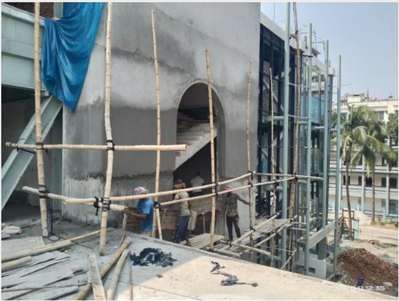
Stair no.2 Outside plaster on 11-10-21
