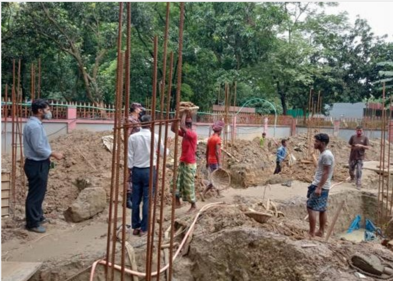
Sub-station grade beam earth cutting wor on 02-08-21
