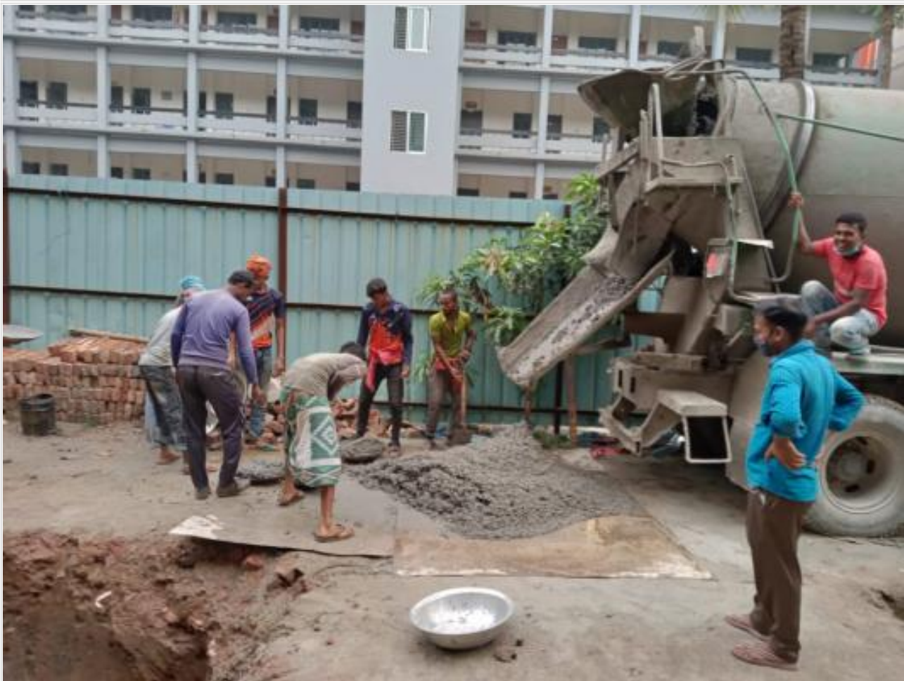
Canopy Base Concreting on 03-05-21
