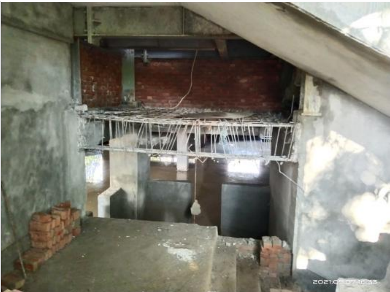
Beam dismantling for MDB Room on 07-09-21
