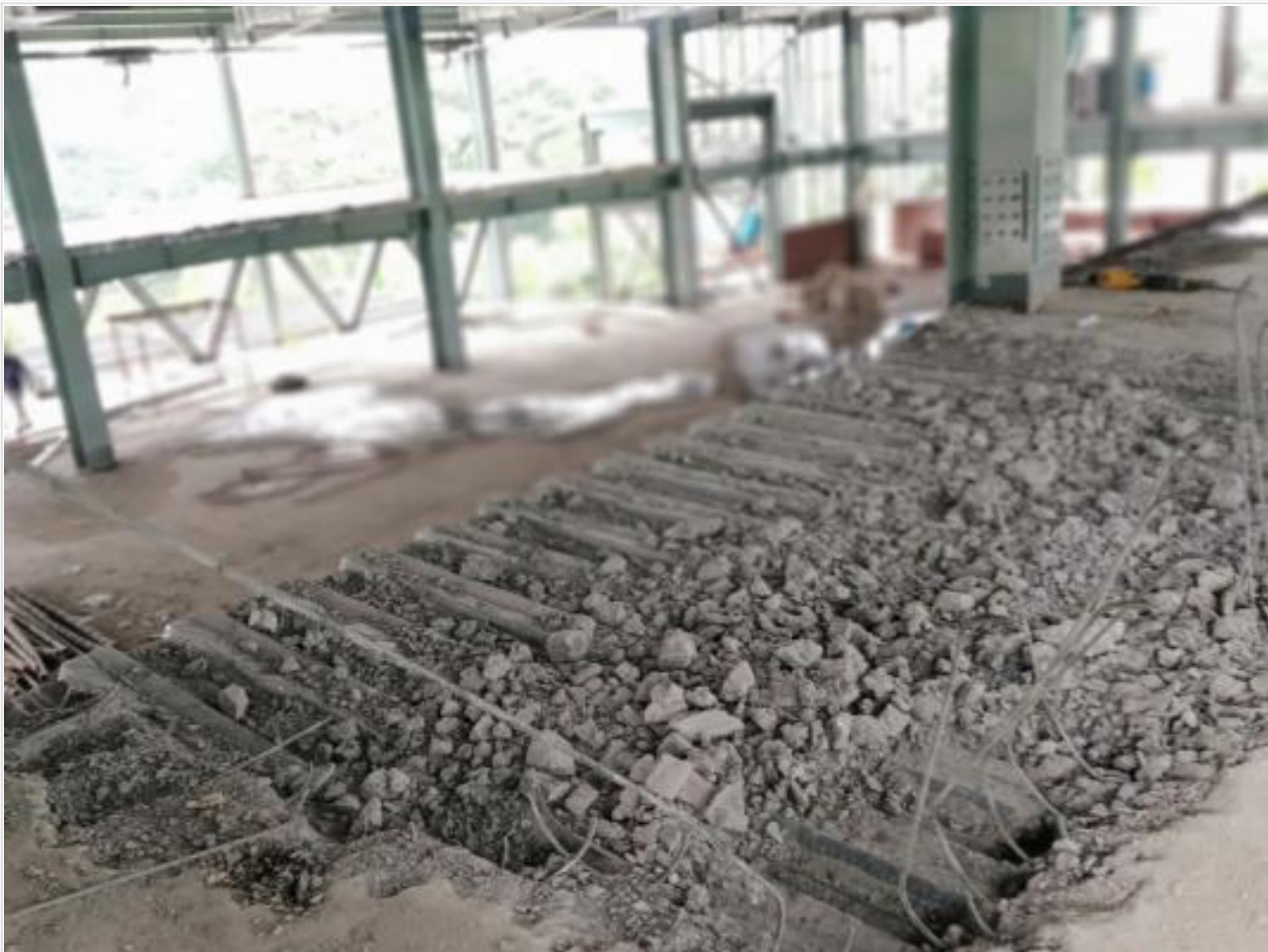
FF Mezzanine floor dismantling work on 18-08-21
