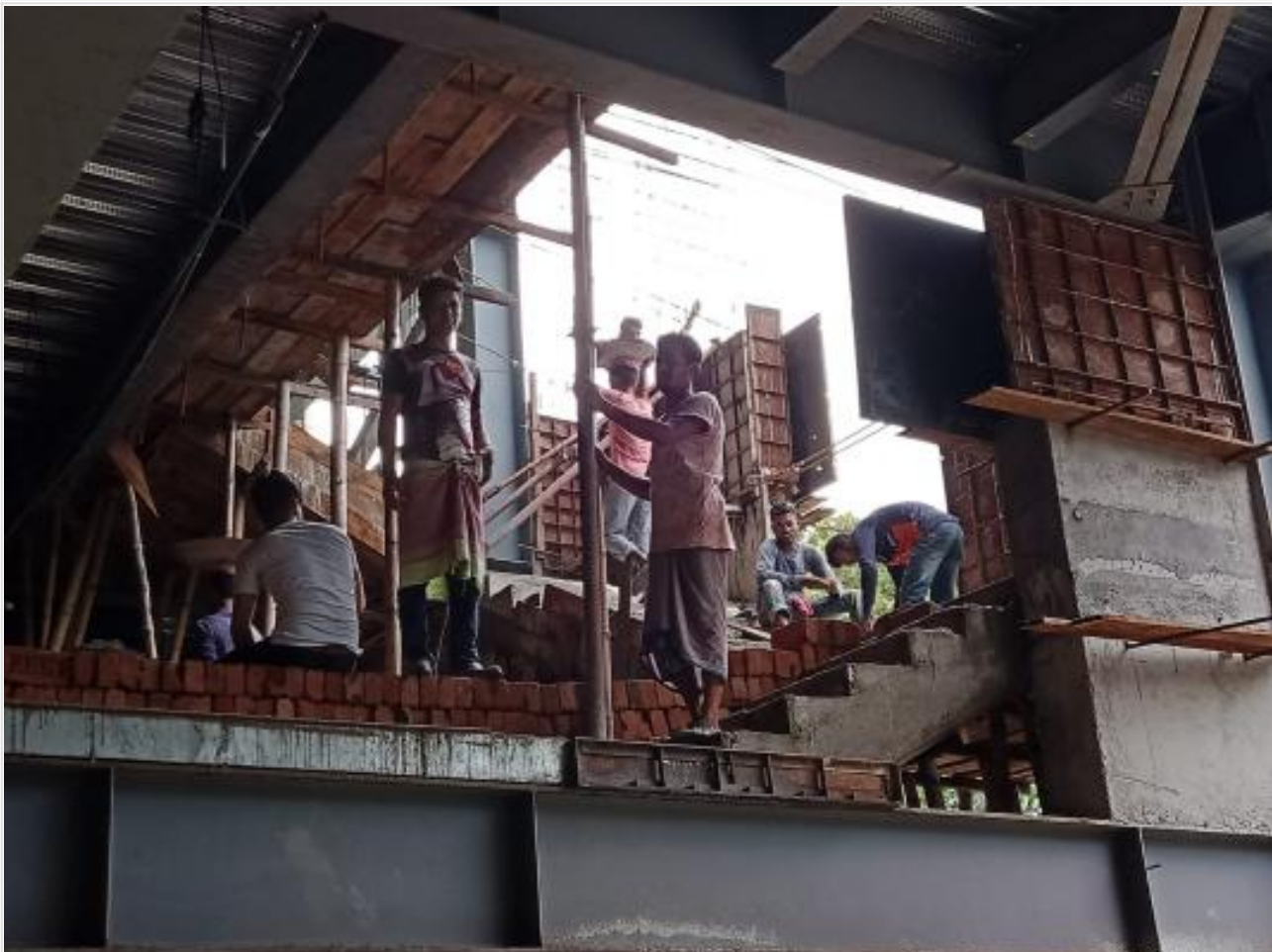
GF Mazzanine stair wall casting on 04-08-21
