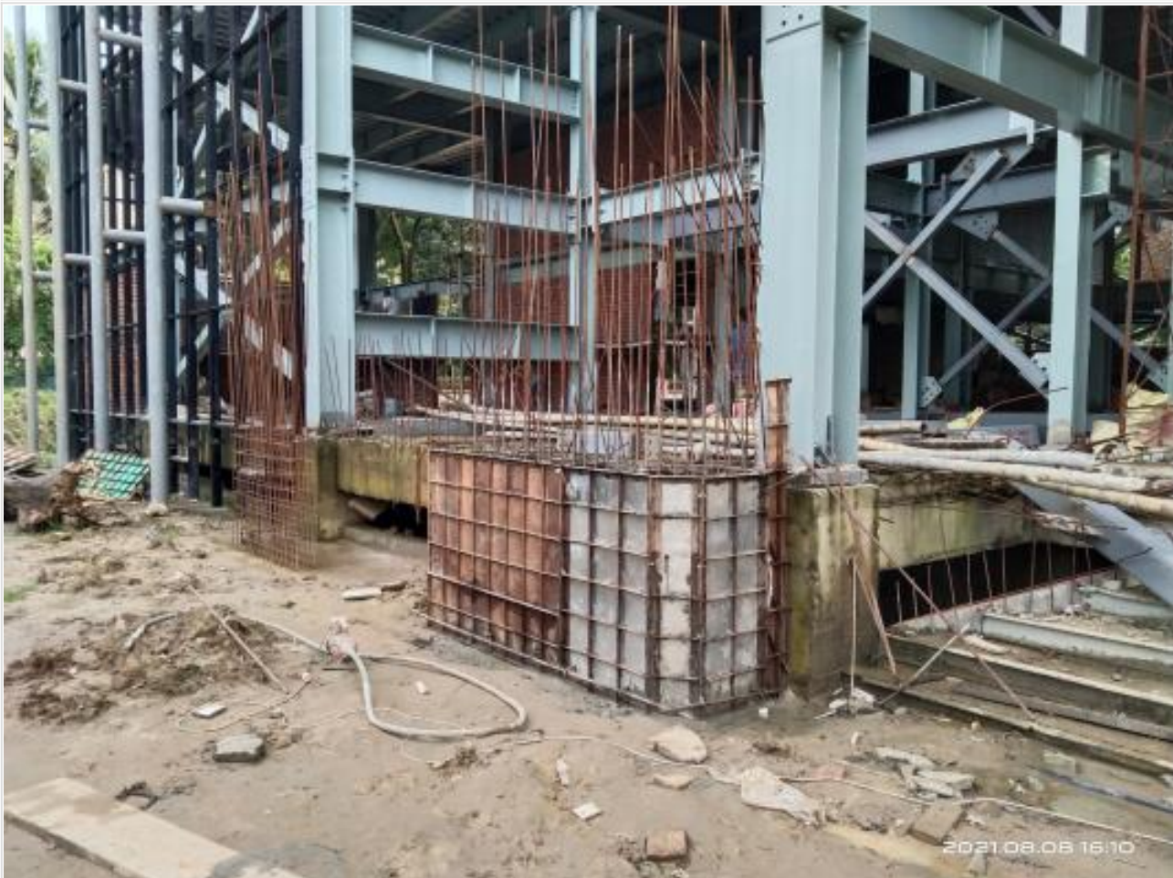
GF Stair no-3 shuttering and casting on 08-08-21
