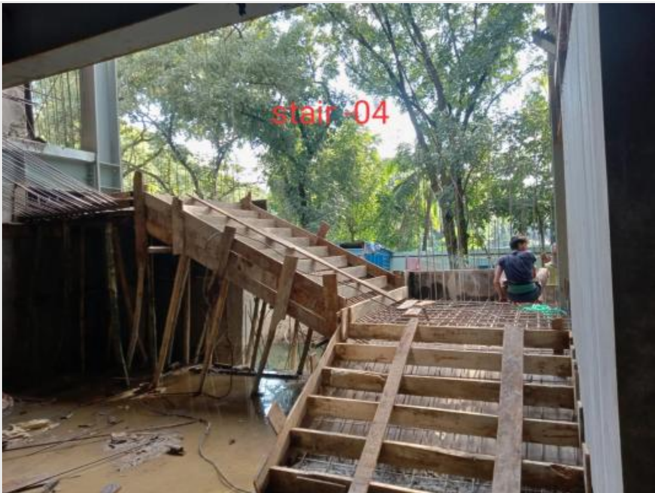
GF Stair casting on 31-08-21
