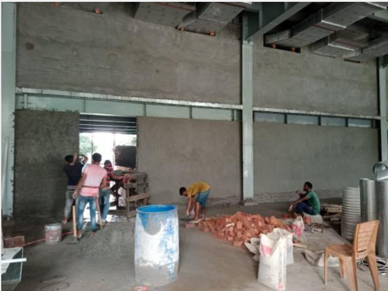
GF plaster work on 13-08-21
