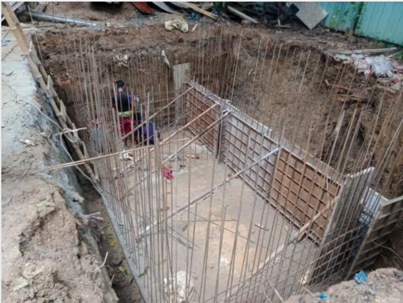
Spptic tank RCC Base casting on 17-09-21
