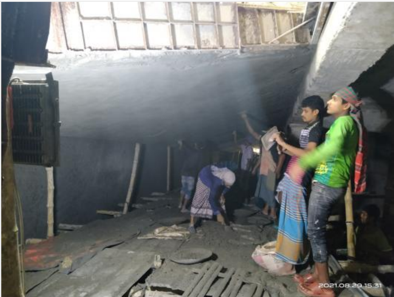
Basement ceiling plaster on 29-08-21
