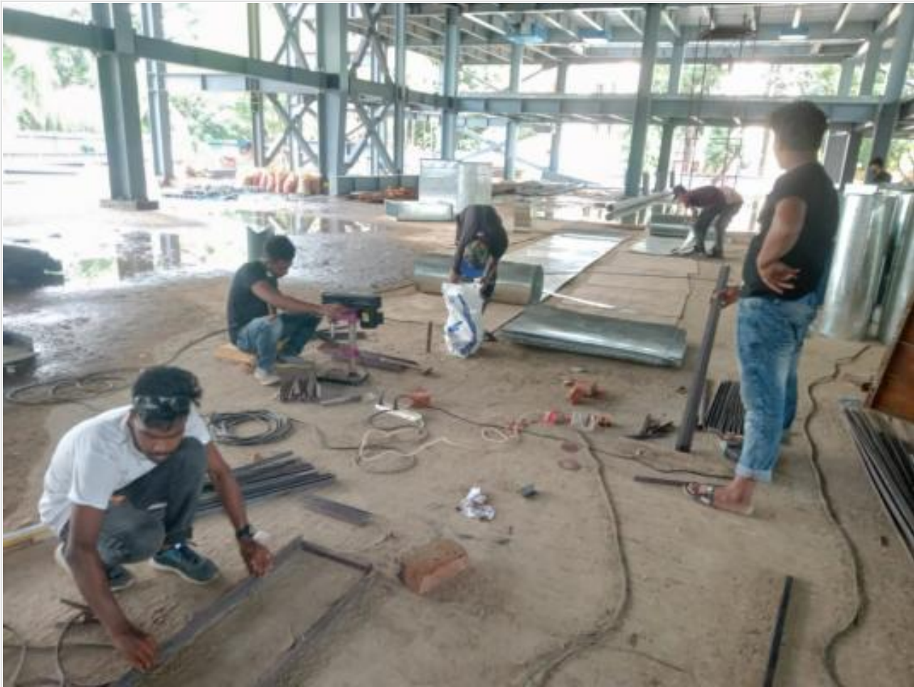
AC Duct Making on 19-05-21
