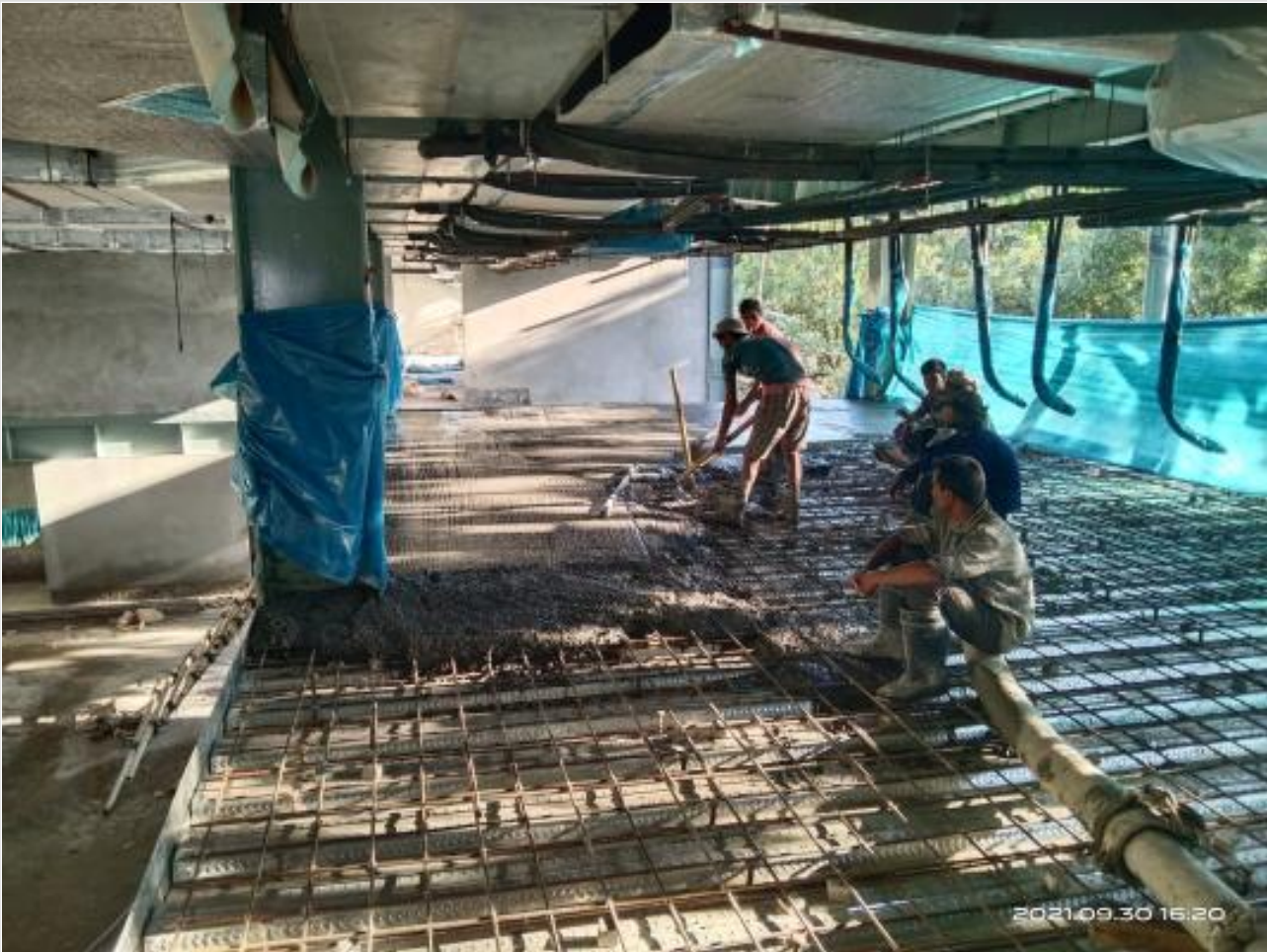
1F Mezzanine Slab Concreting on 30-09-21
