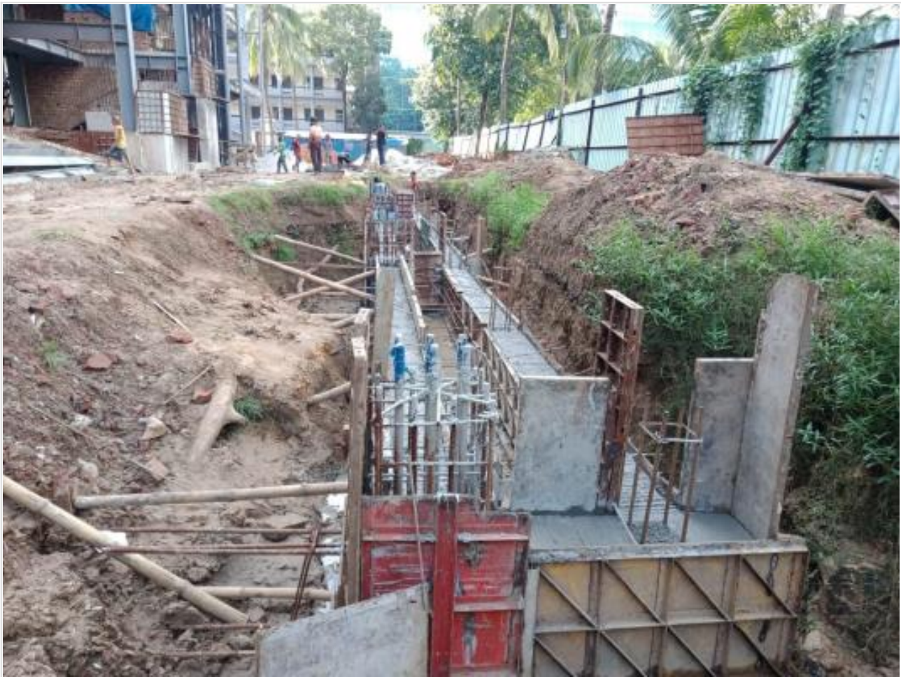
Porch Grade Beam Beam Concreting on 25-06-21
