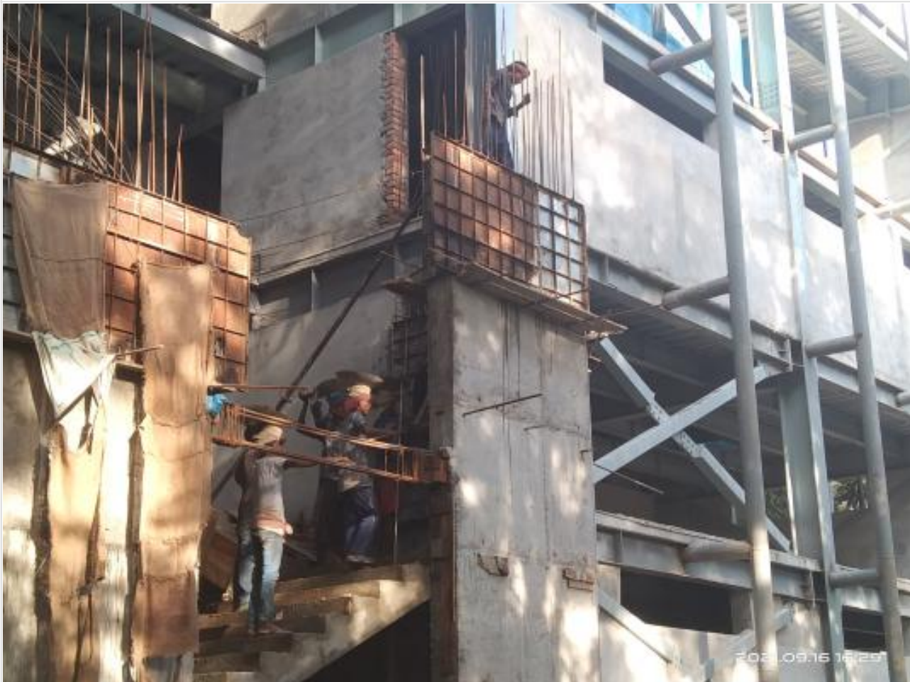
Stair wall casting on 16-09-21
