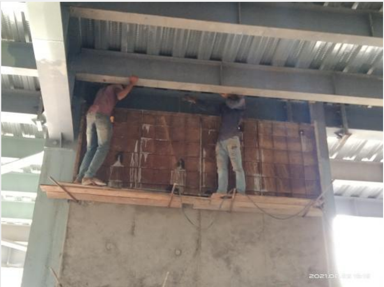
GF Stair Shuttering on 23-08-21
