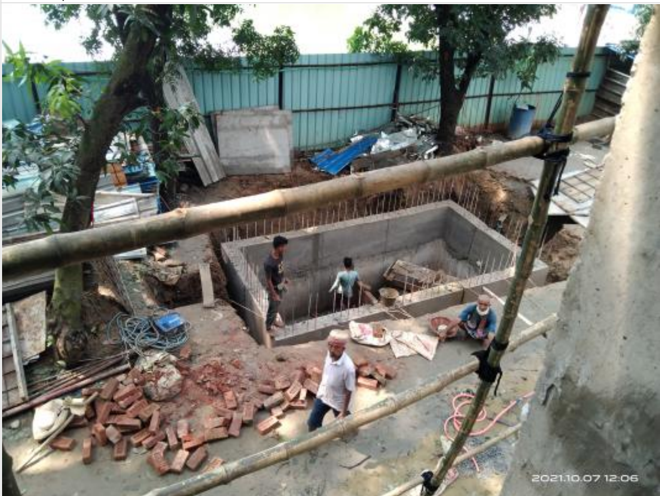
Septic partition wall on 07-10-21
