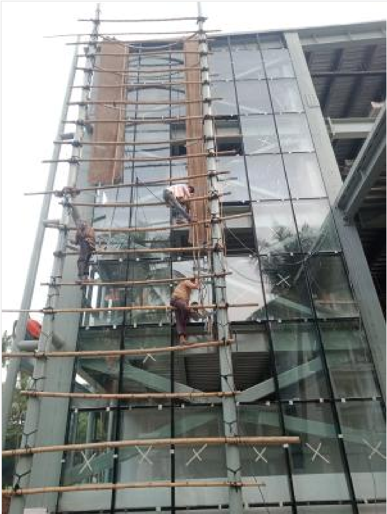
ACP angle frame setting on 11-10-21
