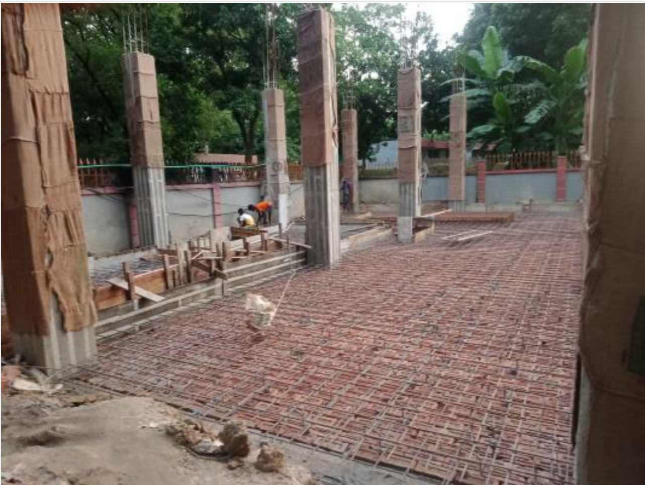
Generator room floor rod binding on 06-09-21
