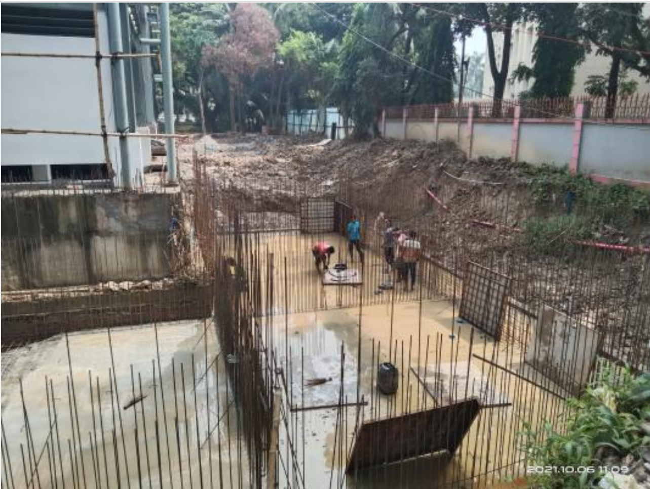
Fire tank wall shuttering on 06-10-21
