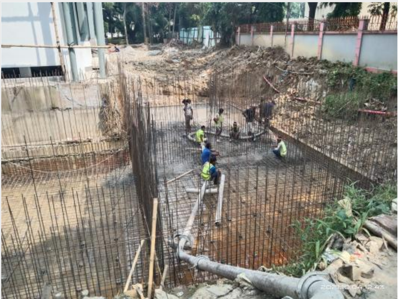
Fire tank base casting on 04-10-21
