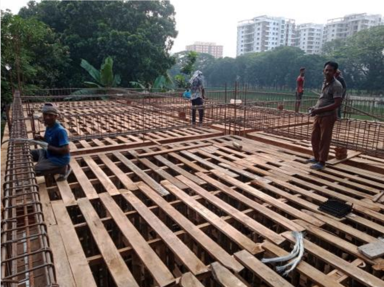
Generator room slab shuttering on 26-09-21
