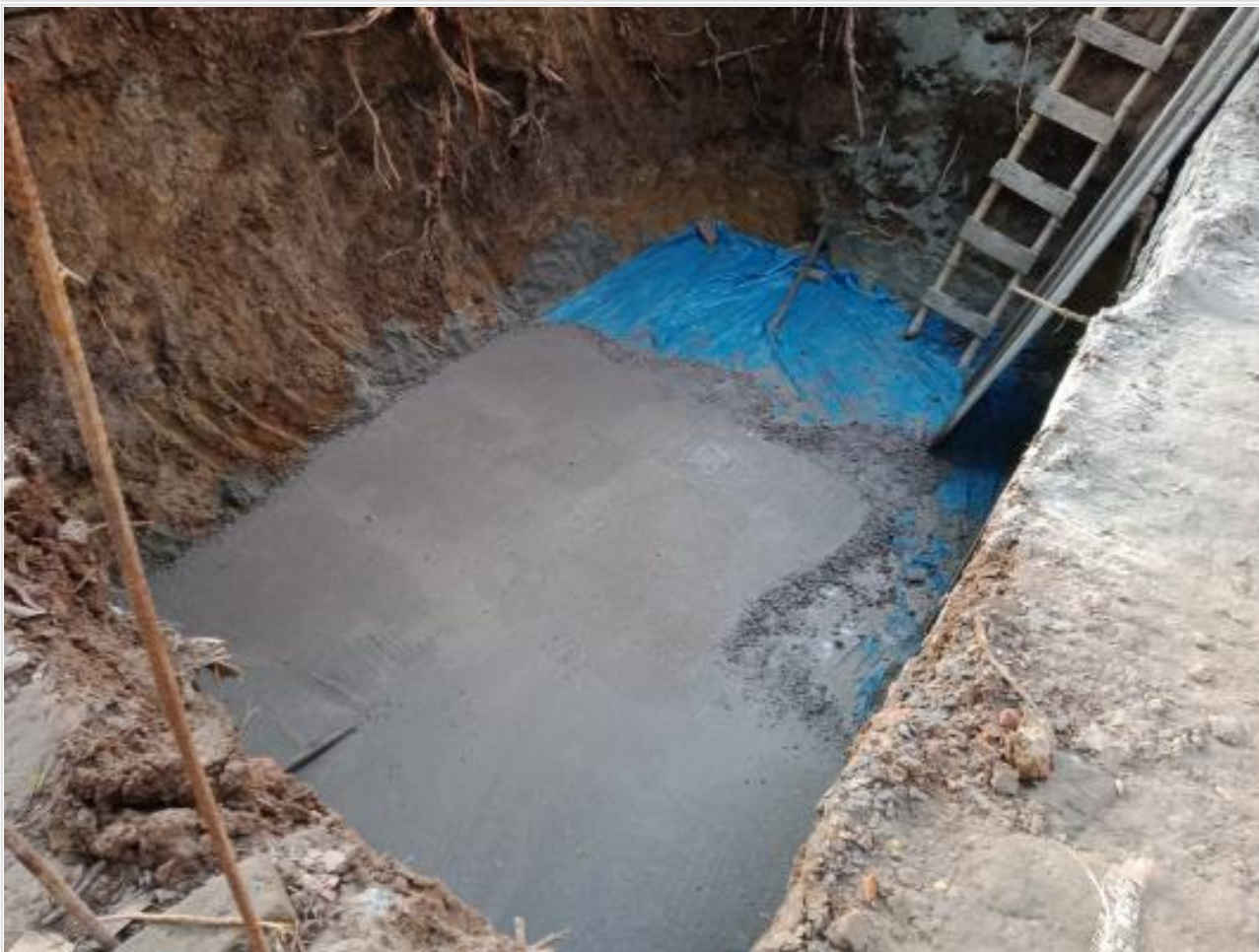
Septic tank cc work on 15-09-21
