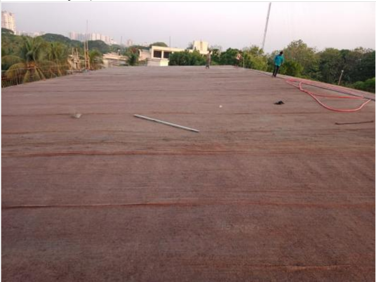
Hessian Cloth Covering after Concreting on 07-05-21
