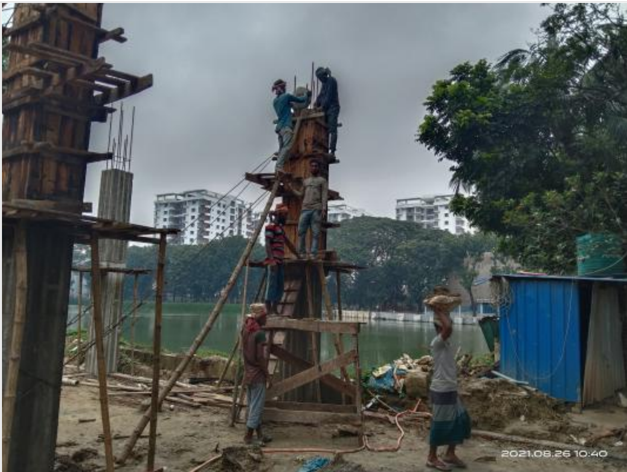
Generator room Column casting on 26-08-21
