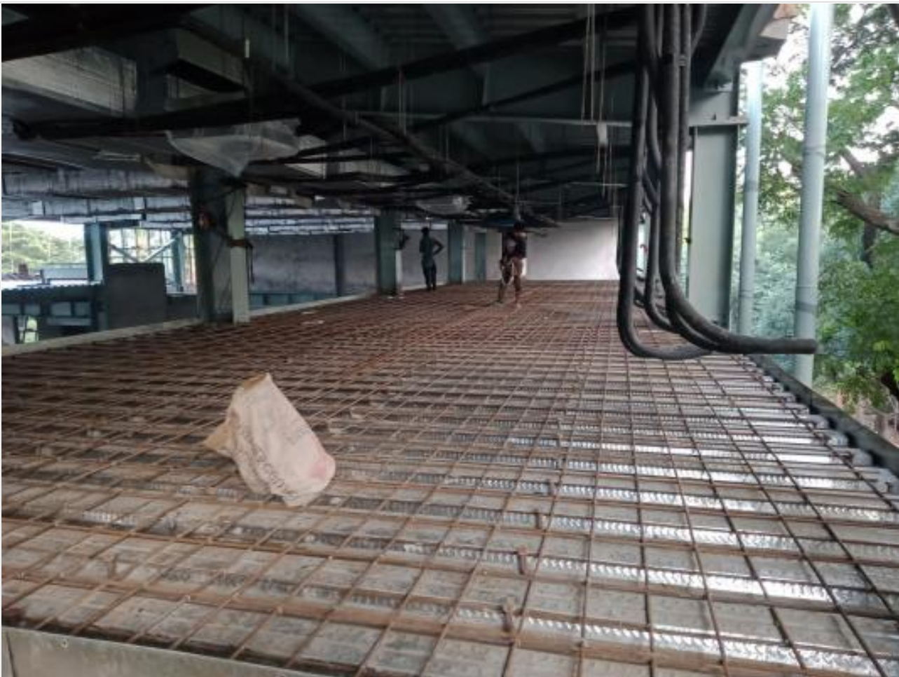
Rod binding at 1st floor mezzanine on 26-09-21
