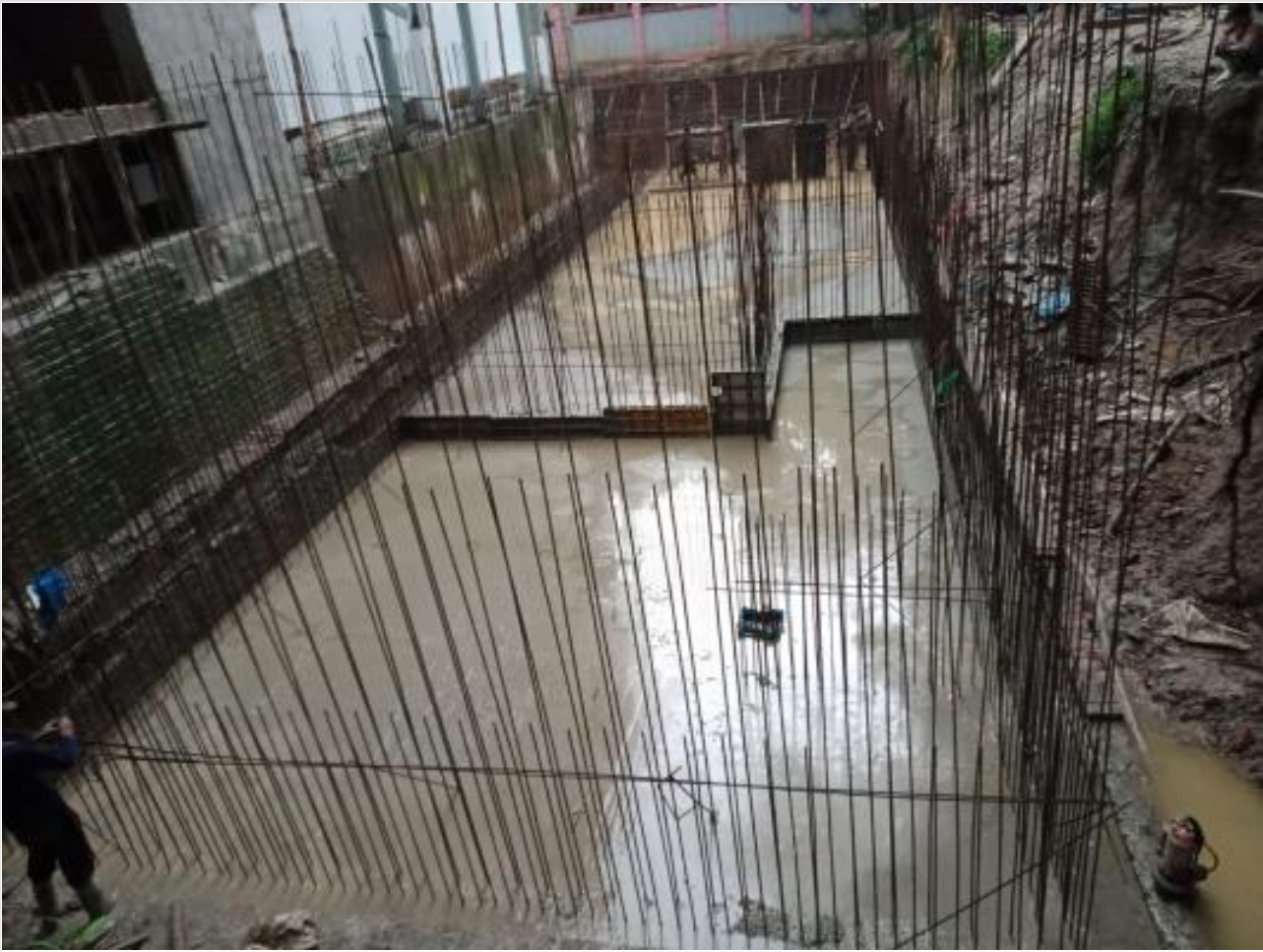
Fire Tank base casting on 20-10-21
