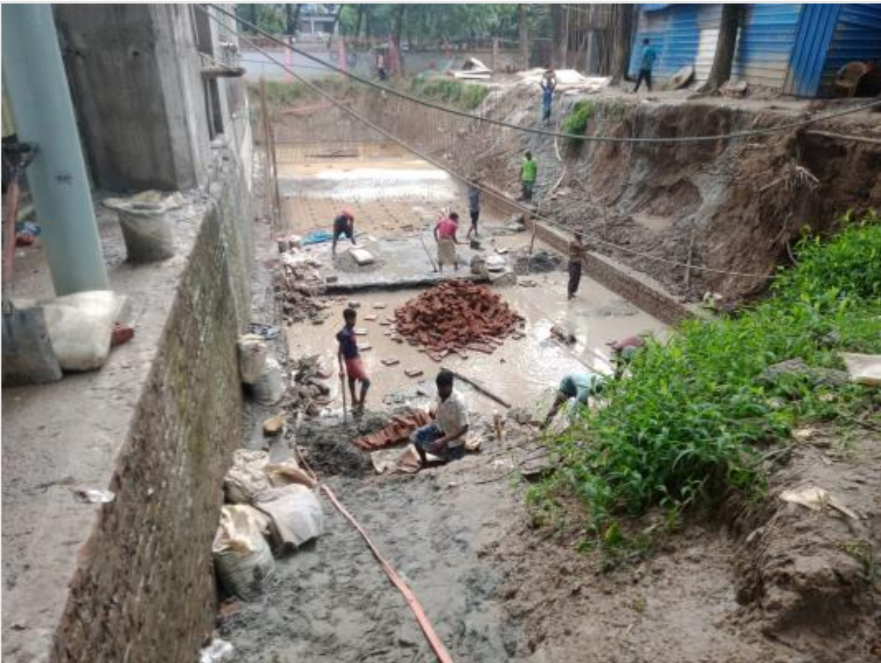
Fire Tank clay protection wall making on 08-10-21
