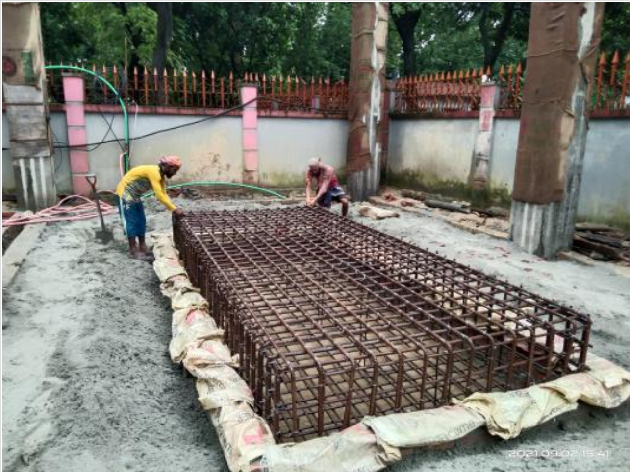
Generator foundation rod binding on 02-09-21
