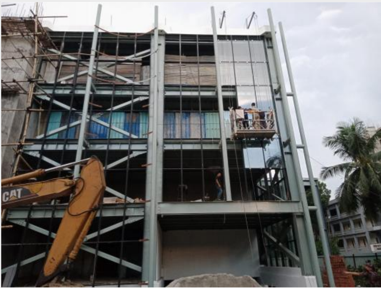
Glass fitting work on 27-09-21
