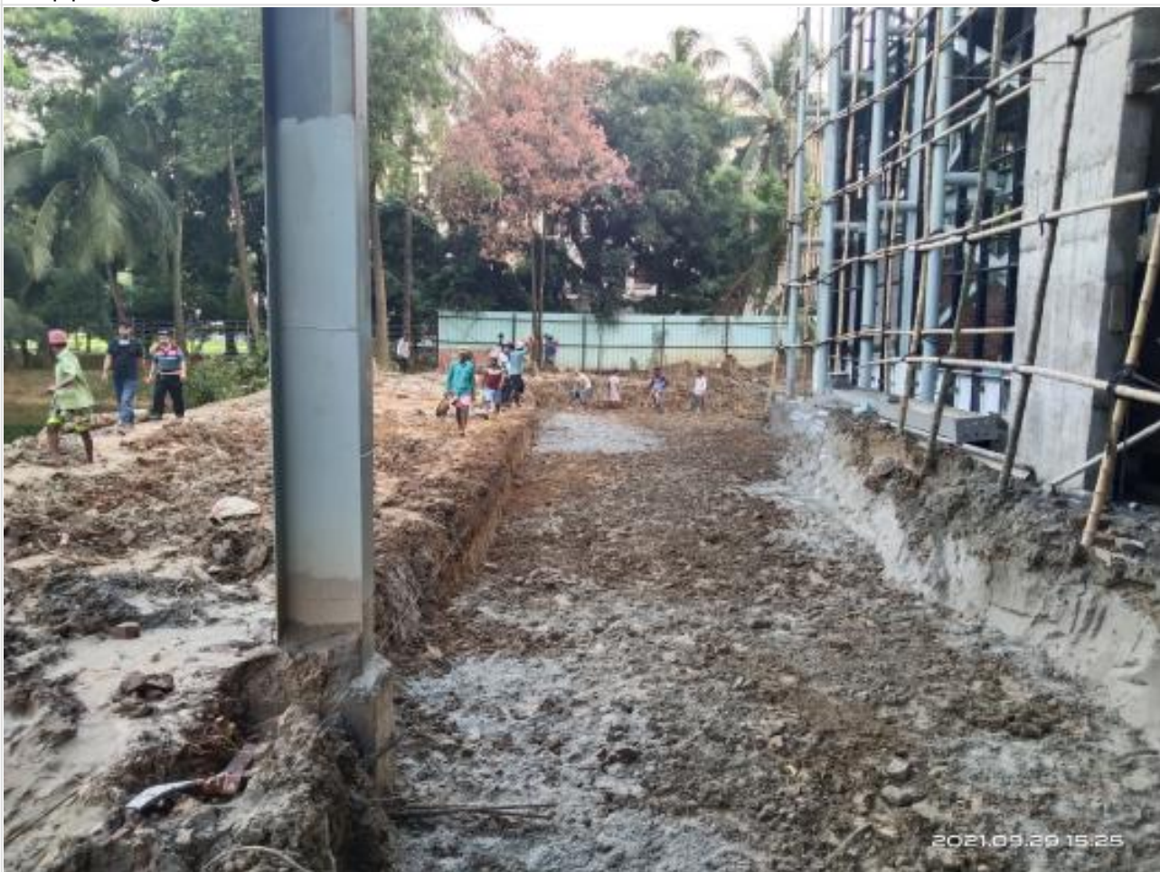
Preperation of subgrade bed of road on 29-09-21
