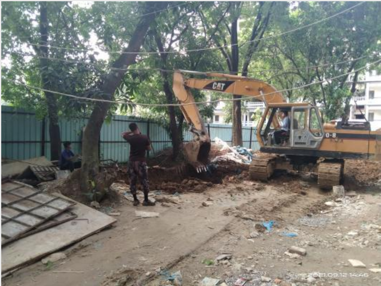
Earth excavation work for septic tank on 12-09-21
