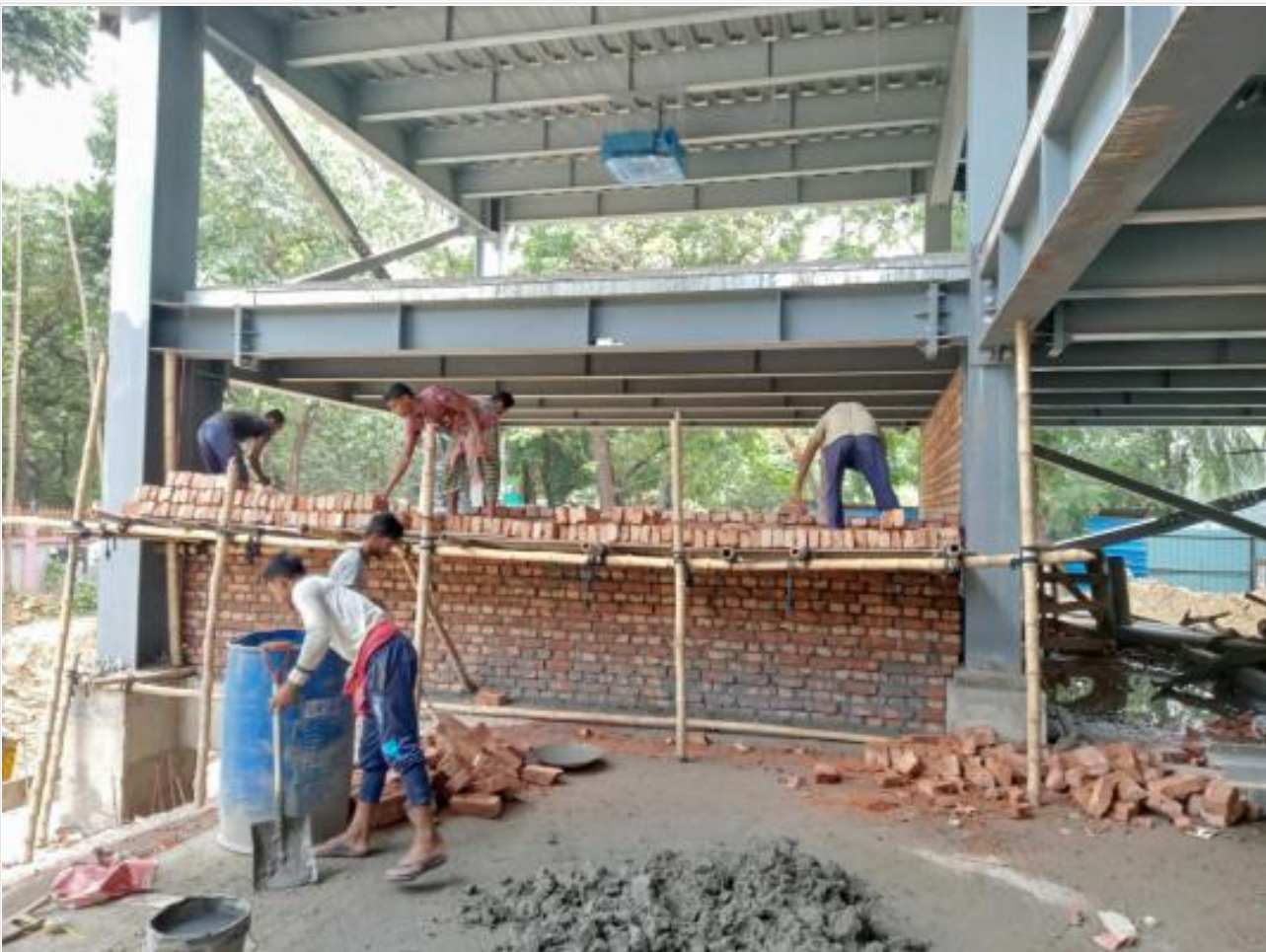
Ground Floor Brick Work on 25-05-21
