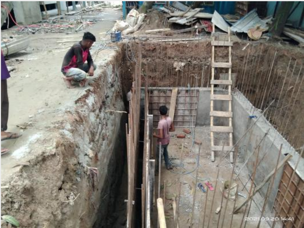
Septic Tank wall shuttering and casting on 20-09-21
