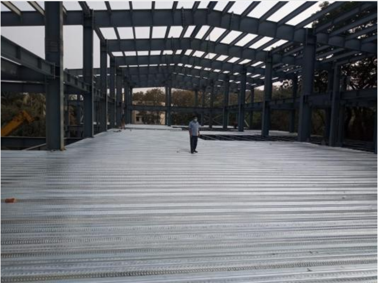
Decking Slab installation on 22-03-21
