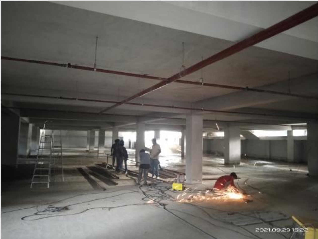
Fire pipe fitting at basement floor on 29-09-21
