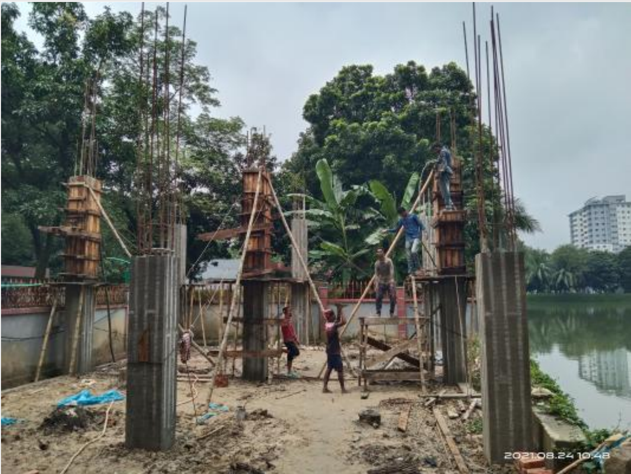
Generator room column casting on 24-08-21
