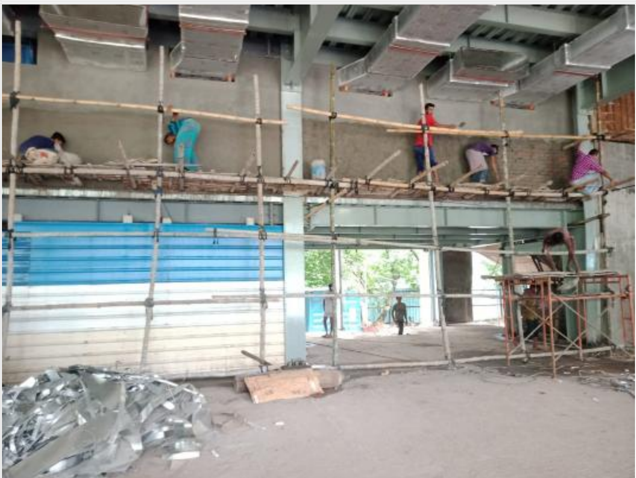
Ground Floor Mezzanine Plastering on 06-08-21
