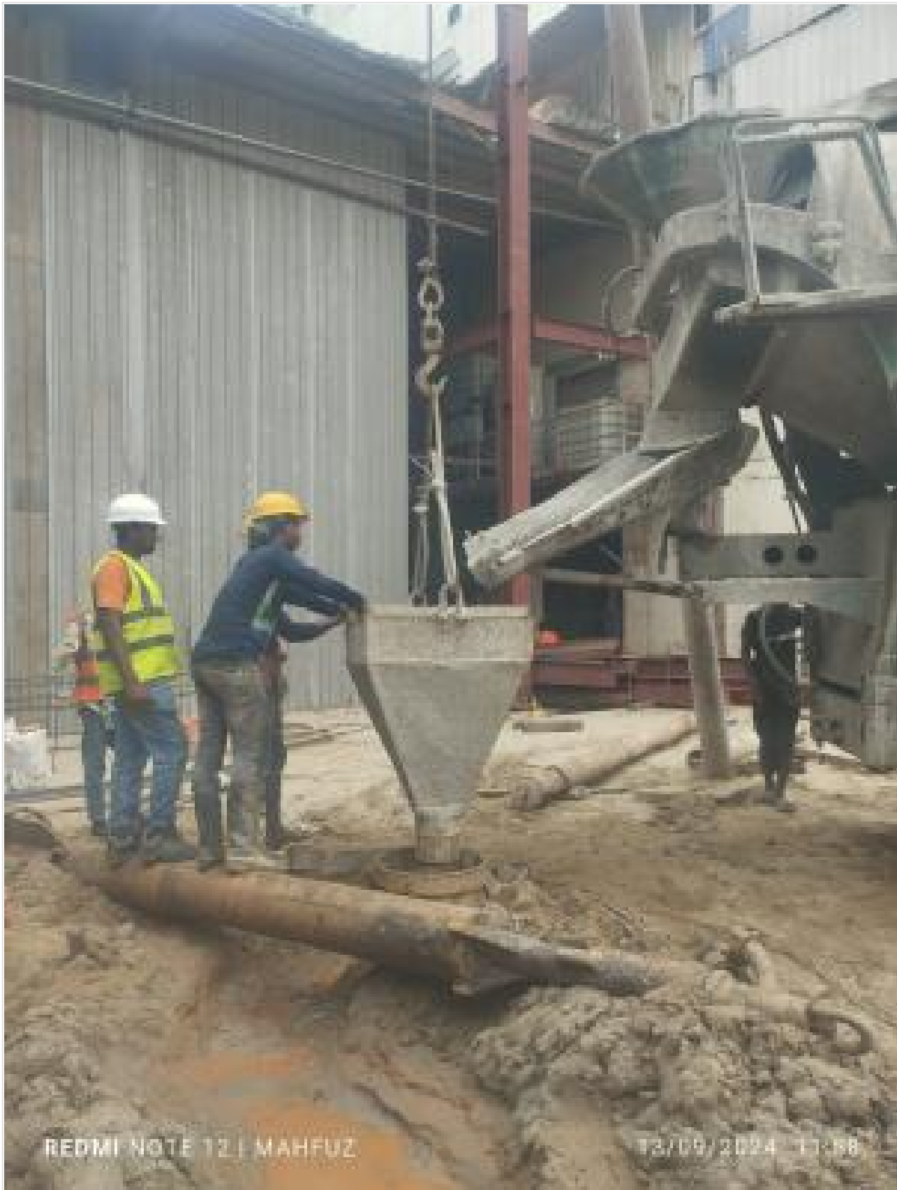
Pile concreting on 13-09-24
