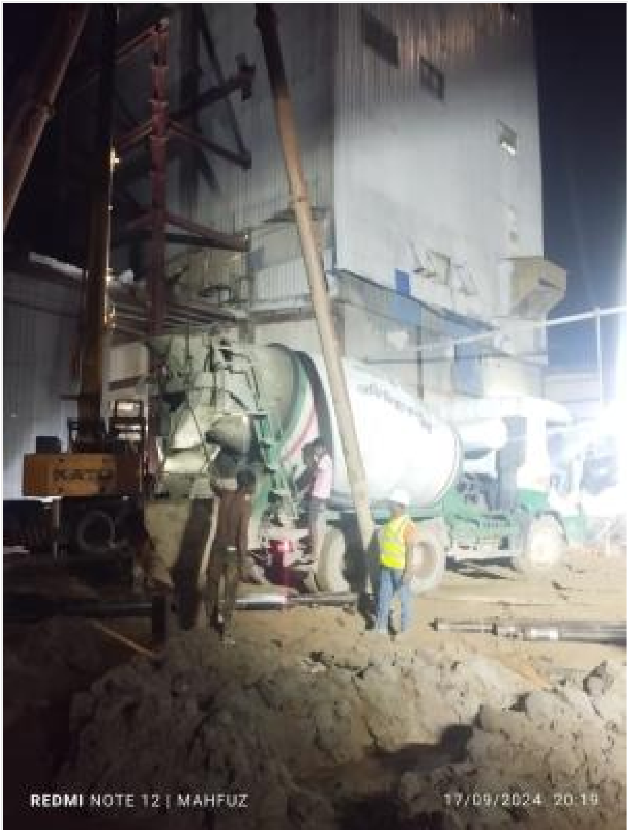
Pile concreting on 17-09-24
