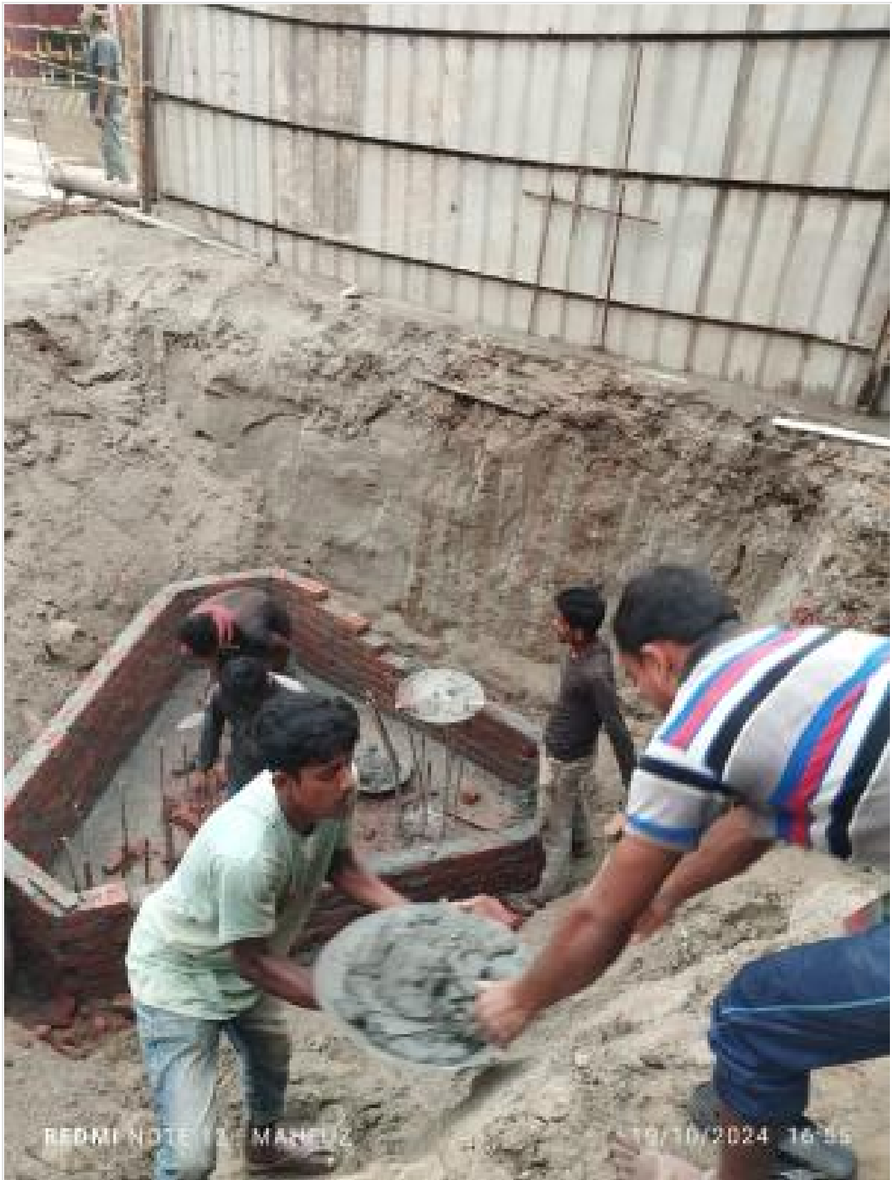
Pile Cap Brick Shuttering on 19-10-24
