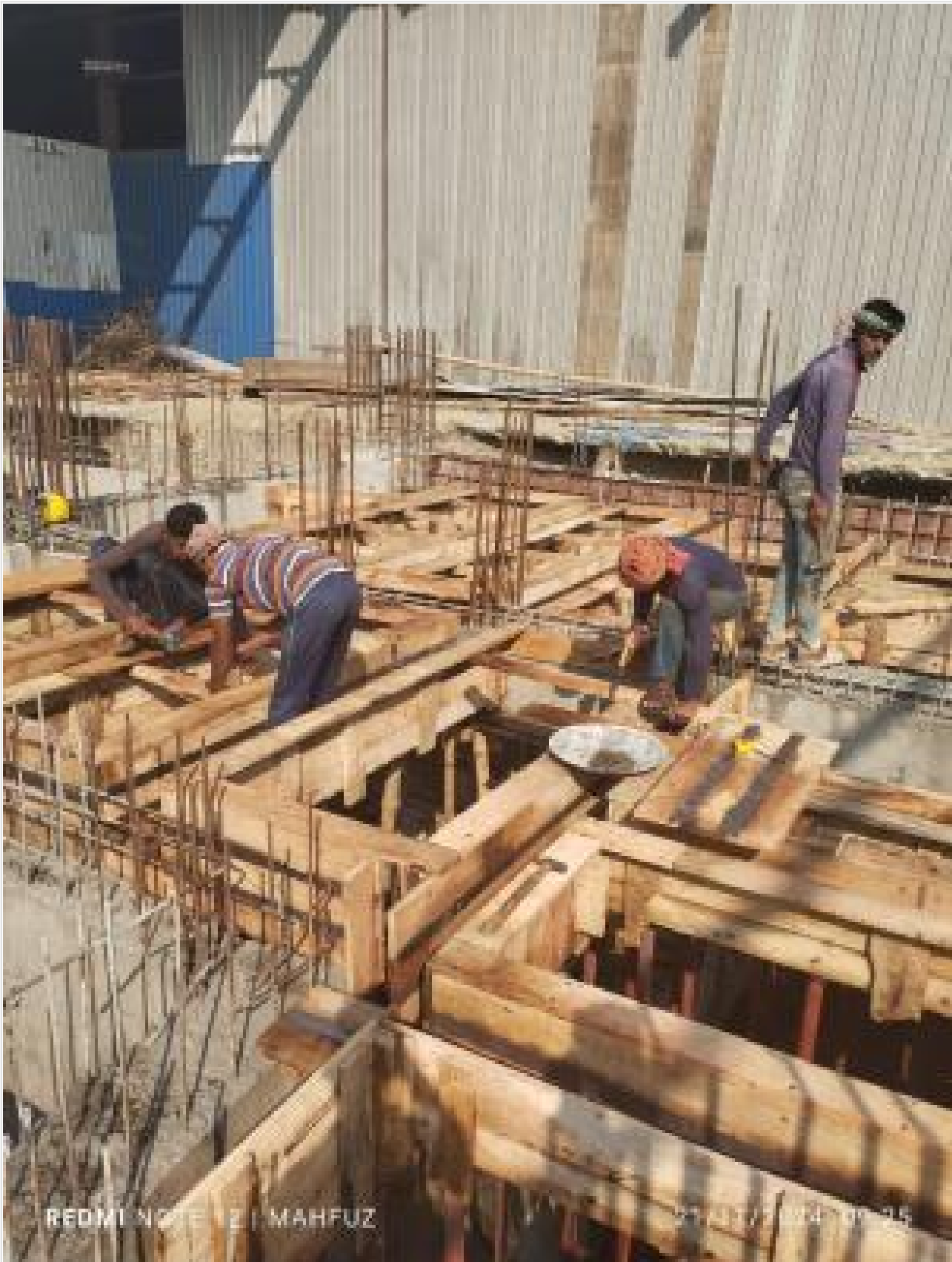
Tank slab shuttering on 22-11-24
