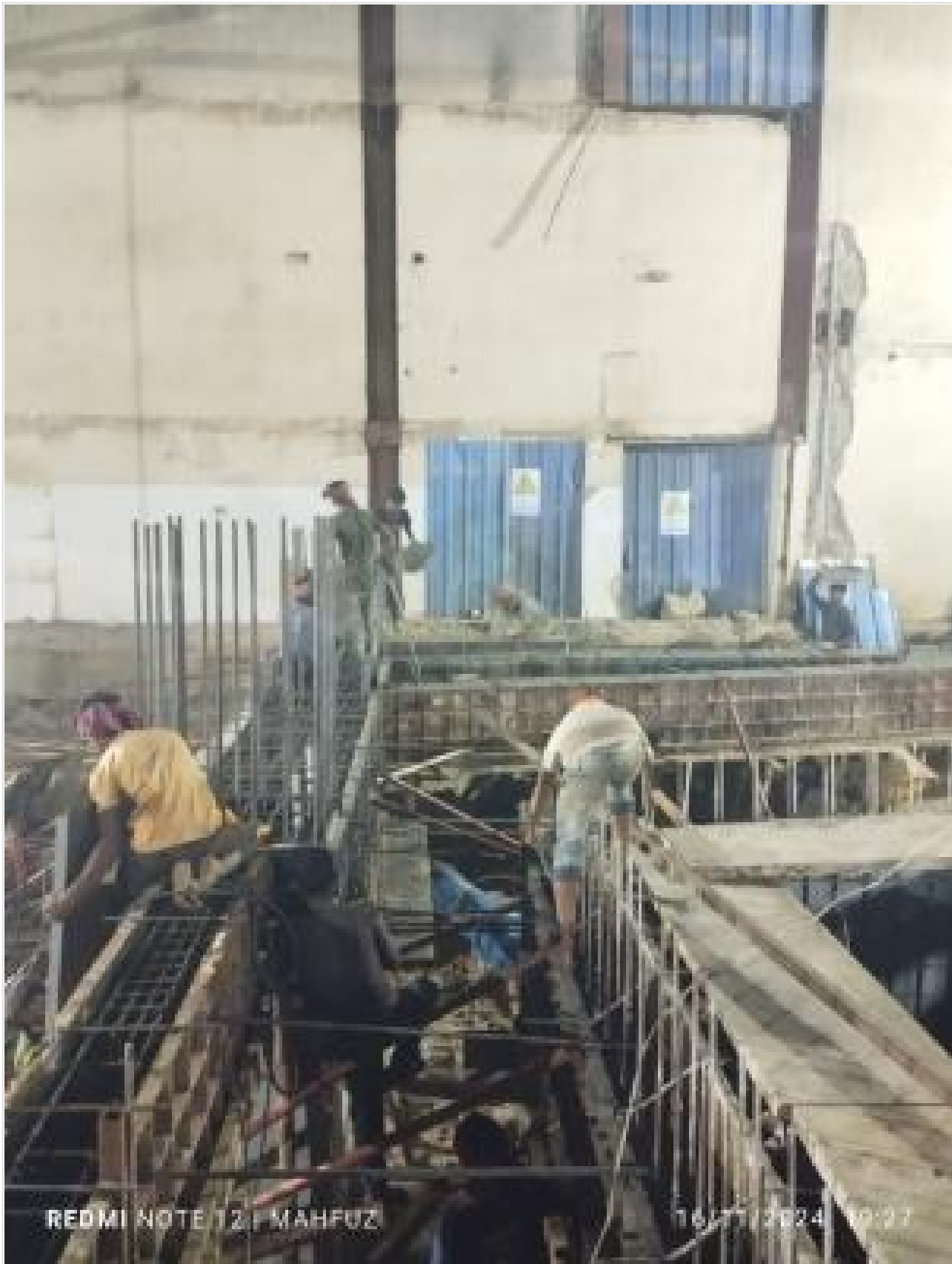
Foundation beam concreting on 16-11-24
