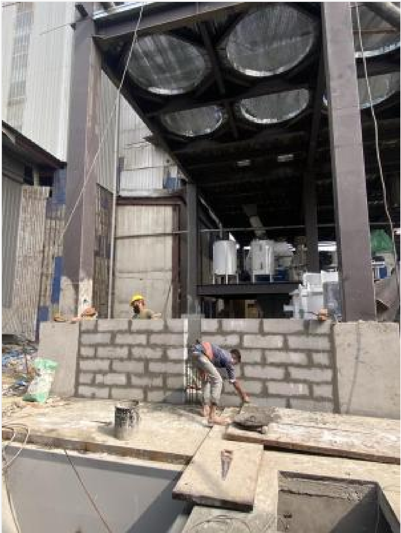
AAC block work on 23-01-25
