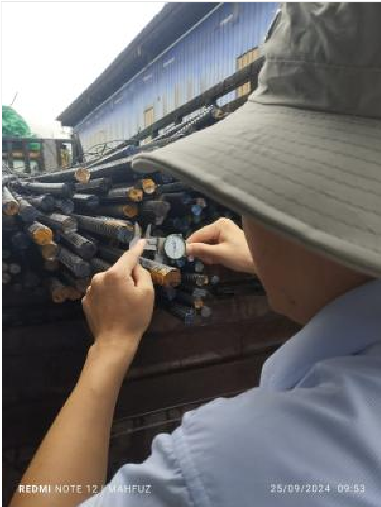
Pile cap re-bar dia checking on 25-09-24
