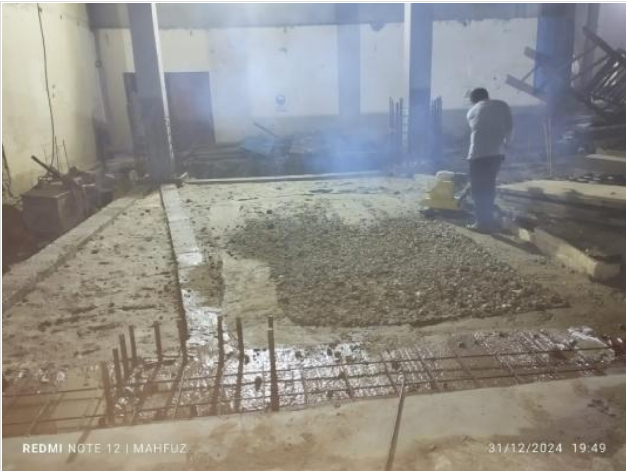
Sub-base mechanical compaction on 31-12-24
