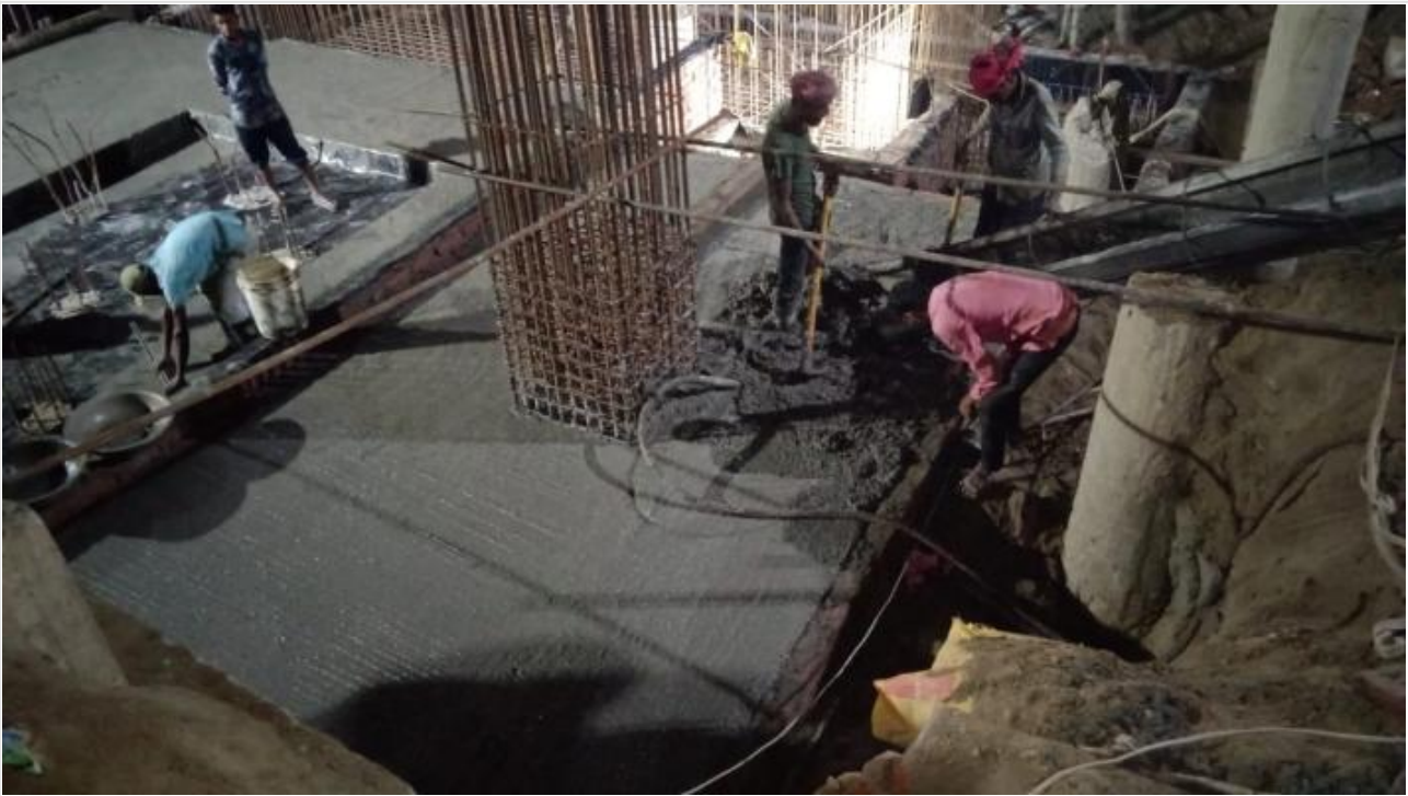
Pile cap concreting on 25-10-24
