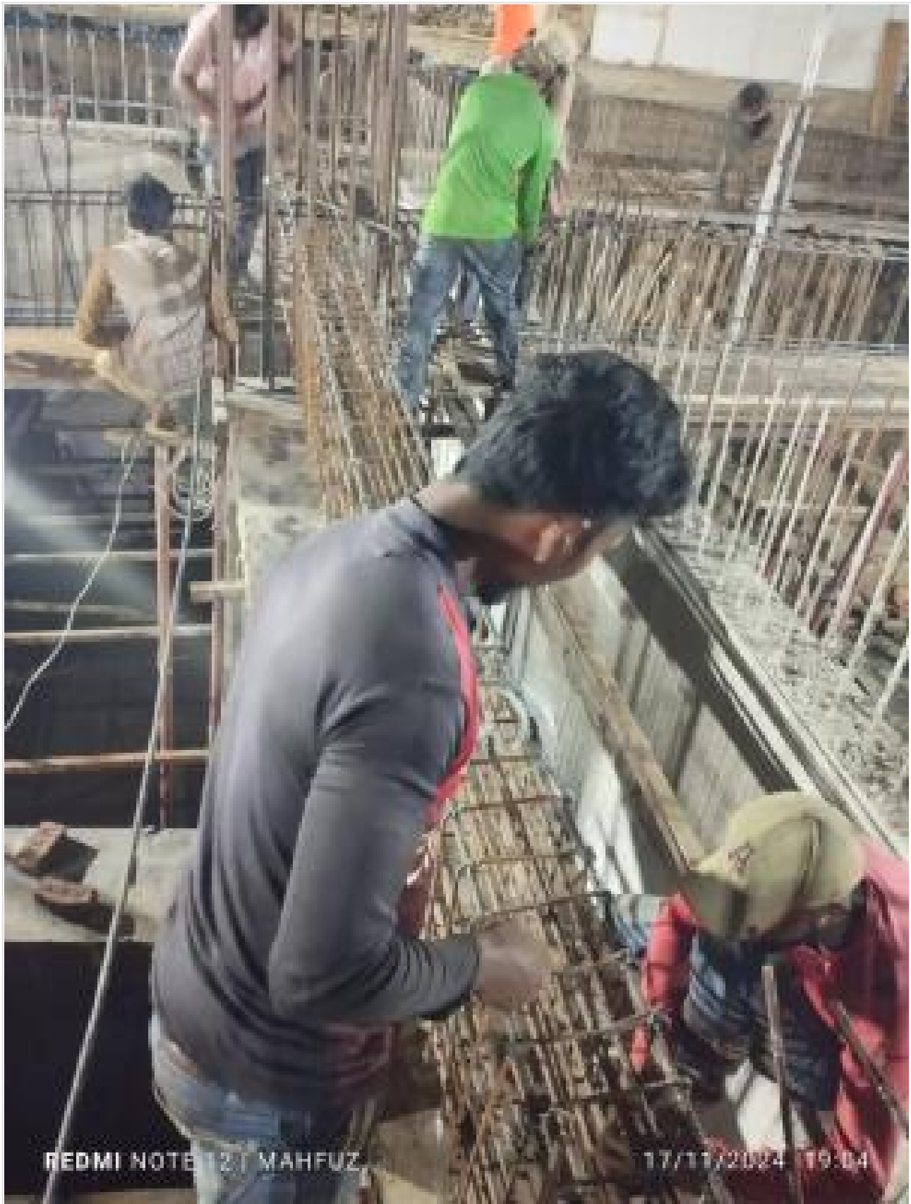
Foundation beam rebar work on 17-11-24
