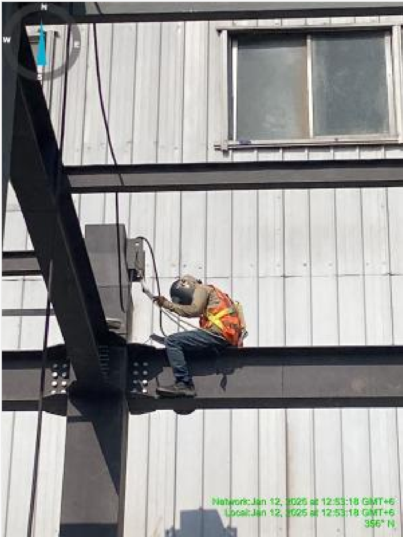
Welding steel structure on 12-01-25
