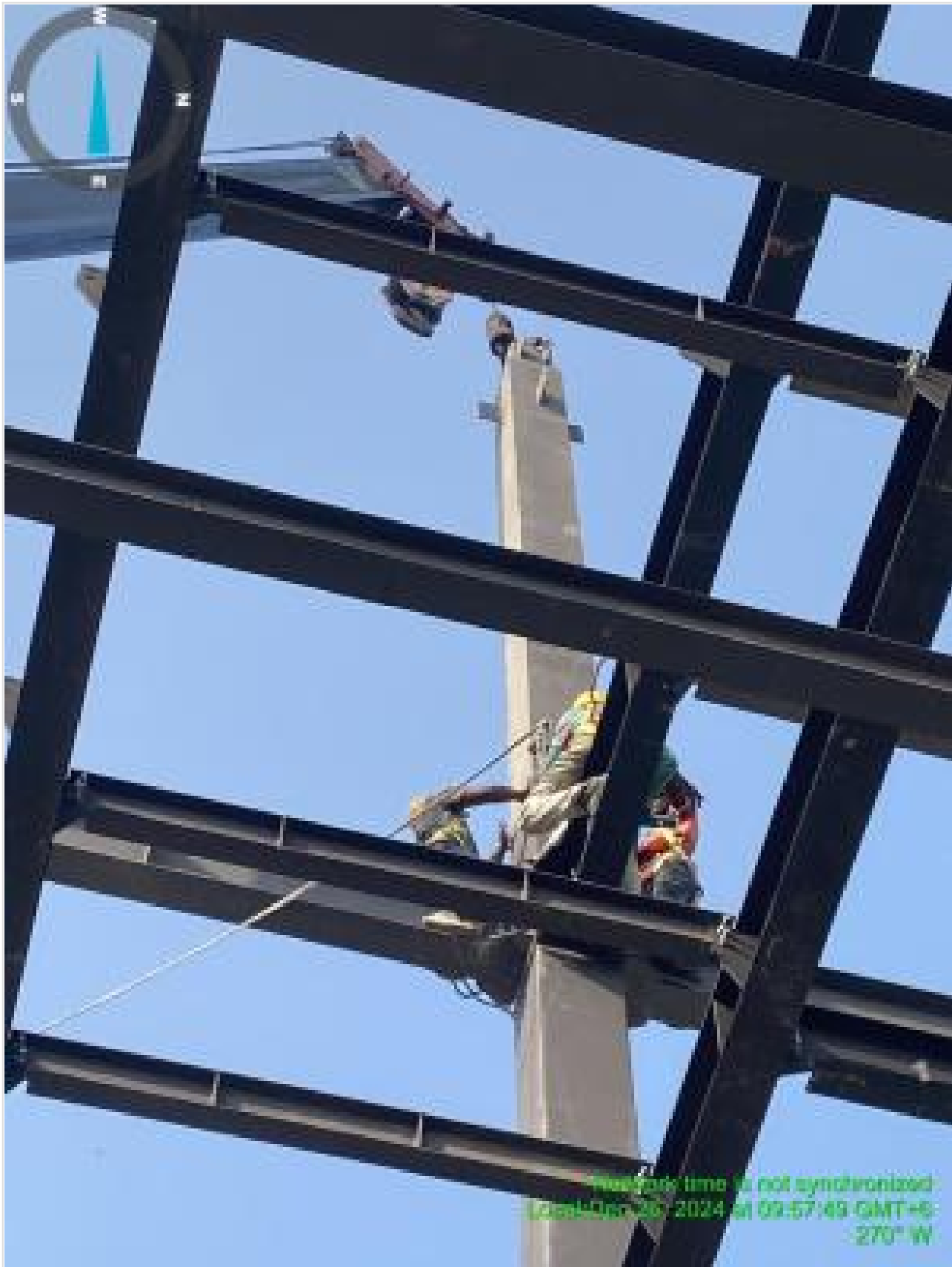
Steel structure erection at 4th floor on 26-12-24
