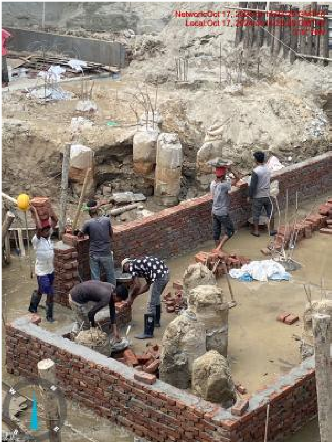
Water tank base brick wall shuttering on 17-10-24
