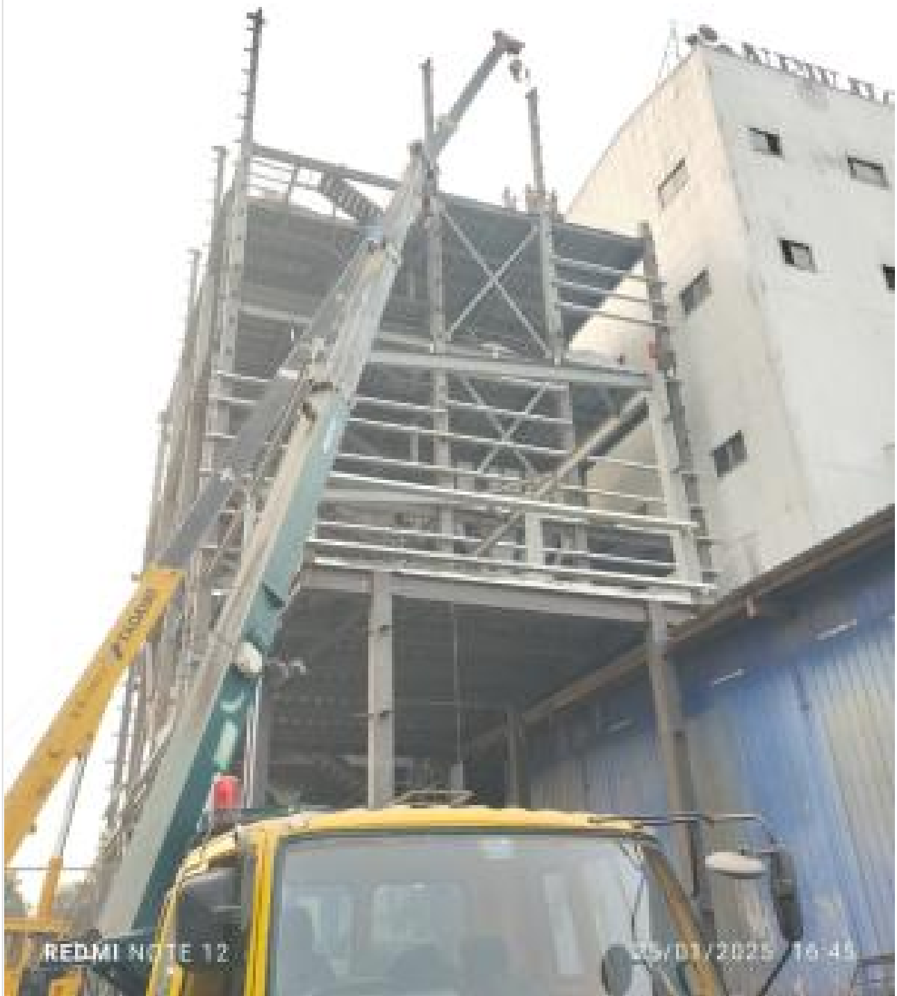
5th floor column installation on 25-01-25
