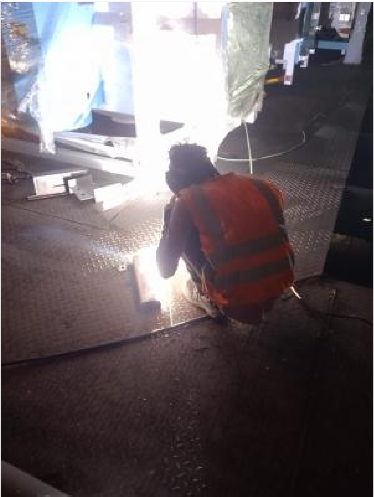
Checked plate welding on 18-01-25
