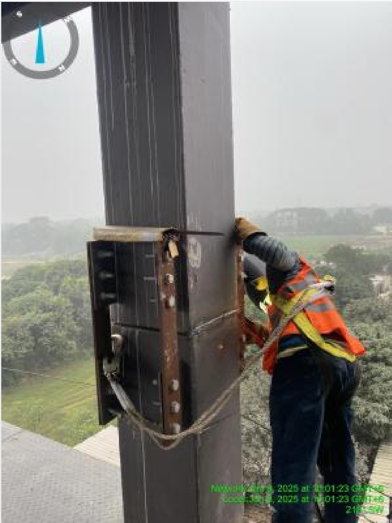
Column Joint working on 08-01-25
