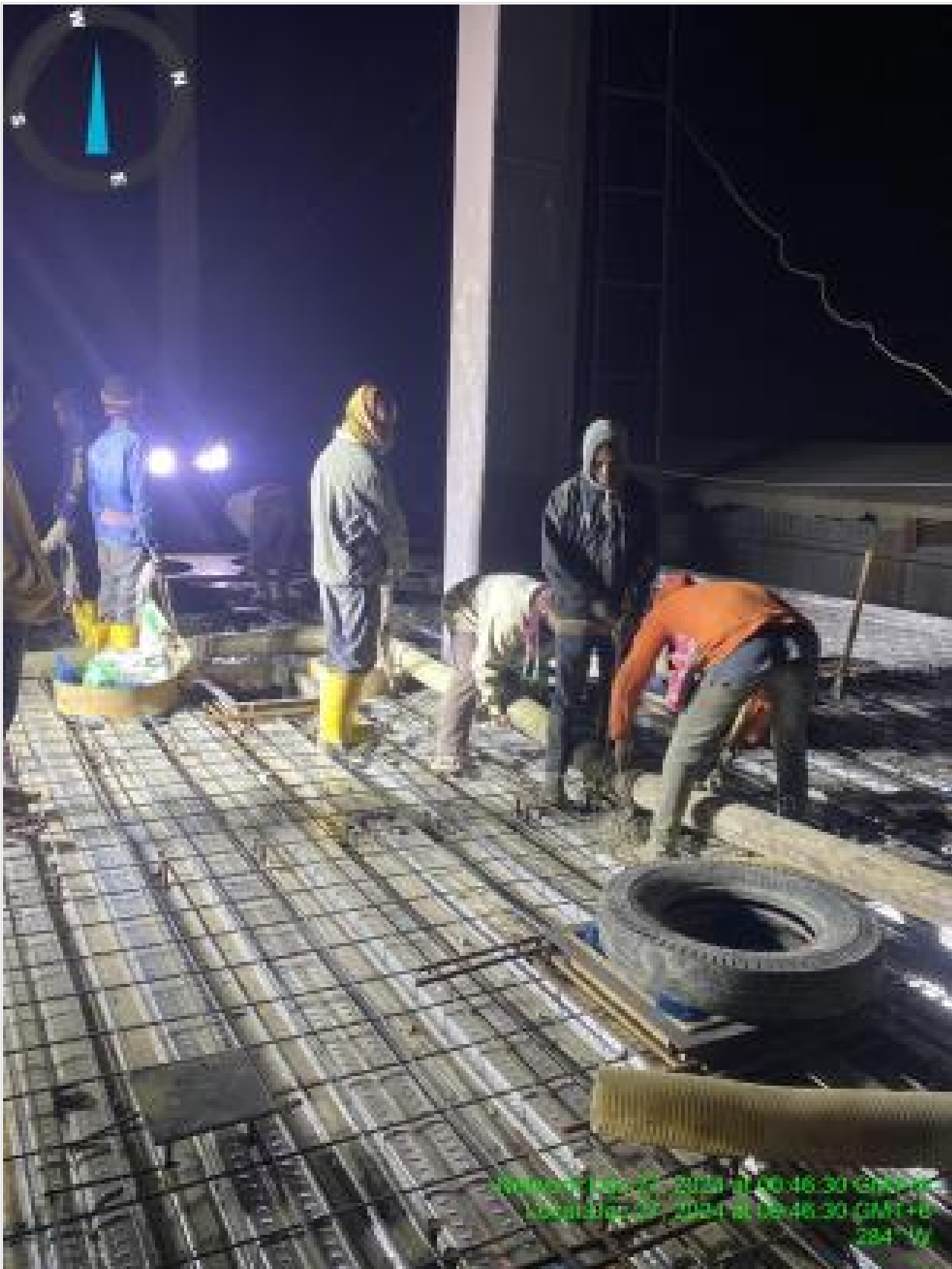
Concreting on Decking slab 7 on 26-12-24
