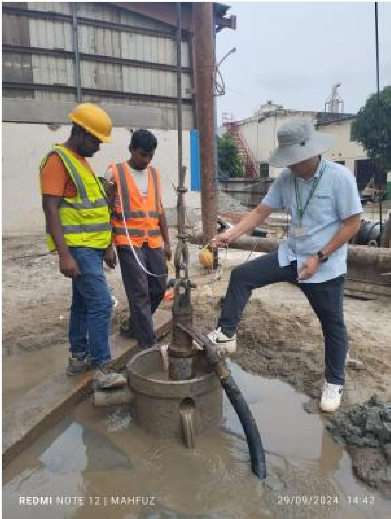
Pile no.47 boring length checking on 29-09-24
