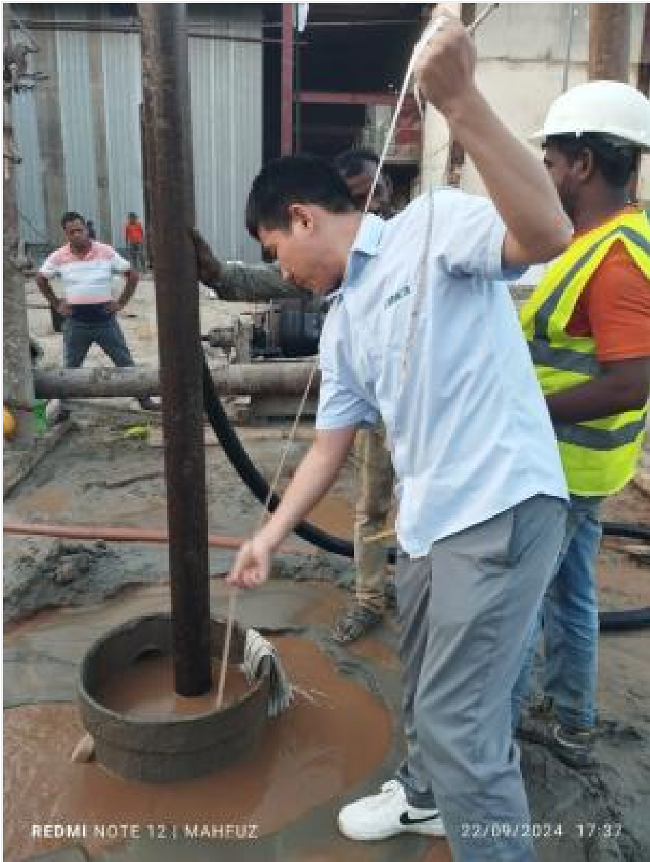
Pile boring length checking on 22-09-24
