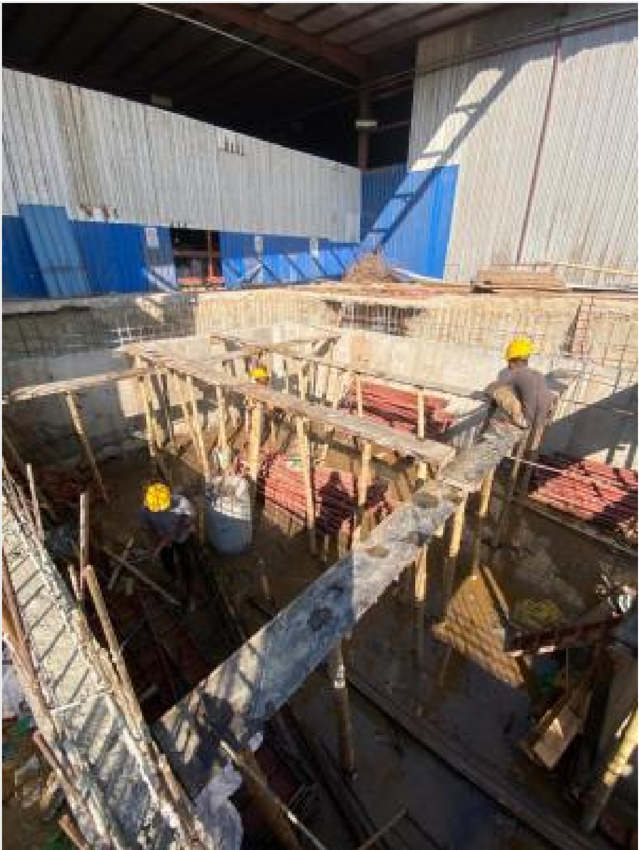
Tank slab shuttering on 20-11-24
