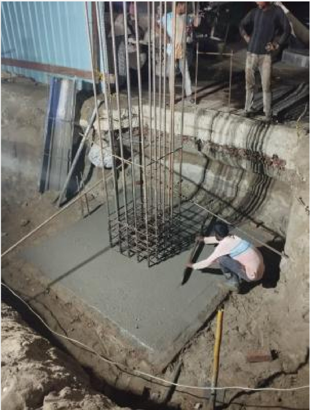
Pile cap concreting on 21-10-24
