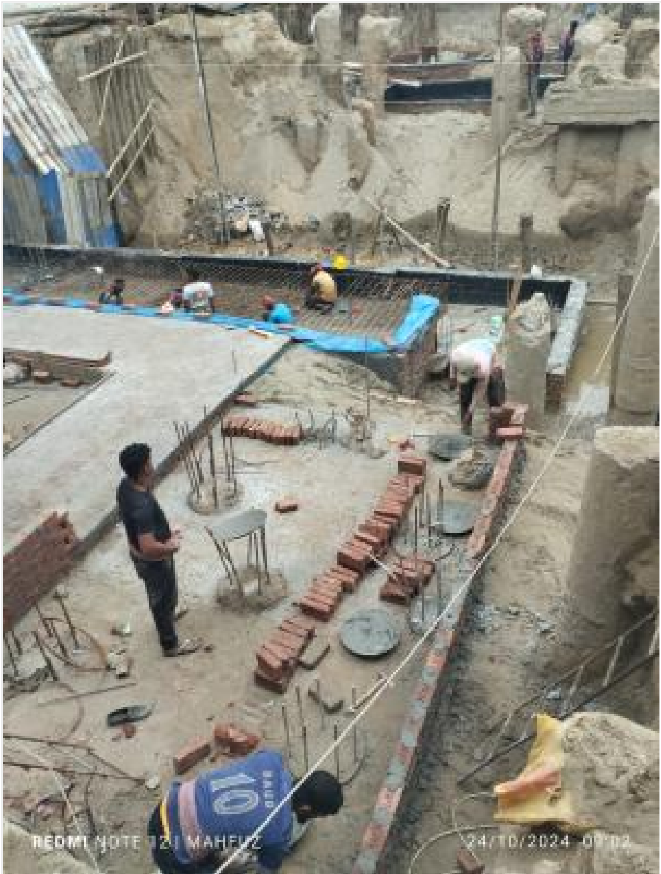
Tank base brick wall shuttering on 24-10-24
