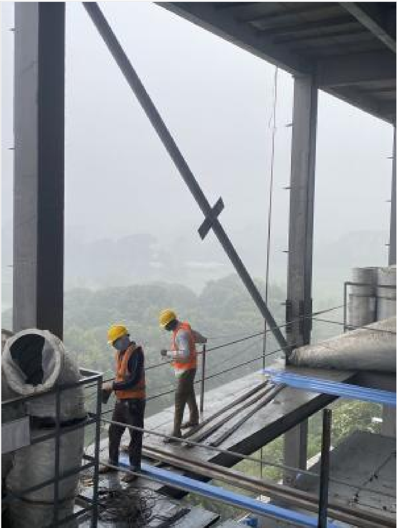
Steel bracing fixing on 24-01-25
