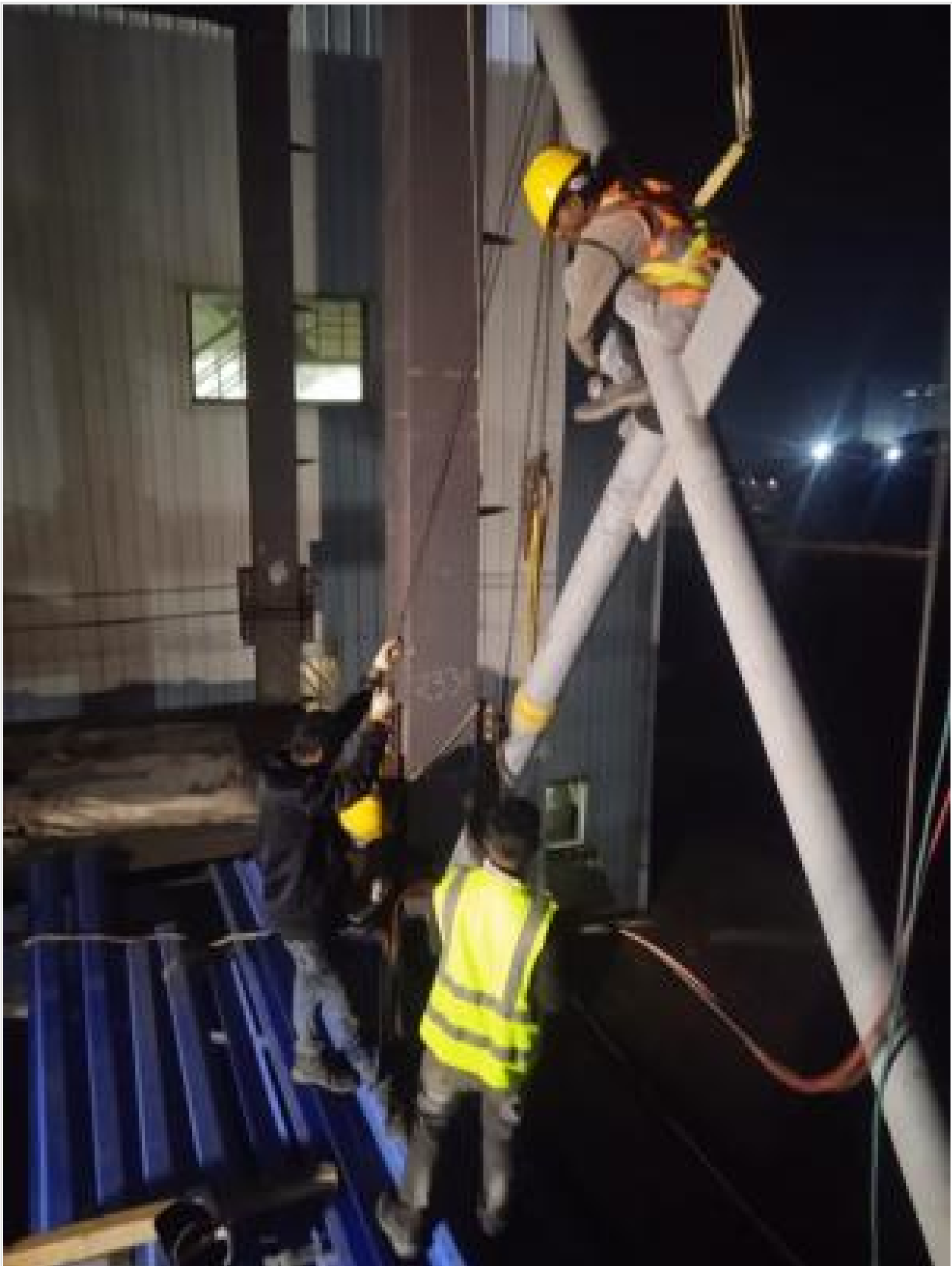
Steel bracing installation on 13-01-25
