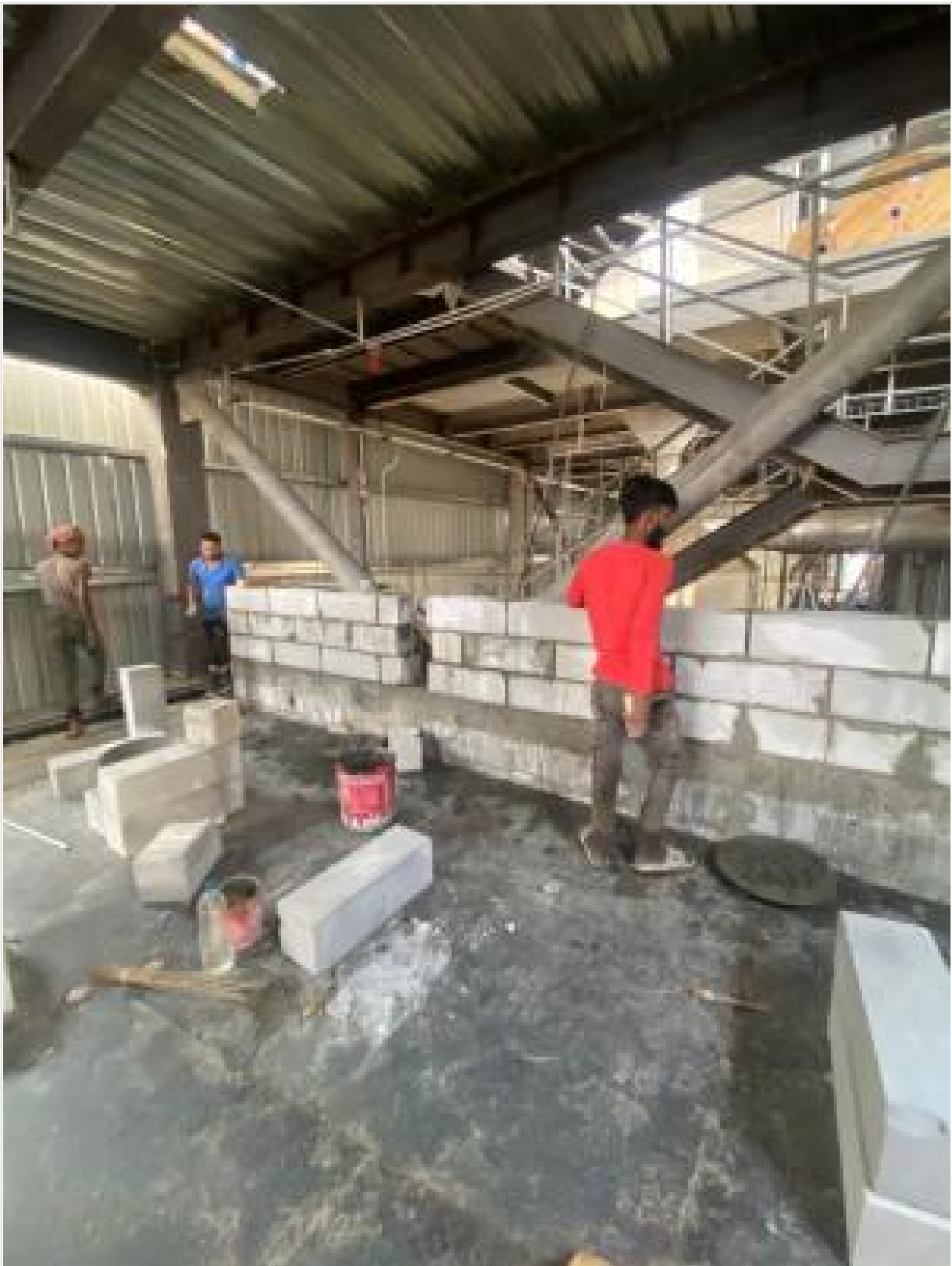
Interior AAC block work on 10-03-25
