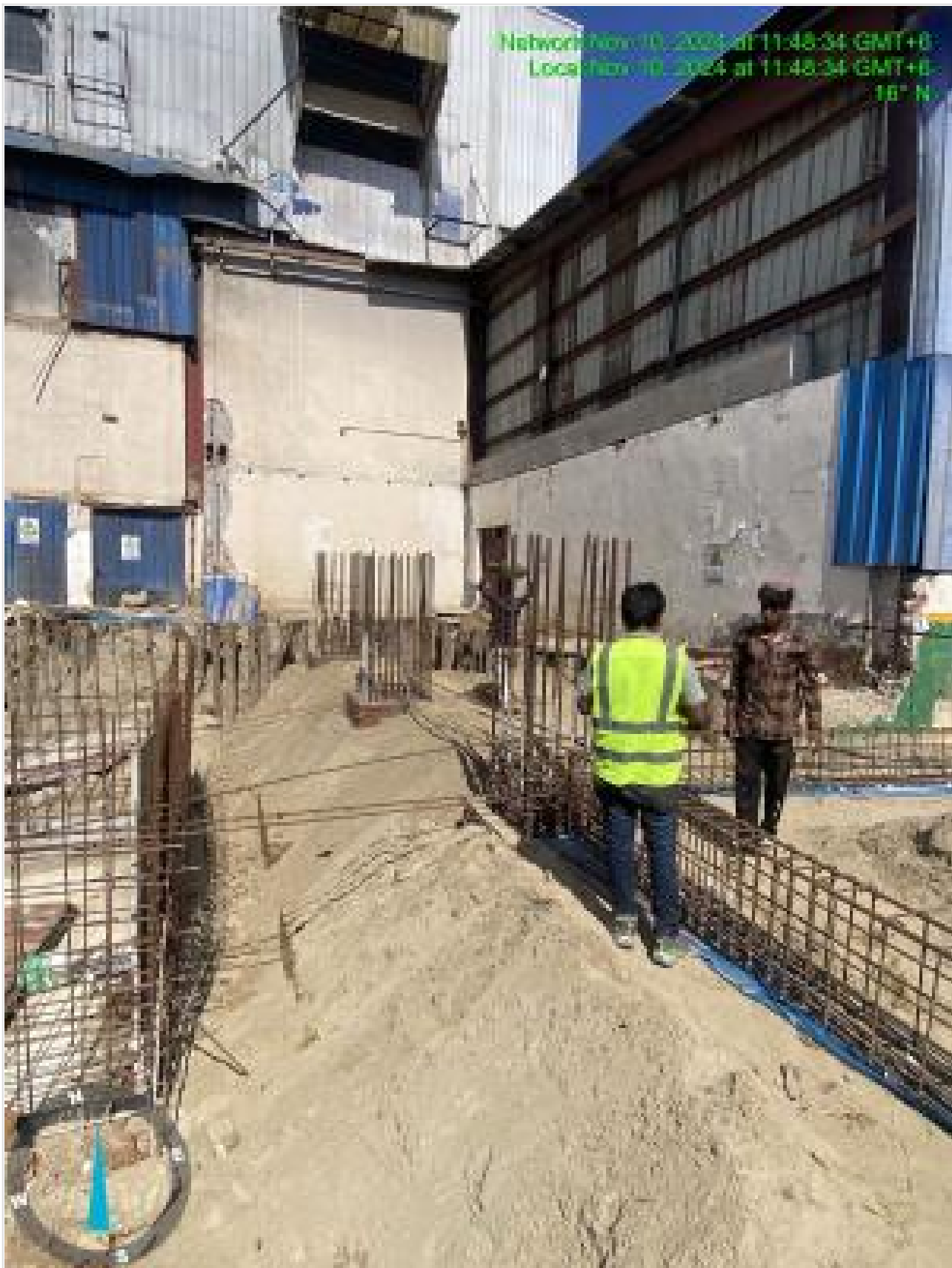
Foundation beam rebar work on 10-11-24
