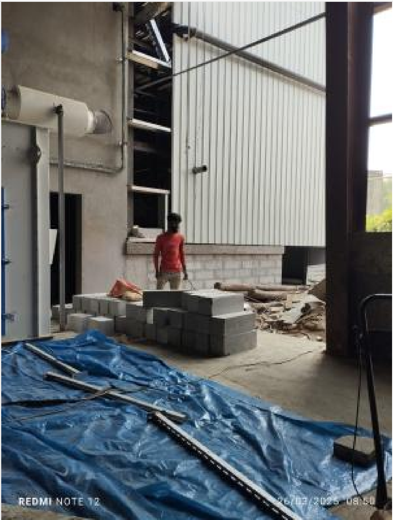
Interior AAC block work on 26-03-25
