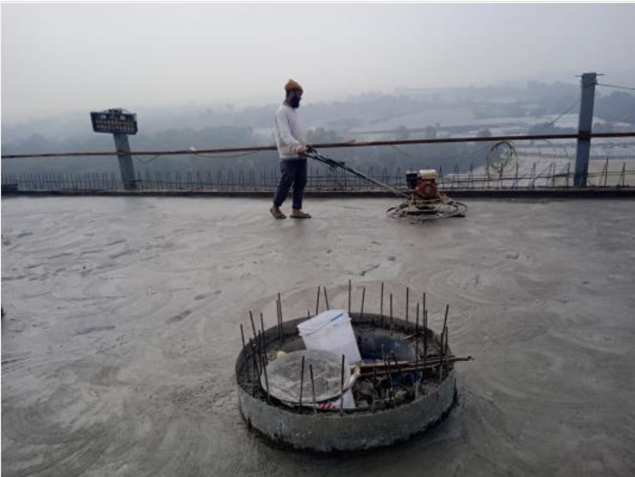
5th Floor roof slab power trowel finishing on 11-02-25
