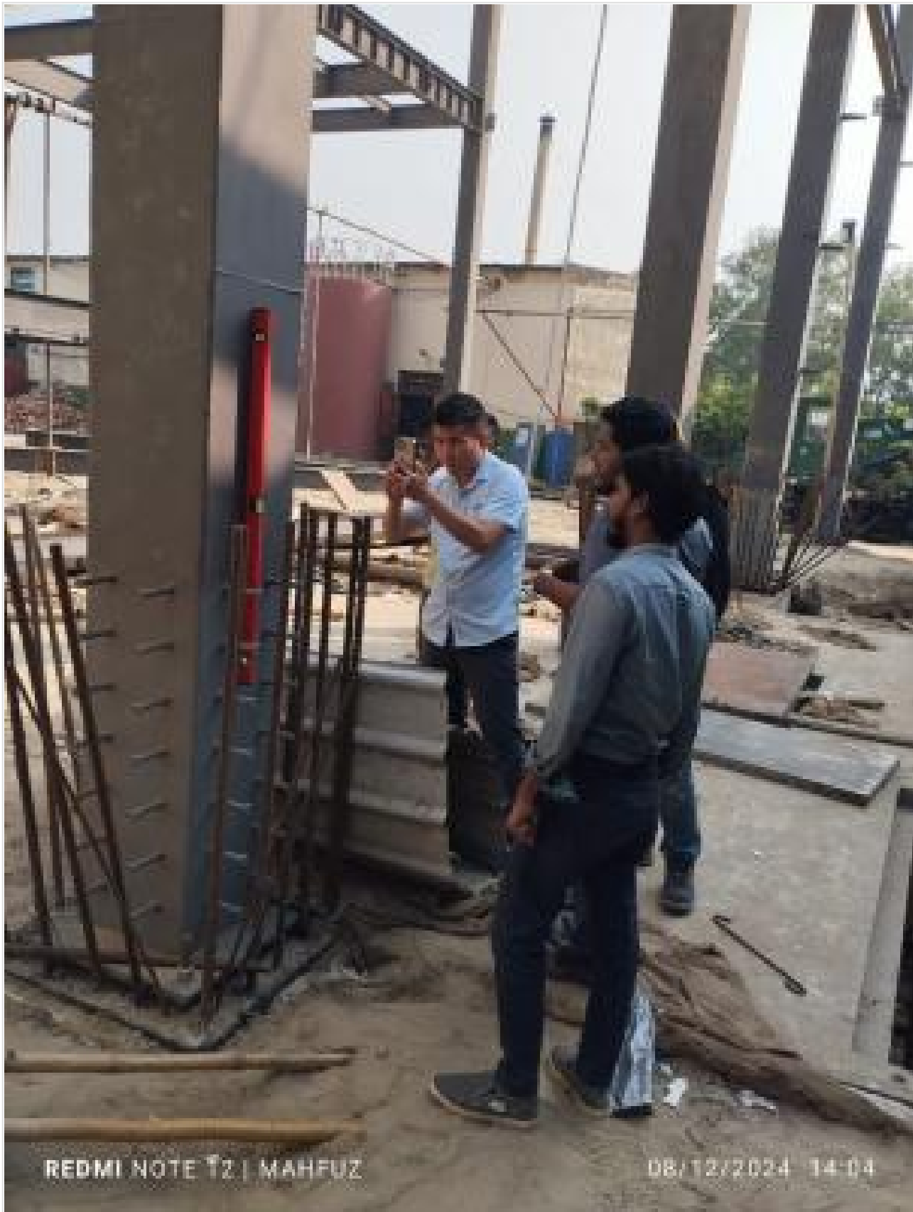
Steel column vertical alignment checking on 08-12-24
