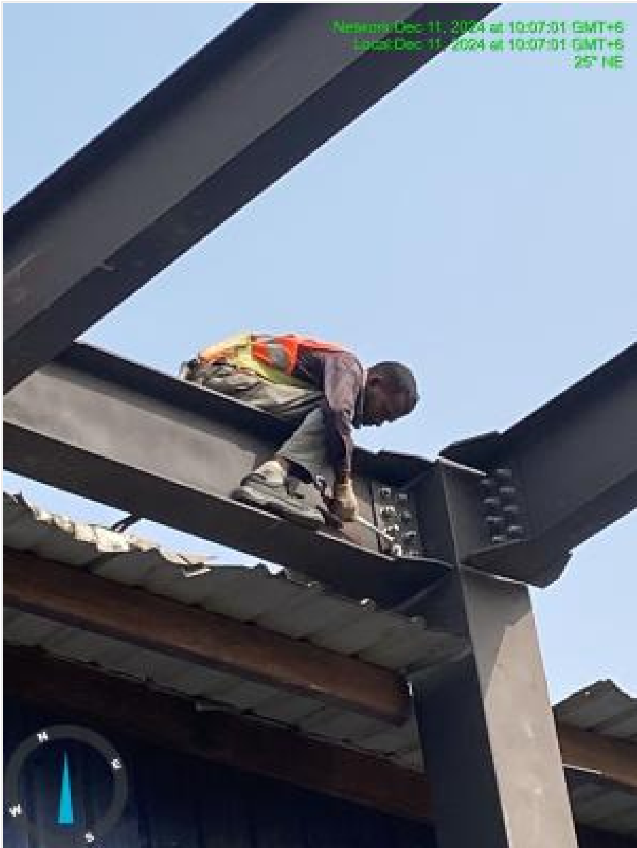
Nut tightening on 11-12-24
