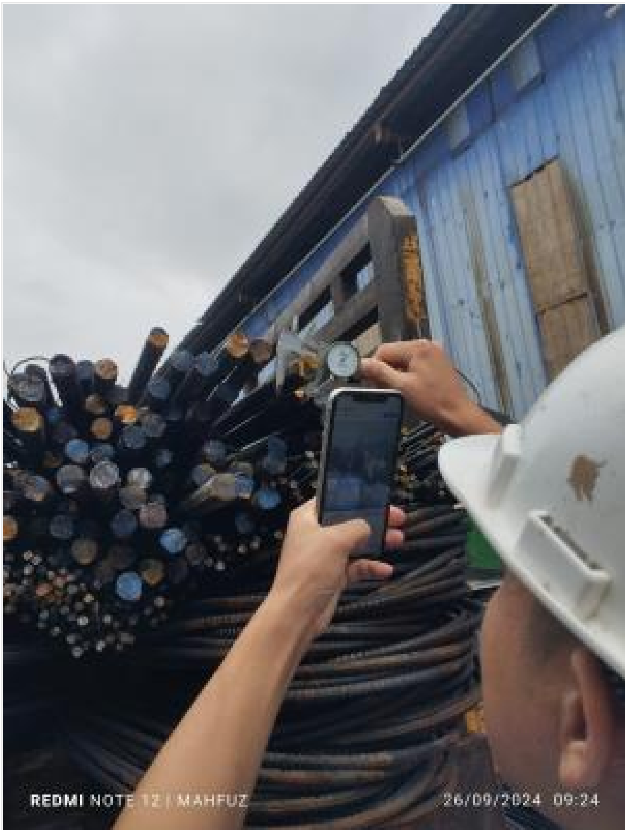
Pile cap re-bar dia checking on 26-09-24
