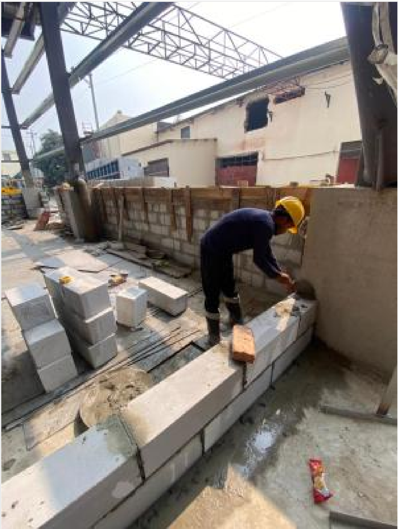
AAC block work on 19-02-25
