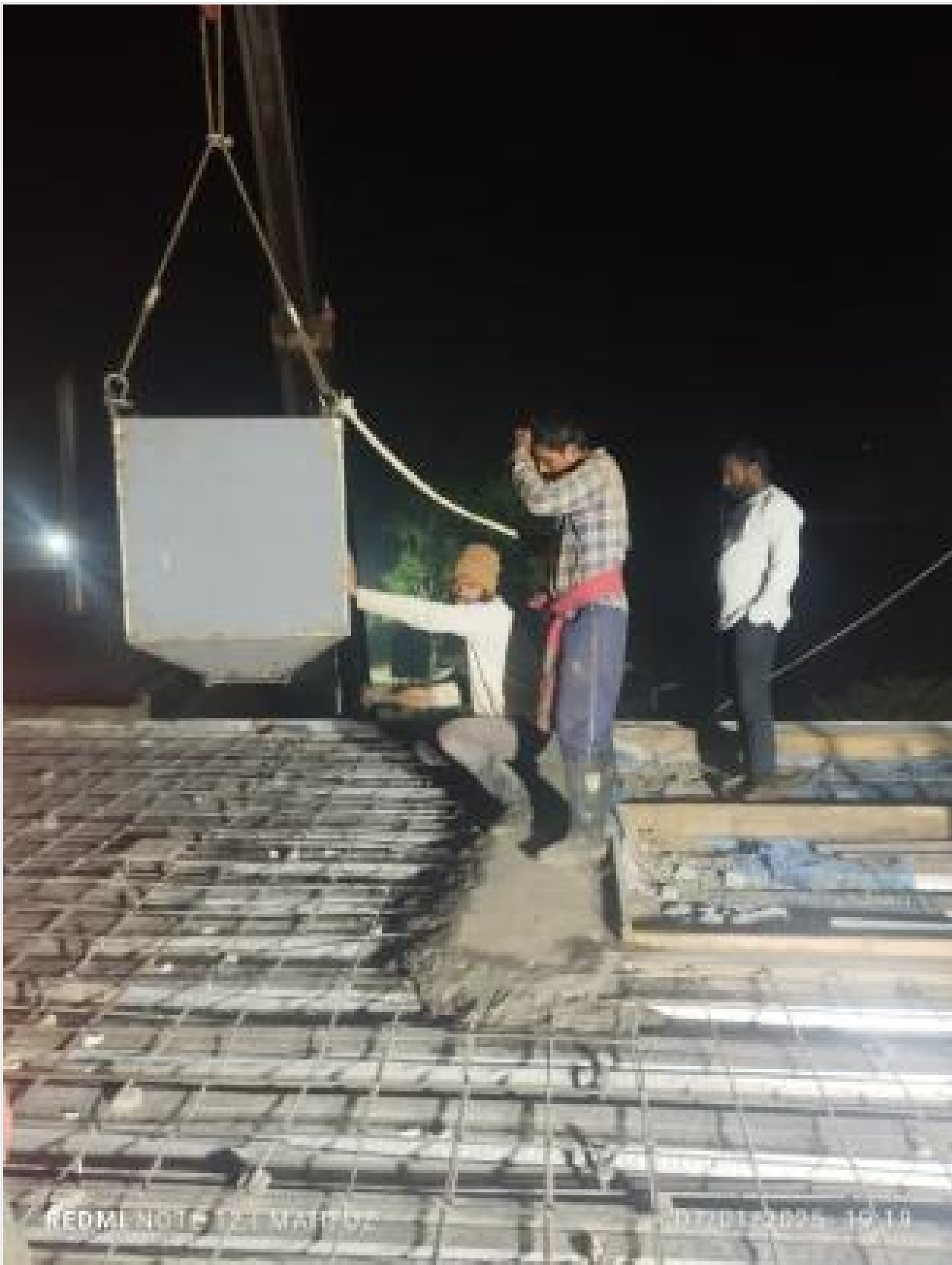
Concreting on Decking Slab-7.5m on 07-01-25
