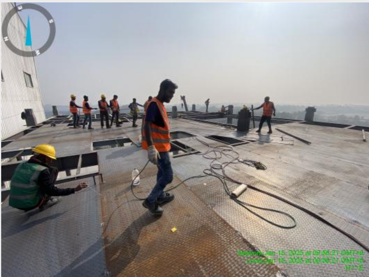
Checked plate fixing on 15-01-25
