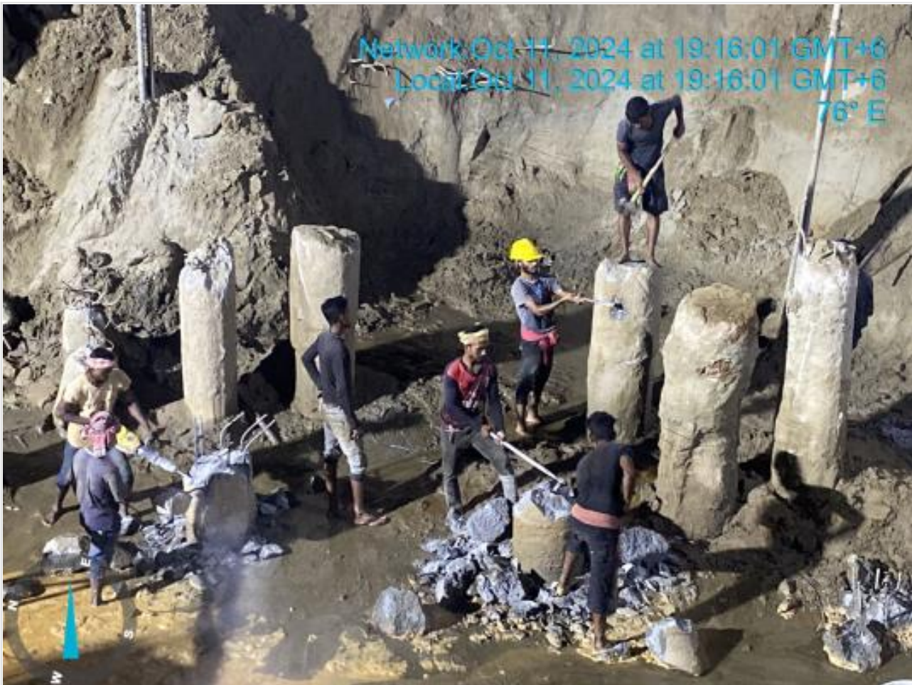
Pile head breaking on 11-10-24
