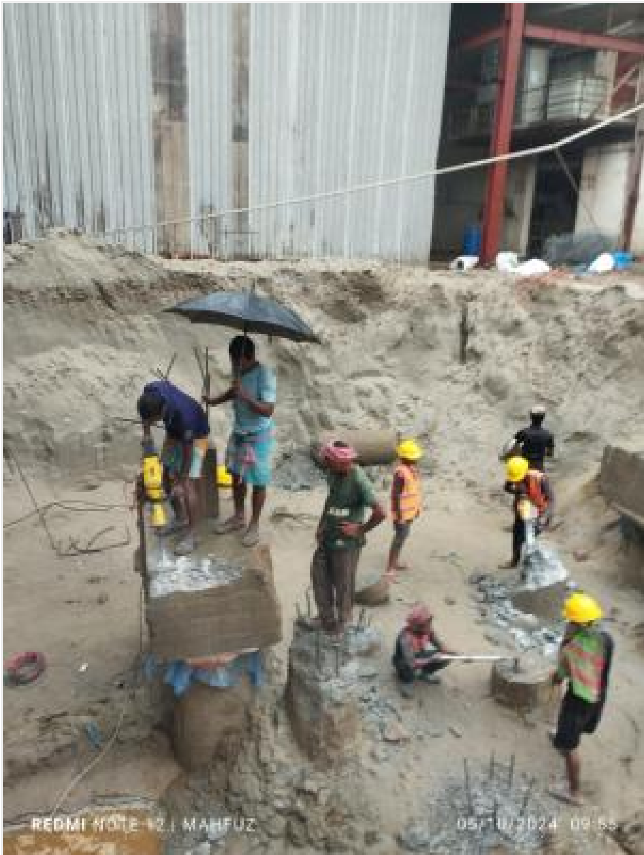
Old base breaking on 05-10-24
