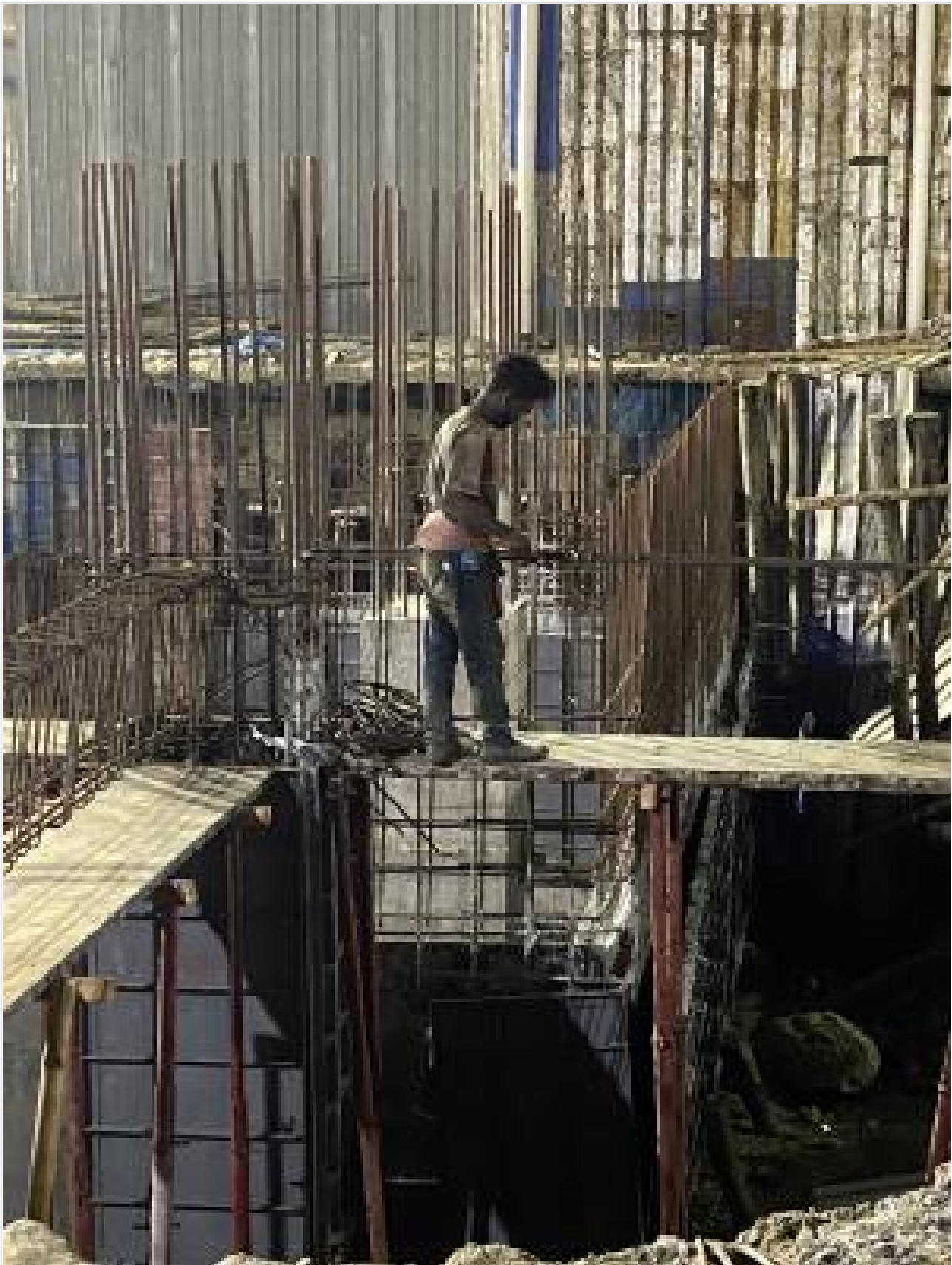
Foundation beam rebar work on 11-11-24
