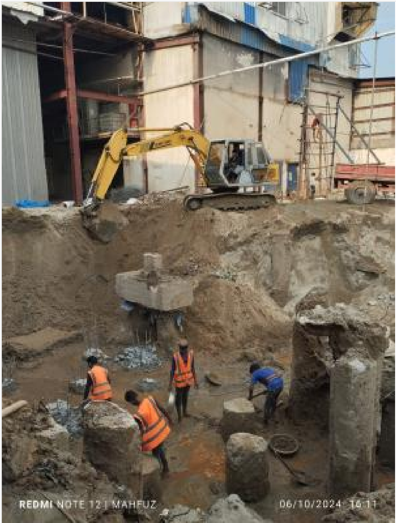
Pile head breaking on 07-10-24
