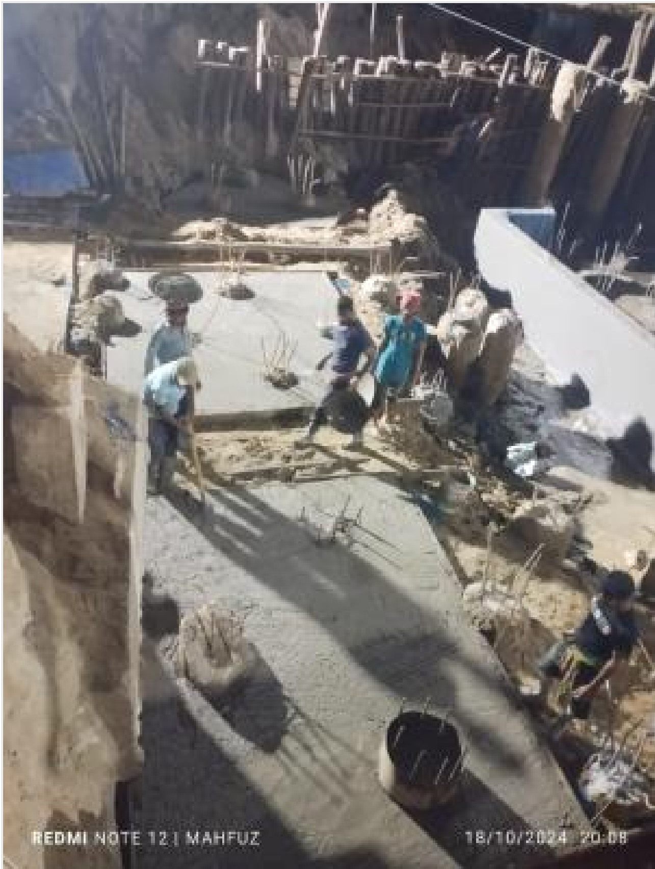
Pile cap lean concreting on 18-10-24
