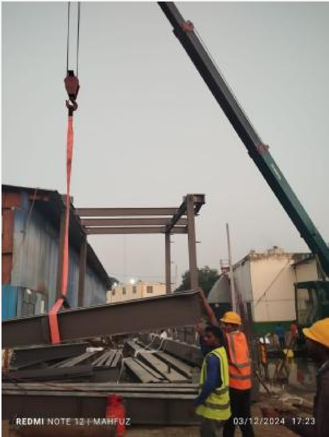
Steel member installation on 03-12-24
