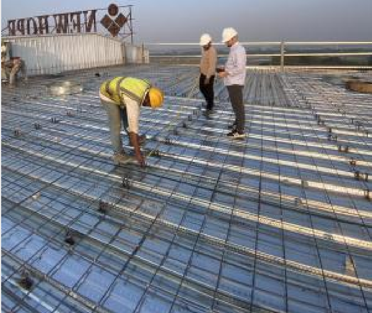
5th Floor roof slab re-bar inspection on 09-02-25
