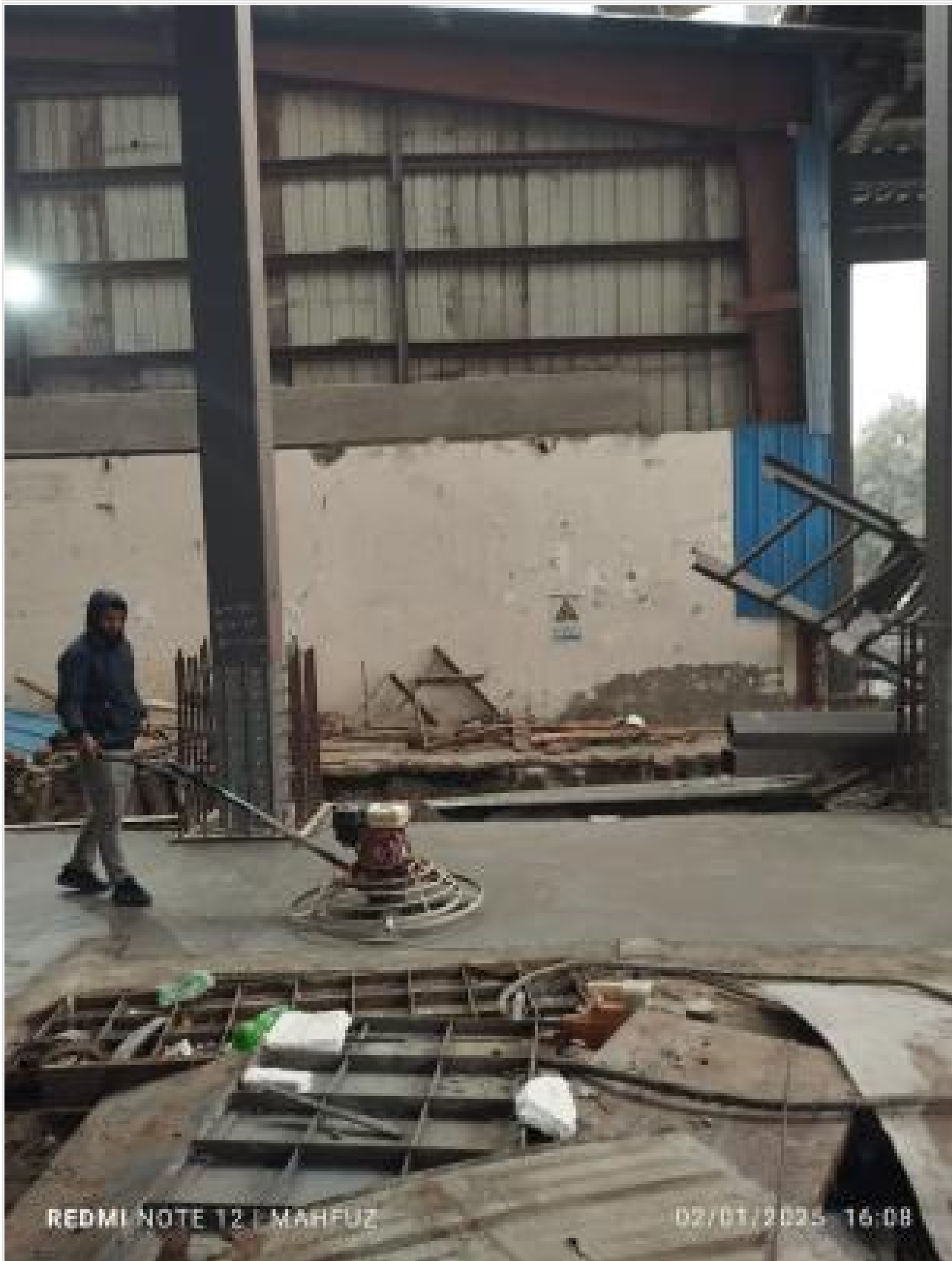
Ground Floor Concrete Mechanical Troweli on 02-01-25
