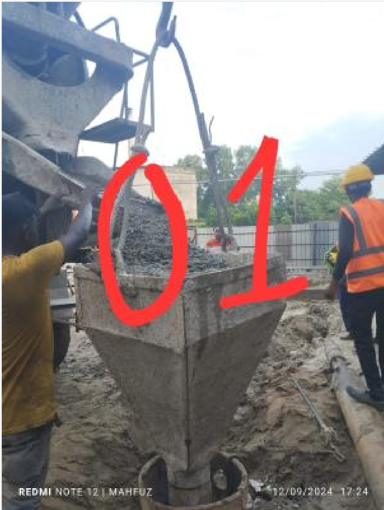
Pile concreting on 12-09-24
