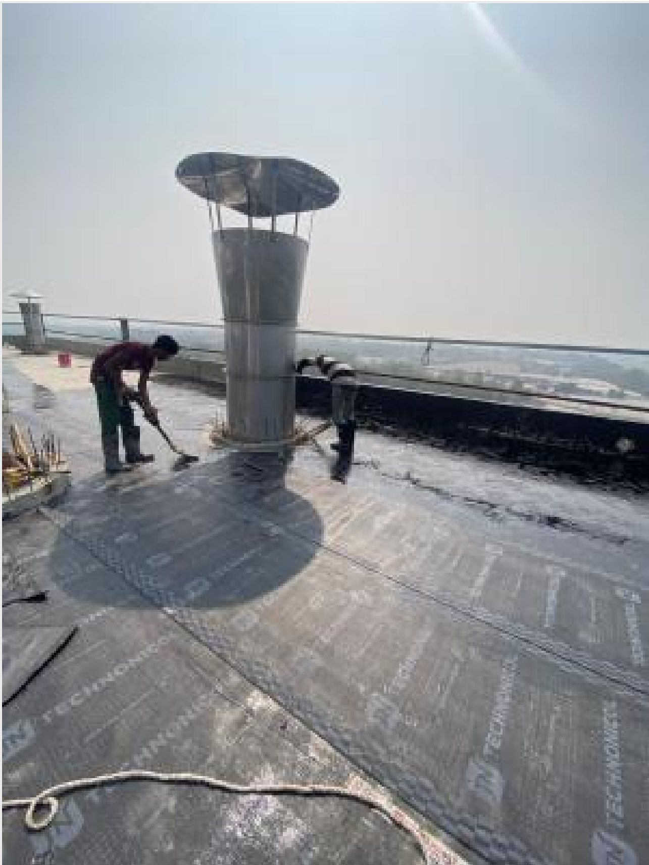
Roof top water proofing membrane laying on 01-03-25
