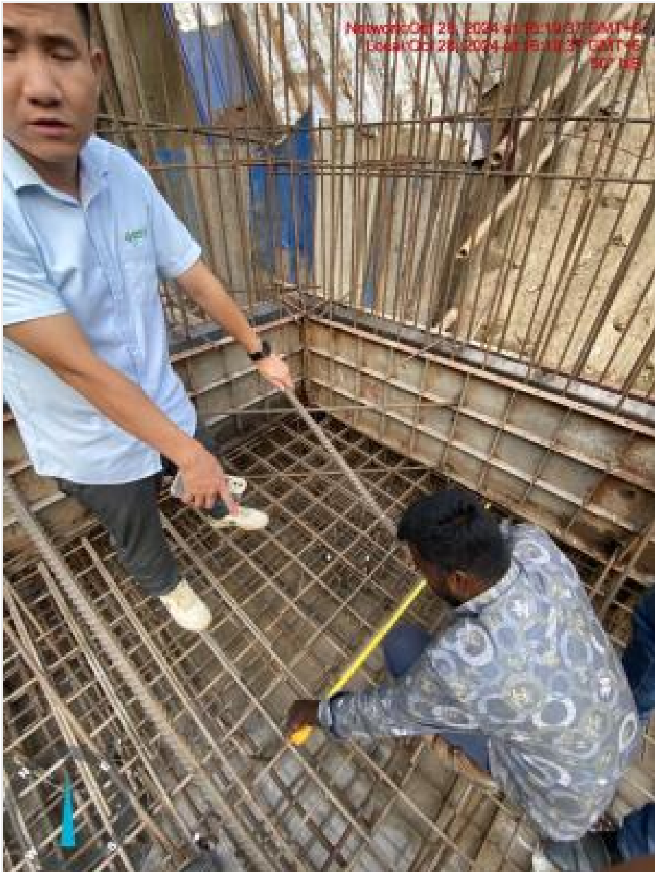
Raft re-bar inspection before concreting on 28-10-24
