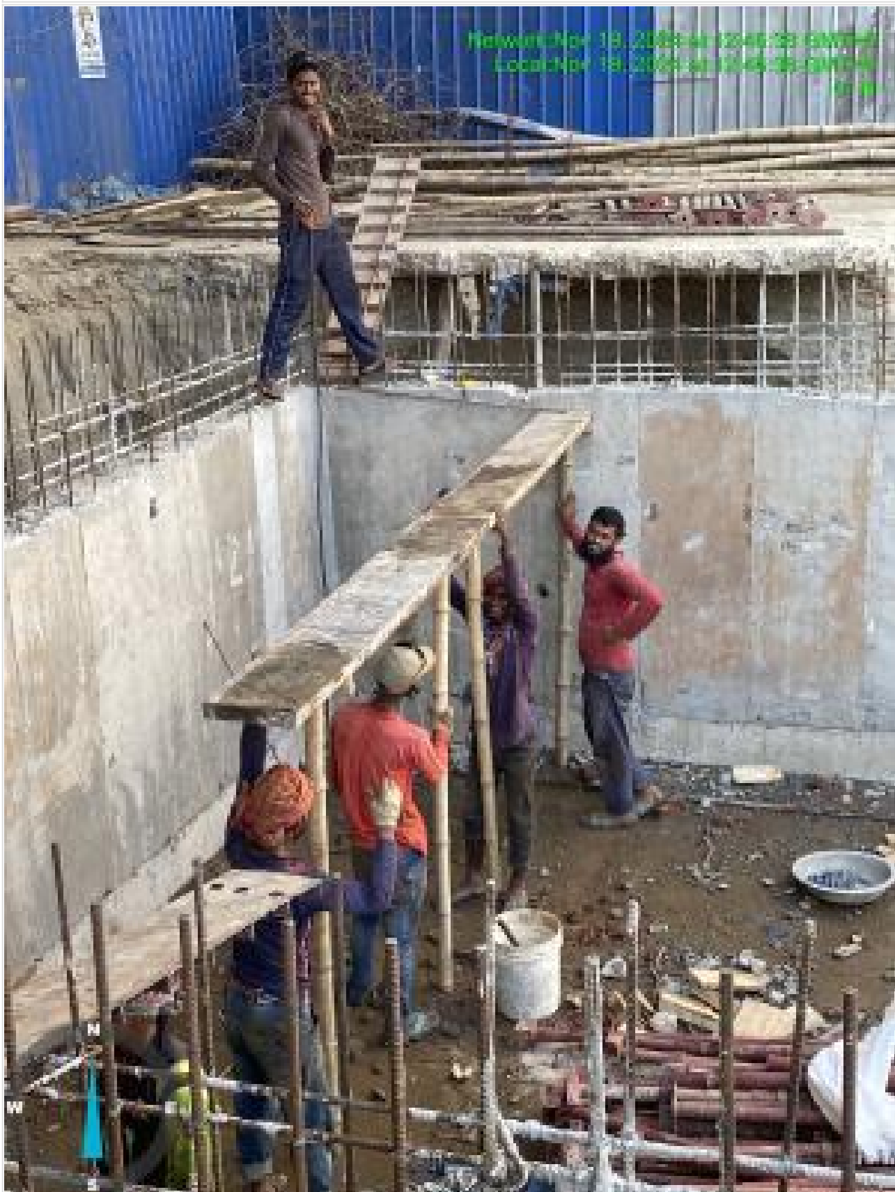
Tank slab shuttering on 19-11-24
