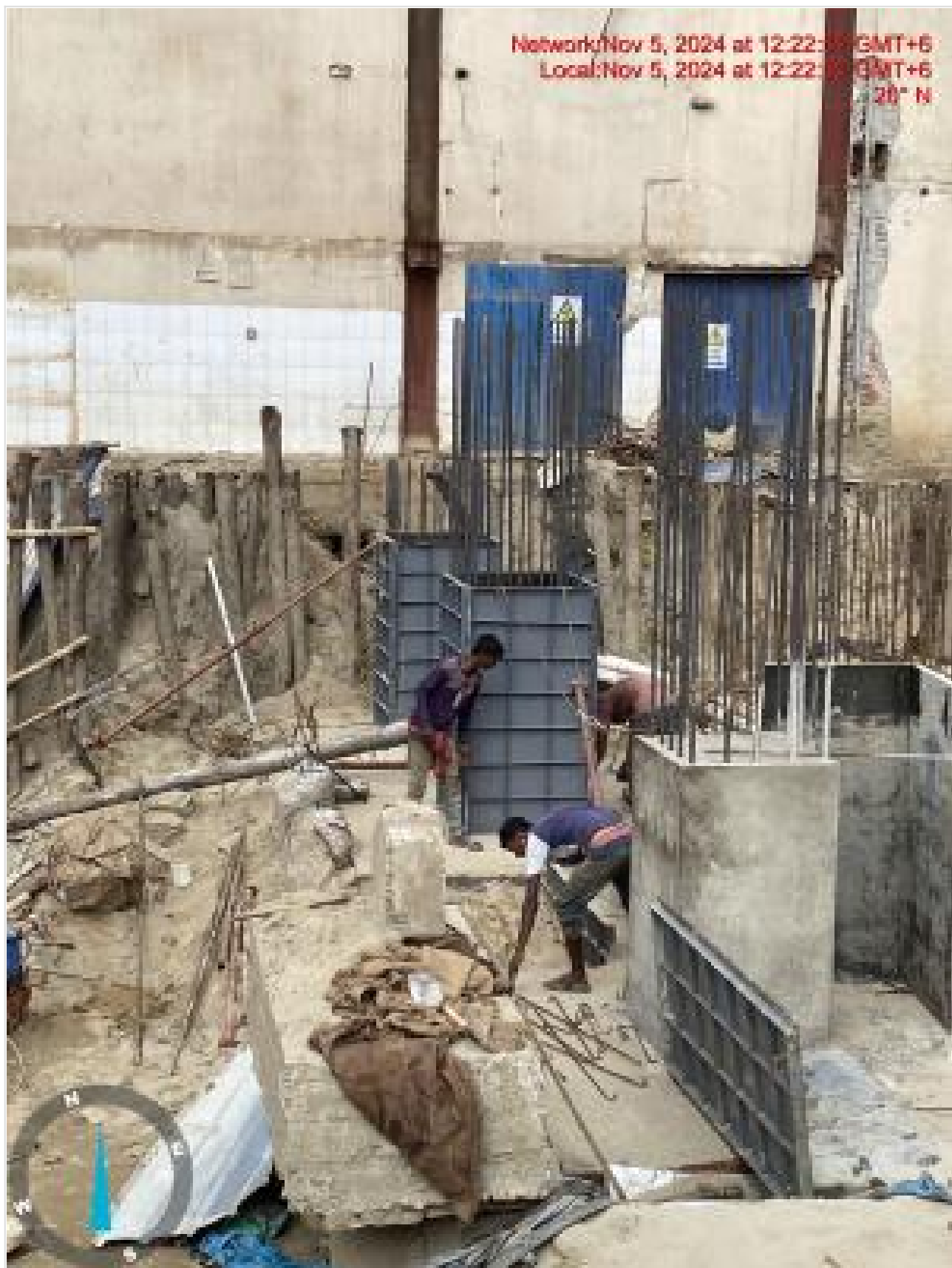
Column shuttering on 05-11-24
