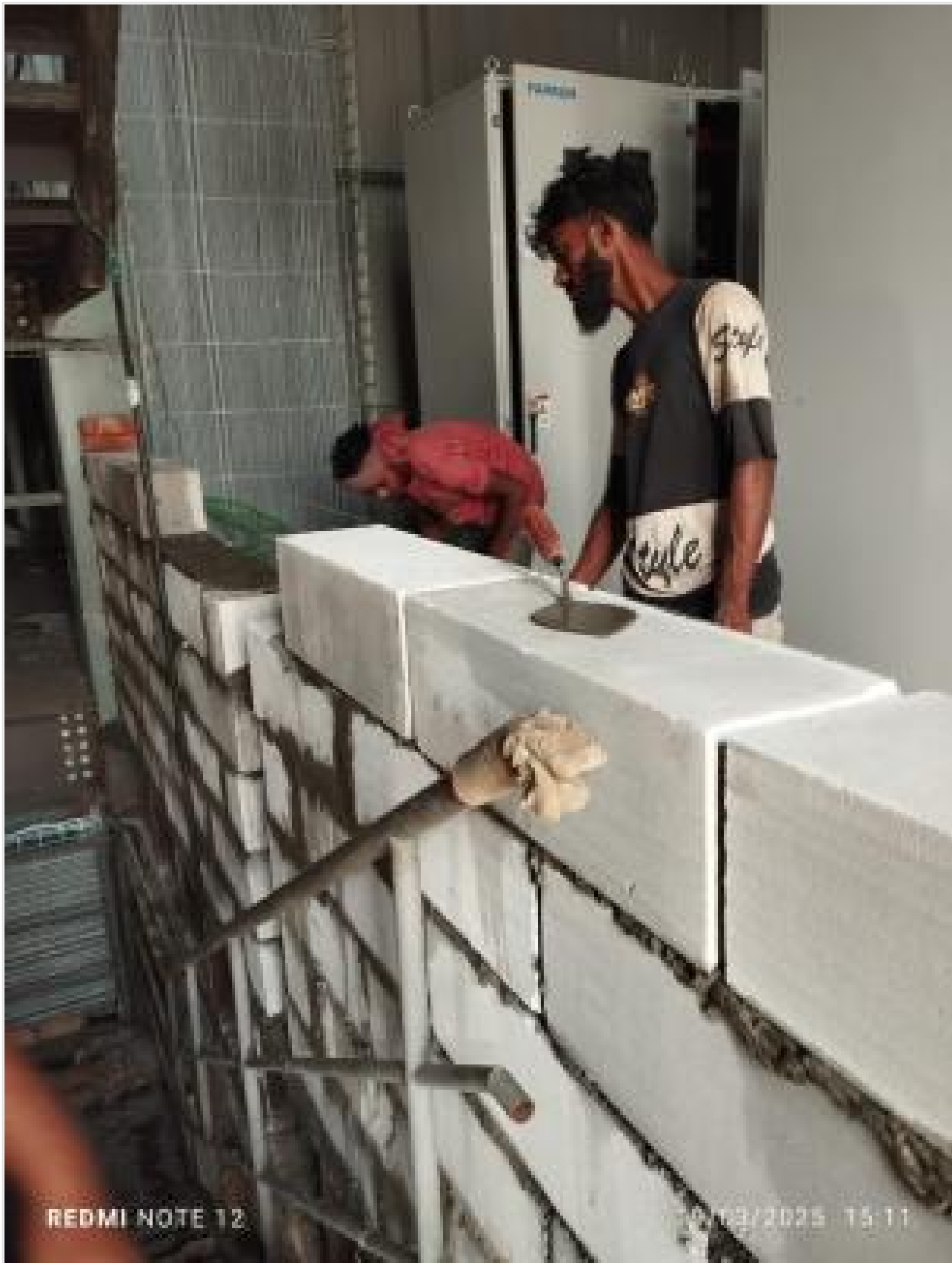
Interior AAC block work on 19-03-25
