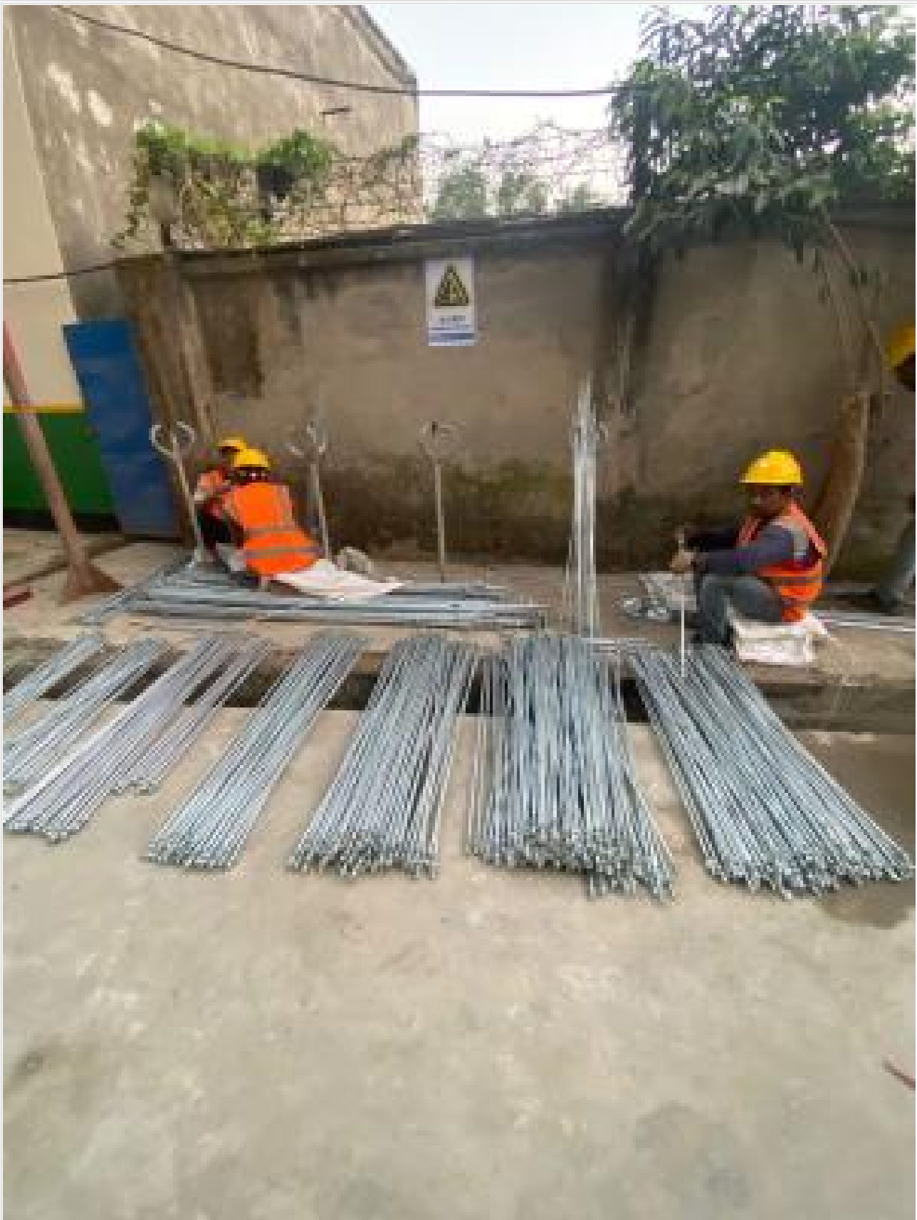
Sag Rod fixing on 17-02-25
