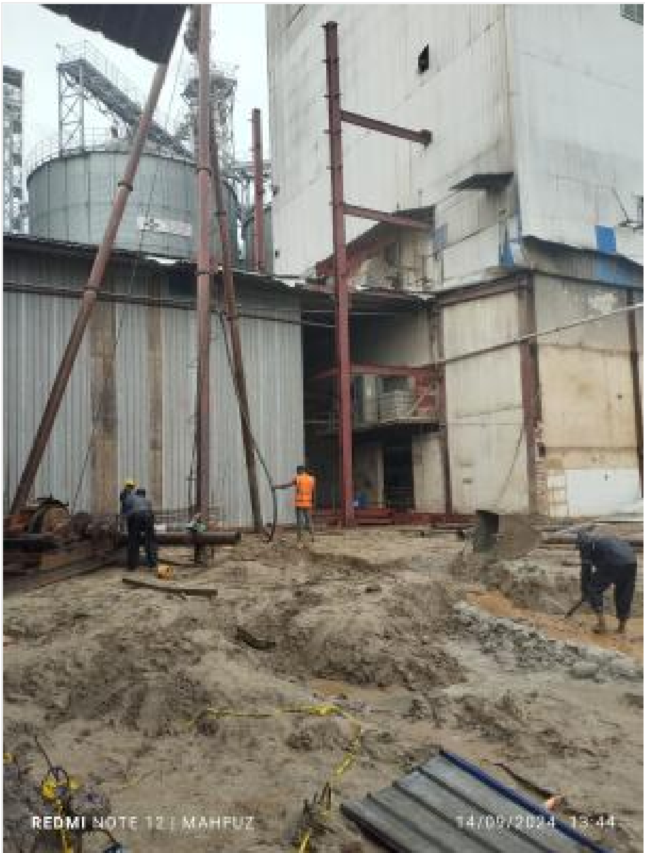
Pile boring on 14-09-24
