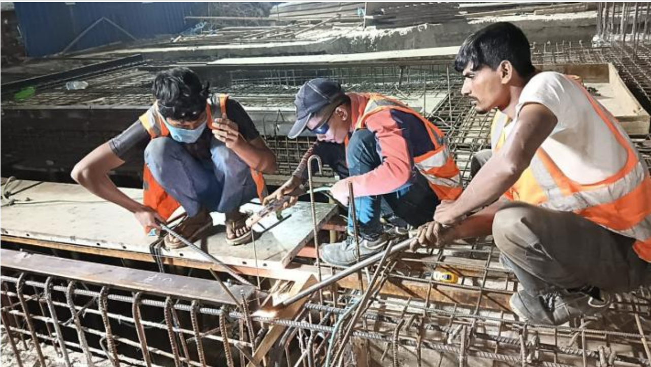
MS Angle Fixing on 24-11-24
