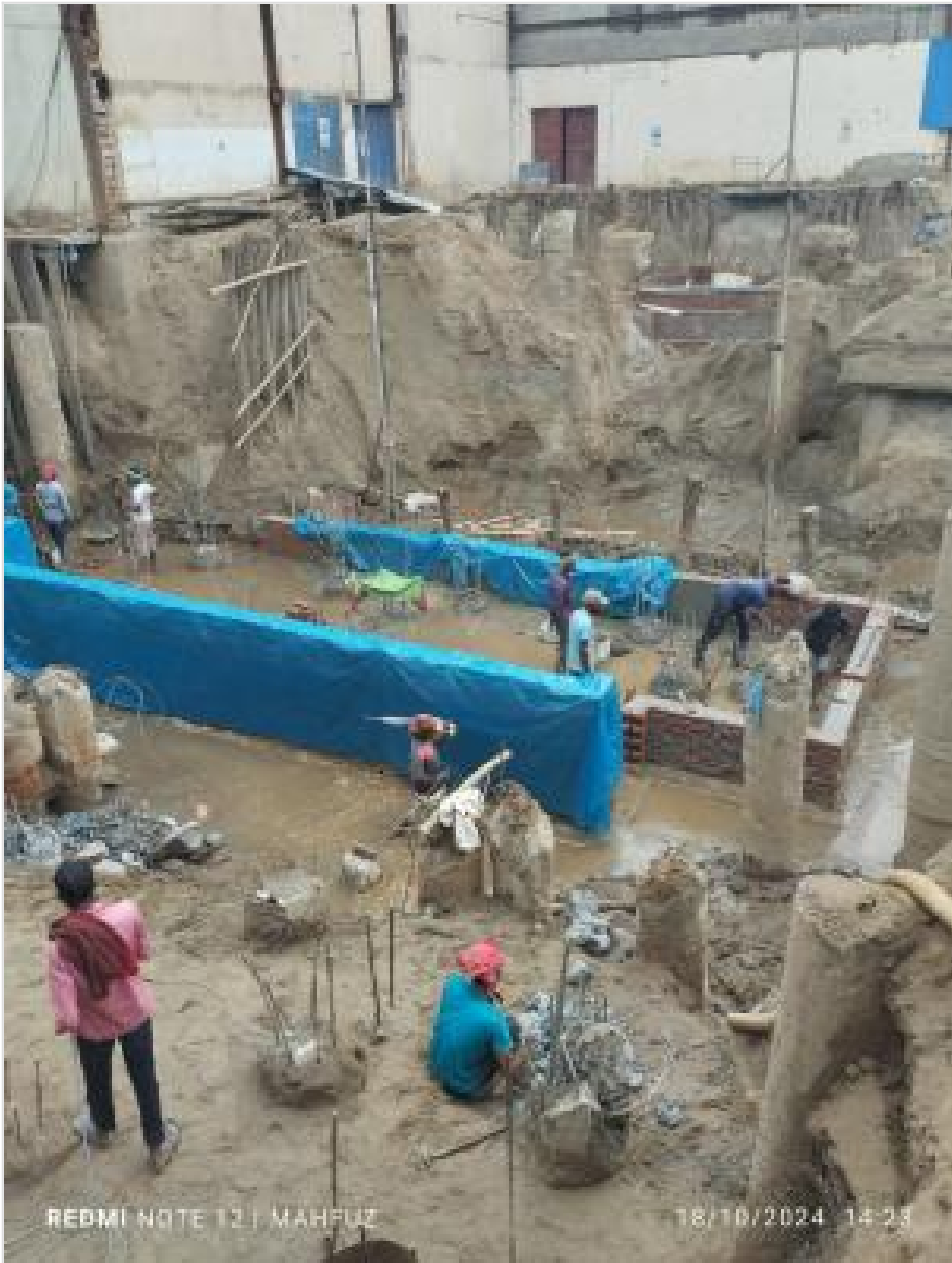
Pile head breaking on 18-10-24
