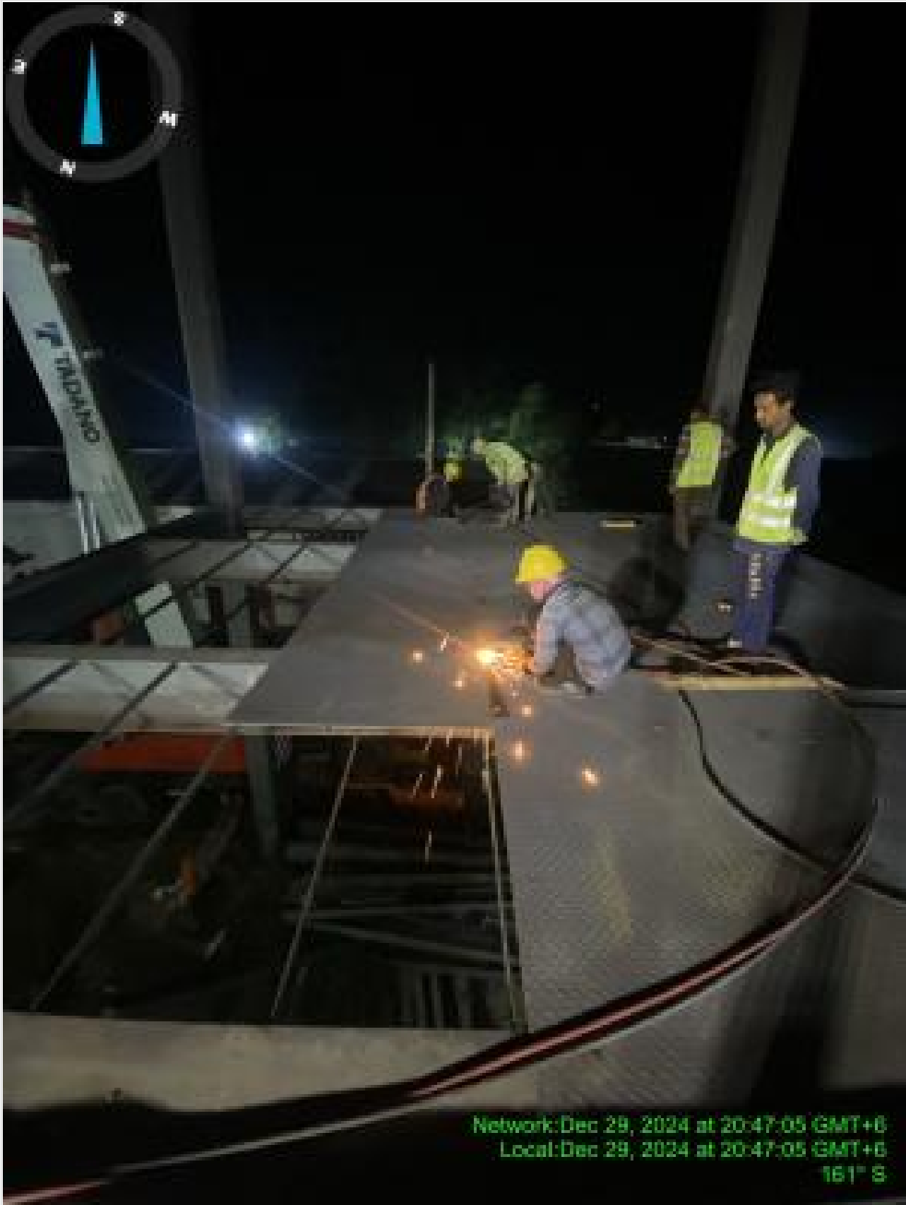
Checked plate fixing on 29-12-24
