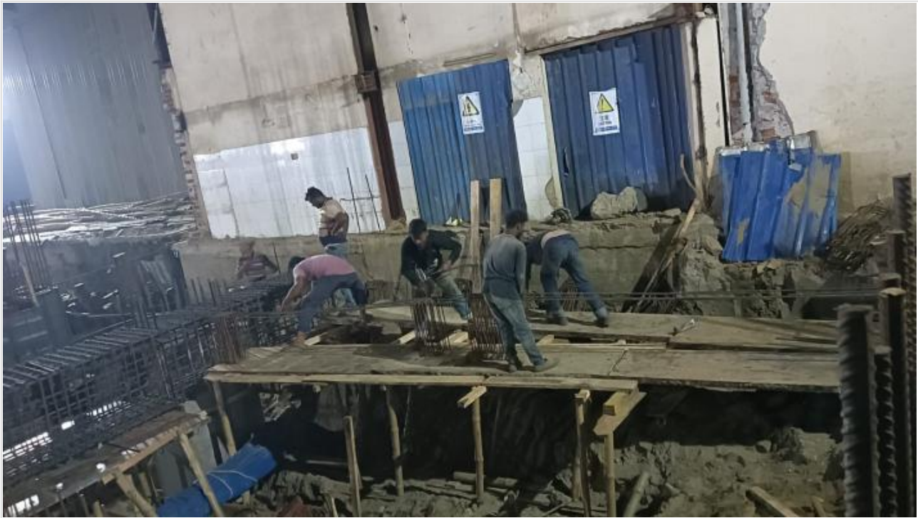
Foundation beam rebar work on 15-11-24
