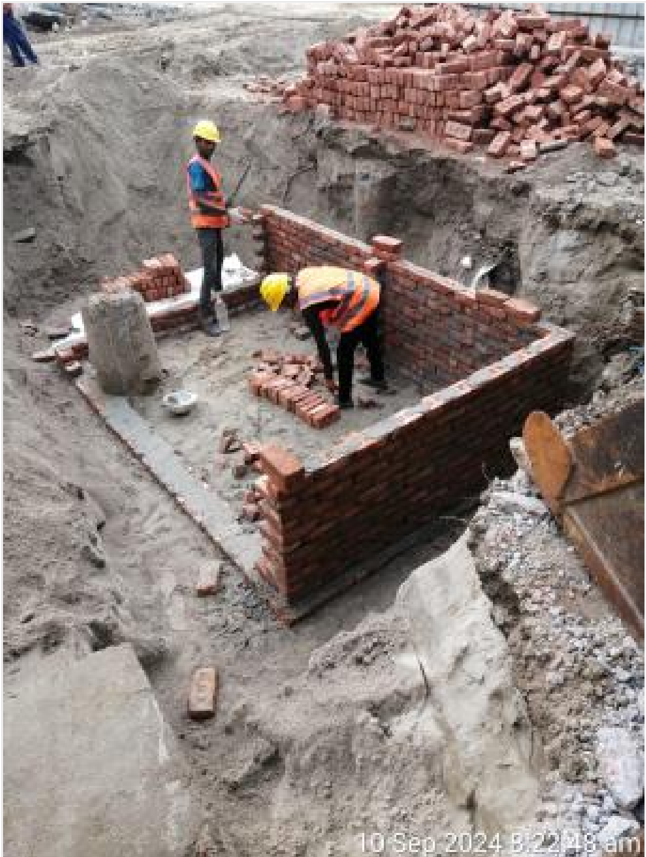
Pile mud tank brick work on 10-09-24
