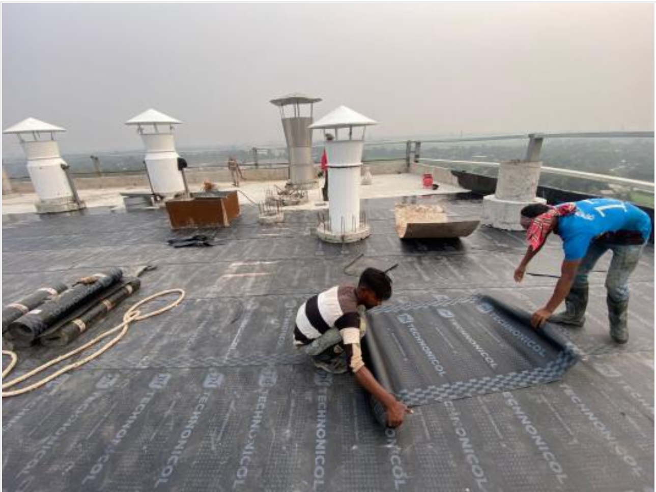
Roof top water proofing membrane laying on 28-02-25
