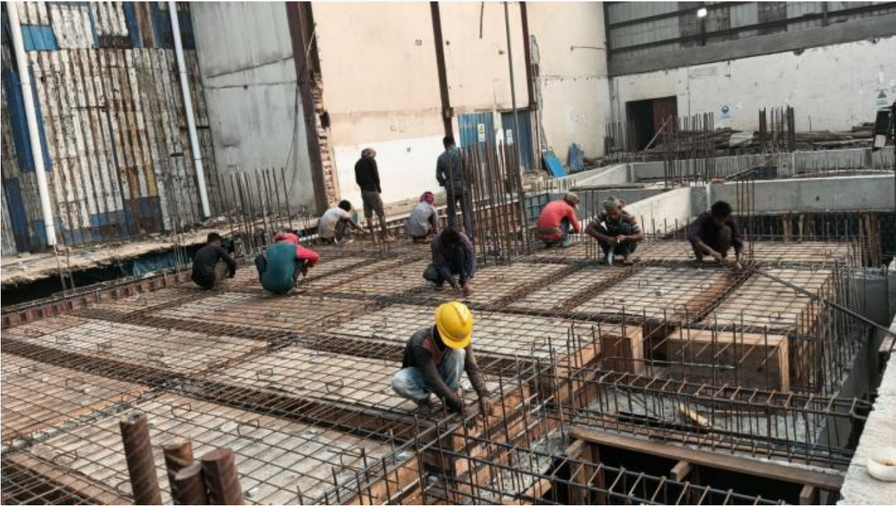
Tank slab re-bar work on 24-11-24
