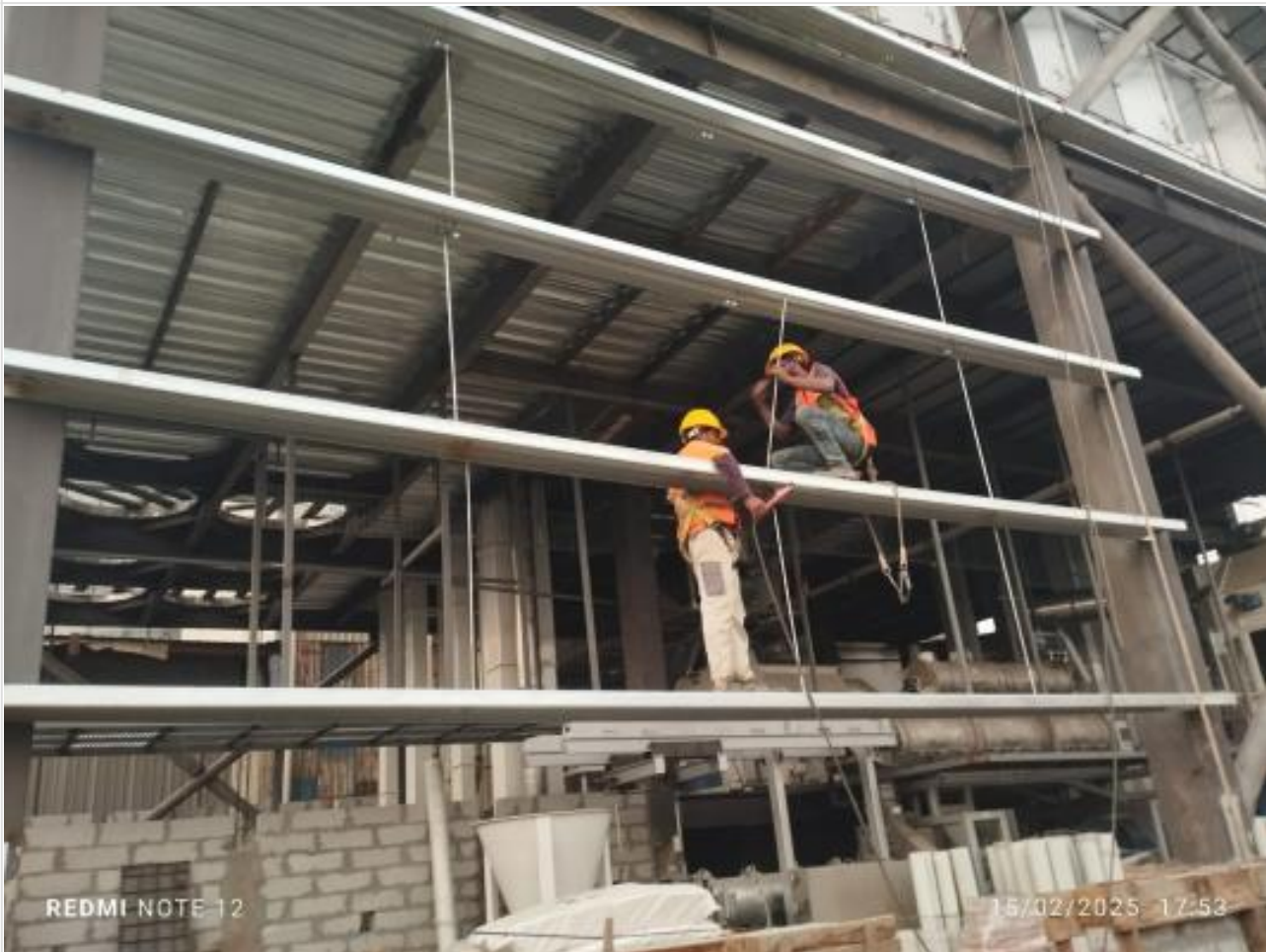
Sag Rod fixing on 15-02-25
