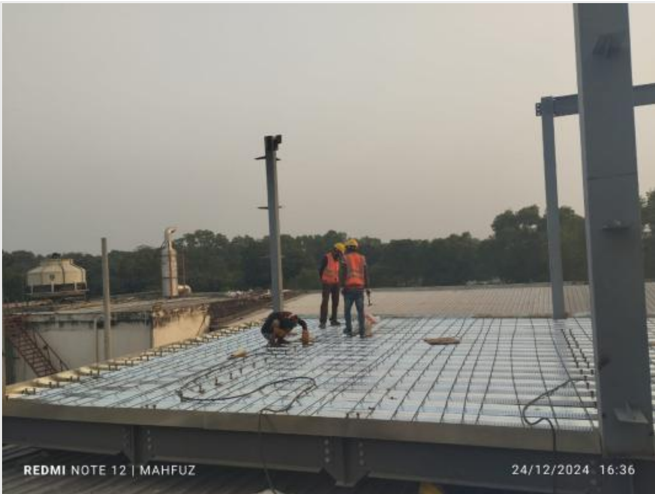
Shear bolt fixing on decking slab on 24-12-24
