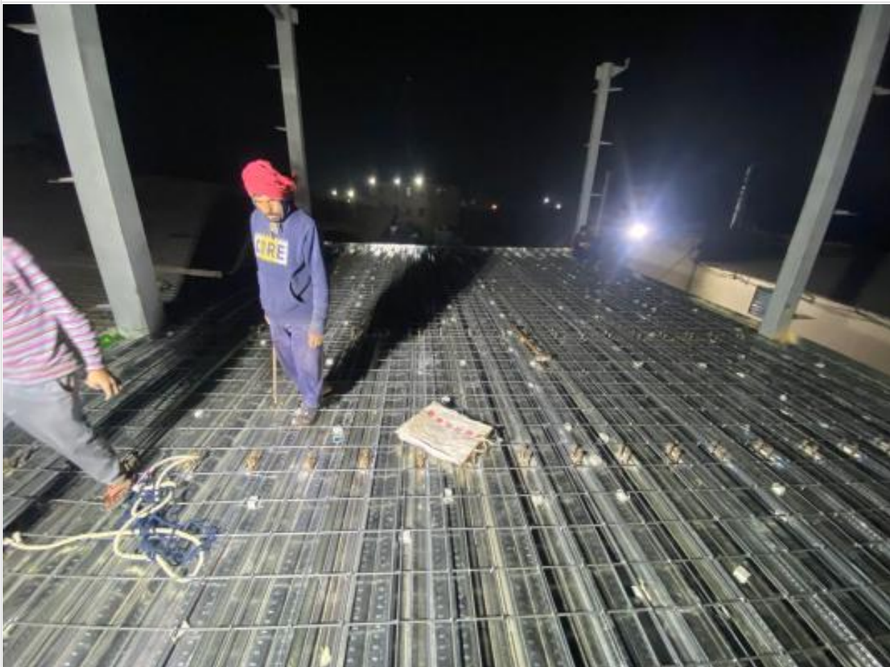
Re-bar fixing on decking slab on 24-12-24
