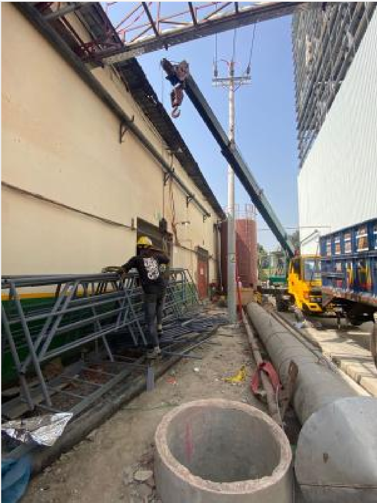
Lifting Roof top rail on 05-03-25
