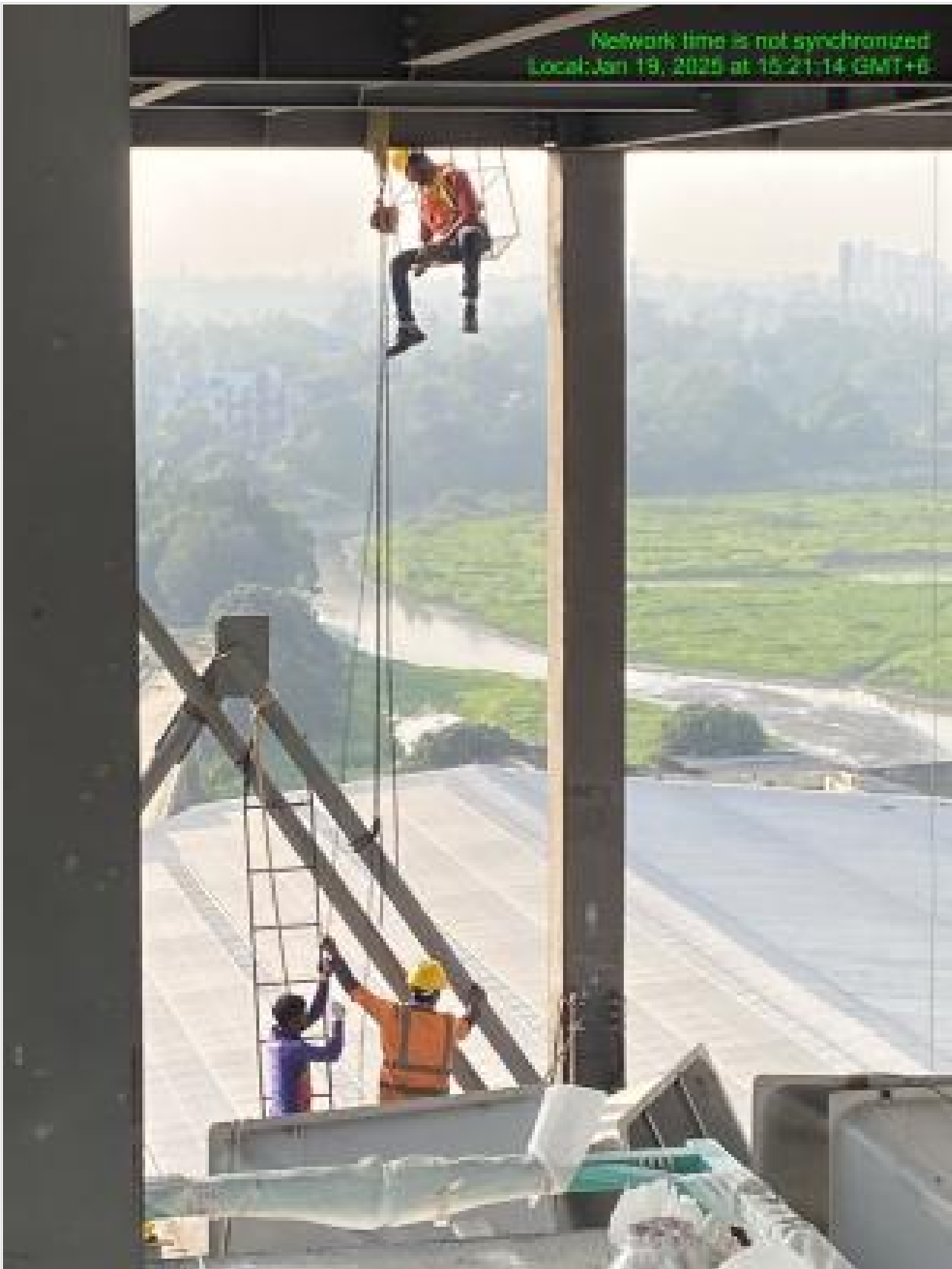
Steel bracing fixing on 19-01-25
