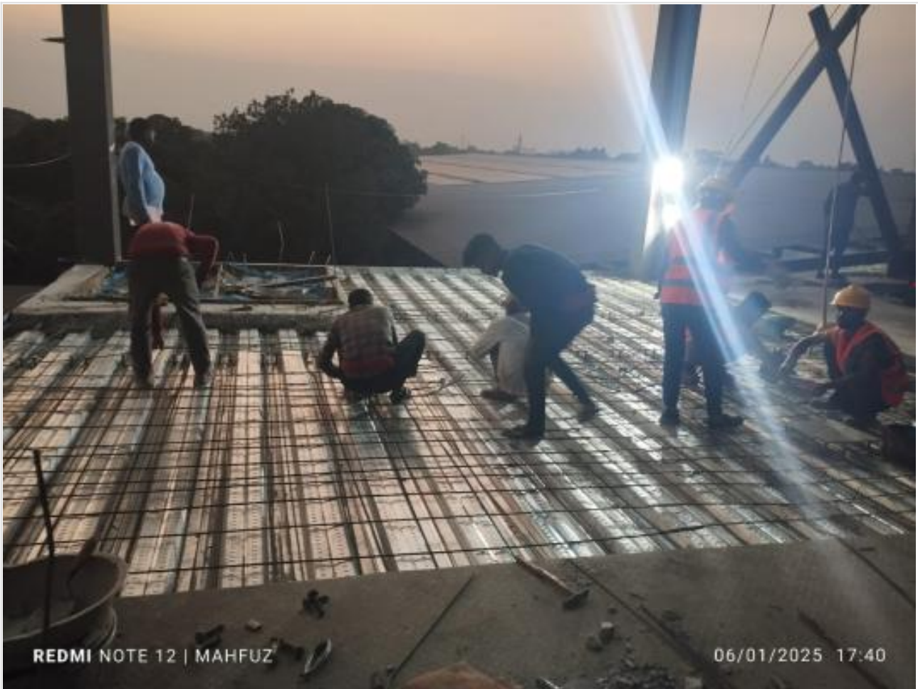
Re-bar fixing on decking slab on 06-01-25
