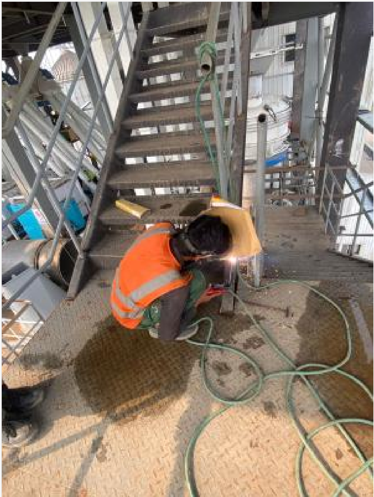
Stair welding on 12-02-25
