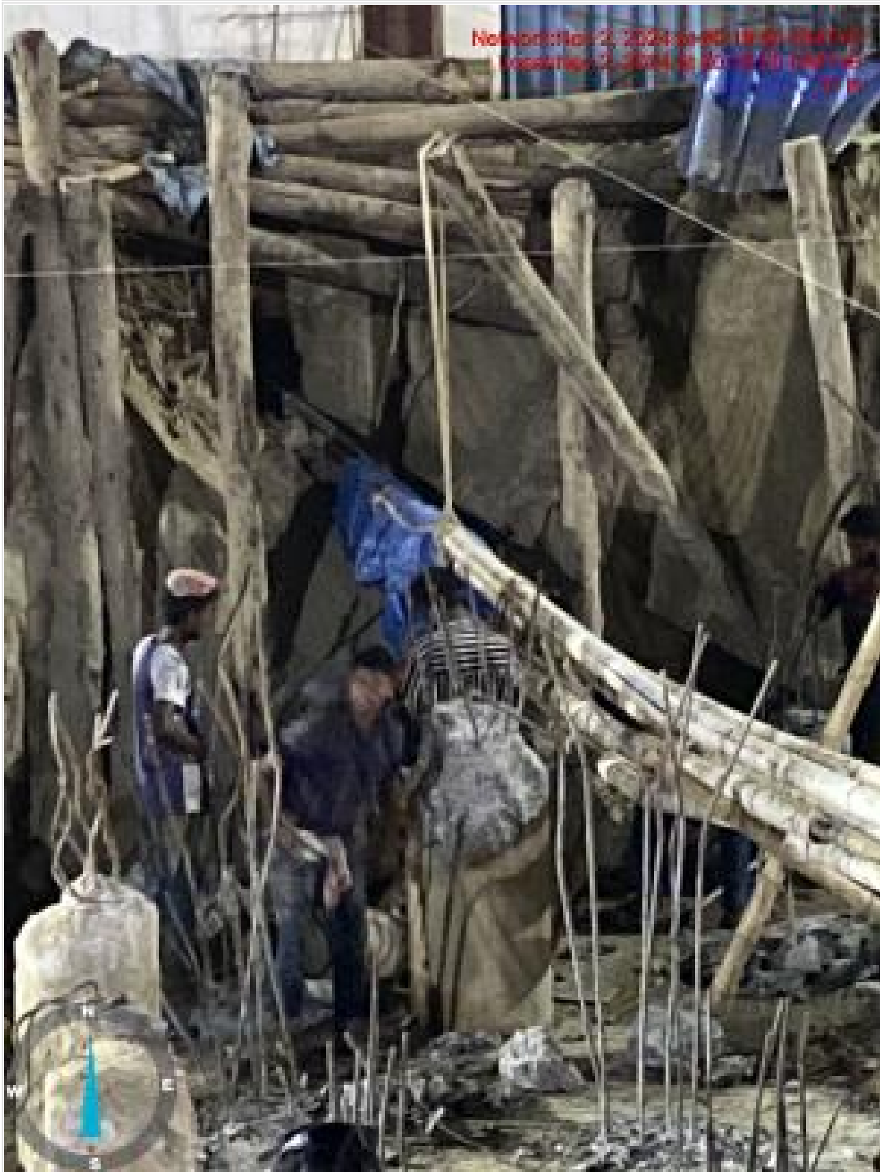
Pile head breaking on 02-11-24
