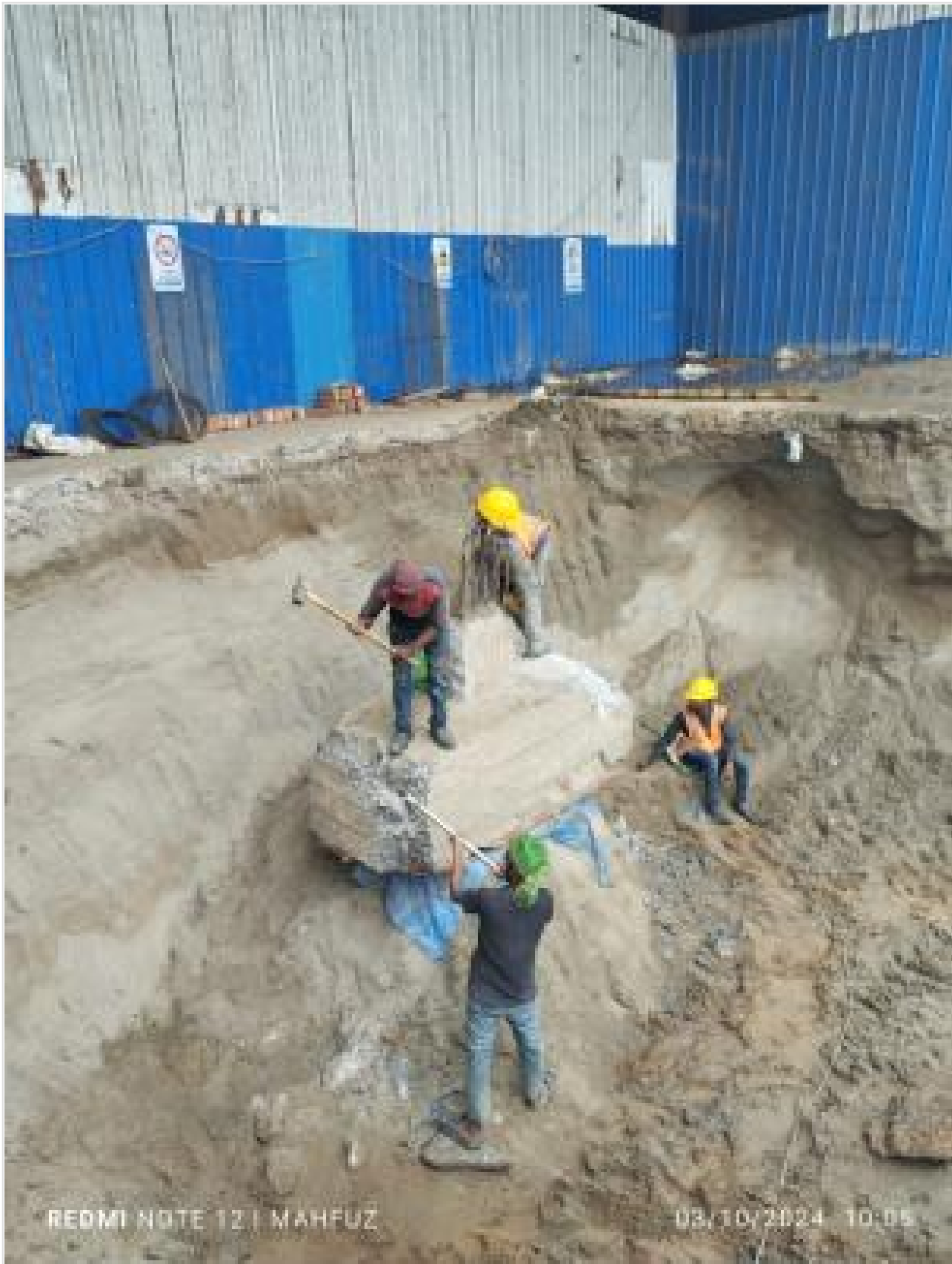
Obstacle RCC dismantling on 03-10-24
