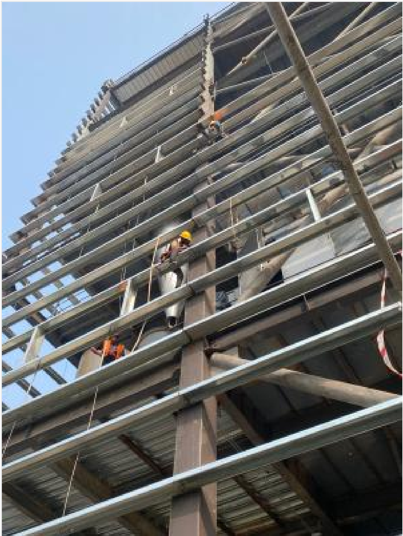
Wall purlin fixing on 20-02-25
