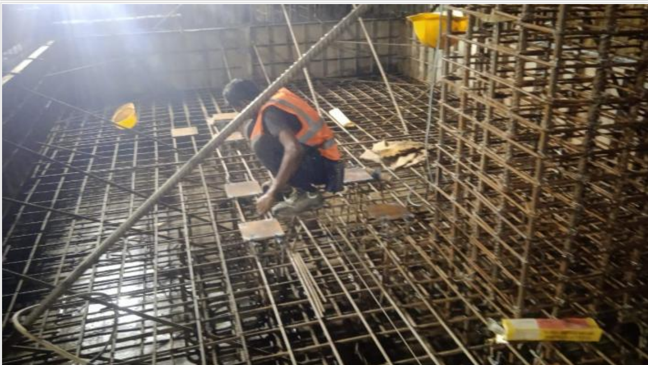
Pile cap re-bar work on 27-10-24
