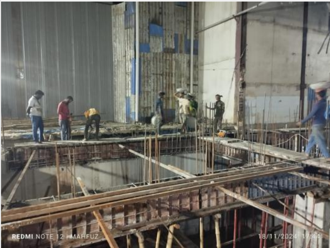
Foundation beam concreting on 18-11-24
