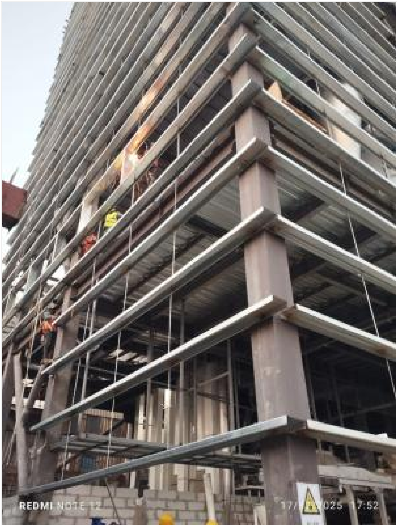
Sag Rod fixing on 17-02-25
