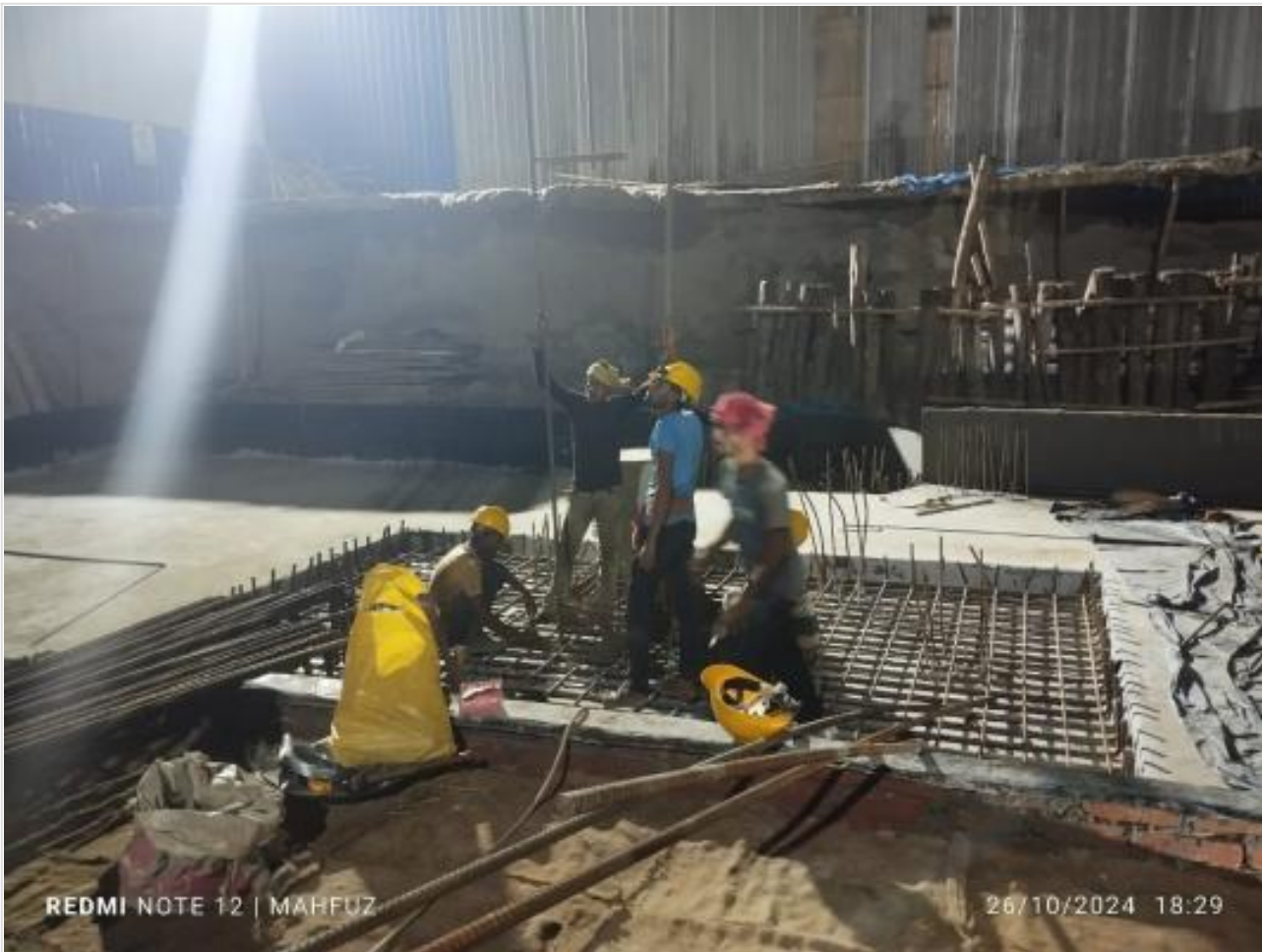
Pile cap re-bar work on 26-10-24
