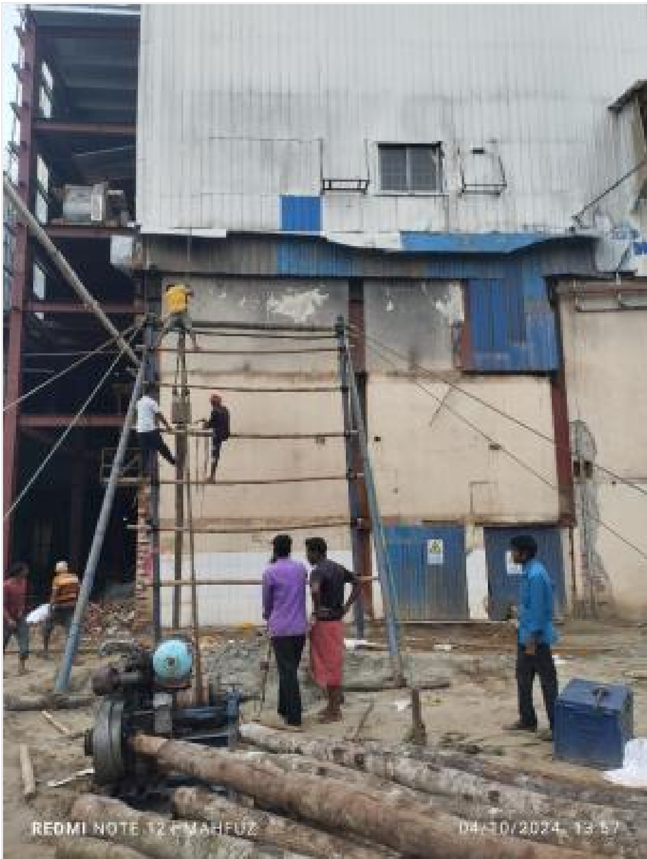
Wooden pile driving on 04-10-24
