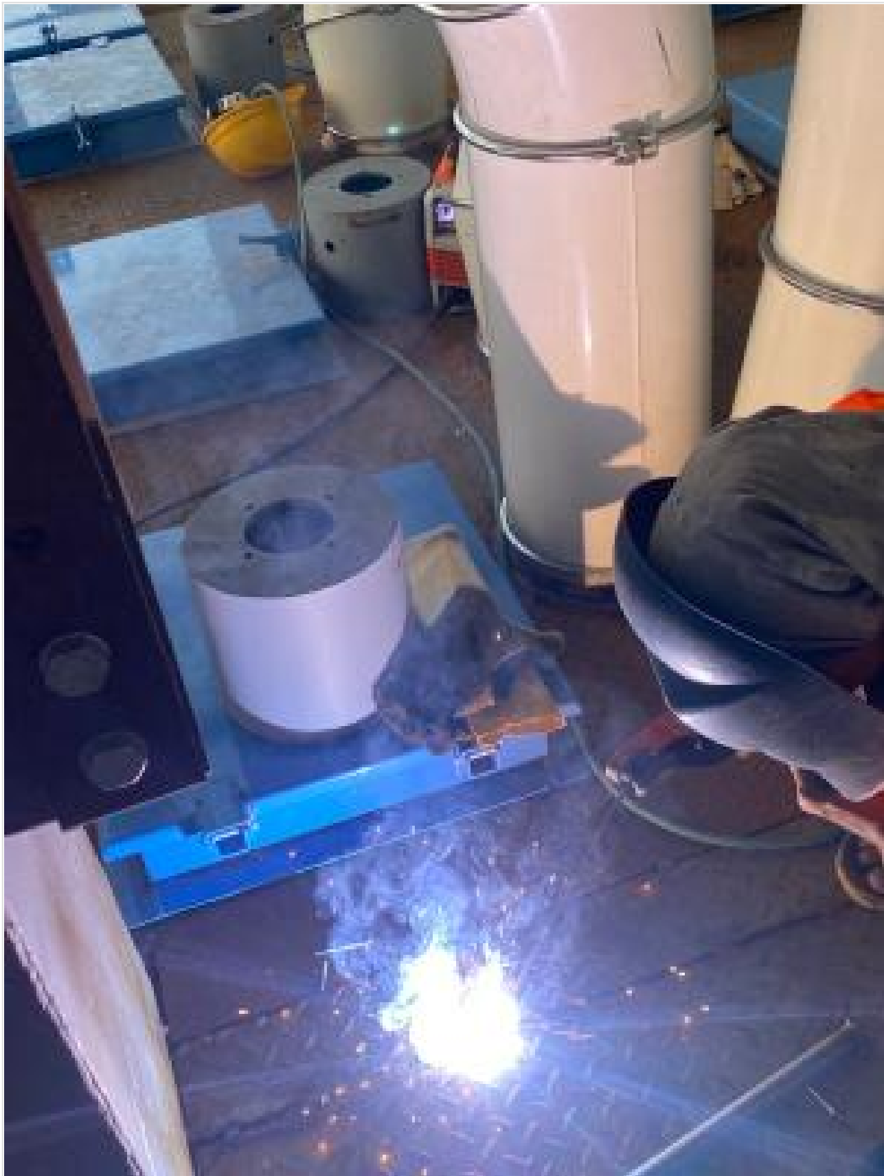
Checked plate welding on 23-02-25
