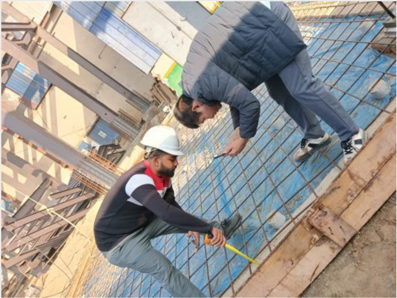
Re- bar inspection before concreting on 16-12-24
