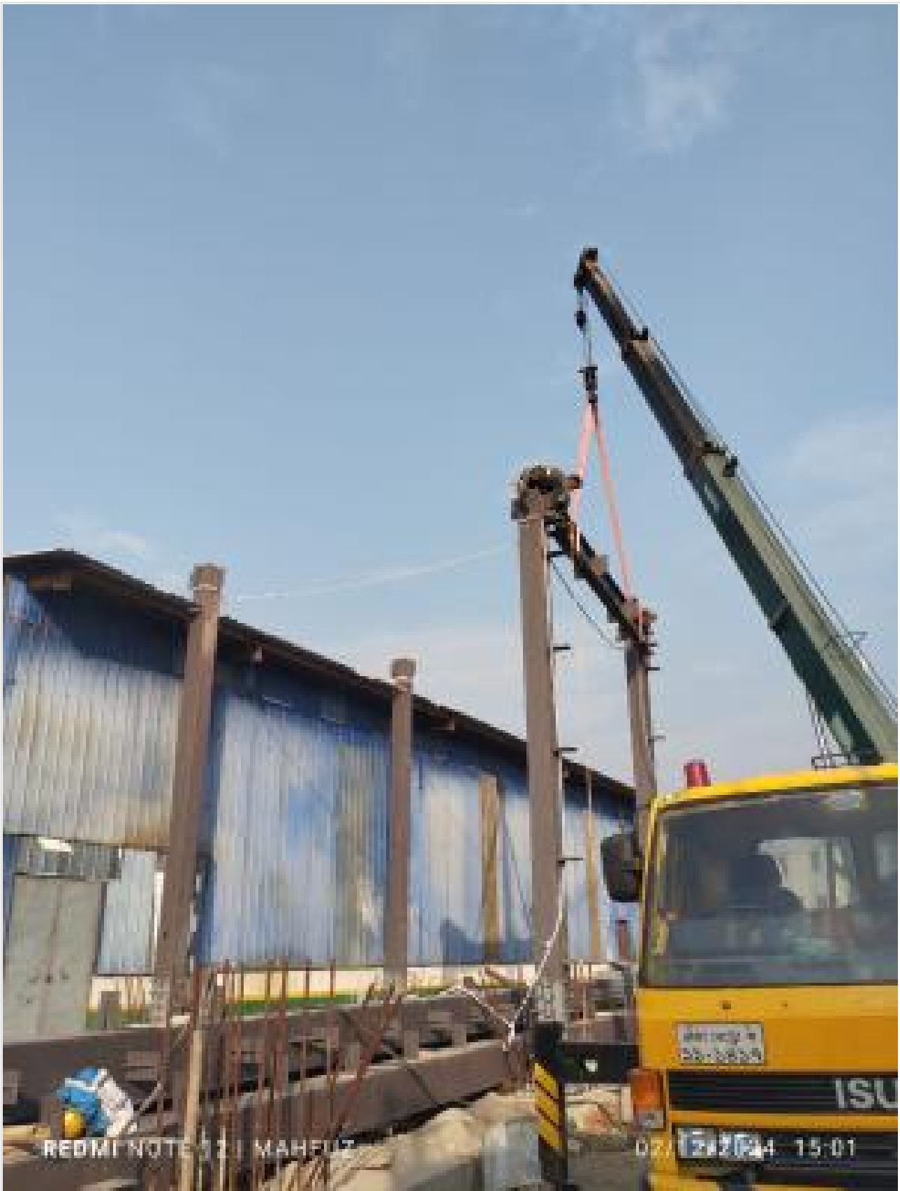
Installing steel beam on 02-12-24
