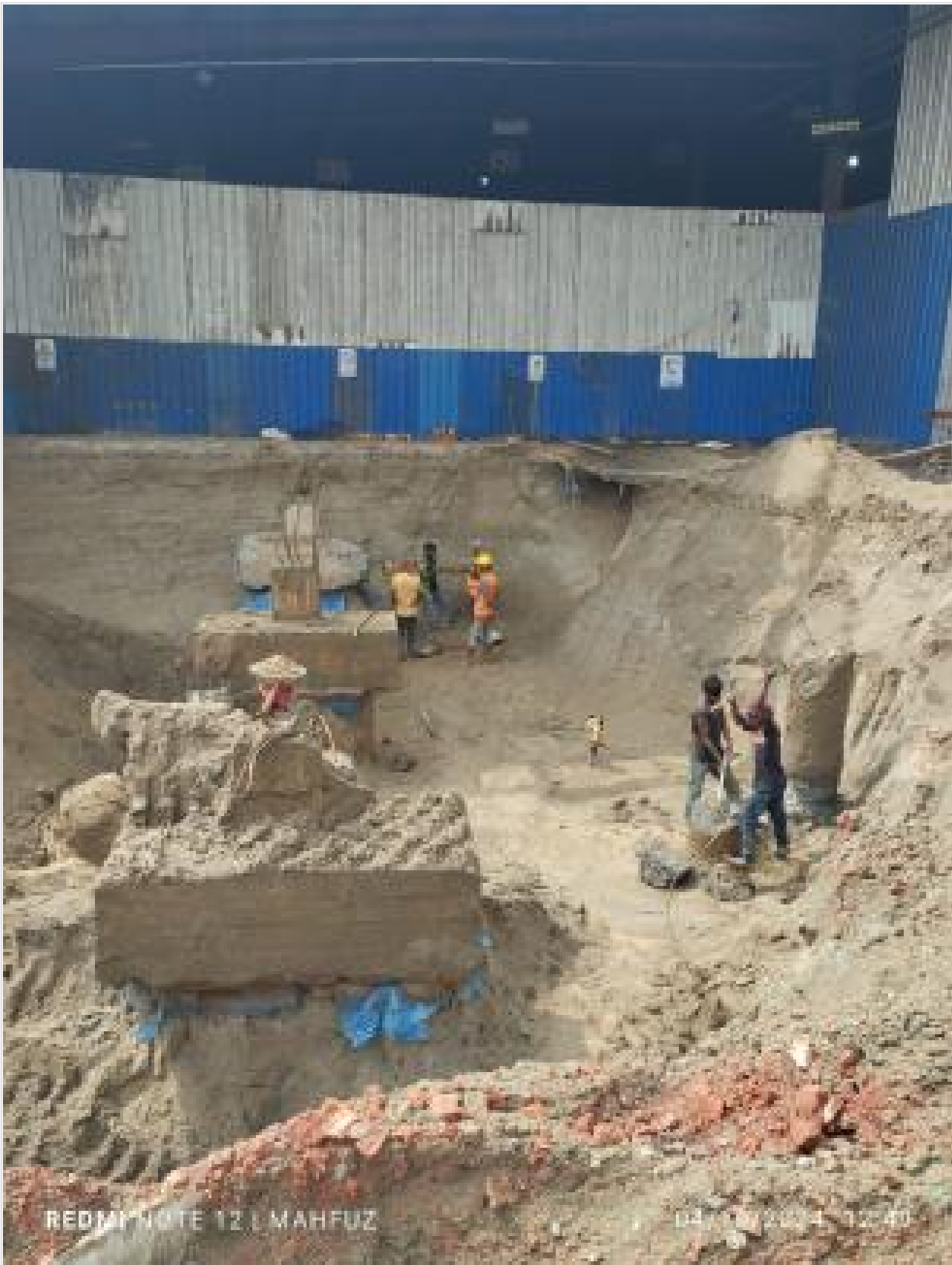
Pile Head breaking on 04-10-24
