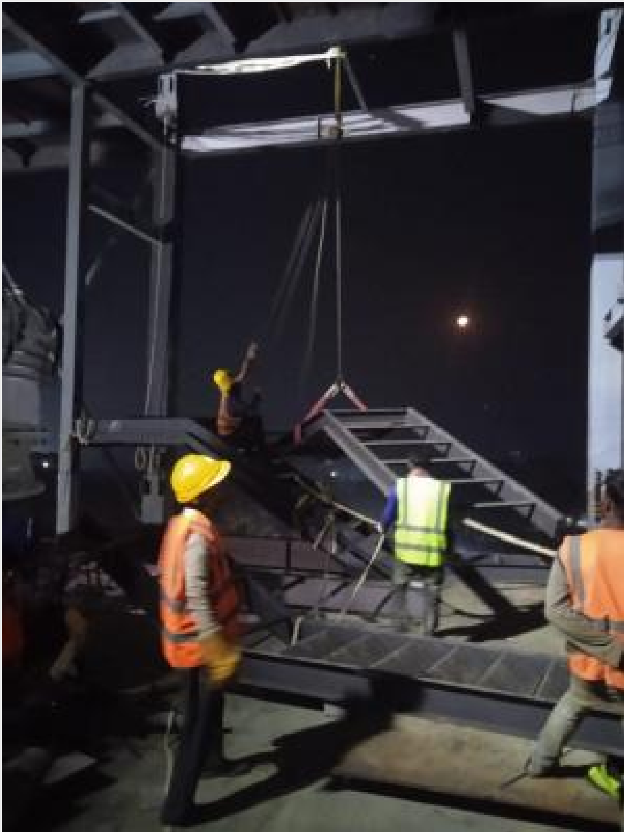
Steel stair installation on 16-01-25
