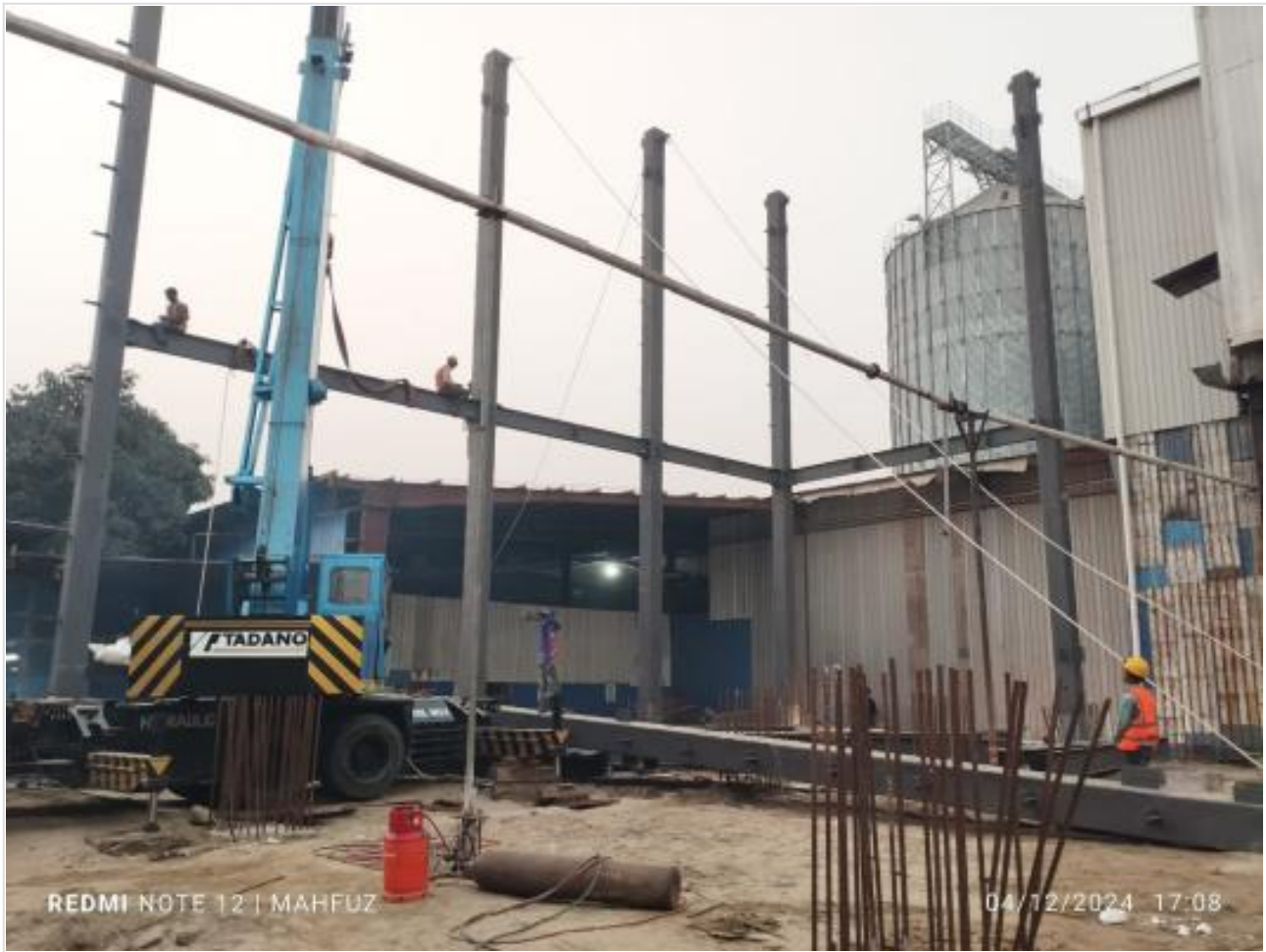
Steel structure installation on 04-12-24
