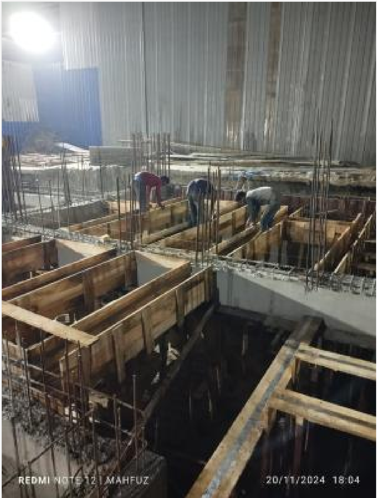
Tank slab shuttering on 20-11-24
