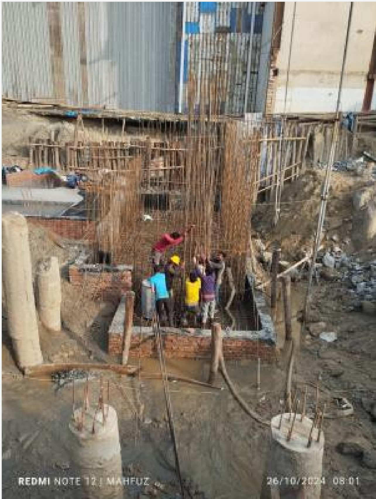
Column re-bar work on 26-10-24
