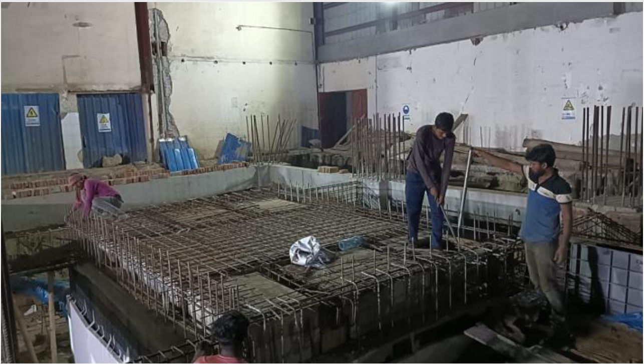
Tank slab re-bar fixing on 28-11-24
