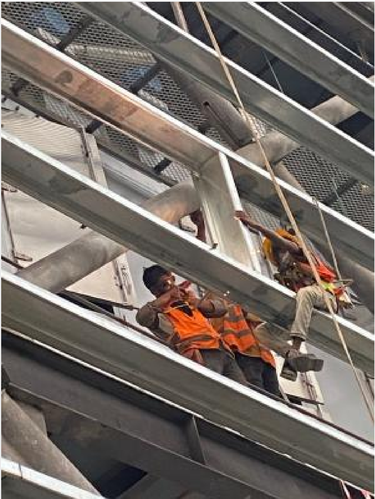
Window frame fixing on 19-02-25
