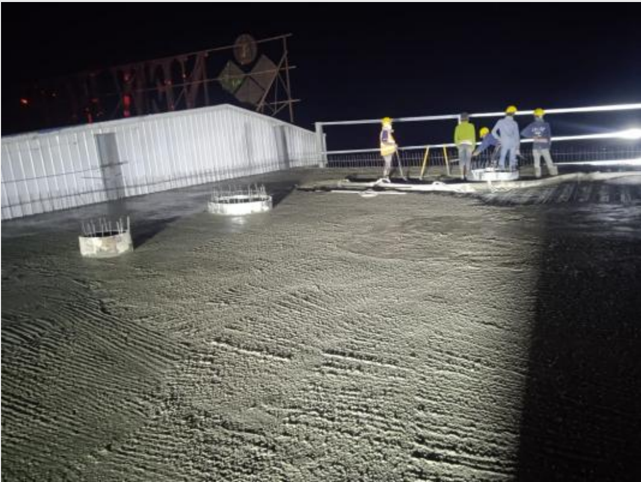
5th Floor roof slab concreting on 10-02-25
