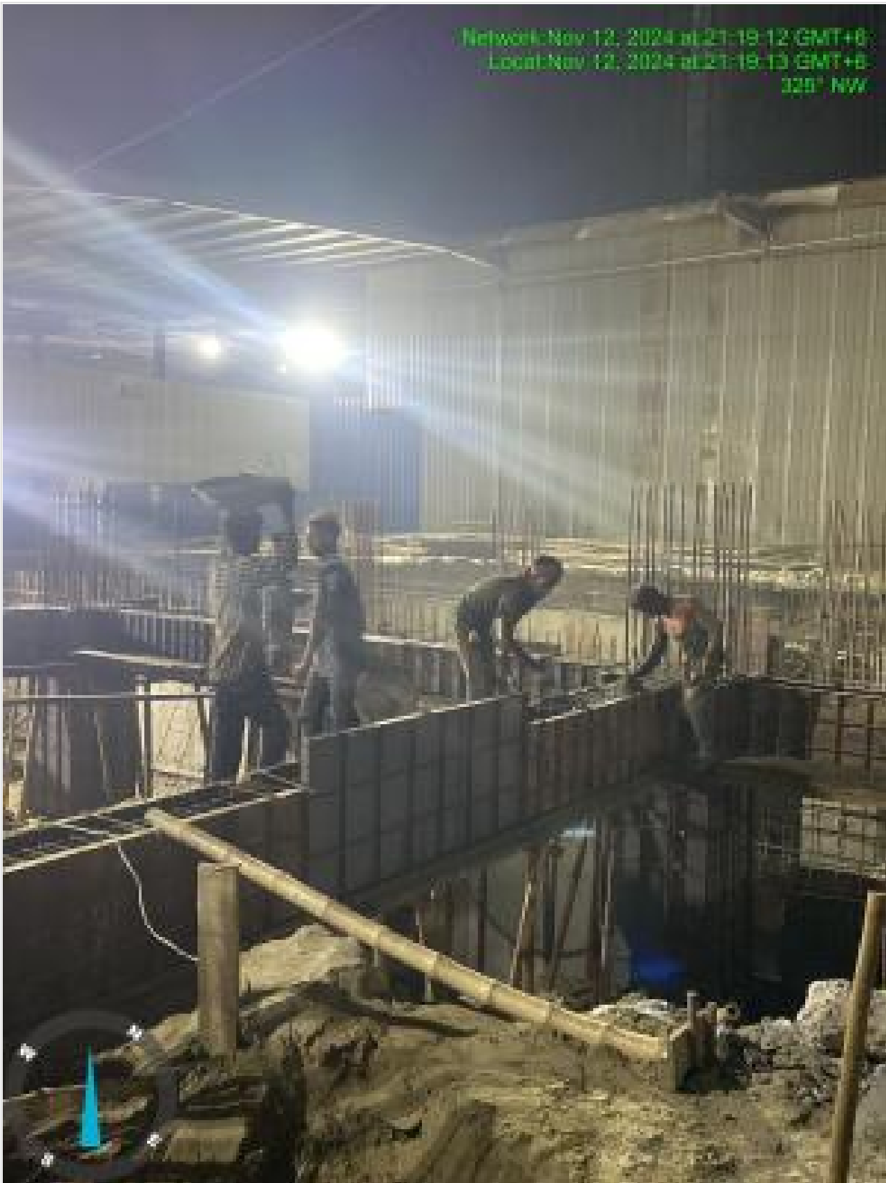
Foundation beam concreting on 12-11-24
