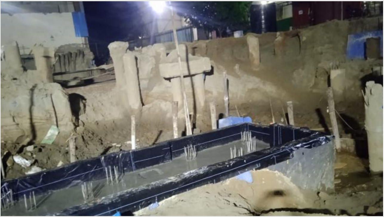
Tank base top mortering on 22-10-24
