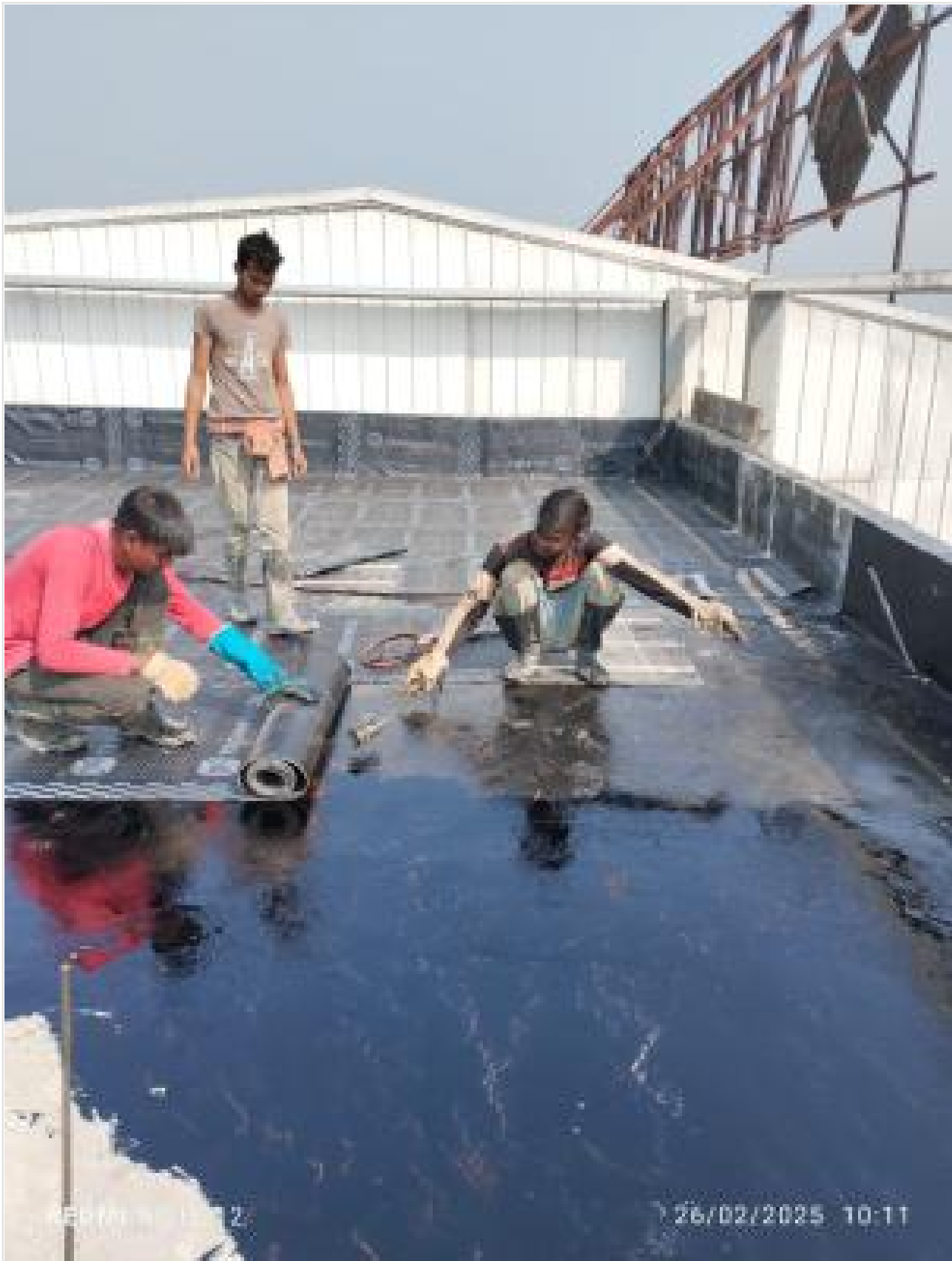
Fixing water proofing membrane on roof top on 26-02-25
