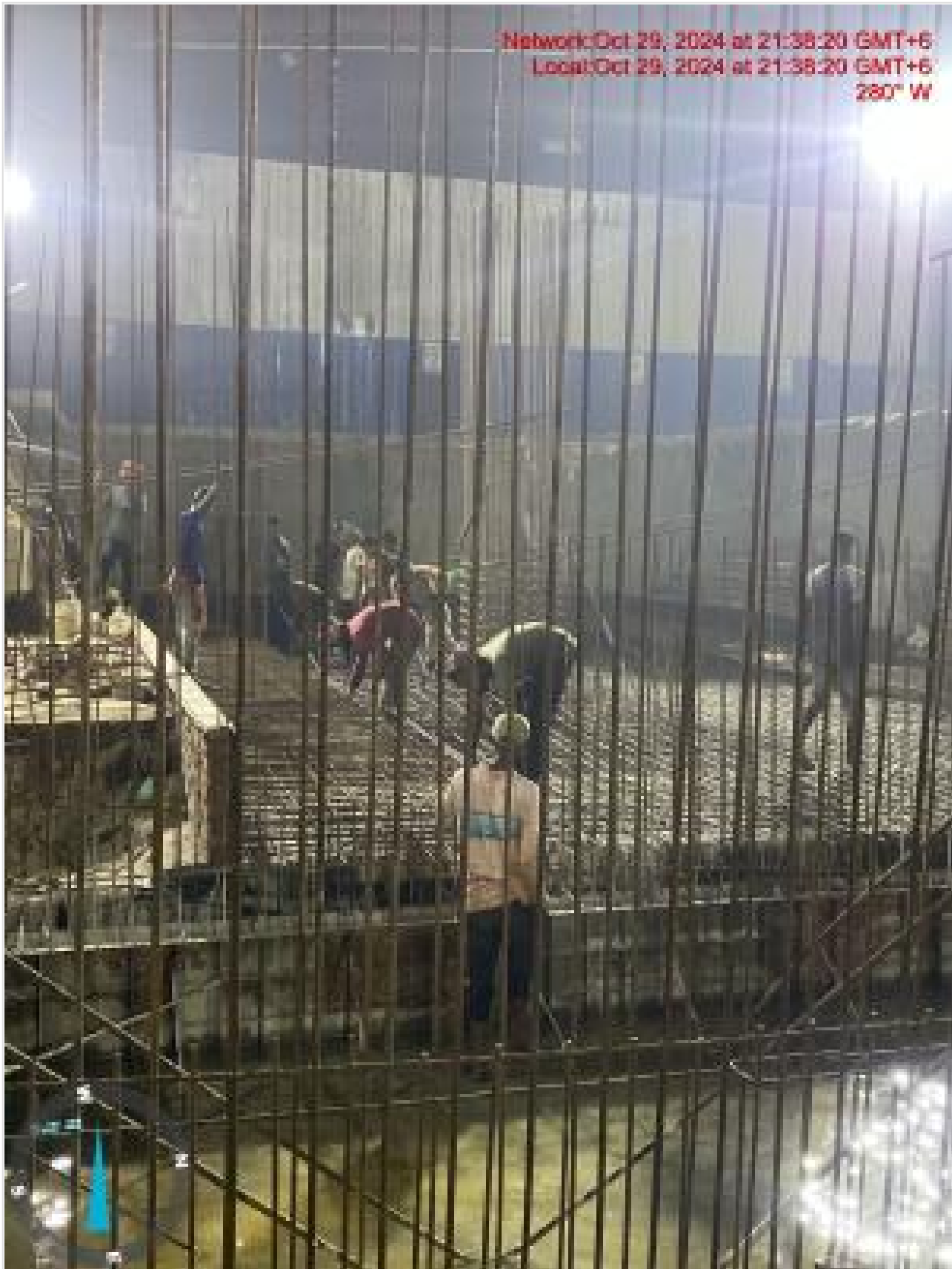
Raft re-bar work on 29-10-24
