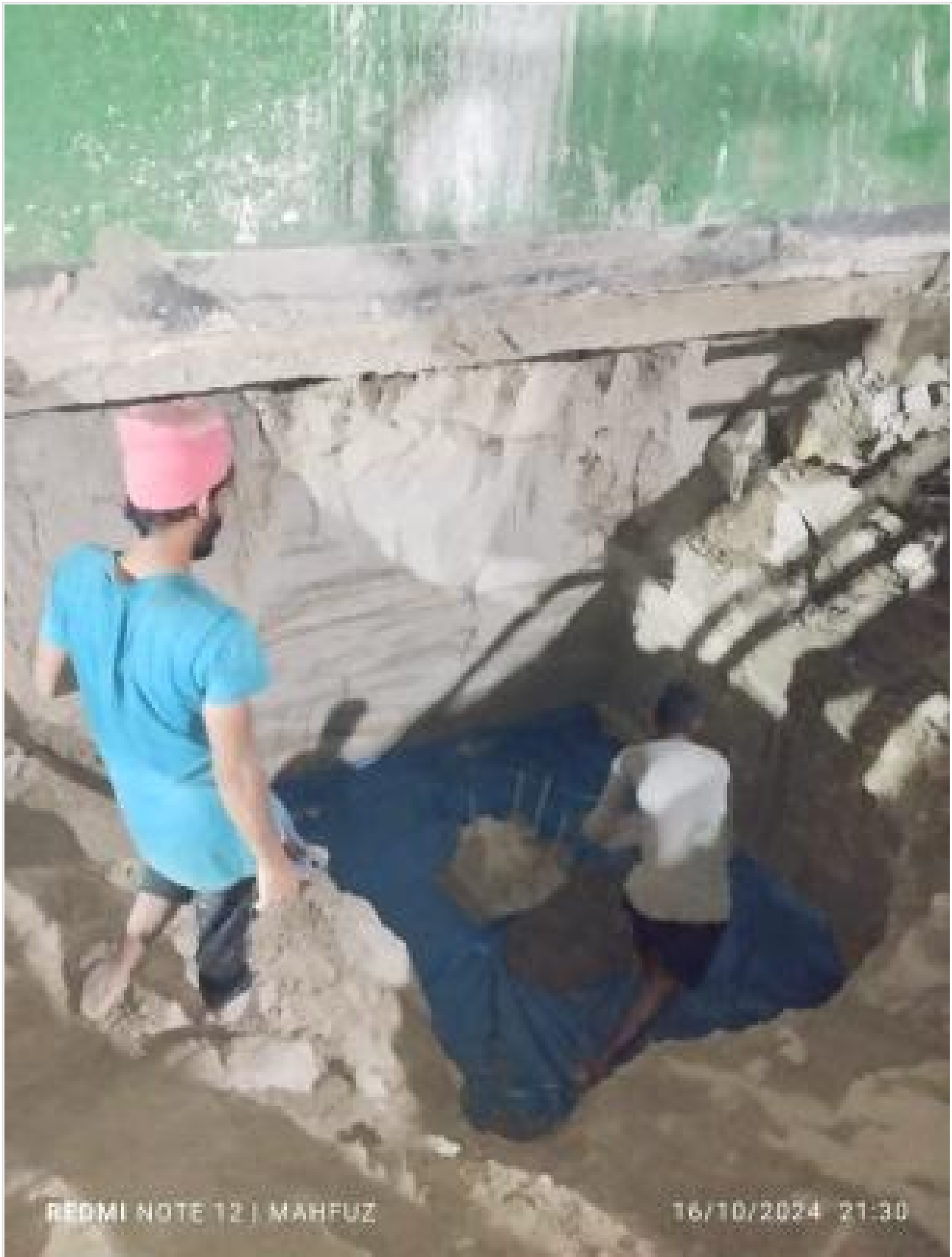
Pile Cap Lean concreting on 16-10-24
