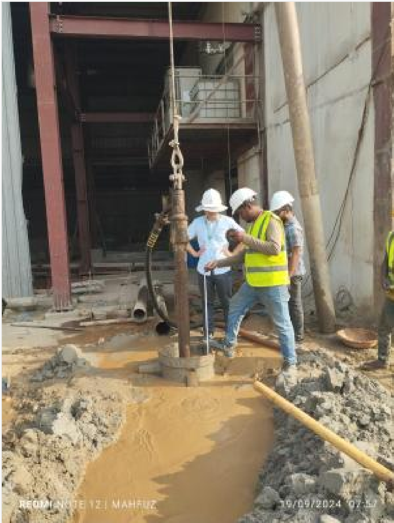
Pile boring length checking on 19-09-24
