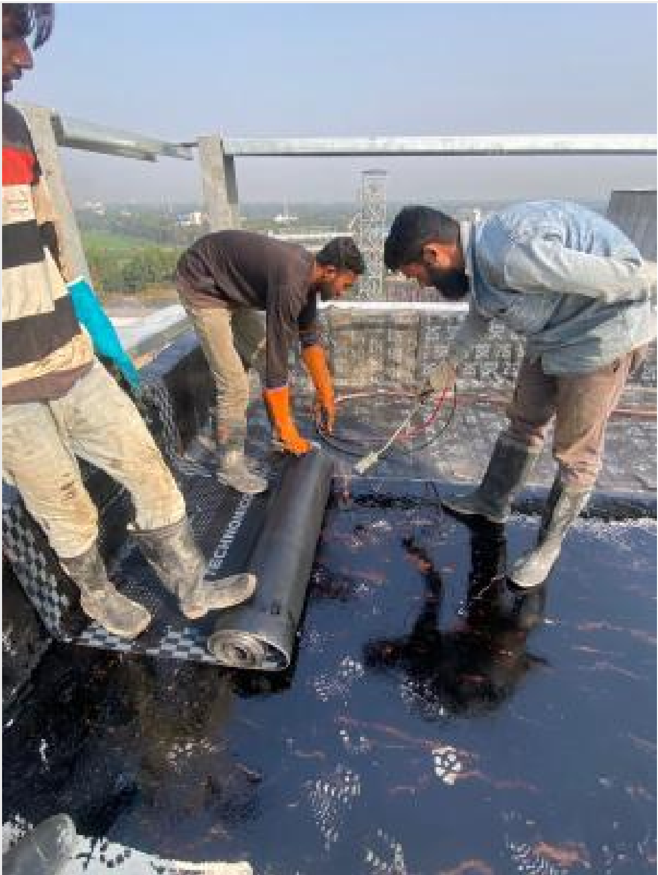
Roof top water proofing on 25-02-25
