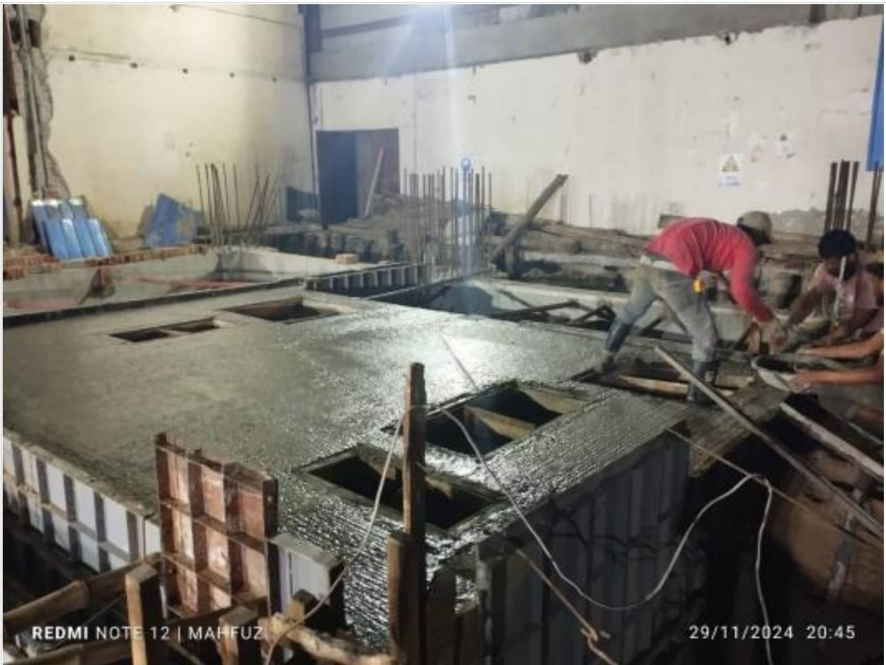
Tank slab concreting on 29-11-24
