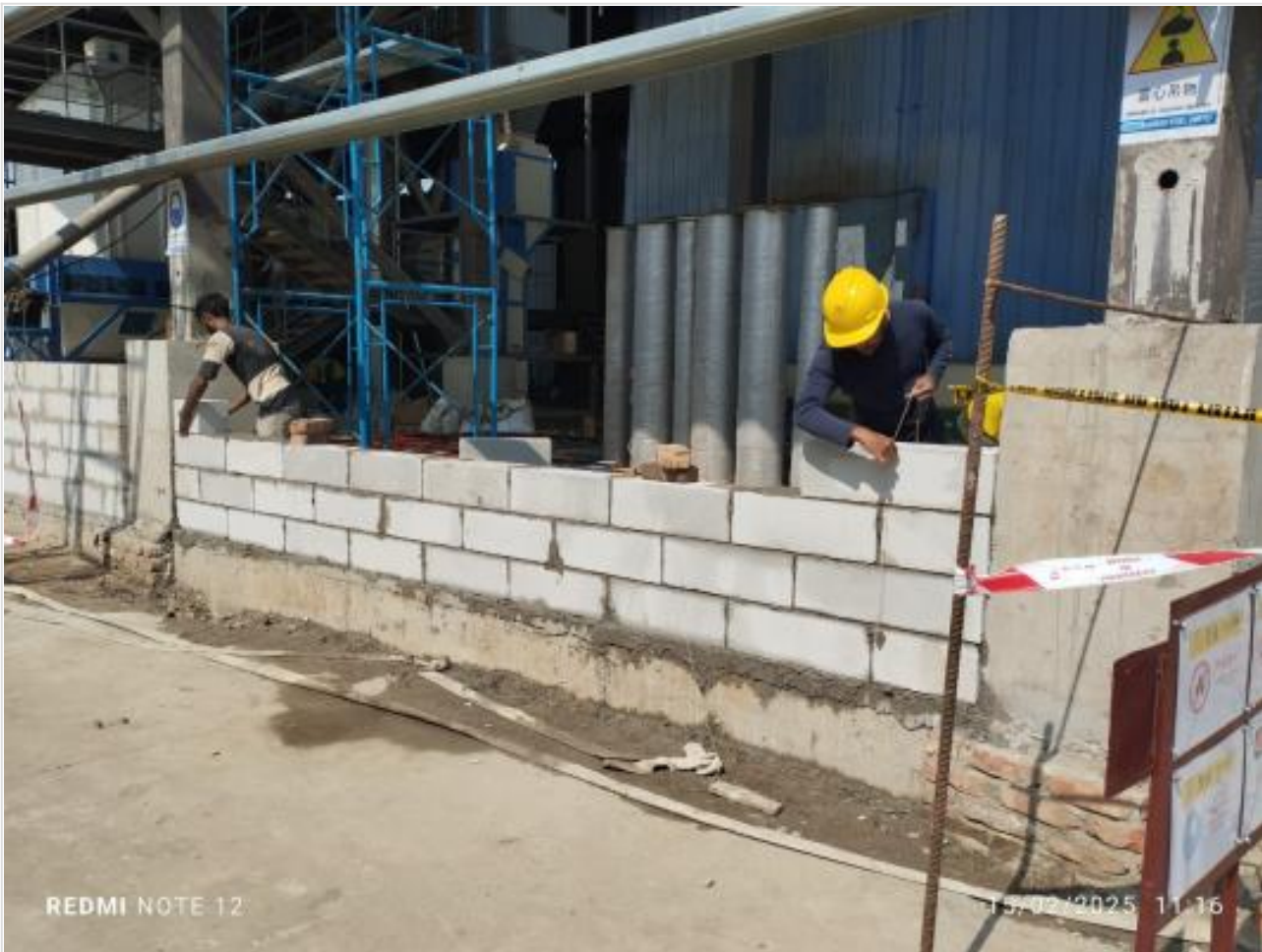
AAC block work on 15-02-25
