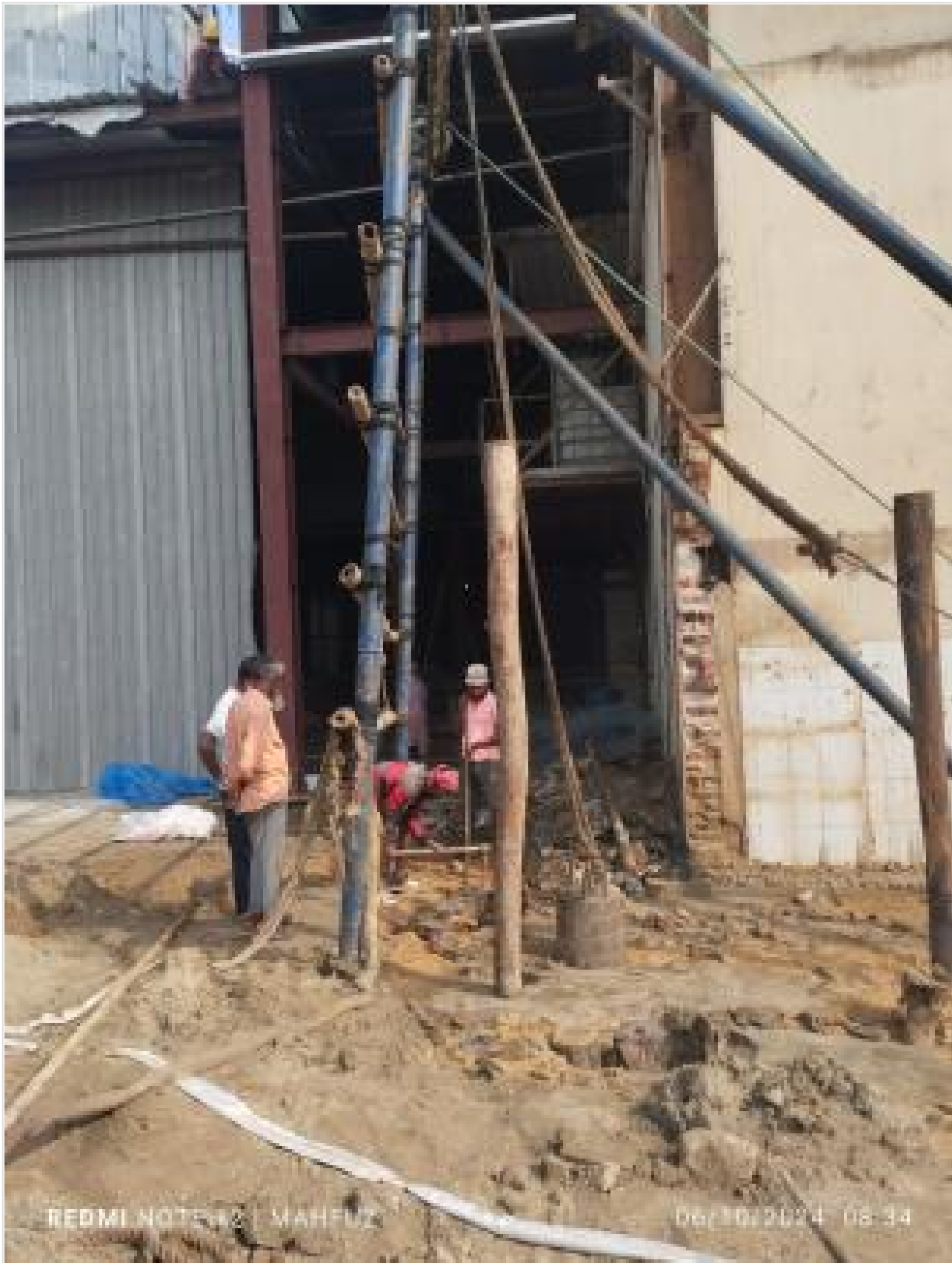
Wooden shore pile driving on 06-10-24
