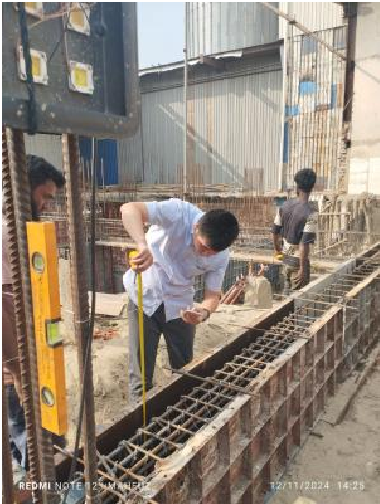
Foundation beam inspection before concrete on 12-11-24
