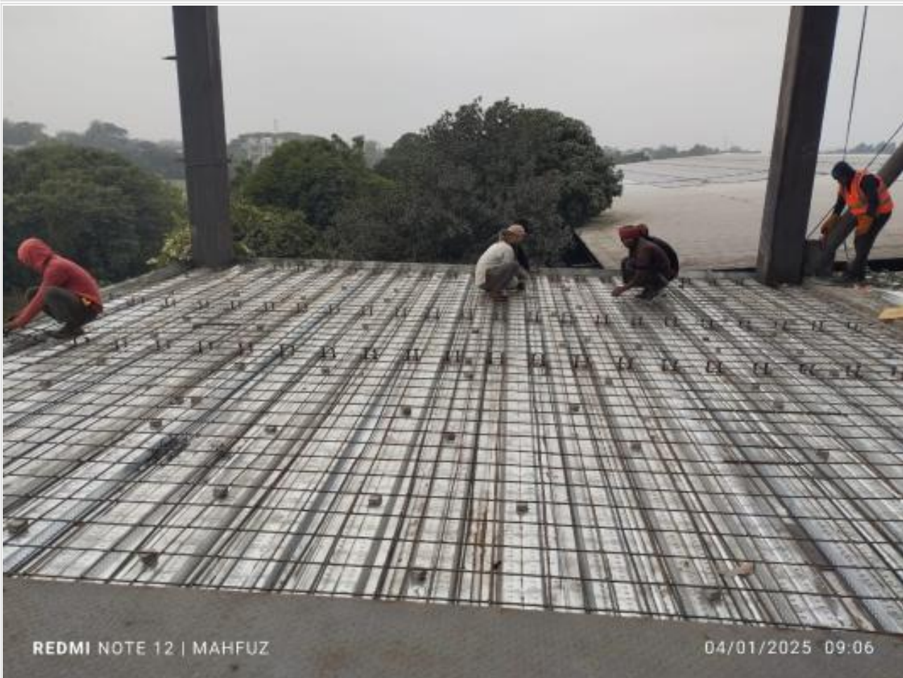
Re-bar fixing on Decking slab on 04-01-25
