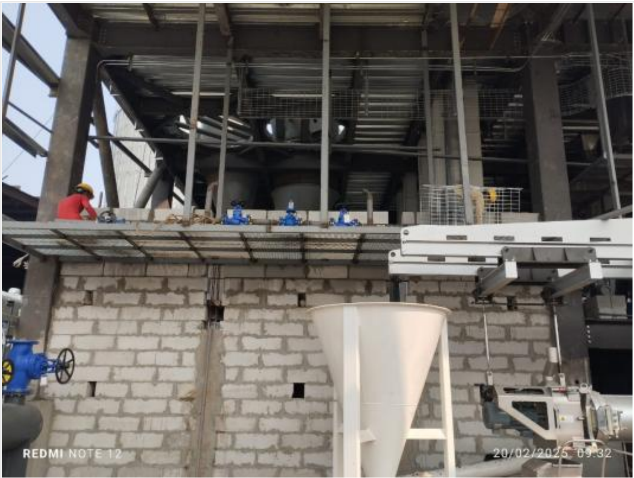
AAC block work on 20-02-25
