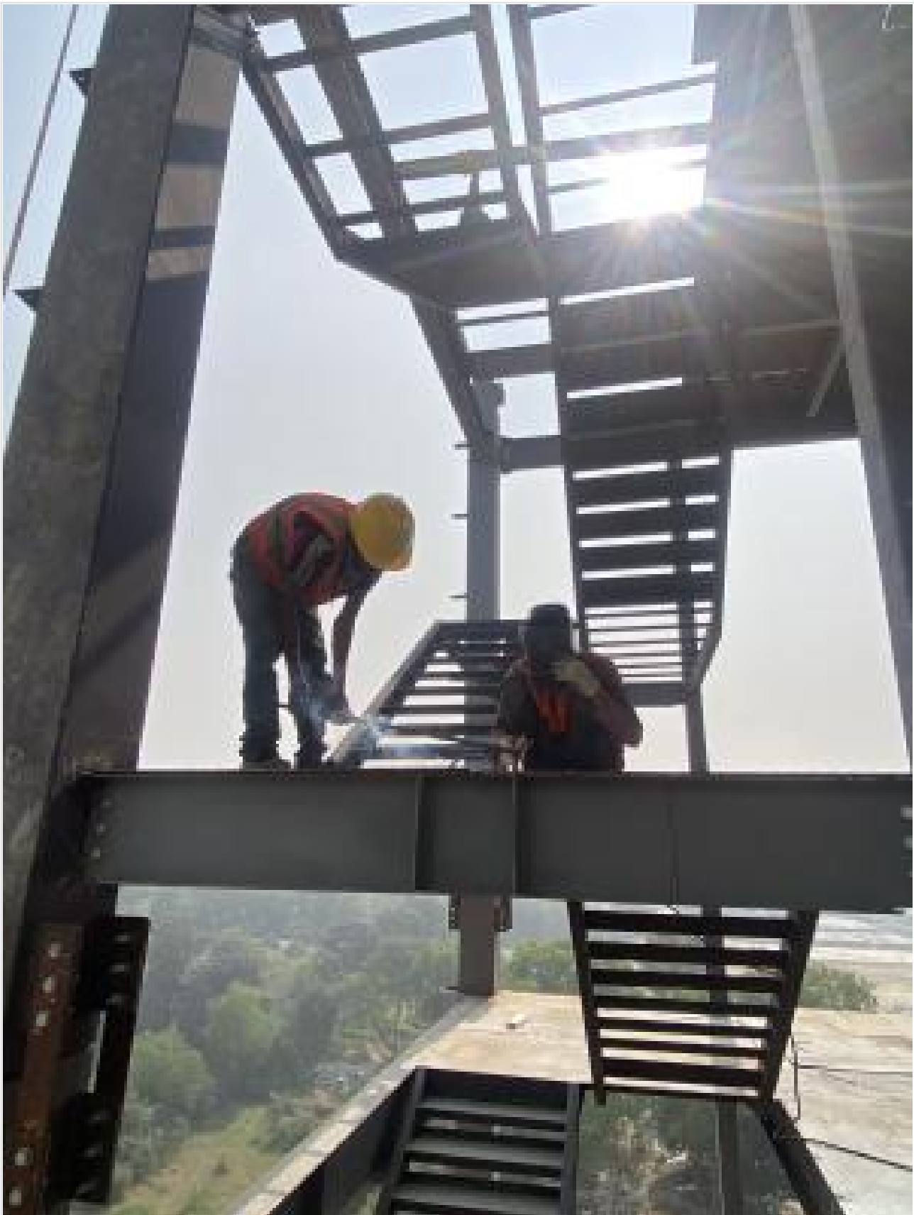
Stair landing checkered plate fixing on 18-01-25
