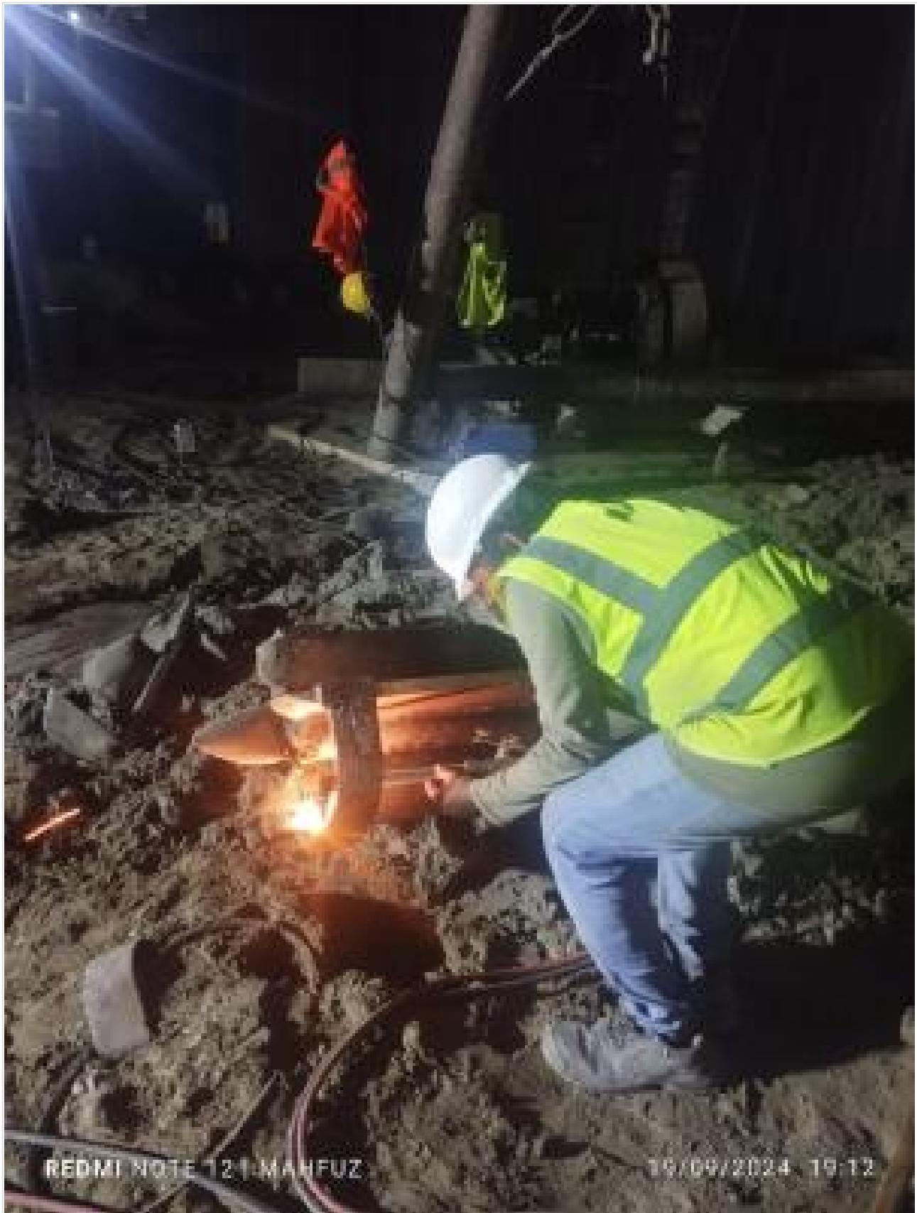
Pile boring chisel repairing on 19-09-24
