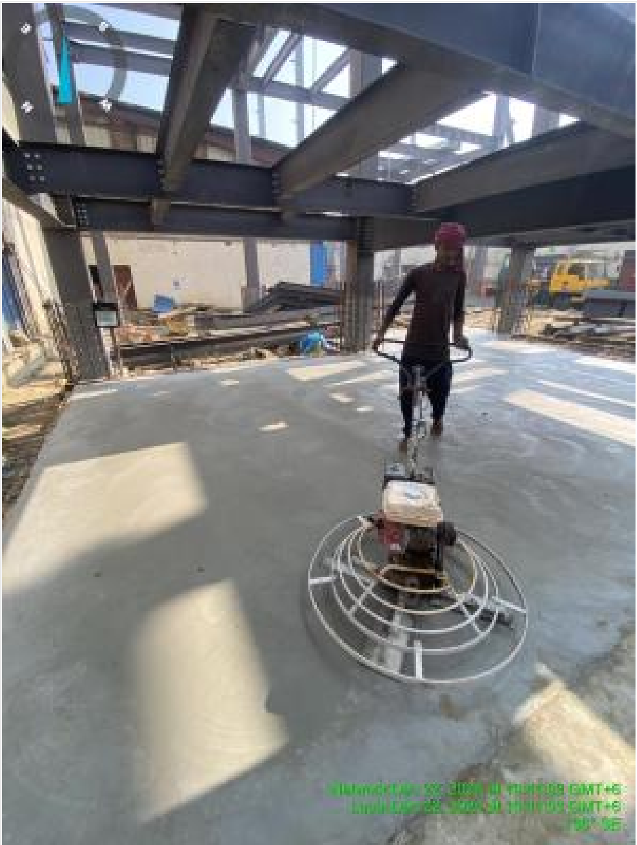
Mechanical troweling on 22-12-24
