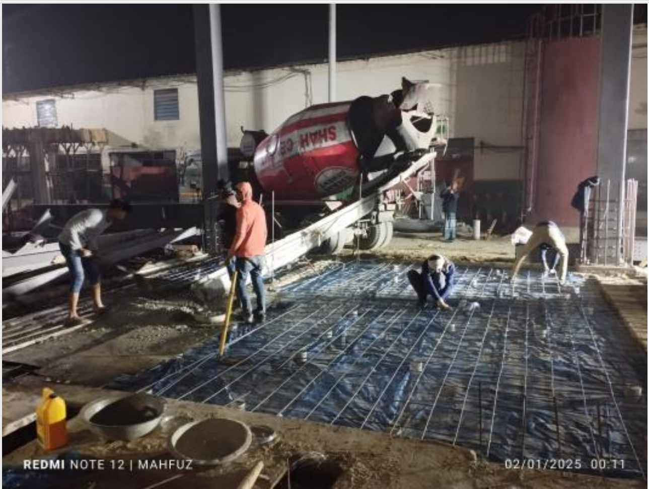
Ground Floor RCC Slab Concreting on 01-01-25
