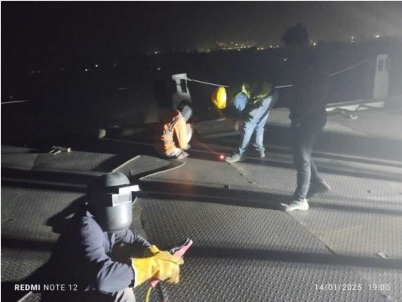
Checked plate fixing on 14-01-25
