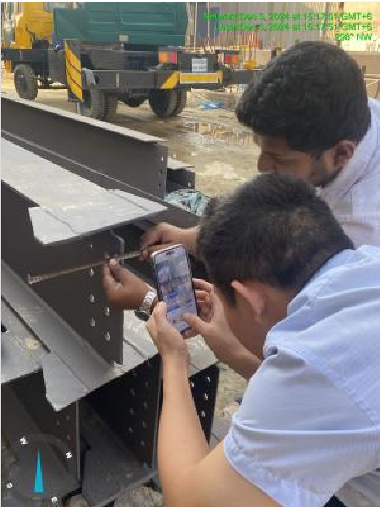
Steel member size checking on 03-12-24
