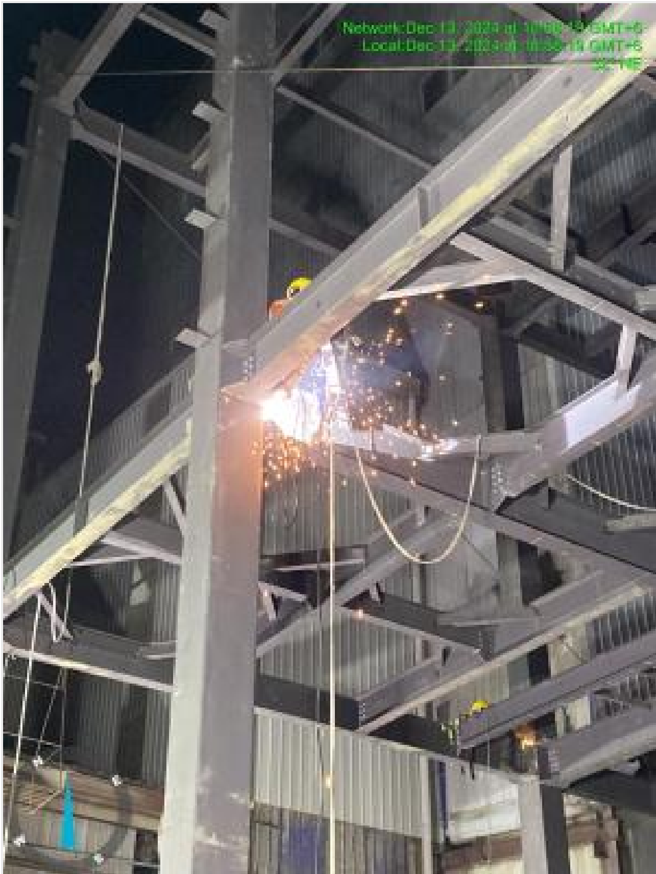
Steel structure wedding work on 13-12-24
