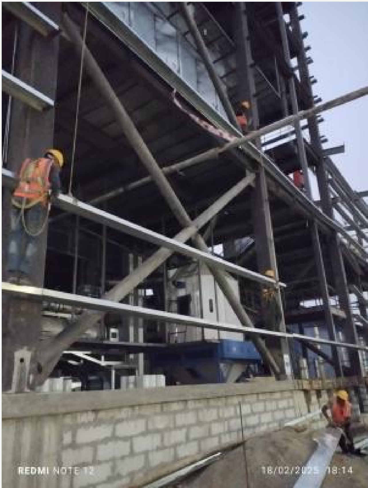
Purlin fixing on 18-02-25
