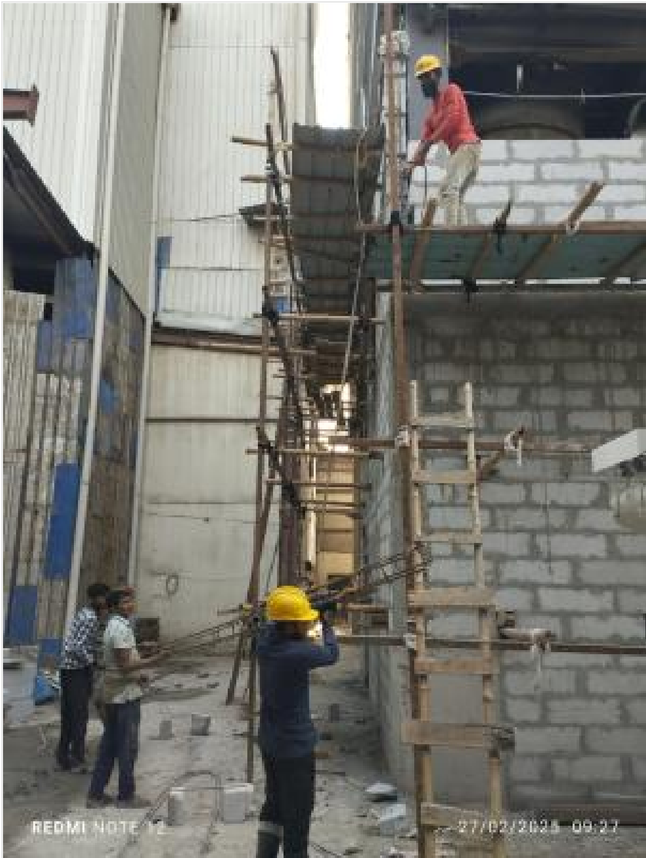
AAC block work on 27-02-25
