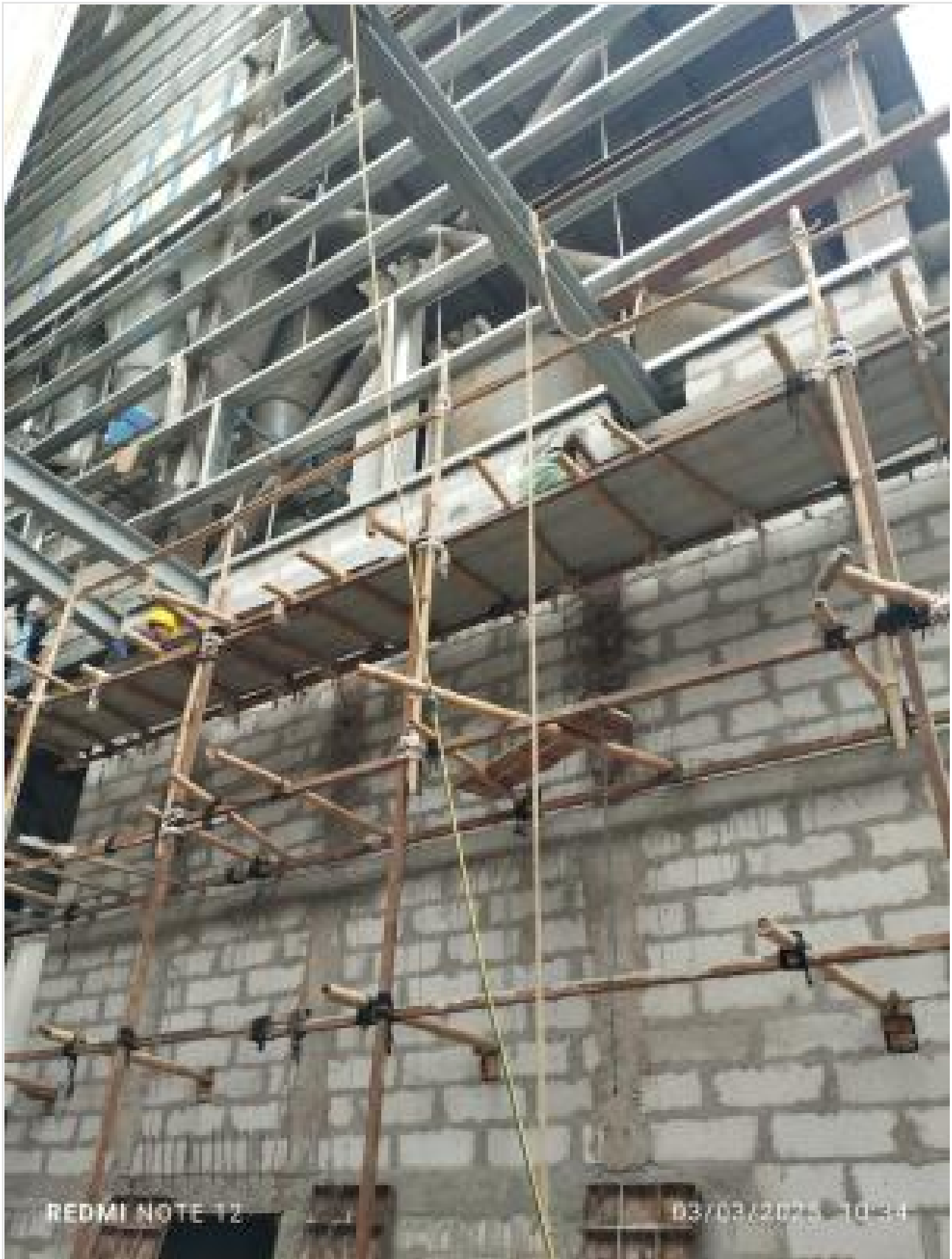
AAC block work on 03-03-25
