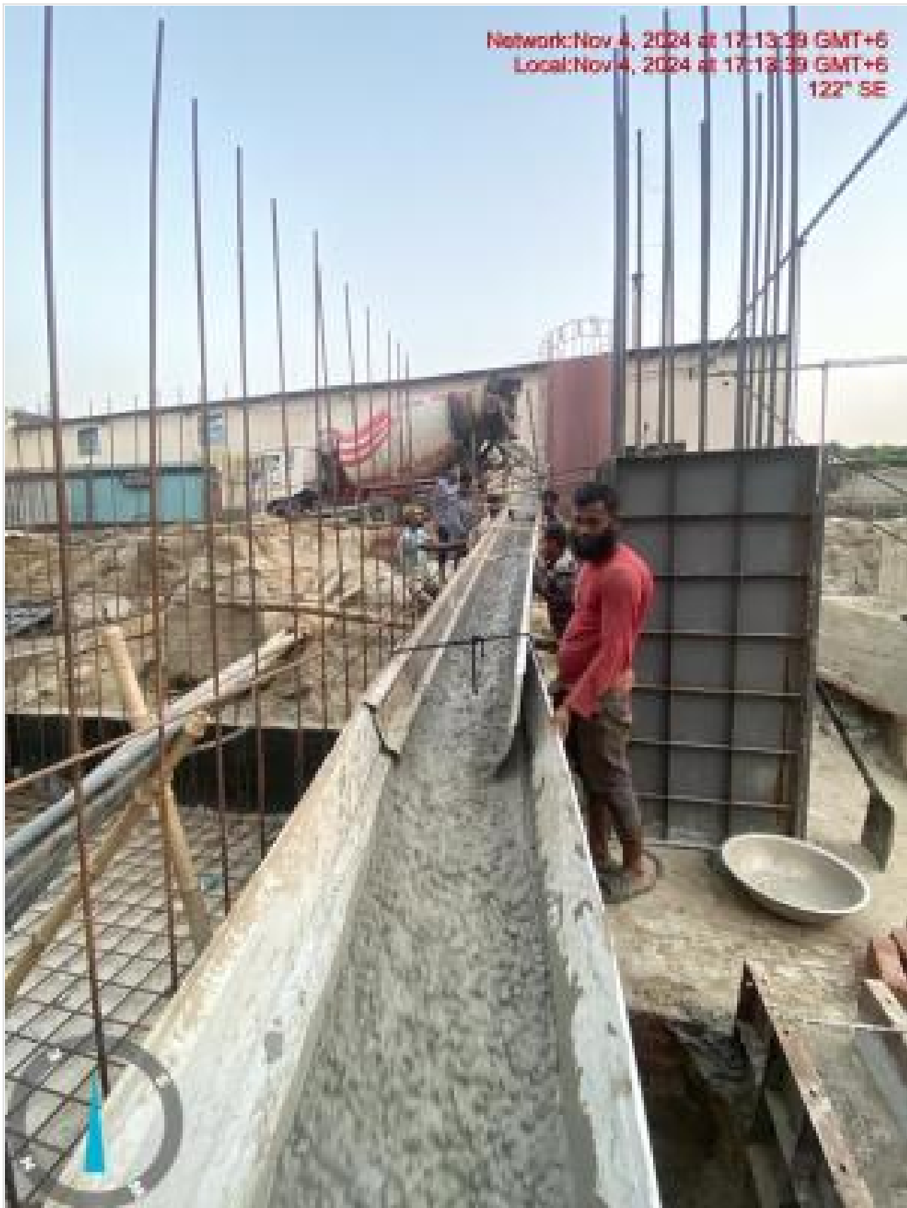
Pile cap Concreting on 04-11-24
