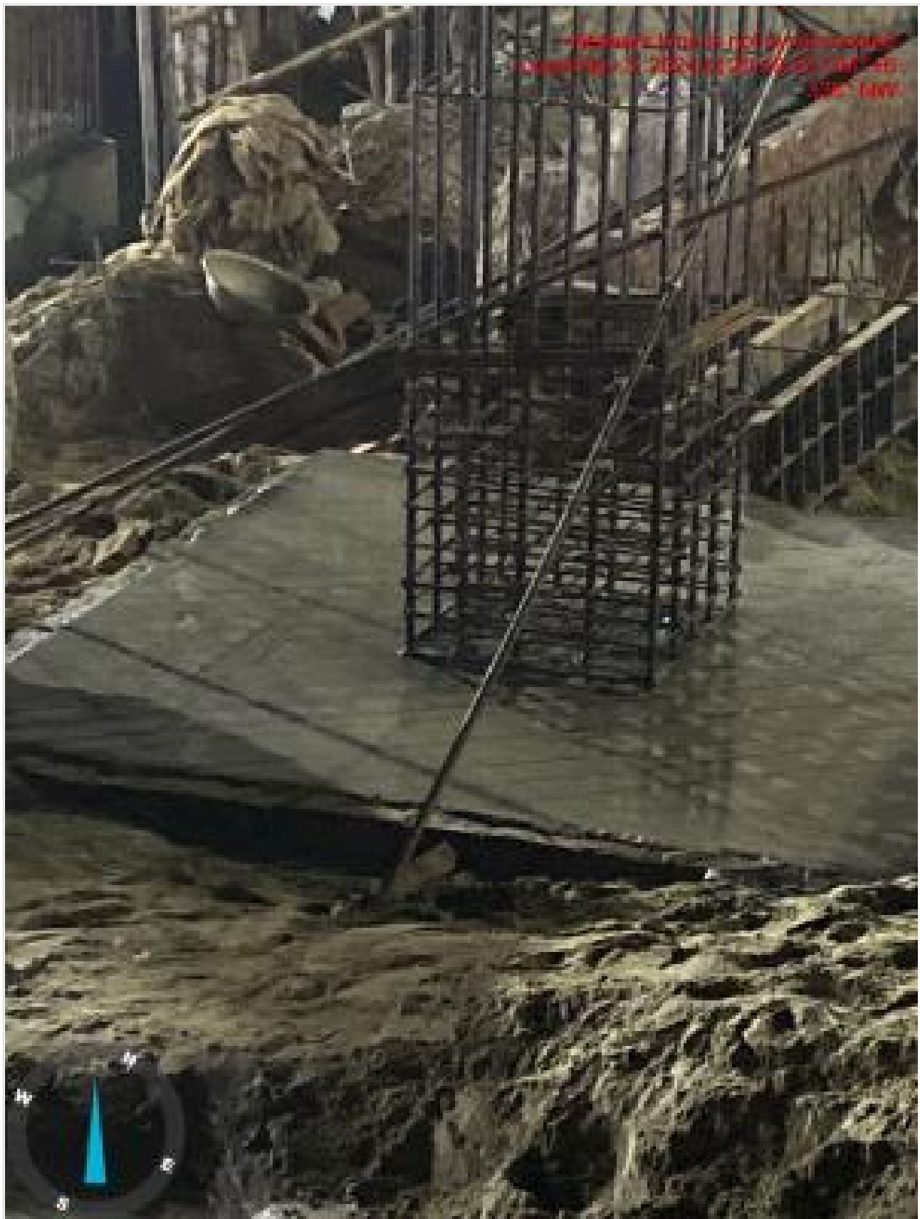
Pile cap concreting on 03-11-24
