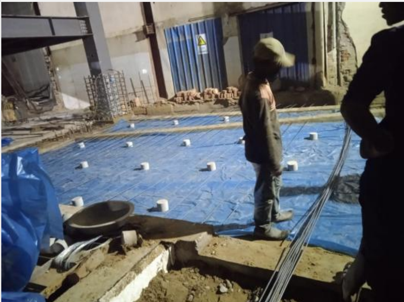
Polythene laying over sub-base on 31-12-24
