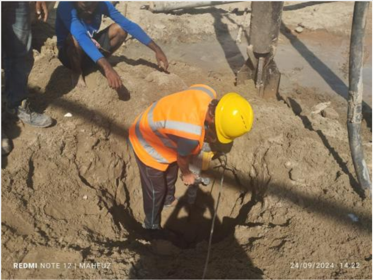
Boring obstacle Old CC breaking on 24-09-24
