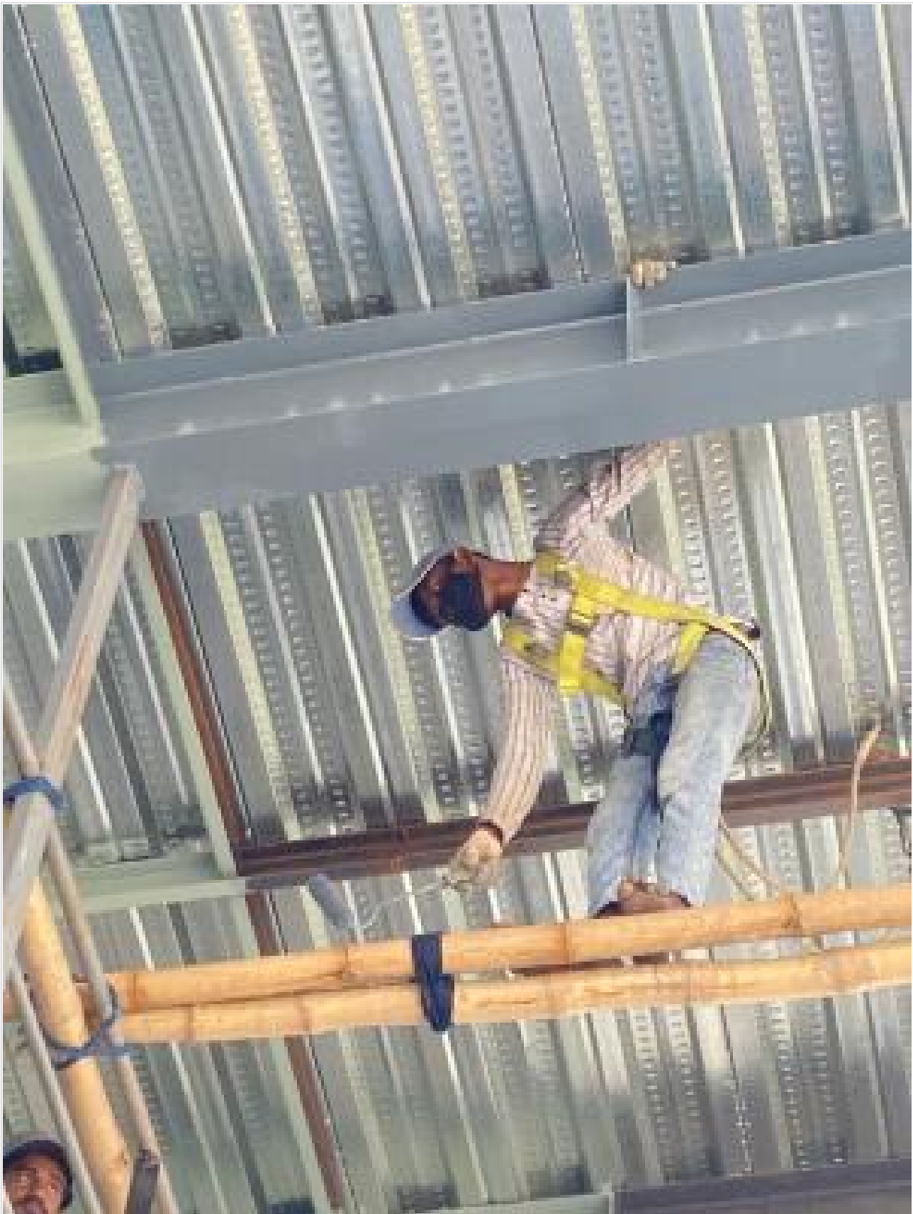
Steel Structure painting on 07-03-25
