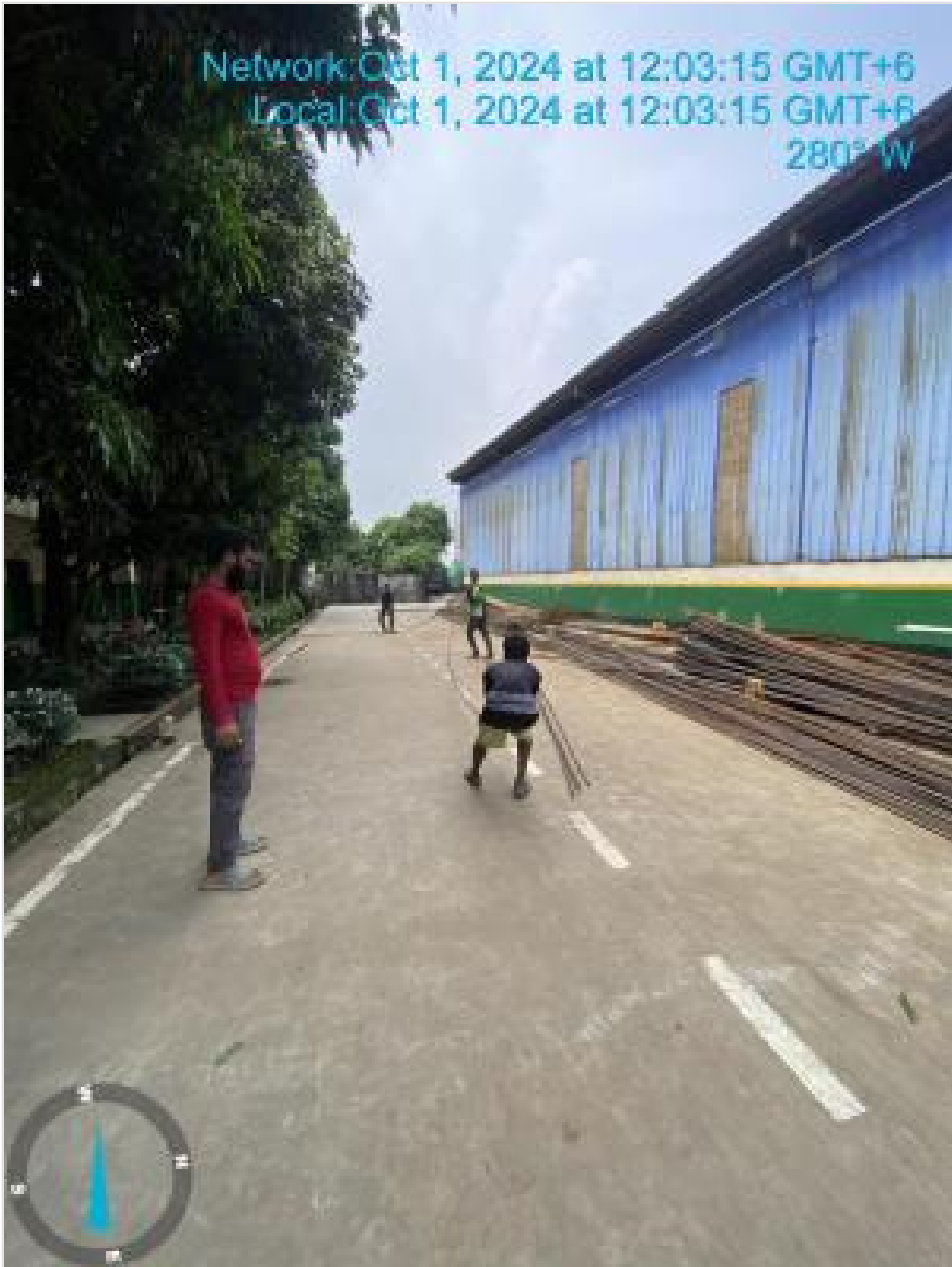
Re-bar straighting on 01-10-24
