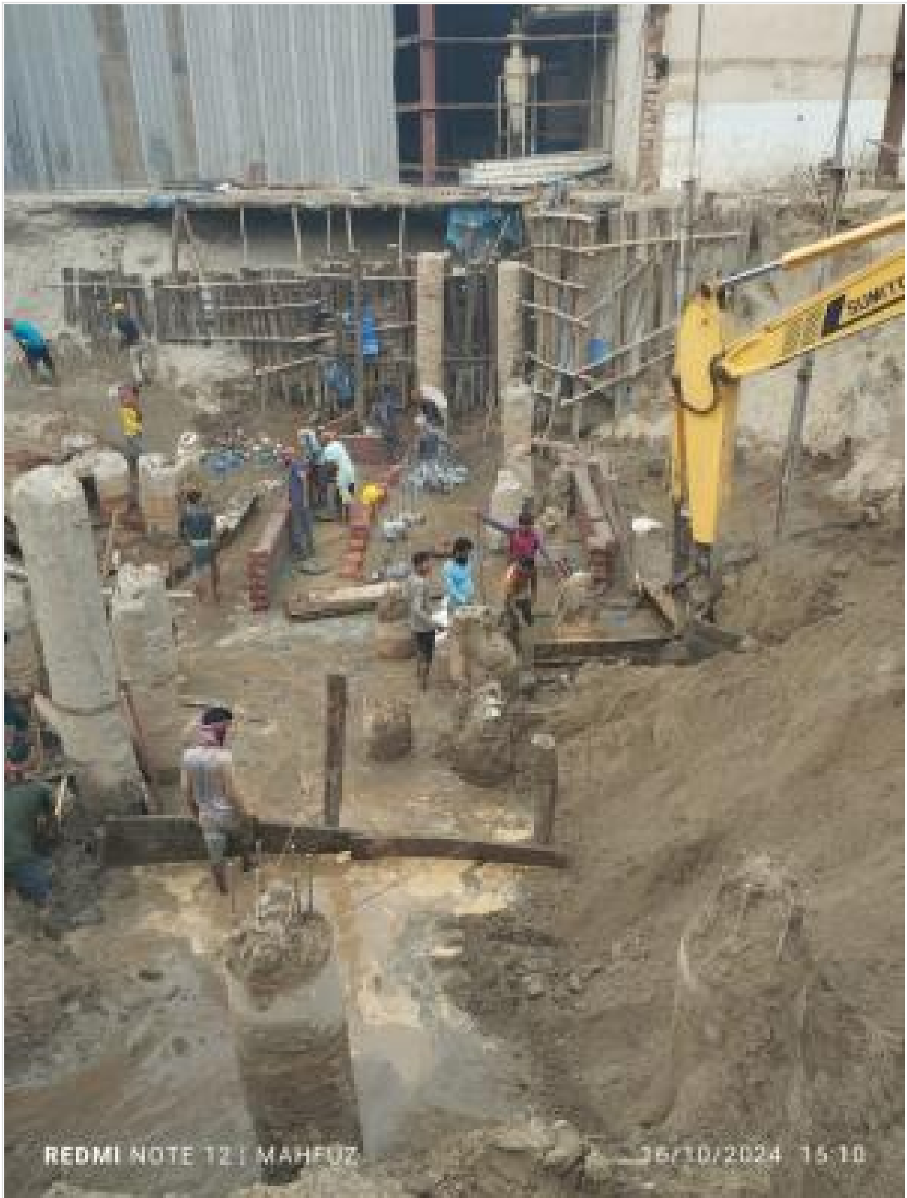
Excavation, brick-shuttering, steel shut on 16-10-24
