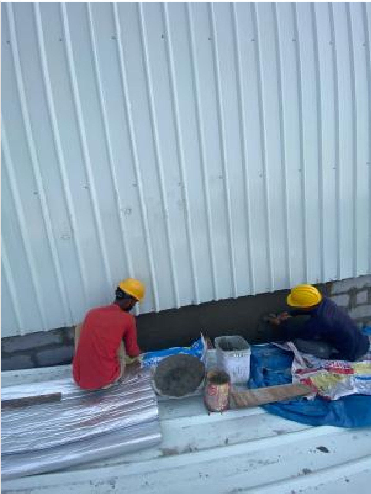
Exterior wall plastering on 05-03-25
