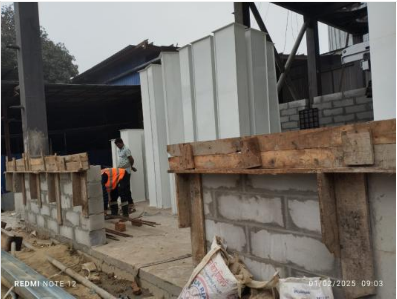
Copping wood shuttering on 01-02-25
