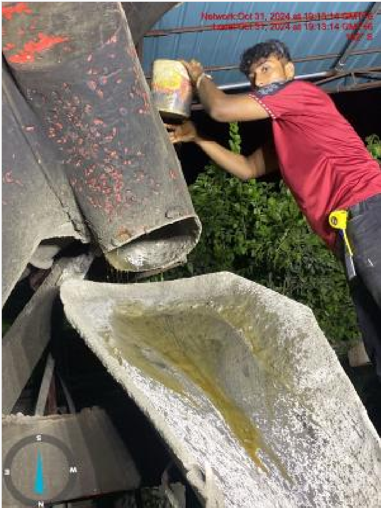
Water proofing admixture adding in concr on 31-10-24
