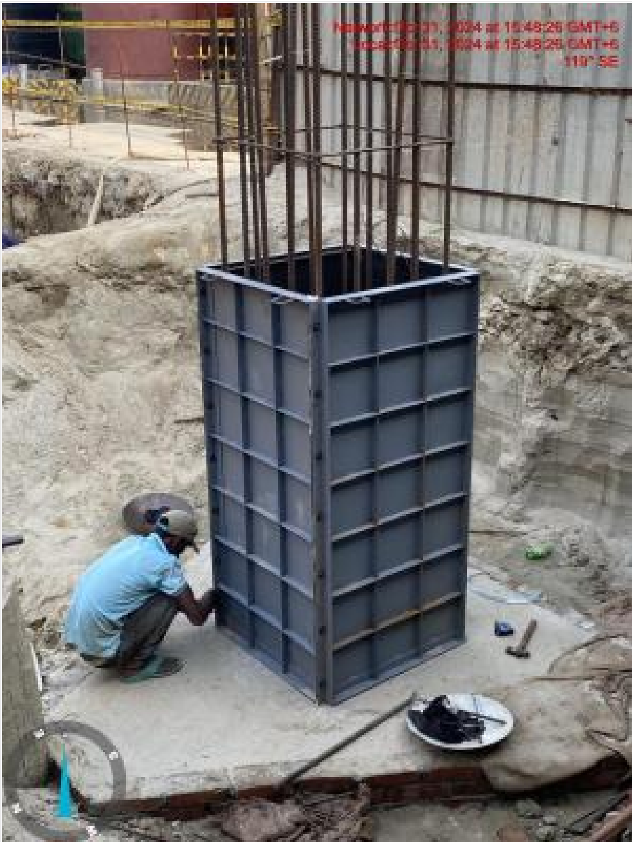
Column Shuttering on 31-10-24
