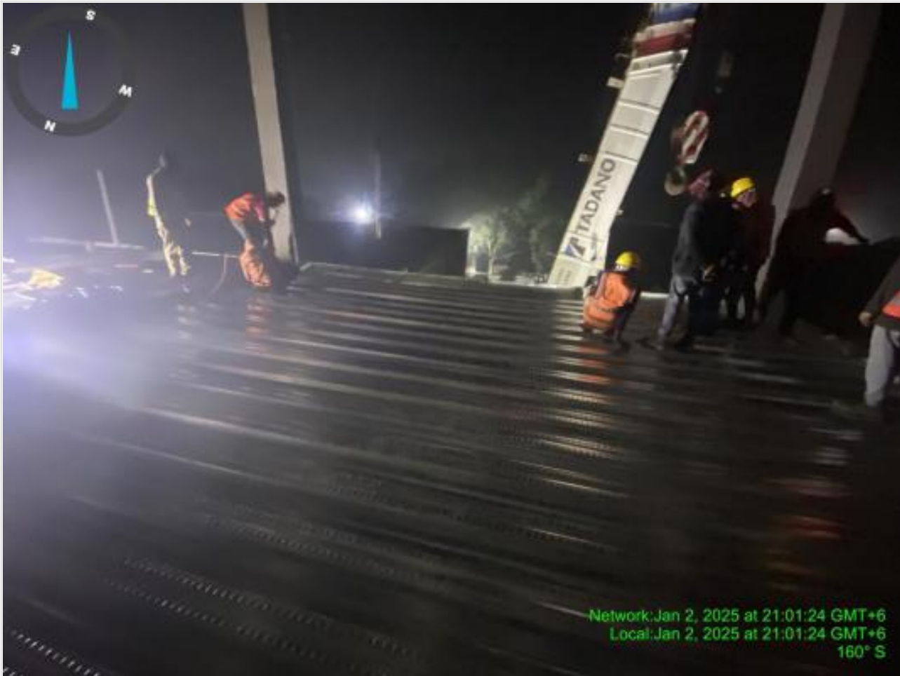
Decking Slab Fixing on 02-01-25
