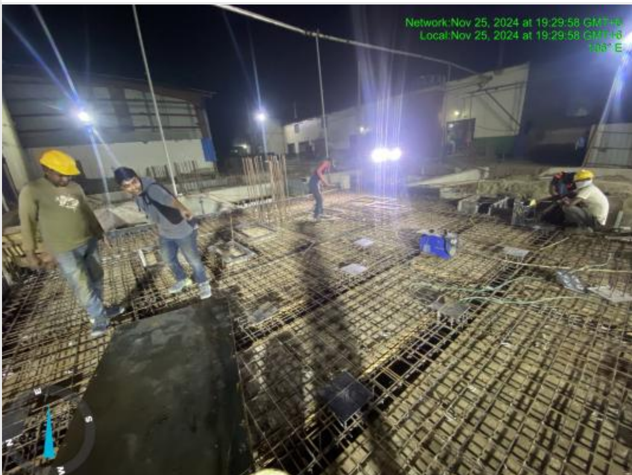
Embedded steel part fixing on 25-11-24
