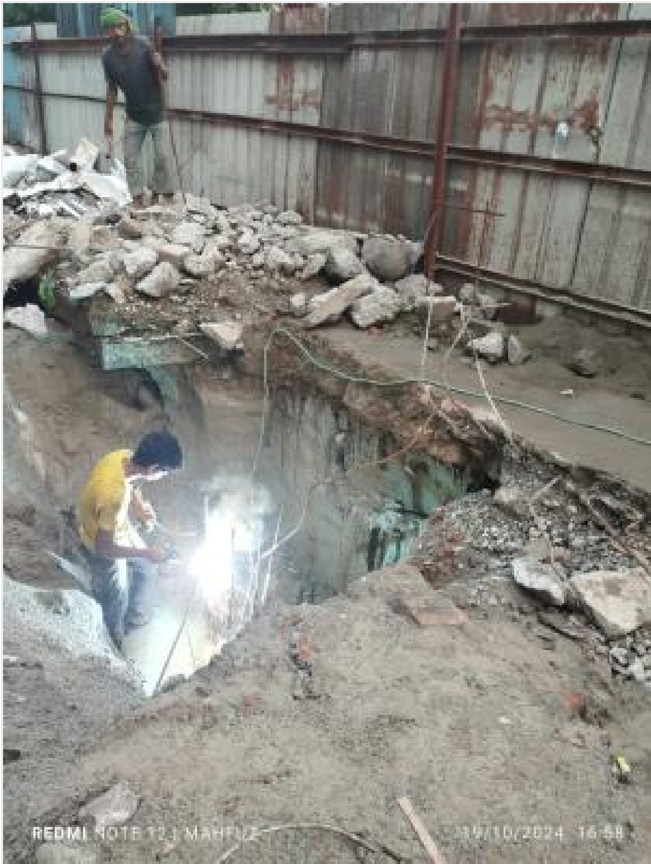
Pile Head Breaking on 19-10-24
