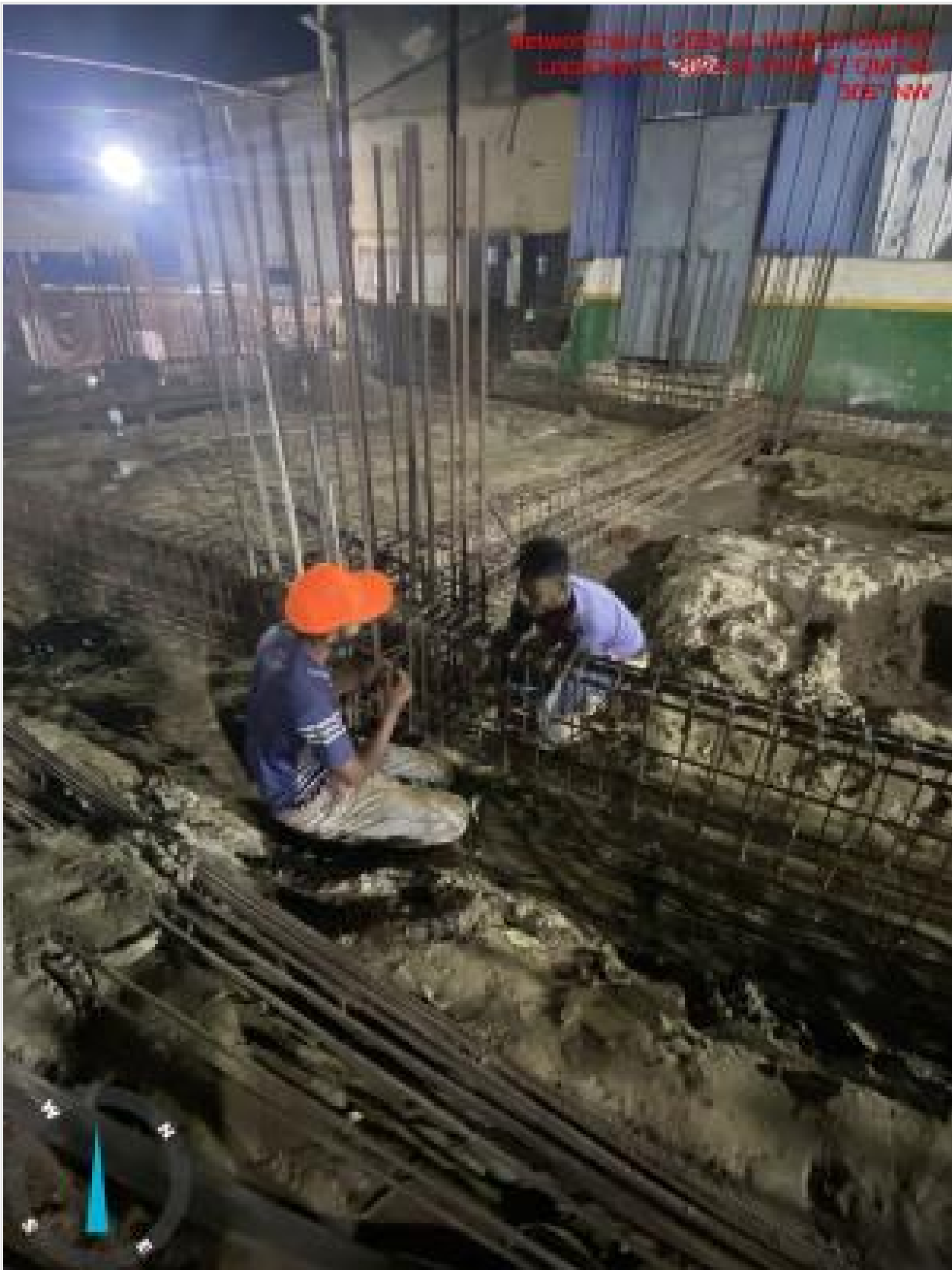
Foundation beam rebar work on 08-11-24
