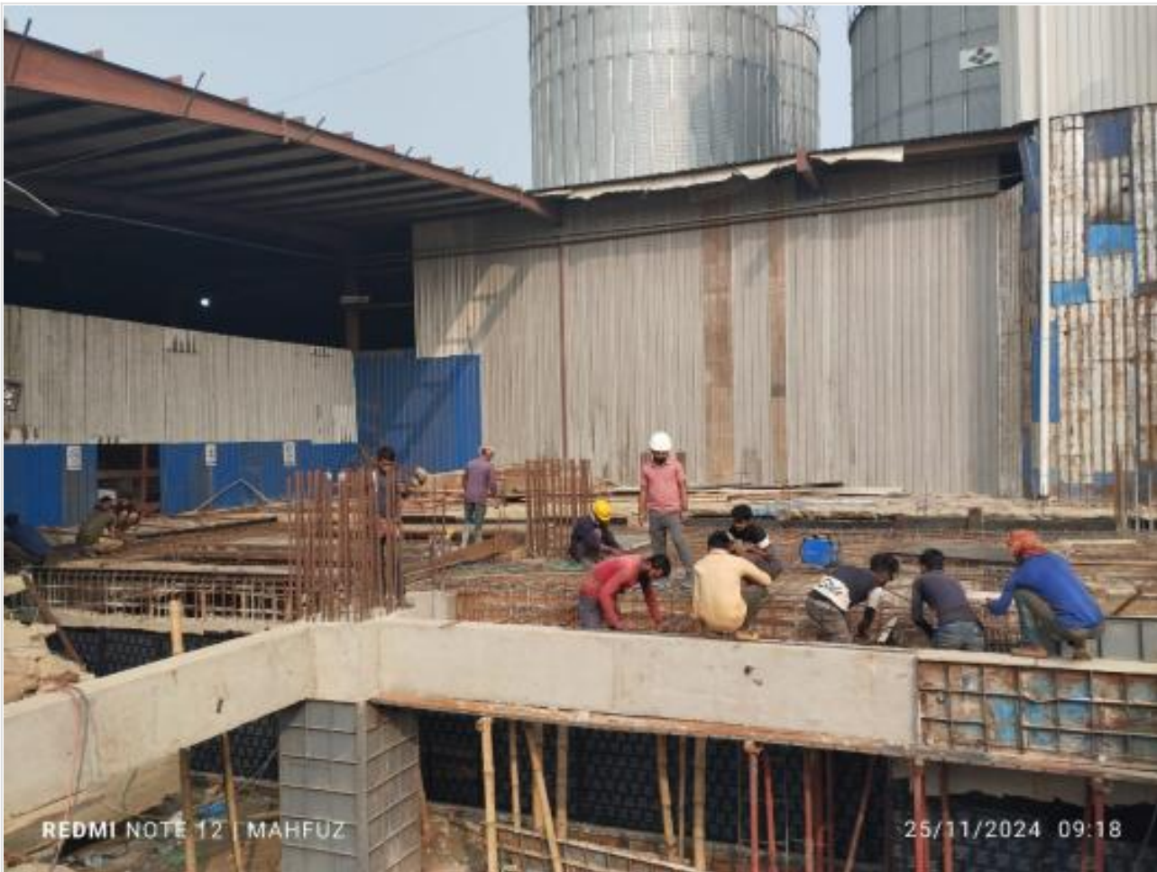
Tank Slab Re-bar work on 25-11-24
