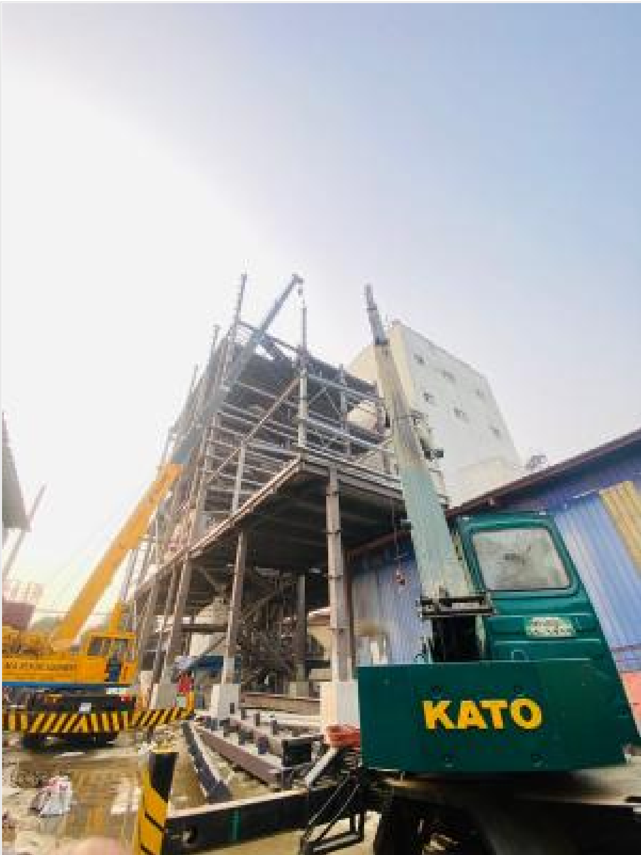
5th floor column installation on 25-01-25
