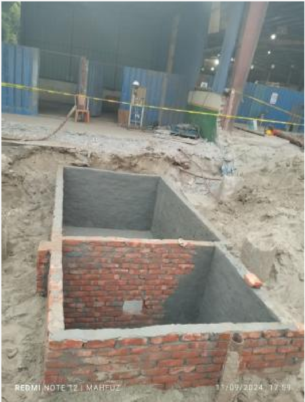
Pile mud tank complete on 11-09-24
