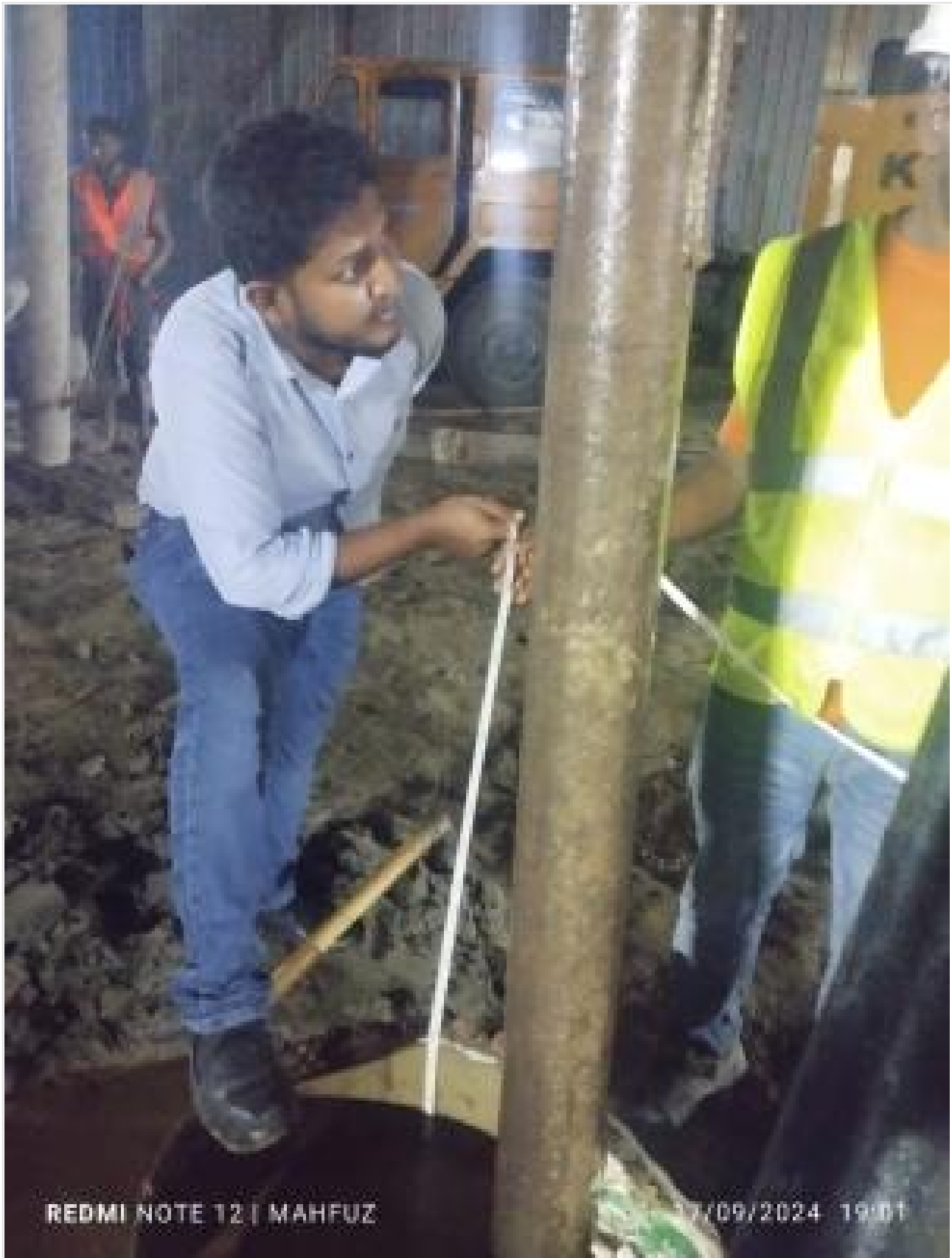
Pile boring length checking on 17-09-24
