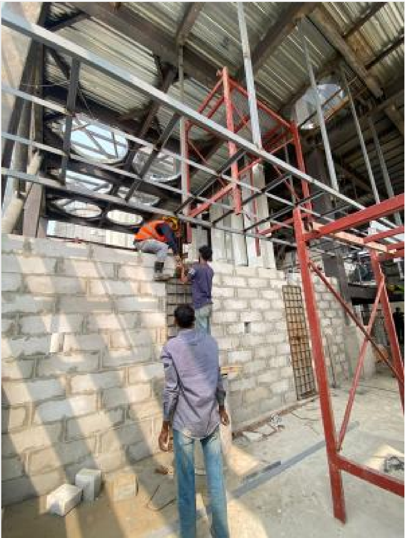
AAC block work on 03-02-25
