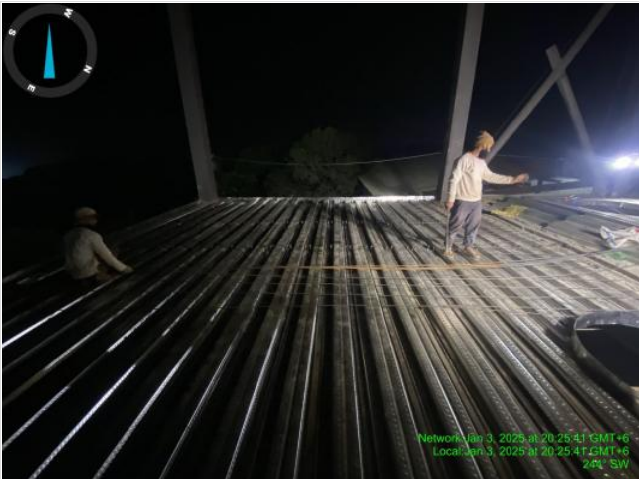
Re-bar Work on Decking Slab on 03-01-25
