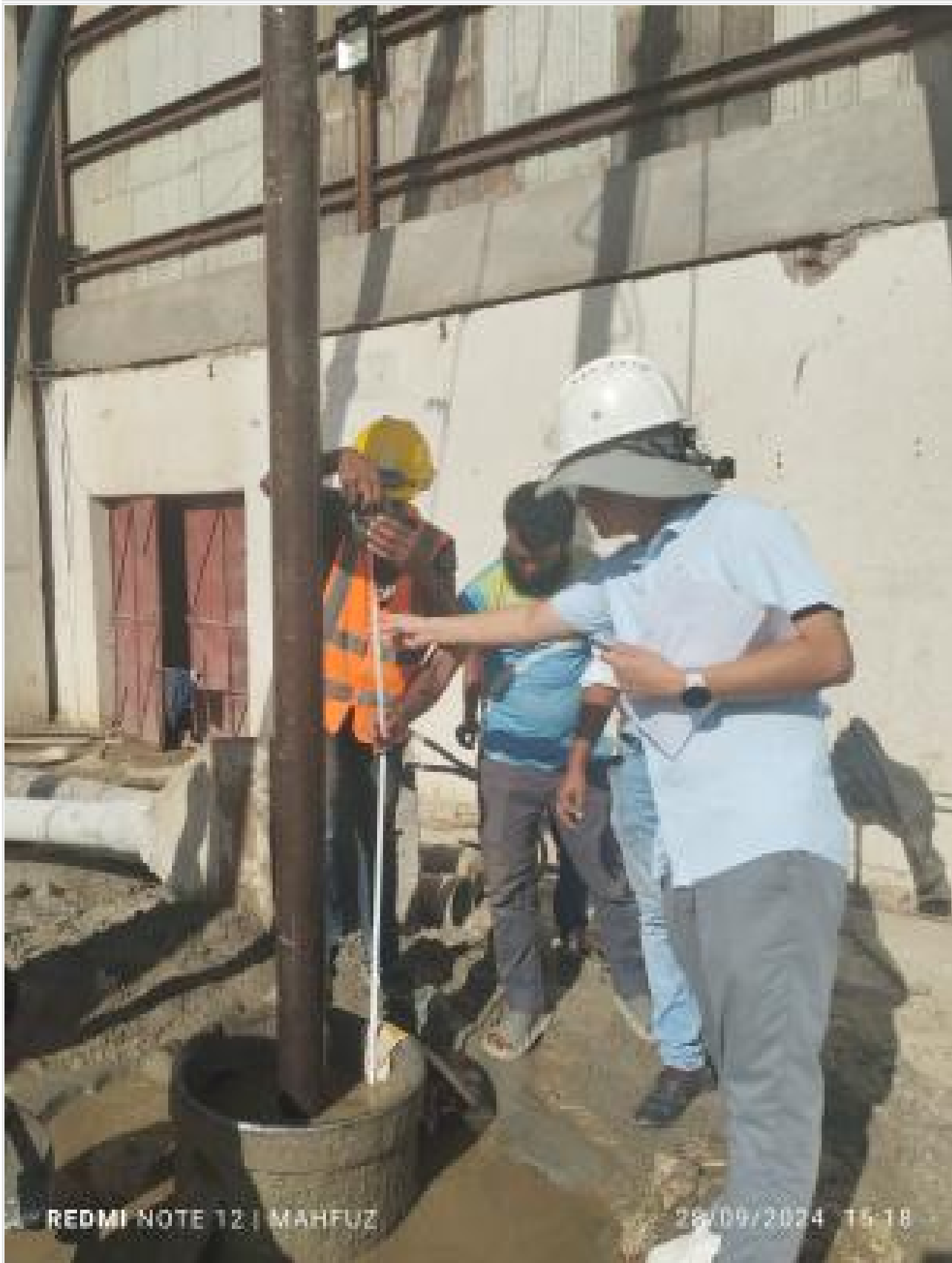
Pile boring depth checking on 28-09-24
