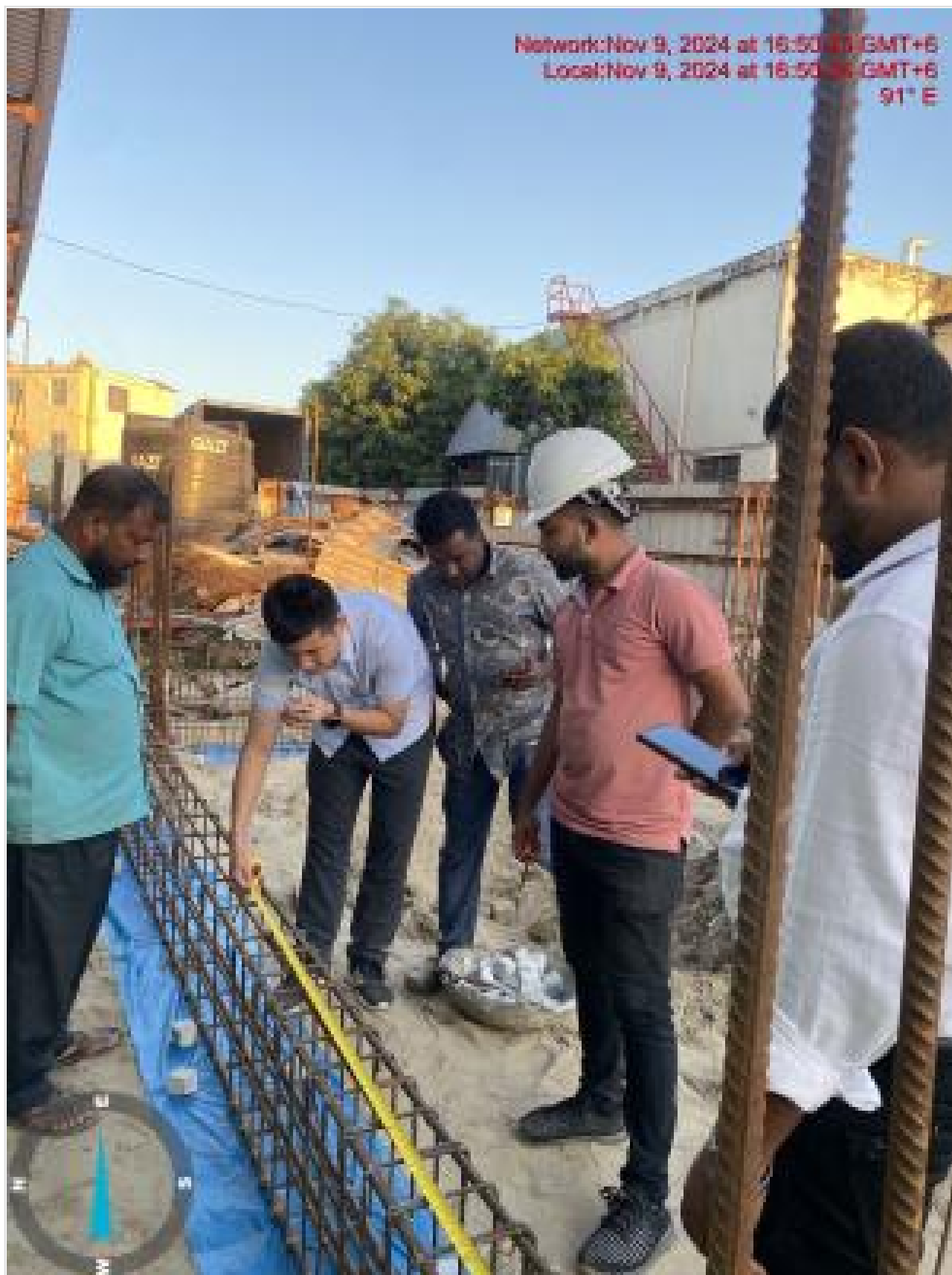
Foundation beam rebar inspection on 09-11-24
