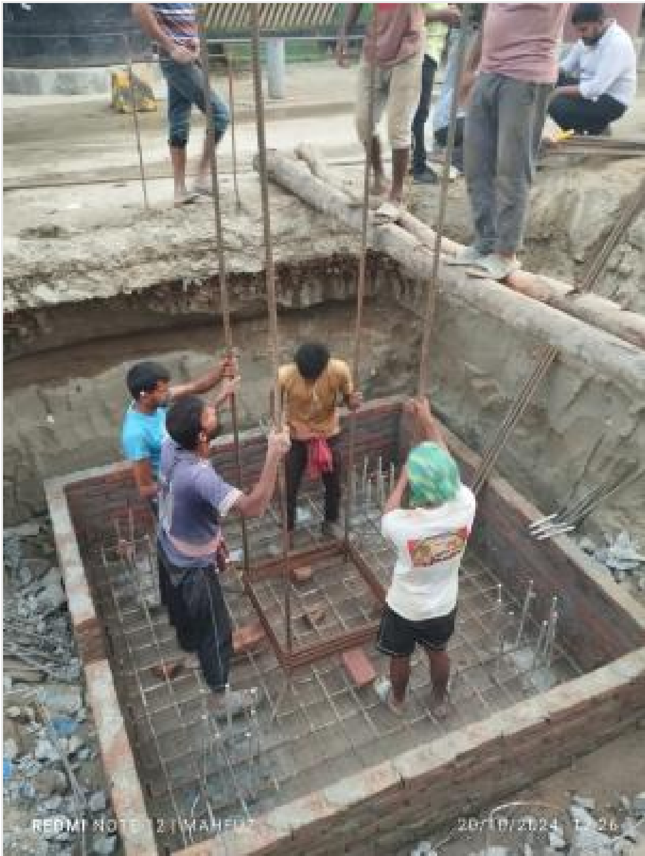
Pile cap re-bar work on 20-10-24
