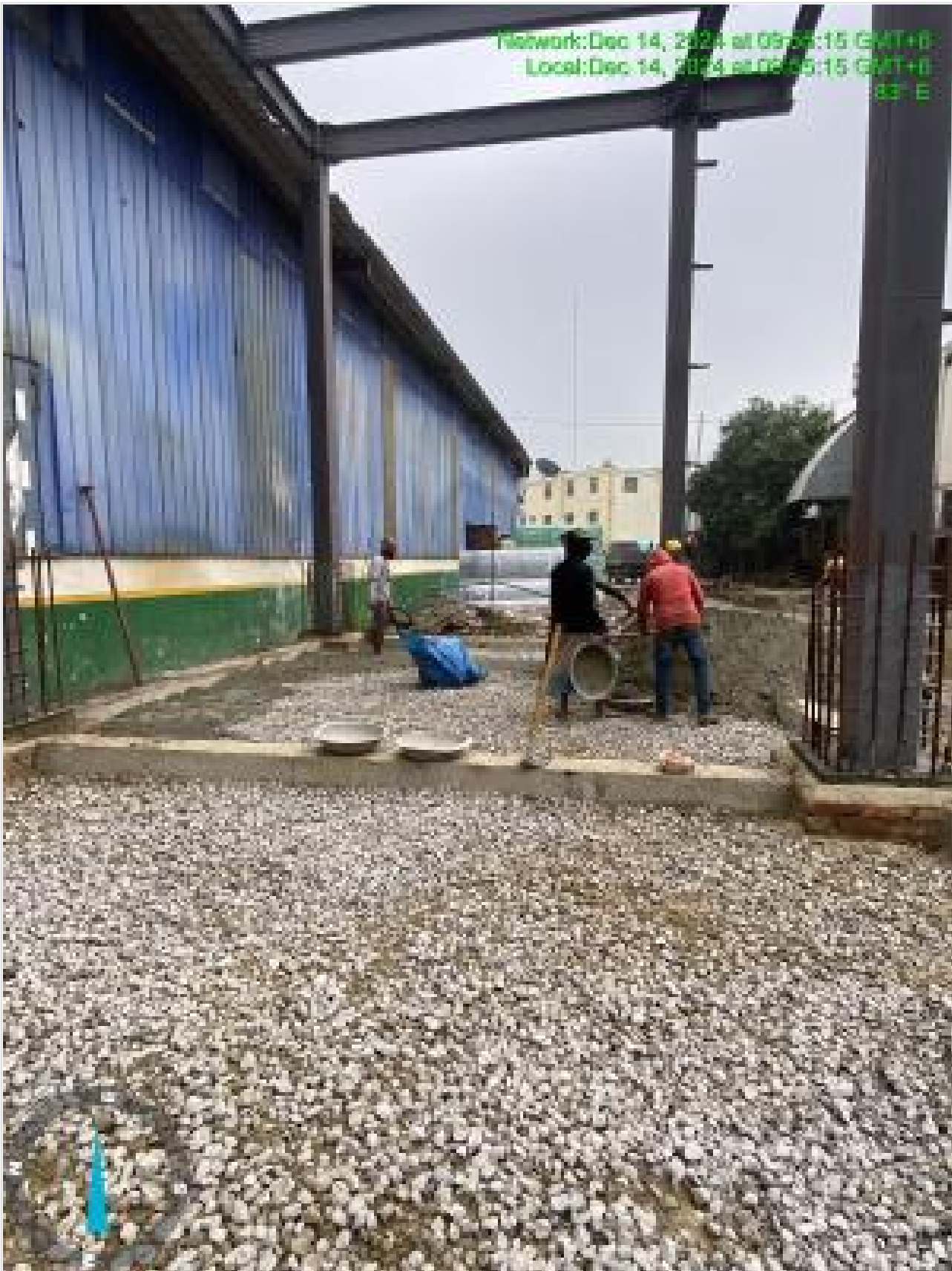
Sub-base work in floor on 14-12-24
