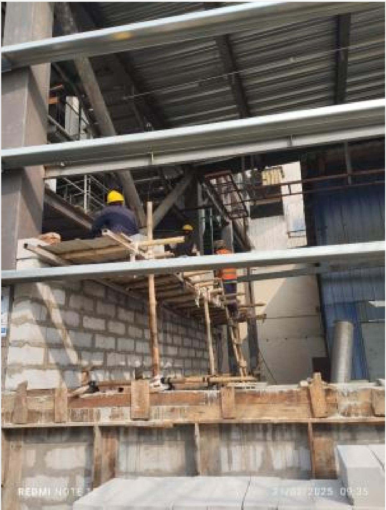
AAC block work on 21-02-25
