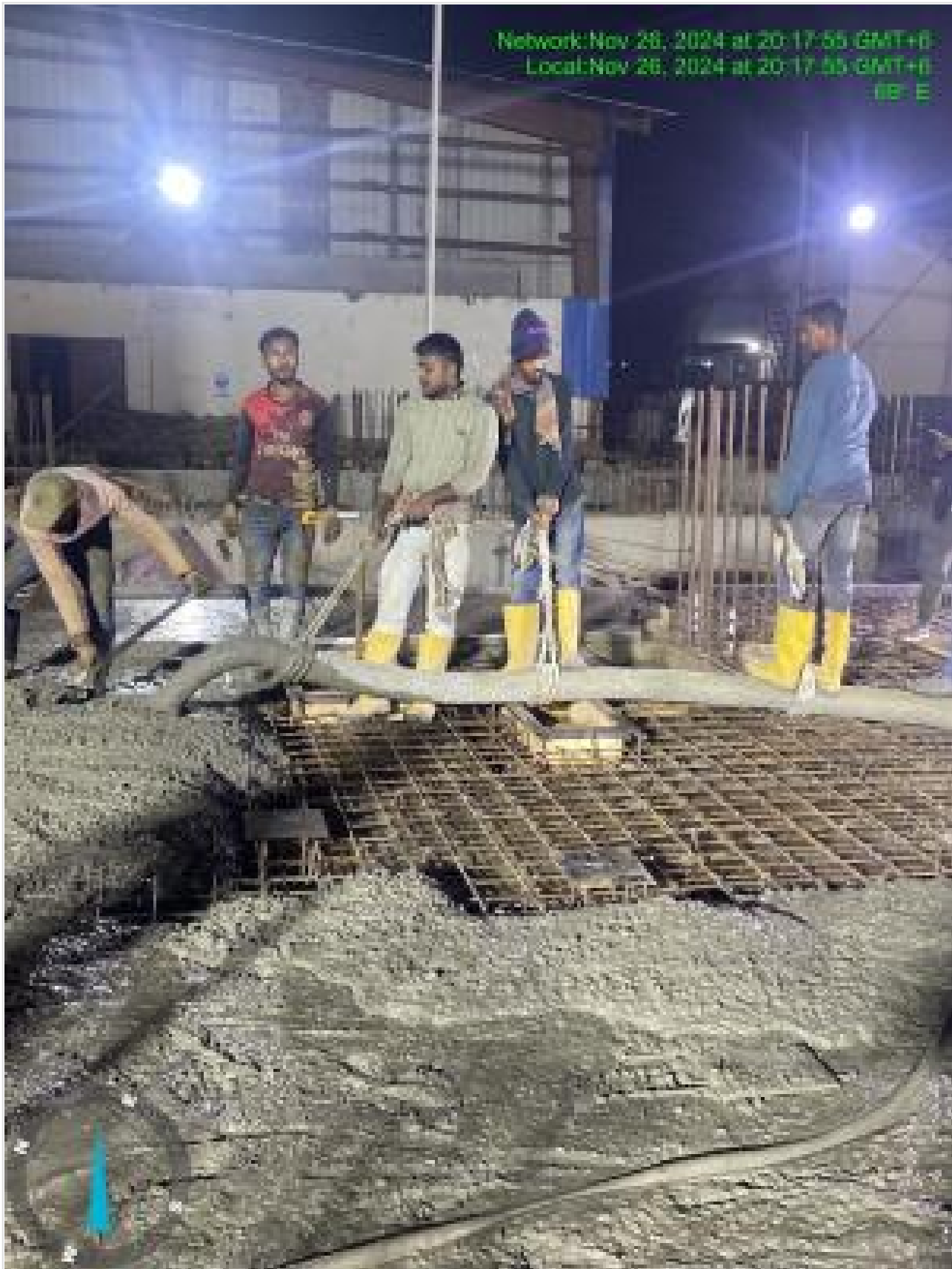
Tank slab concreting on 26-11-24
