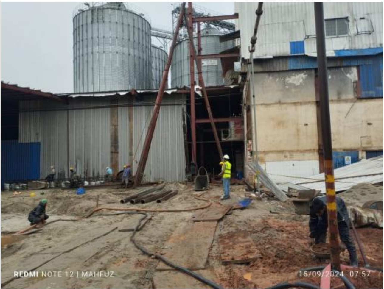
Pile boring on 15-09-24
