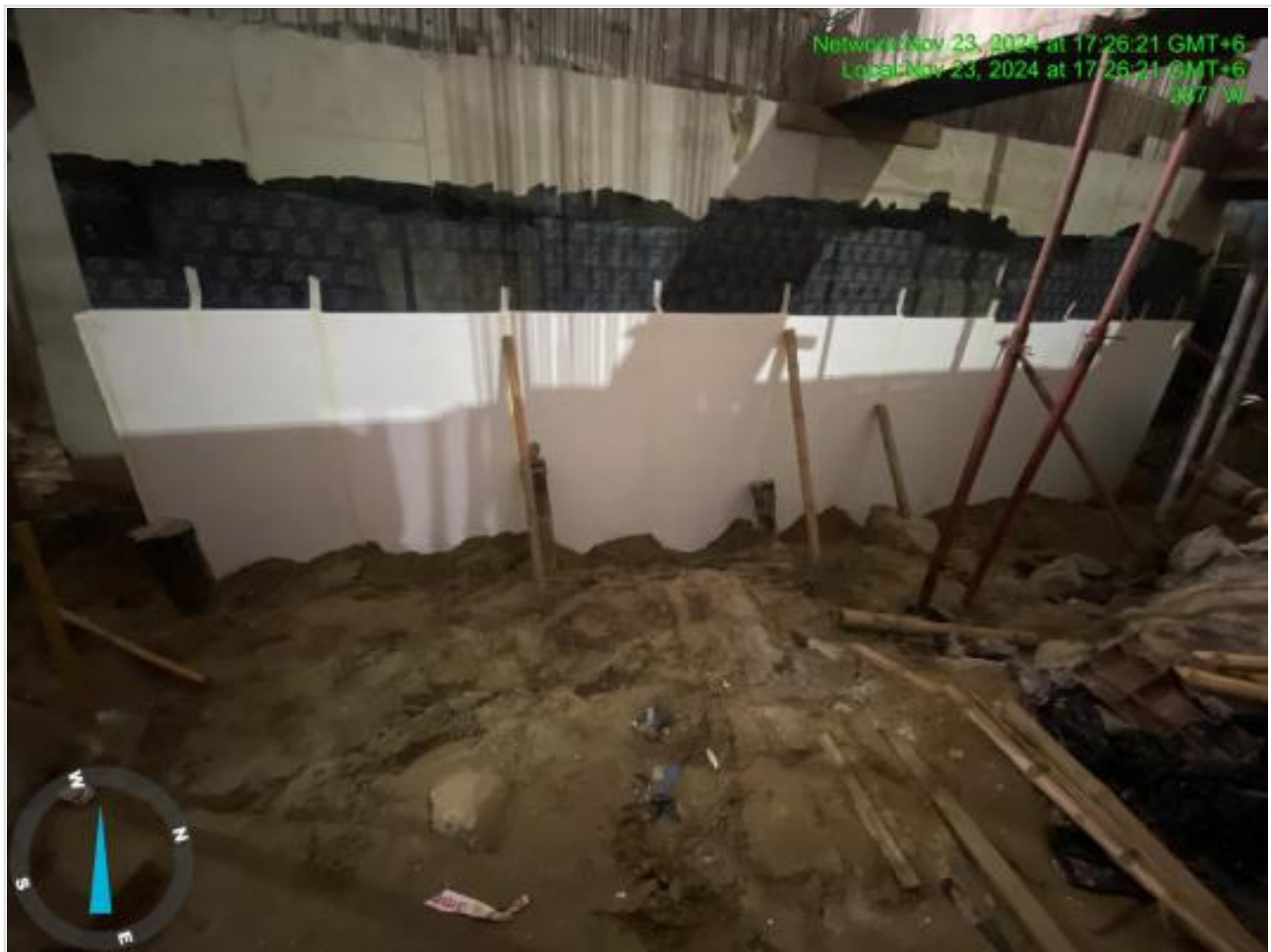
Tank wall stylo foam fixing on 23-11-24
