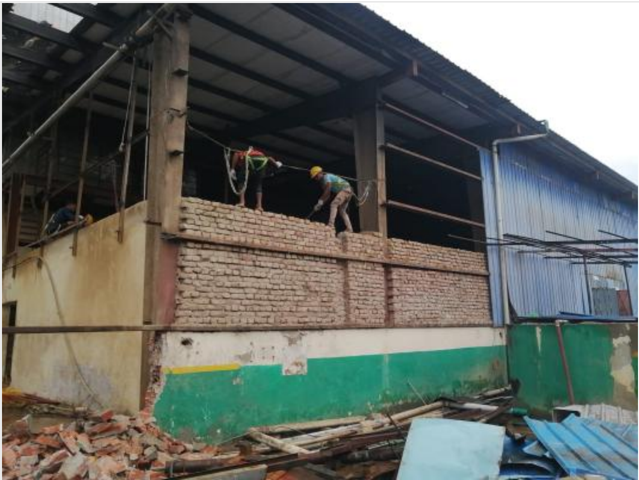
Brick wall dismantling on 03-09-24
