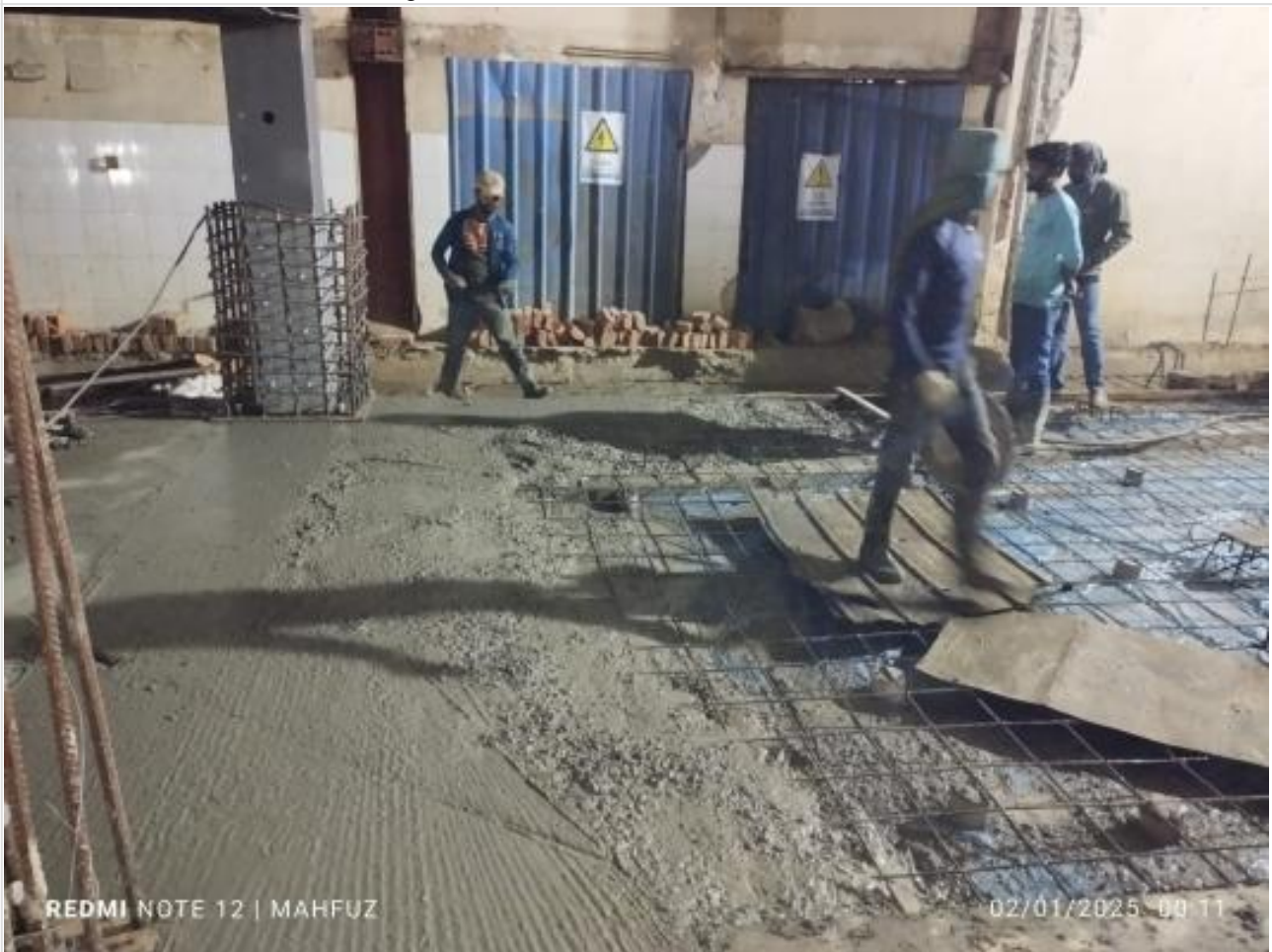
Ground Floor RCC Slab Concreting on 01-01-25
