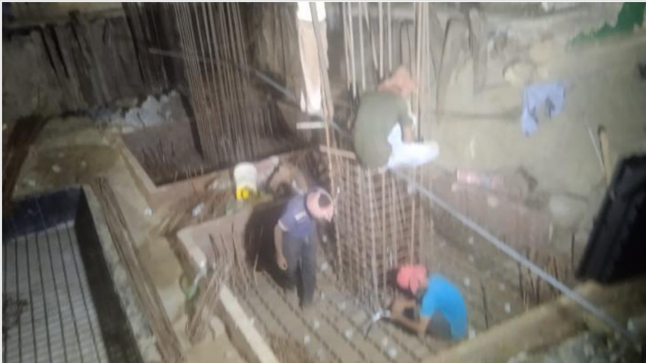
Raft re-bar work on 30-10-24
