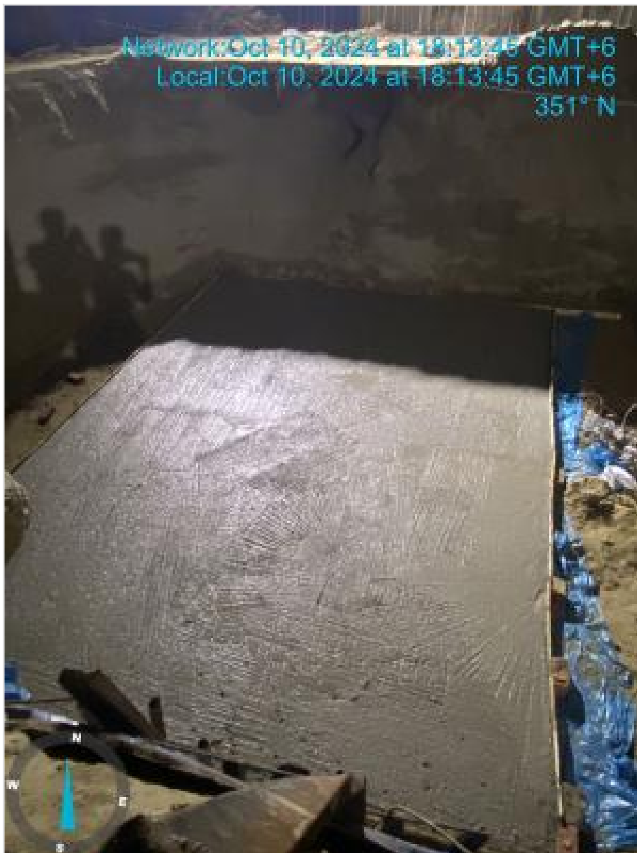
Water Reservoir Base CC-Bottom on 10-10-24
