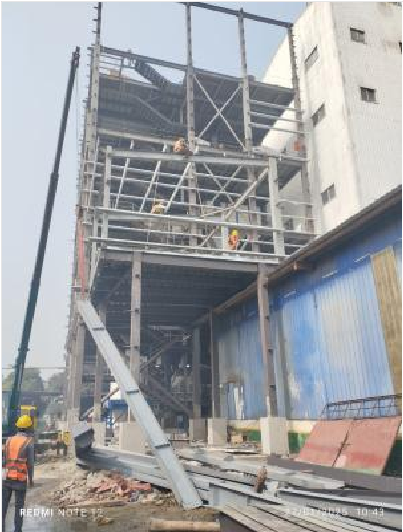
5th Floor Steel structure installation on 27-01-25
