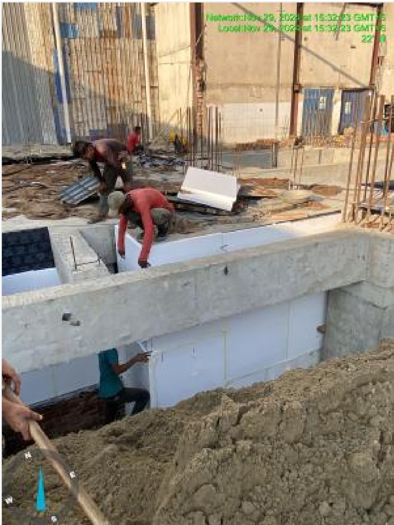
Cork sheet fixing in Tank wall on 29-11-24
