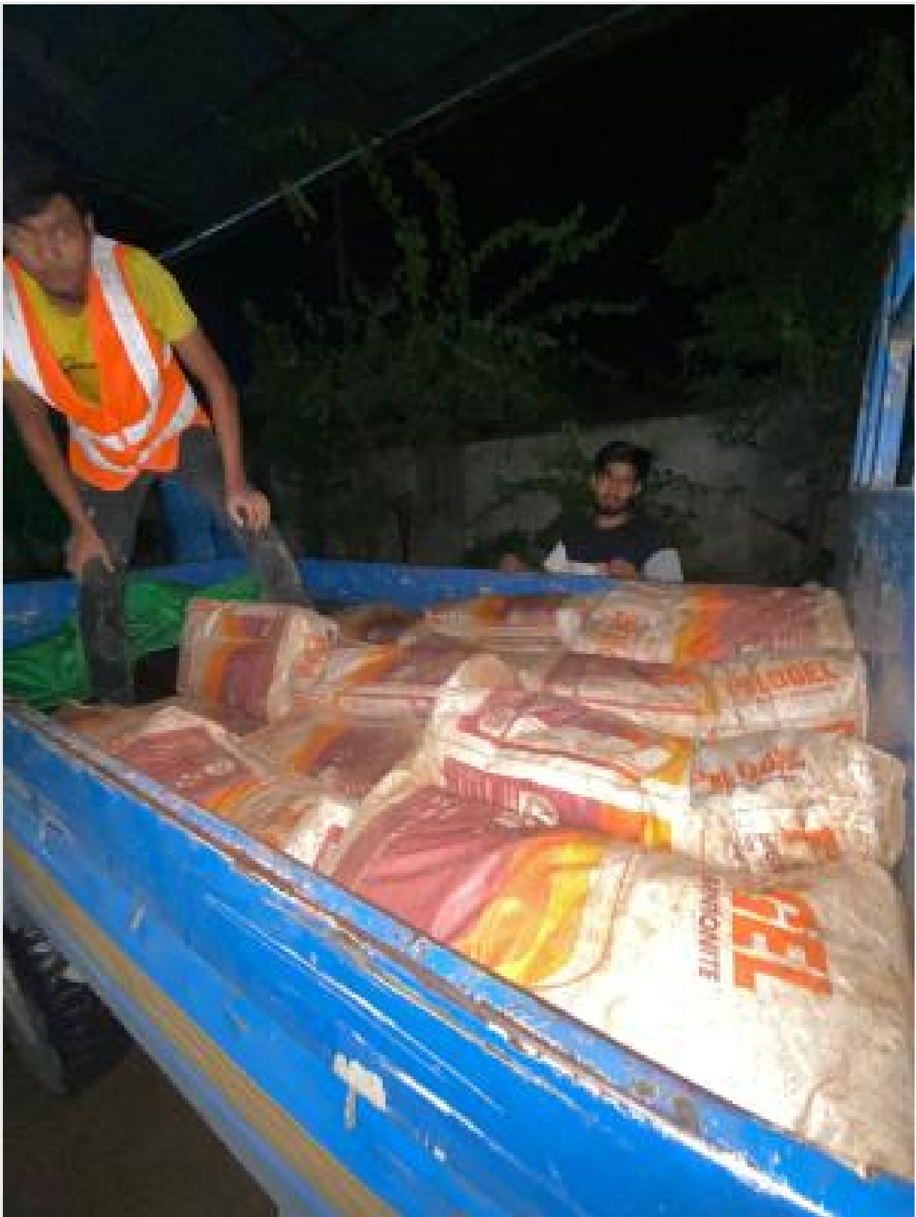
Bentonite received for pile boring on 26-09-24
