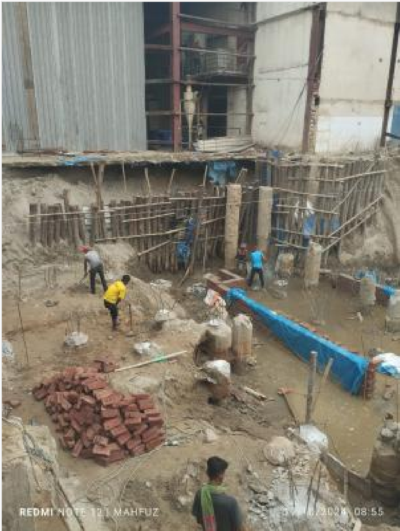
Pile head breaking on 17-10-24
