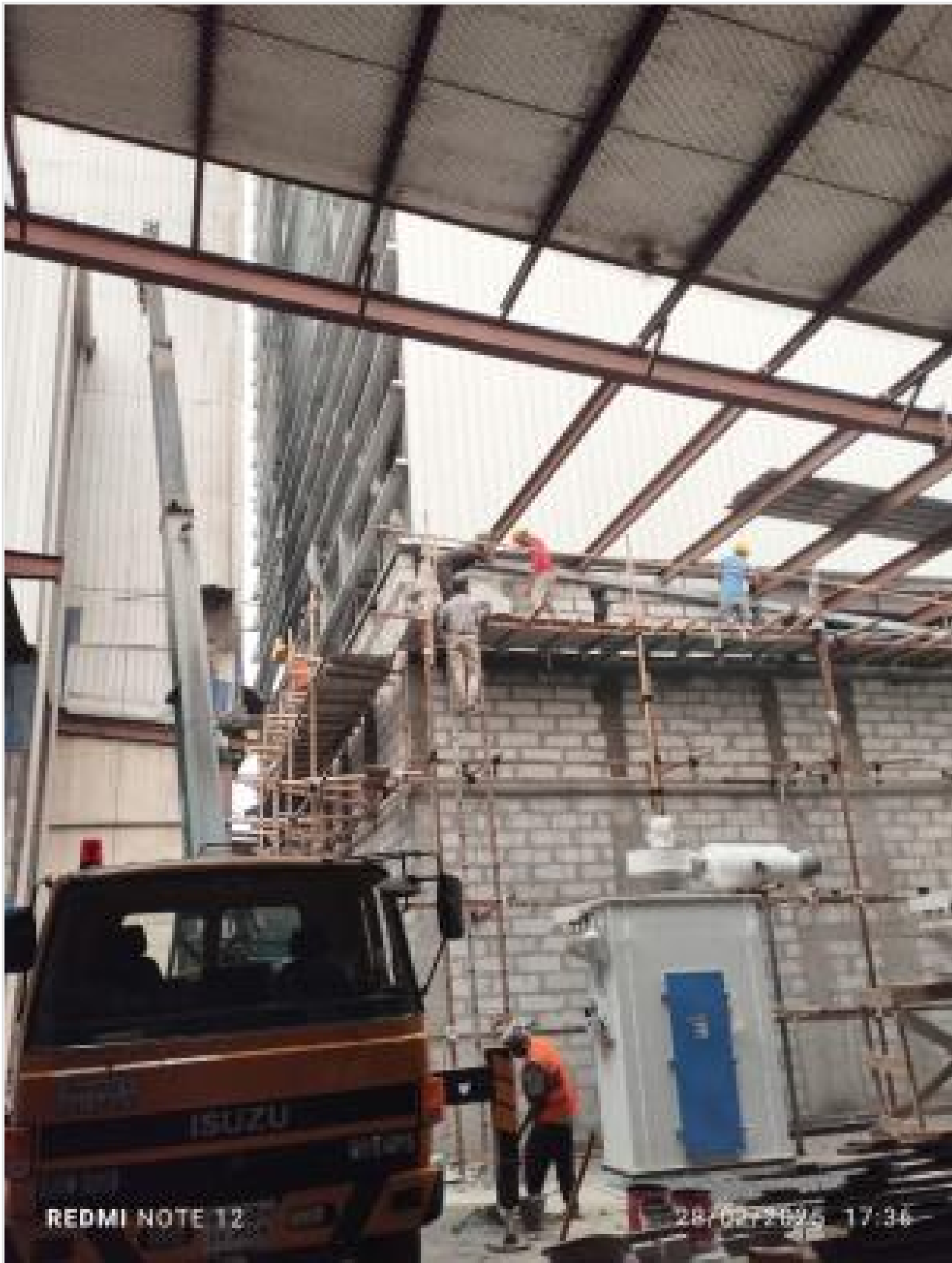
AAC block work on 28-02-25
