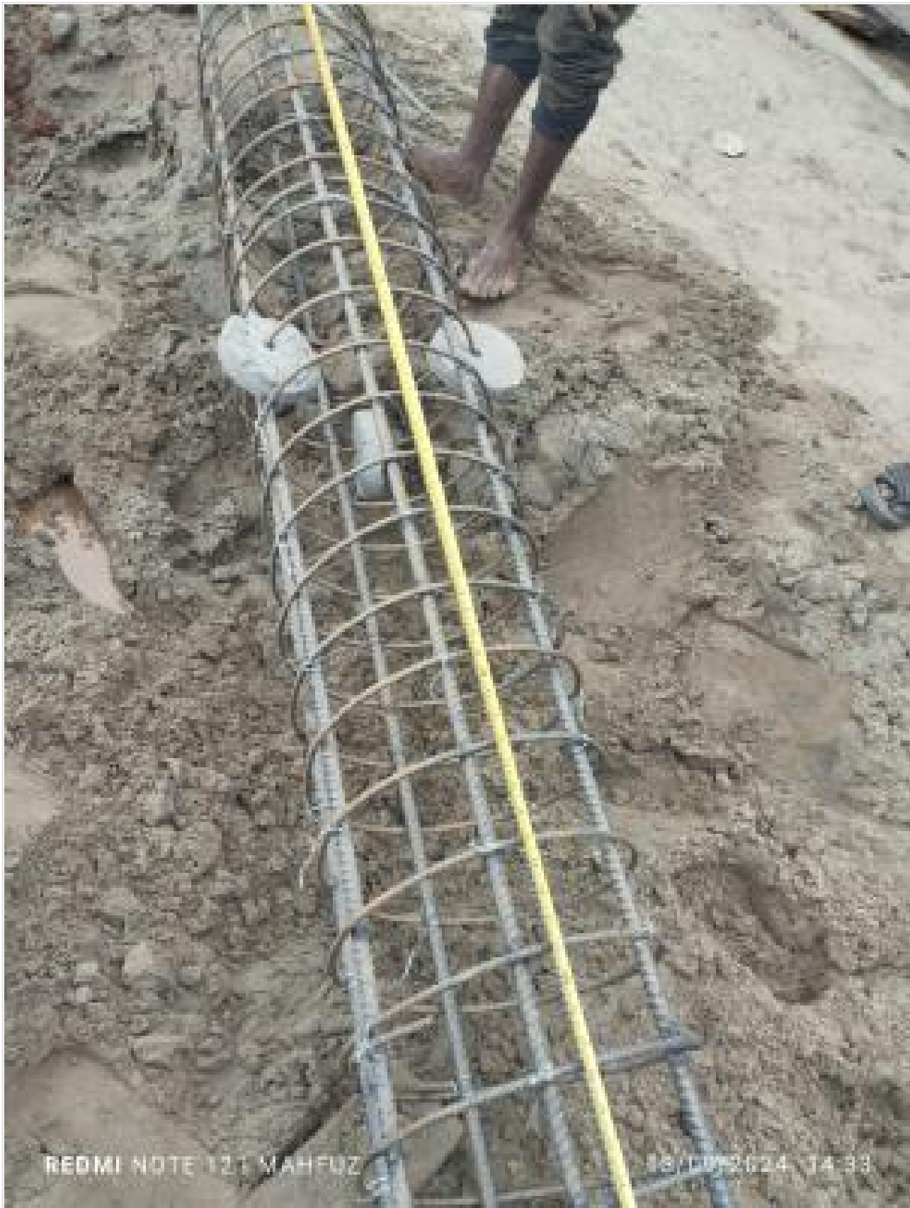
Pile cage length measuring on 13-09-24
