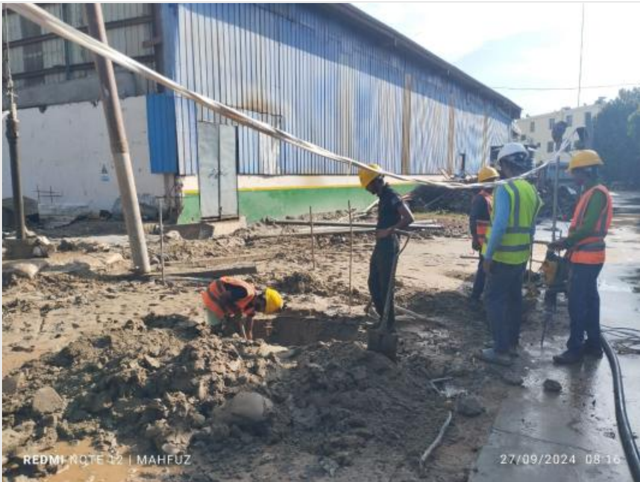
Excavating for pile boring obstacles on 27-09-24
