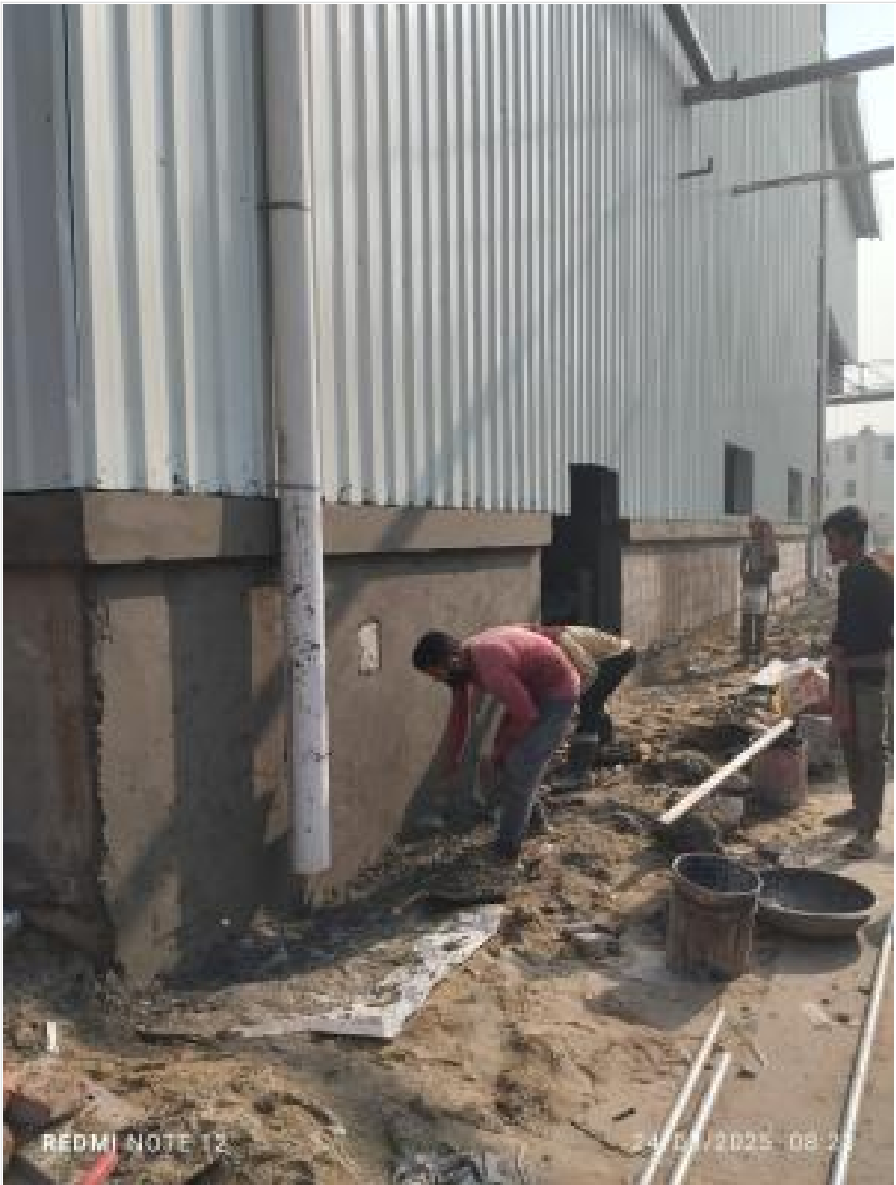
Exterior wall plastering on 24-03-25
