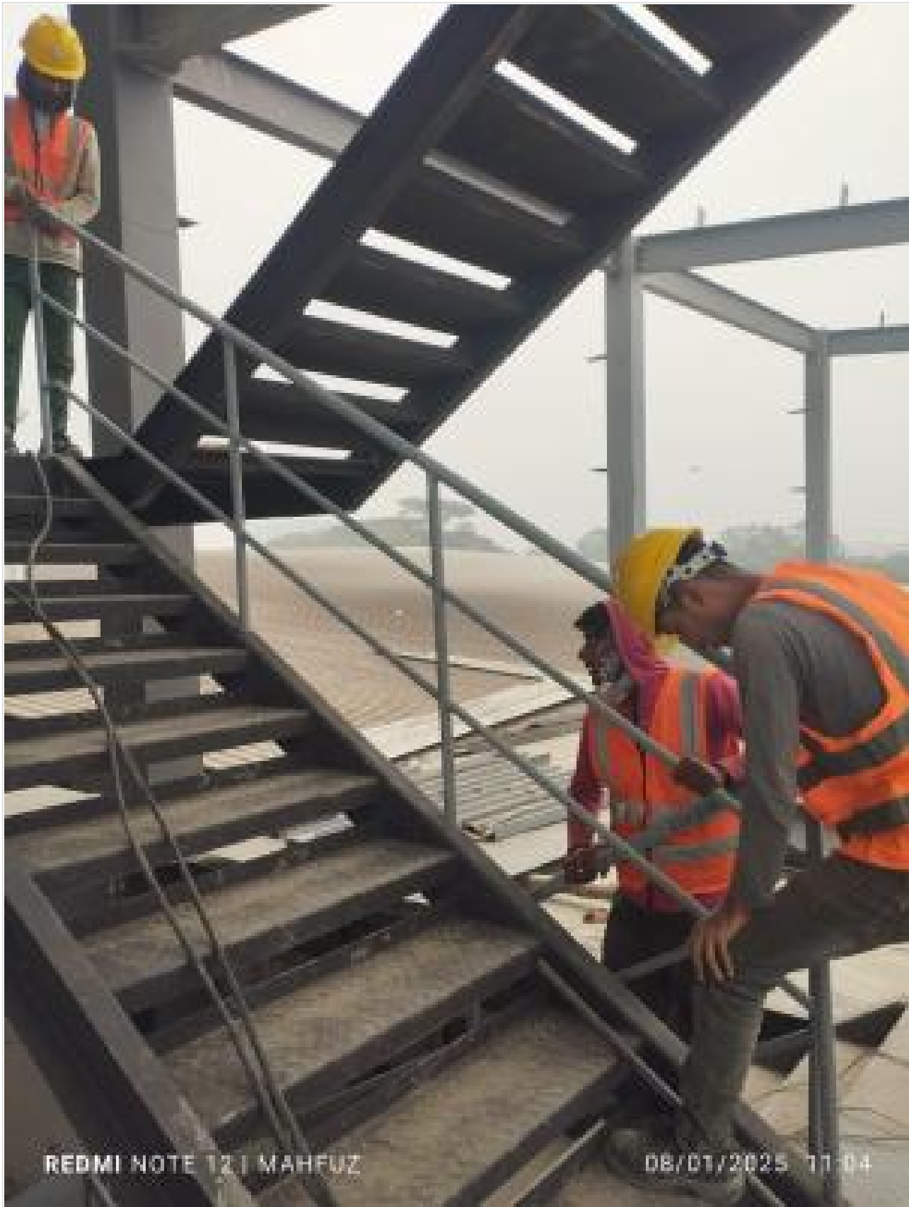
Stair case installation on 08-01-25
