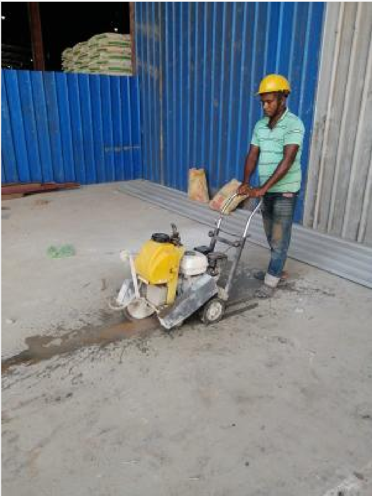
Floor cutting on 02-09-24
