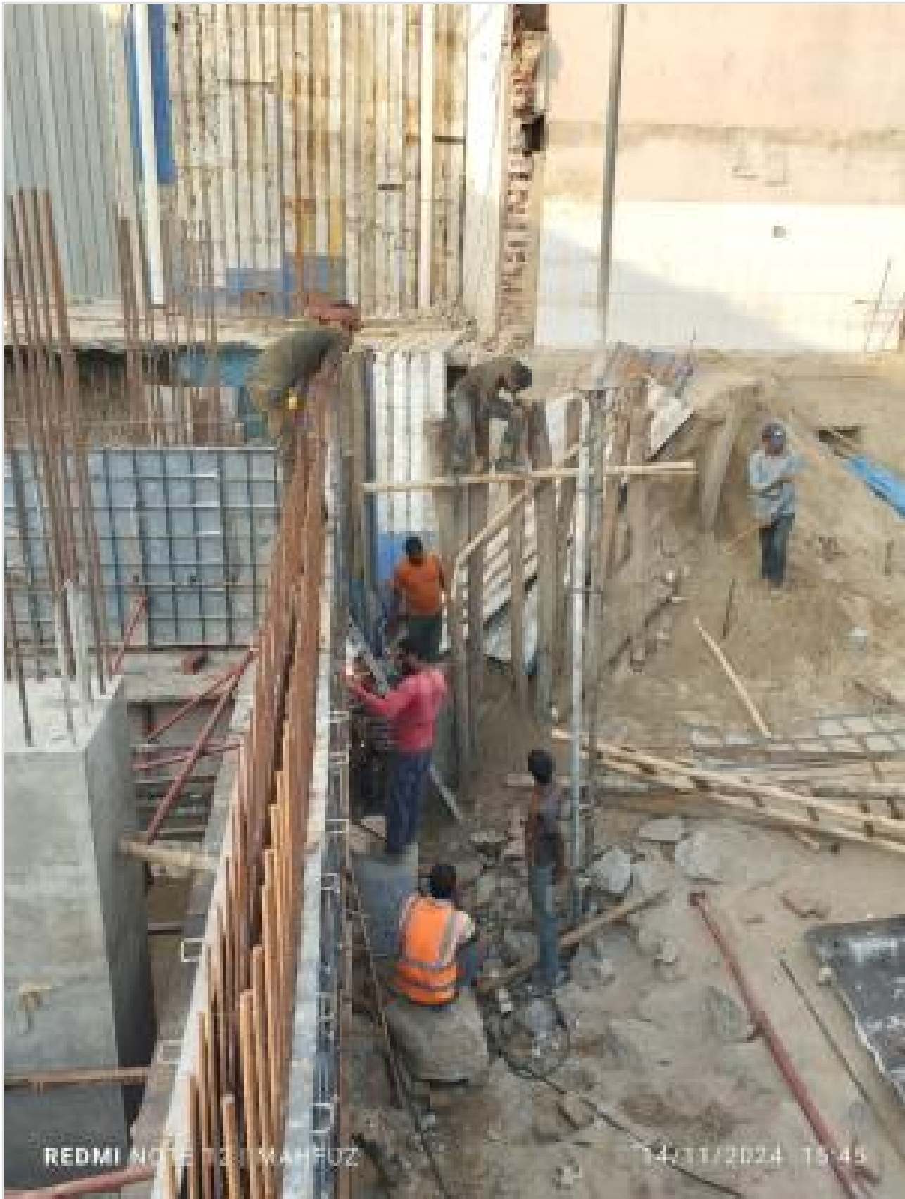
Wall shuttering on 14-11-24
