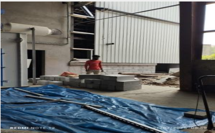
Interior AAC block work on 26-03-25 Site sheeting on 26-03-25
