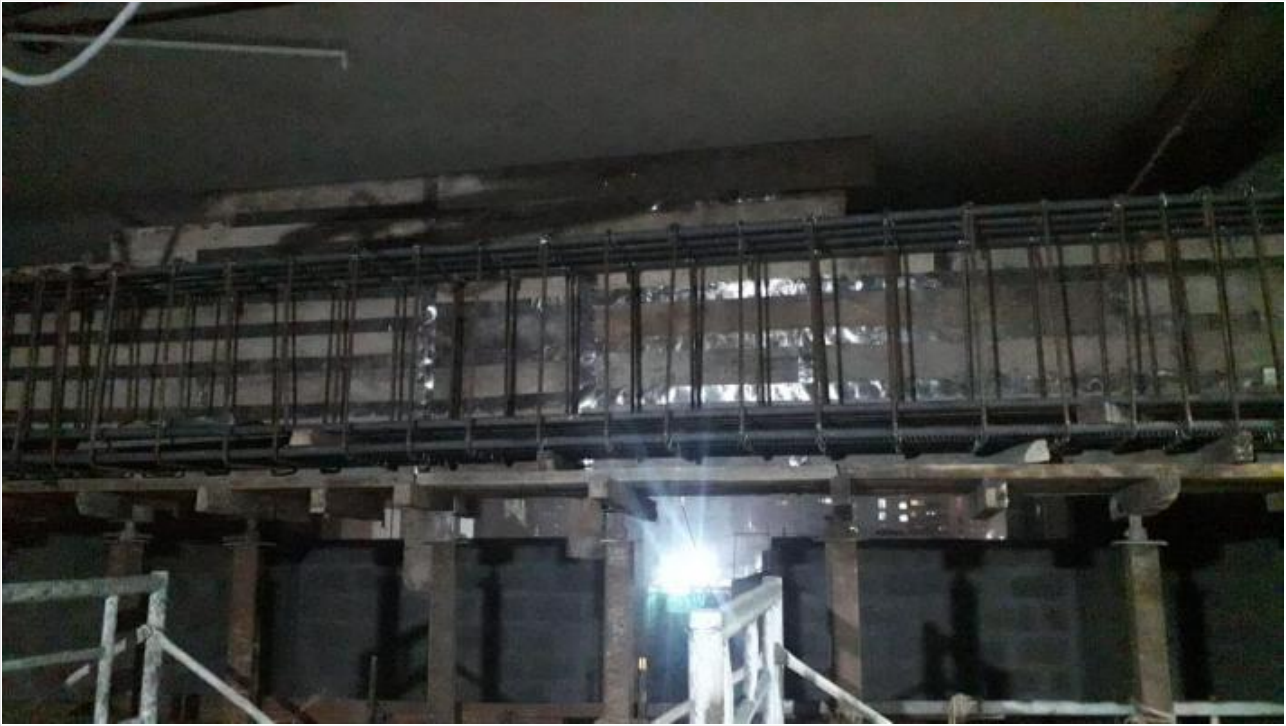
8F-Car Lift Beam Re-bar Work on 15-12-20
