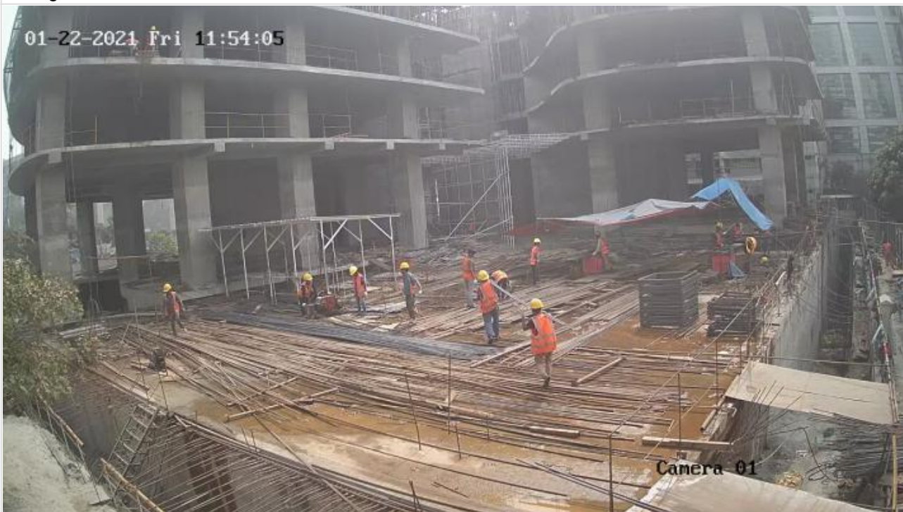
Re-bar Work on 22-01-21
