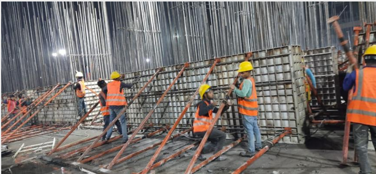
Lift Core Wall Shoring on 14-01-21
