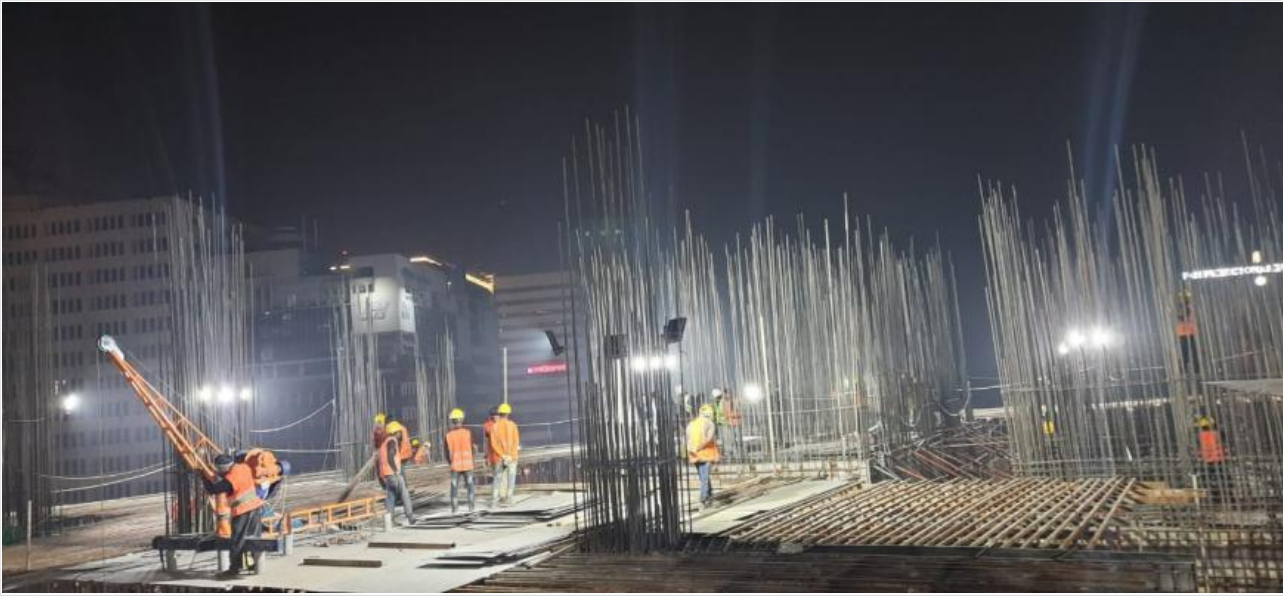
Re-bar Lifting by Roof Hoist on 14-01-21
