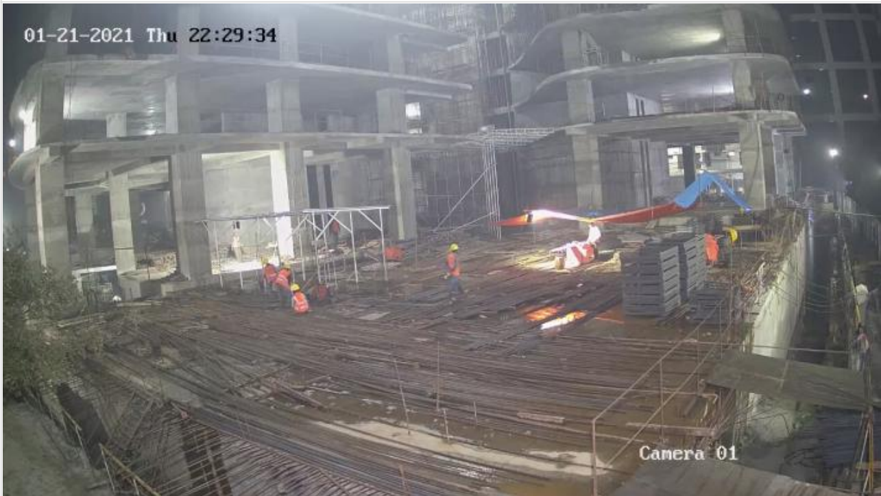
Night Shift Working on 21-01-21
