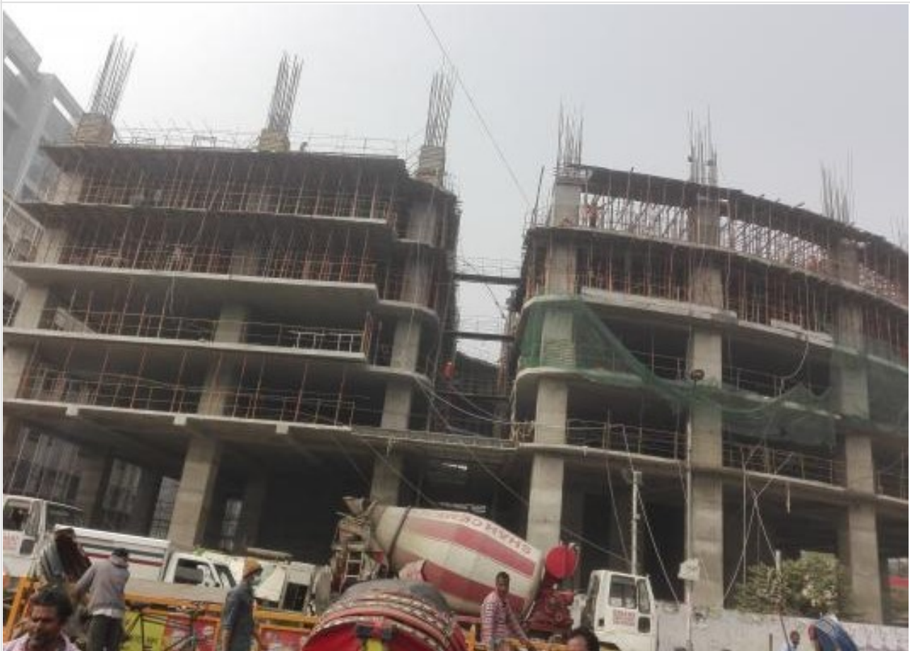
Project Picture on 24-01-21
