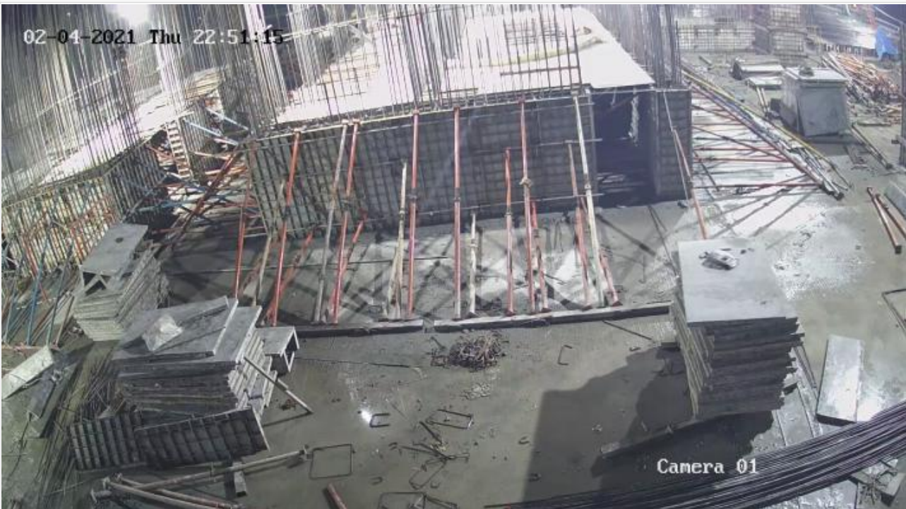
Night Shift Working on 04-02-21
