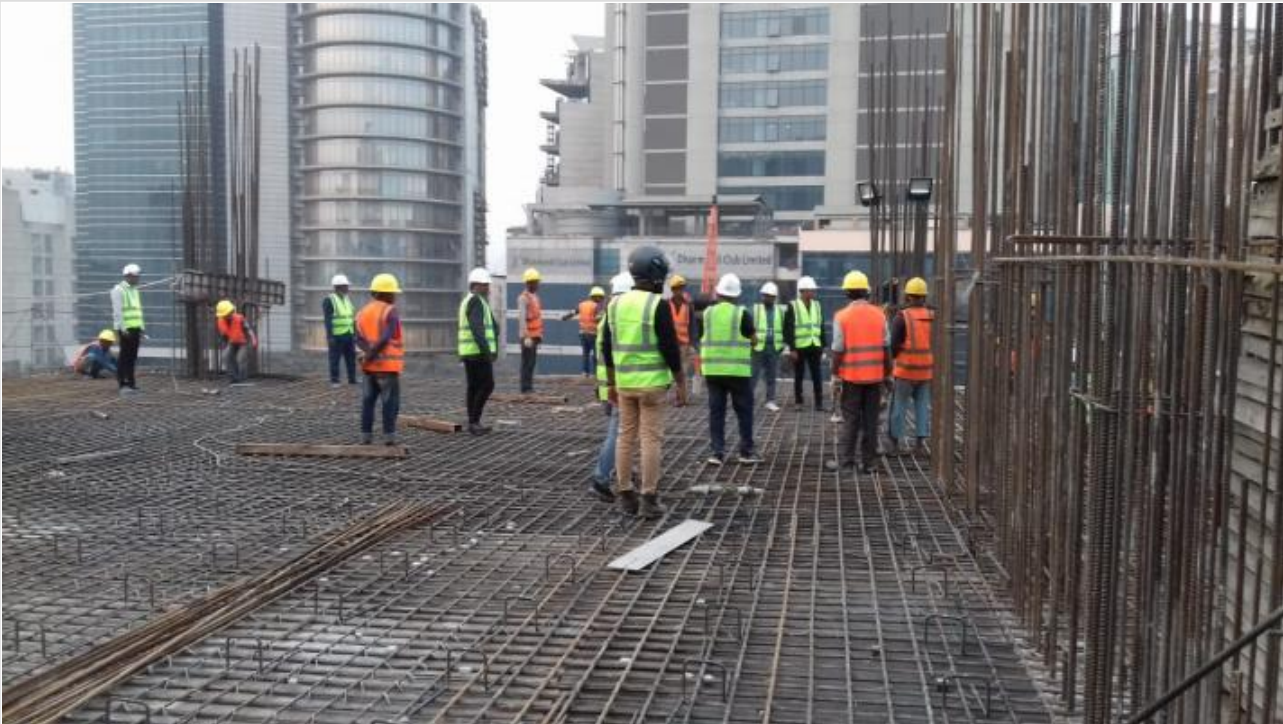
Work Inspection on 30-01-21
