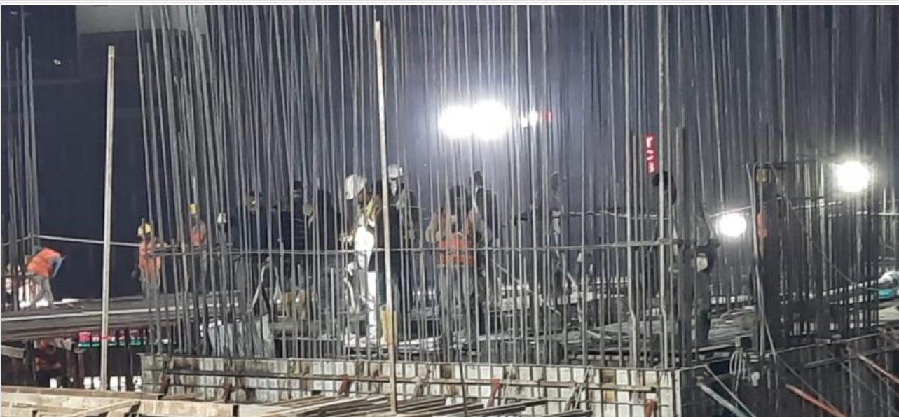
Re-bar Work on 18-01-21
