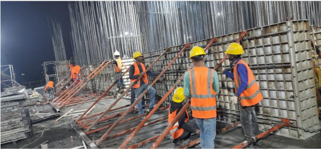
Lift Core Wall Shuttering on 17-01-21
