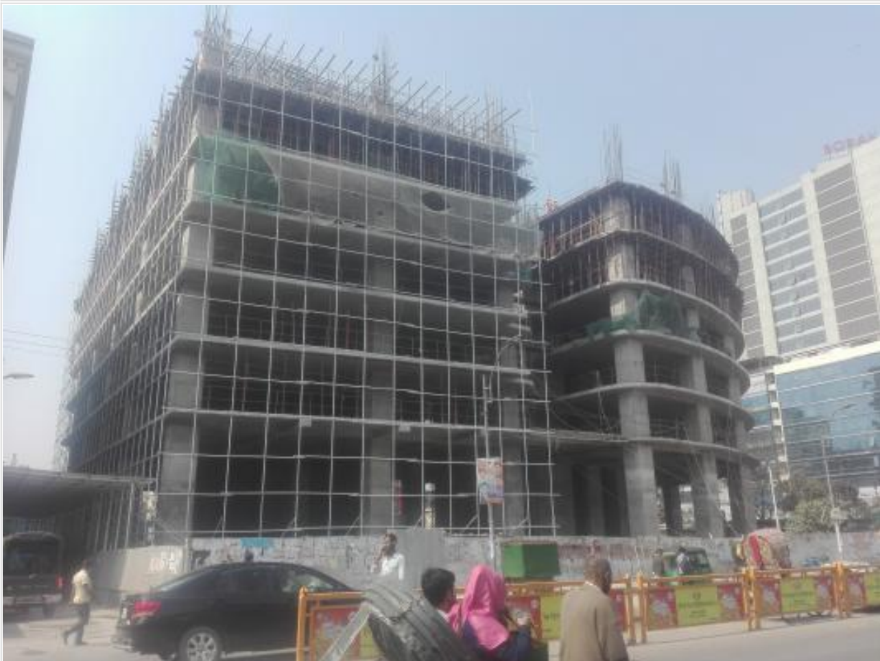
Project View from East Side on 06-02-21
