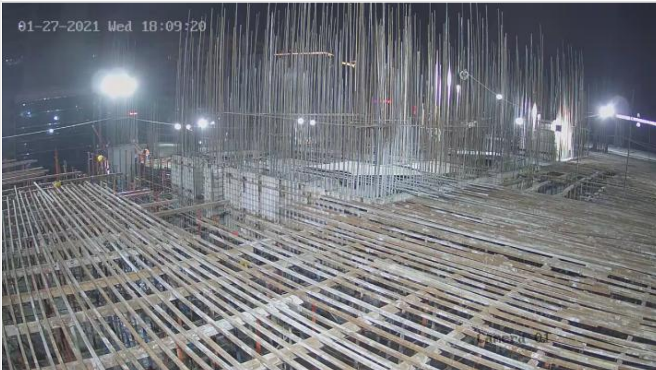
Slab Shuttering on 27-01-21
