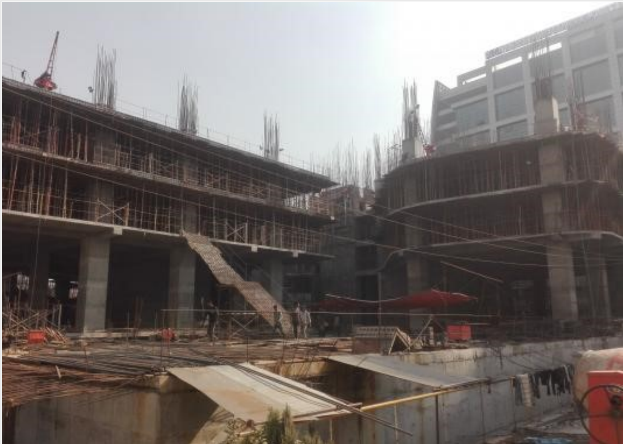
3rd Floor South Tower Slab Complete on 11-01-21
