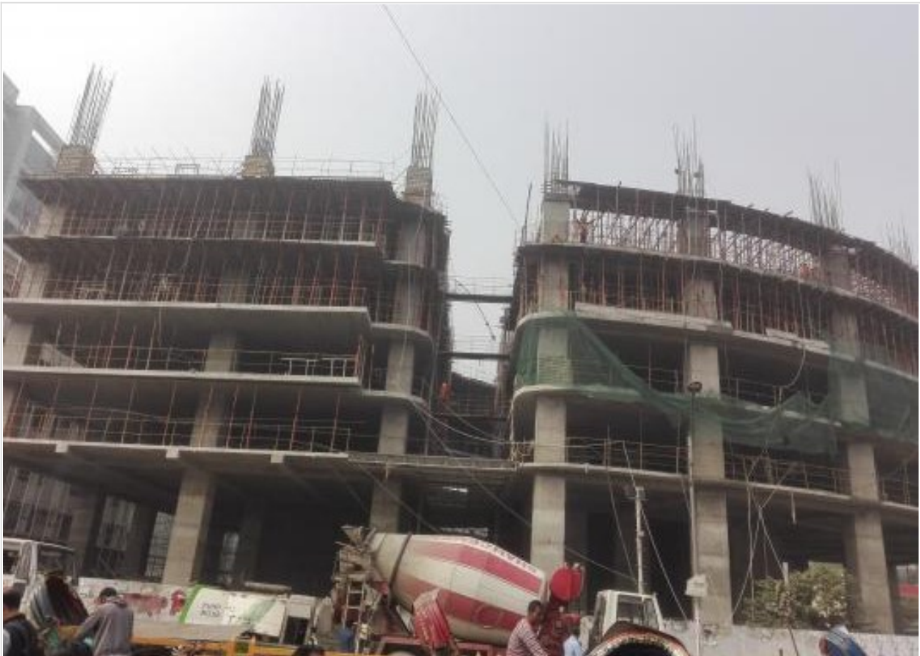
Project Picture on 24-01-21
