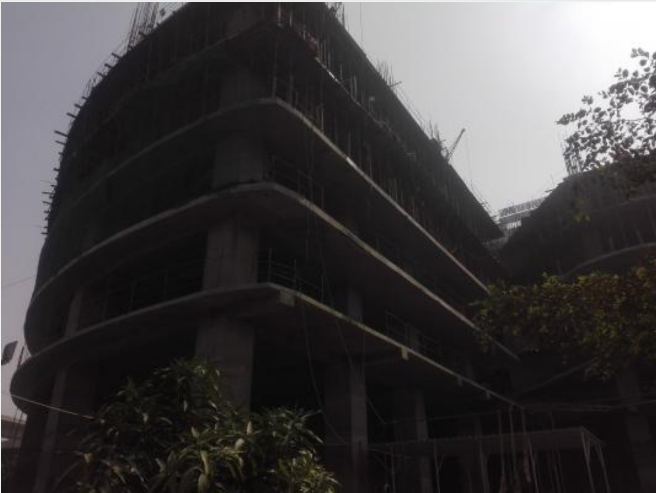
Project Picture on 03-02-21
