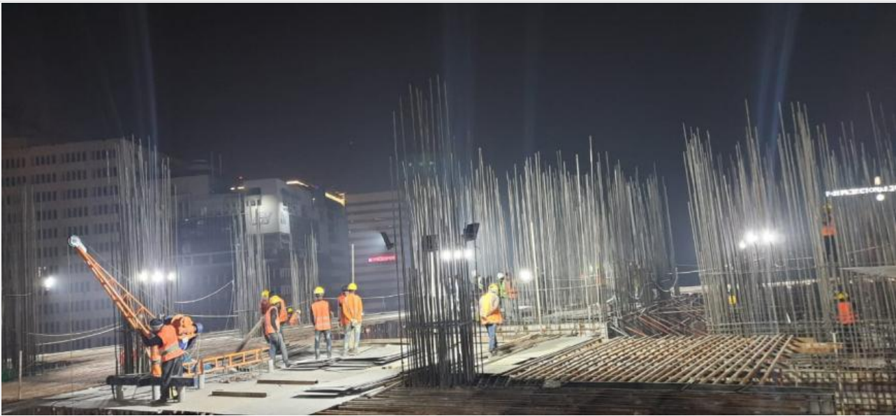
Re-bar Lifting by Roof Hoist on 14-01-21
