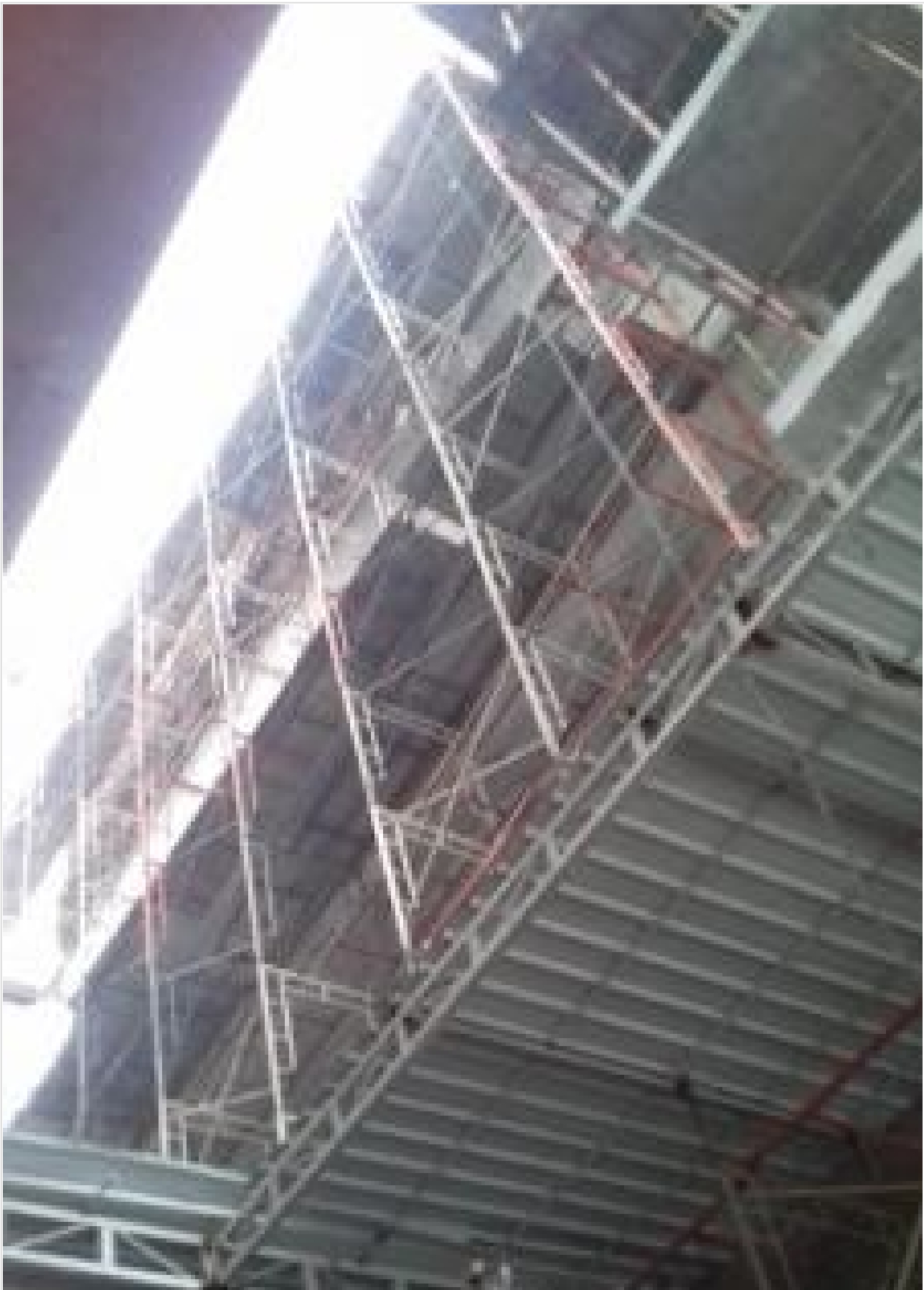
Safety Railing on 03-02-21
