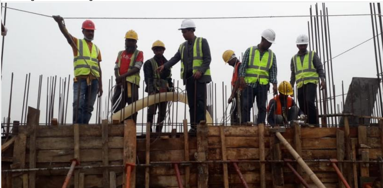
Retaining wall Concreting on 20-02-21
