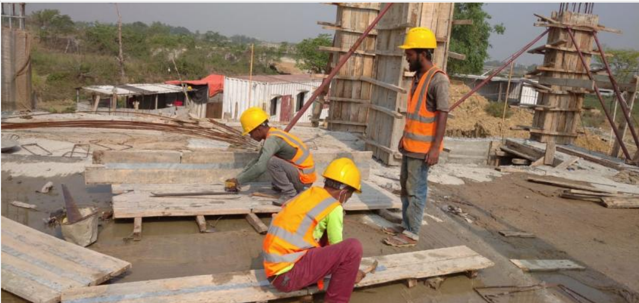
Ground Floor-Column Shuttering Work on 12-05-21
