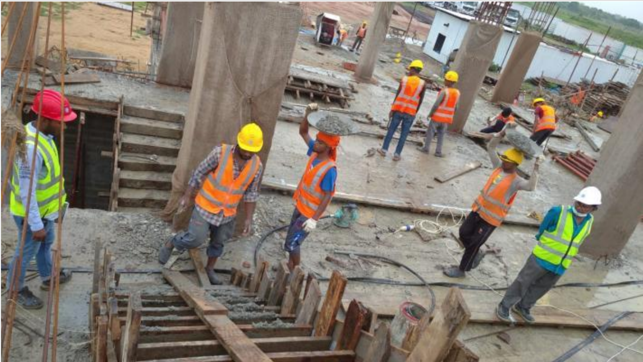
Ground Floor Stair Concreting on 31-05-21
