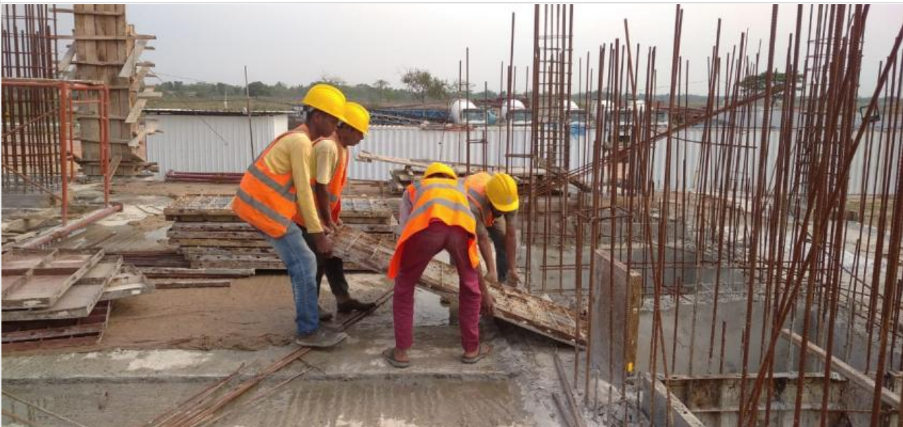
Column Re-bar Work on 08-05-21
