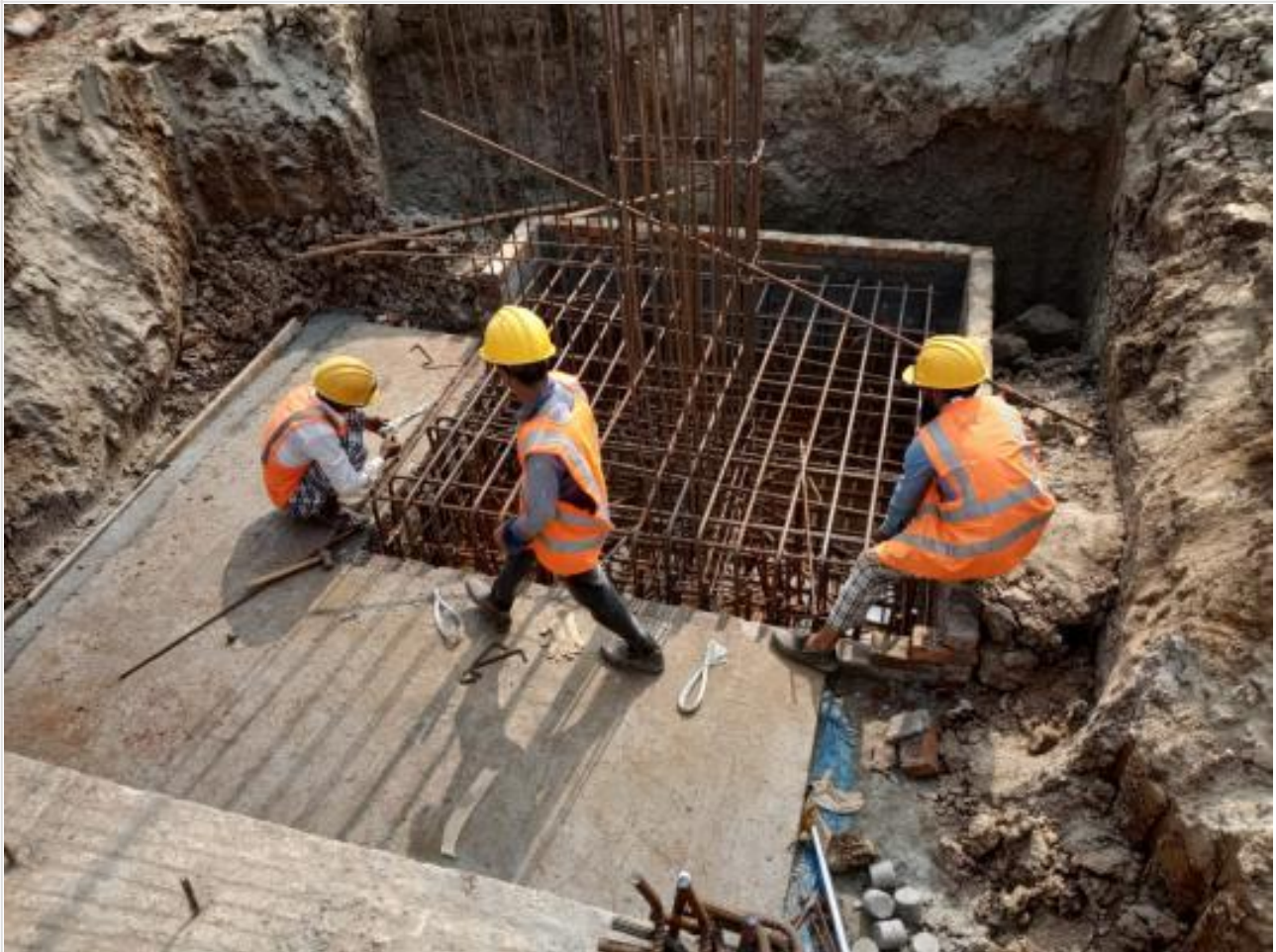
Footing Re-bar Placing on 19-12-20
