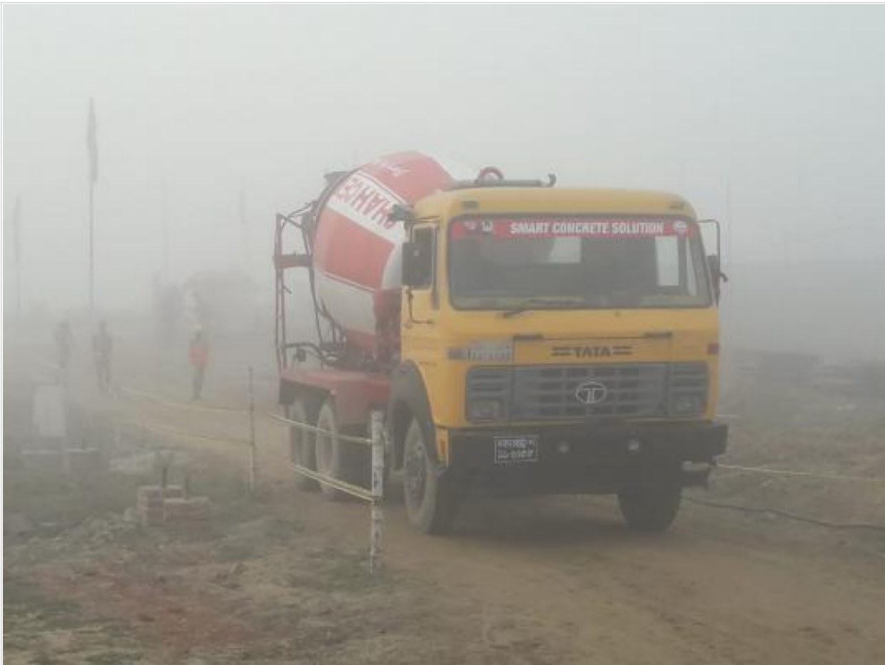
Pile Cap Concreting on 06-12-20
