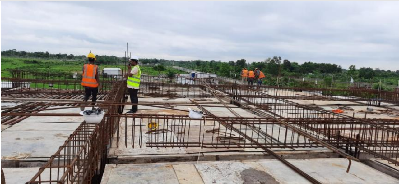
1st floor Slab Shuttering on 12-06-21
