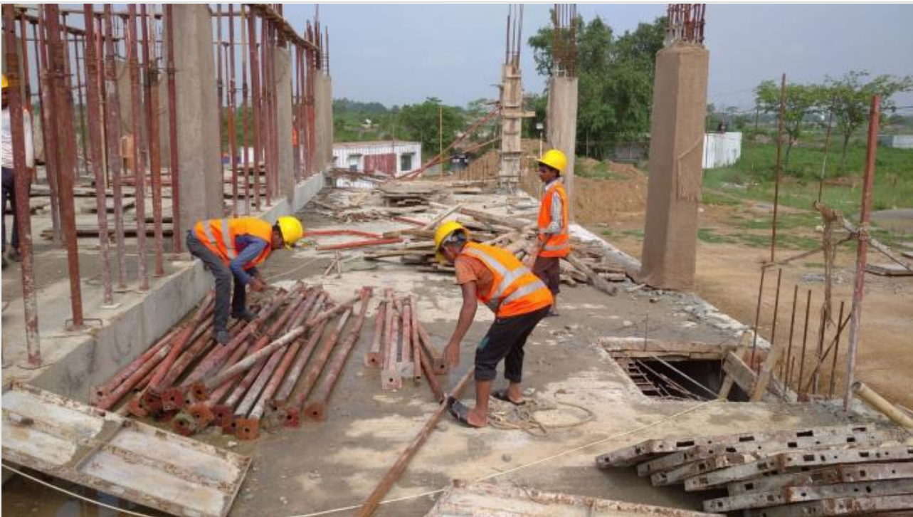
1st Floor Slab Shuttering on 03-06-21
