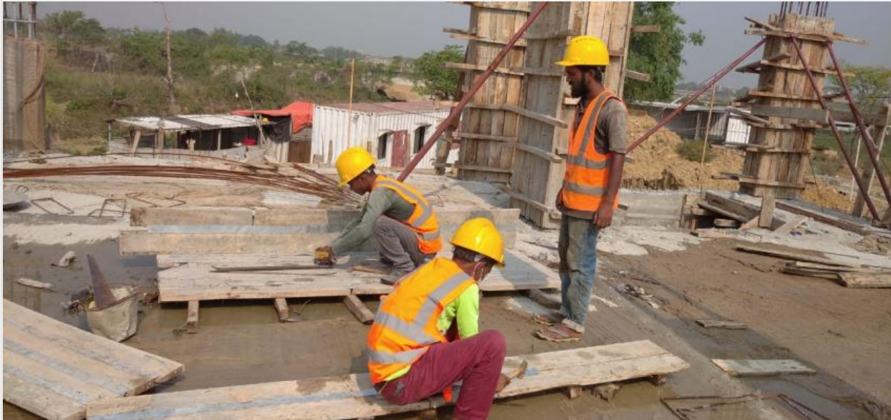
Ground Floor-Column Shuttering Work on 12-05-21
