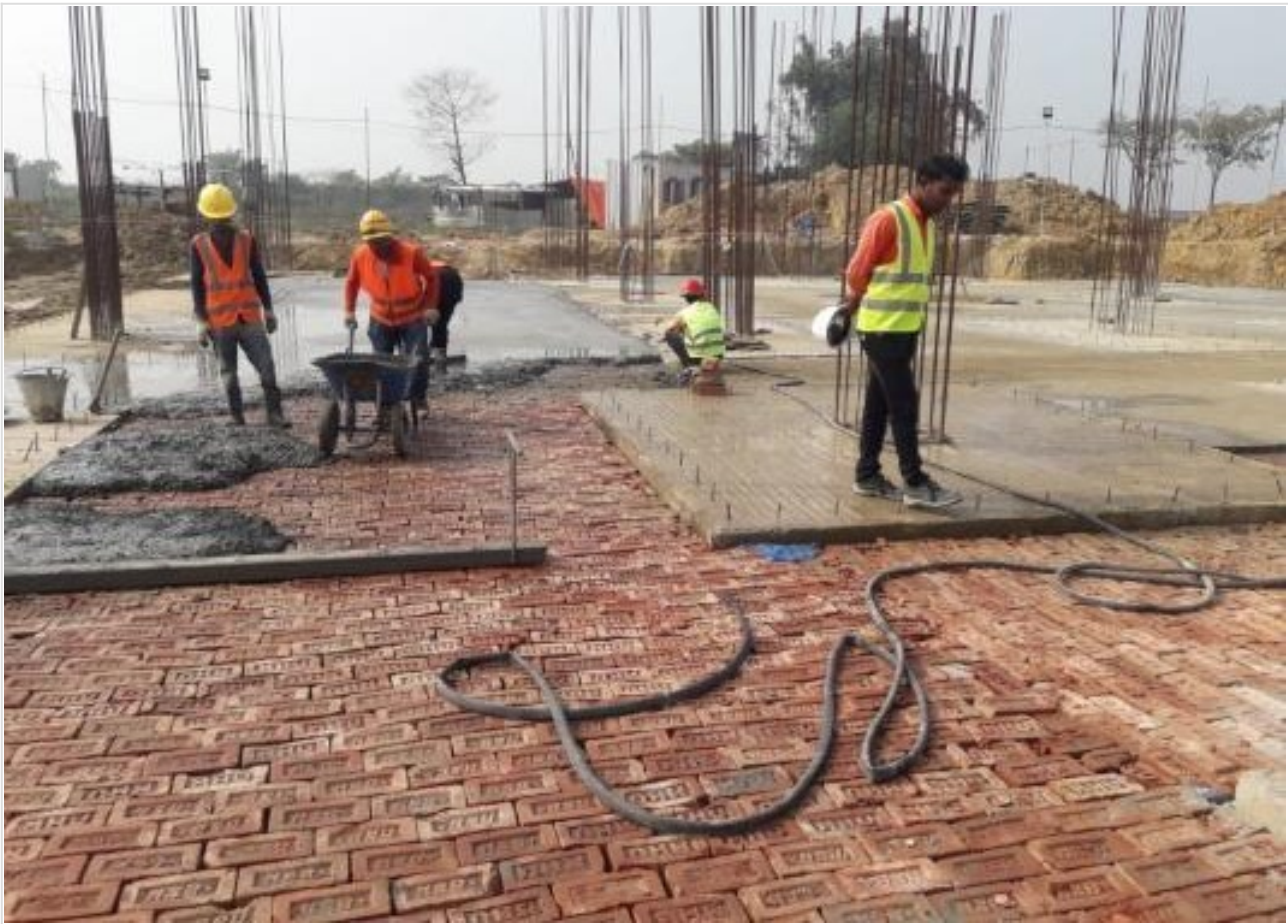
Mat CC Concreting on 15-12-20
