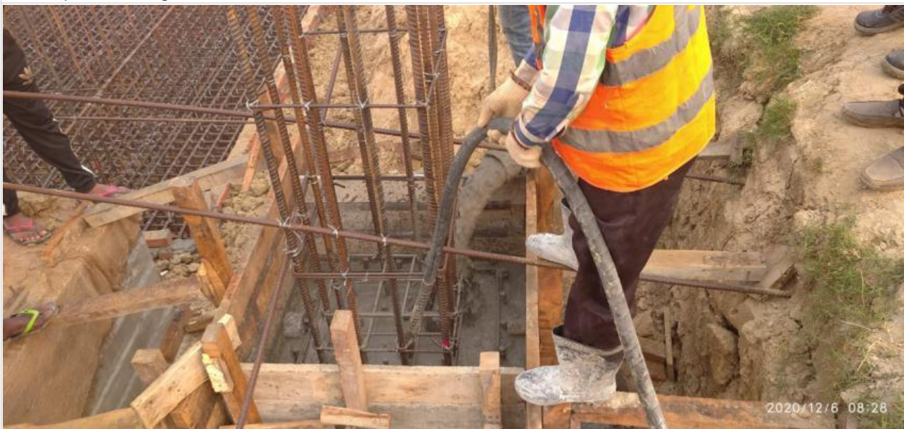
Pile Cap Concreting on 06-12-20
