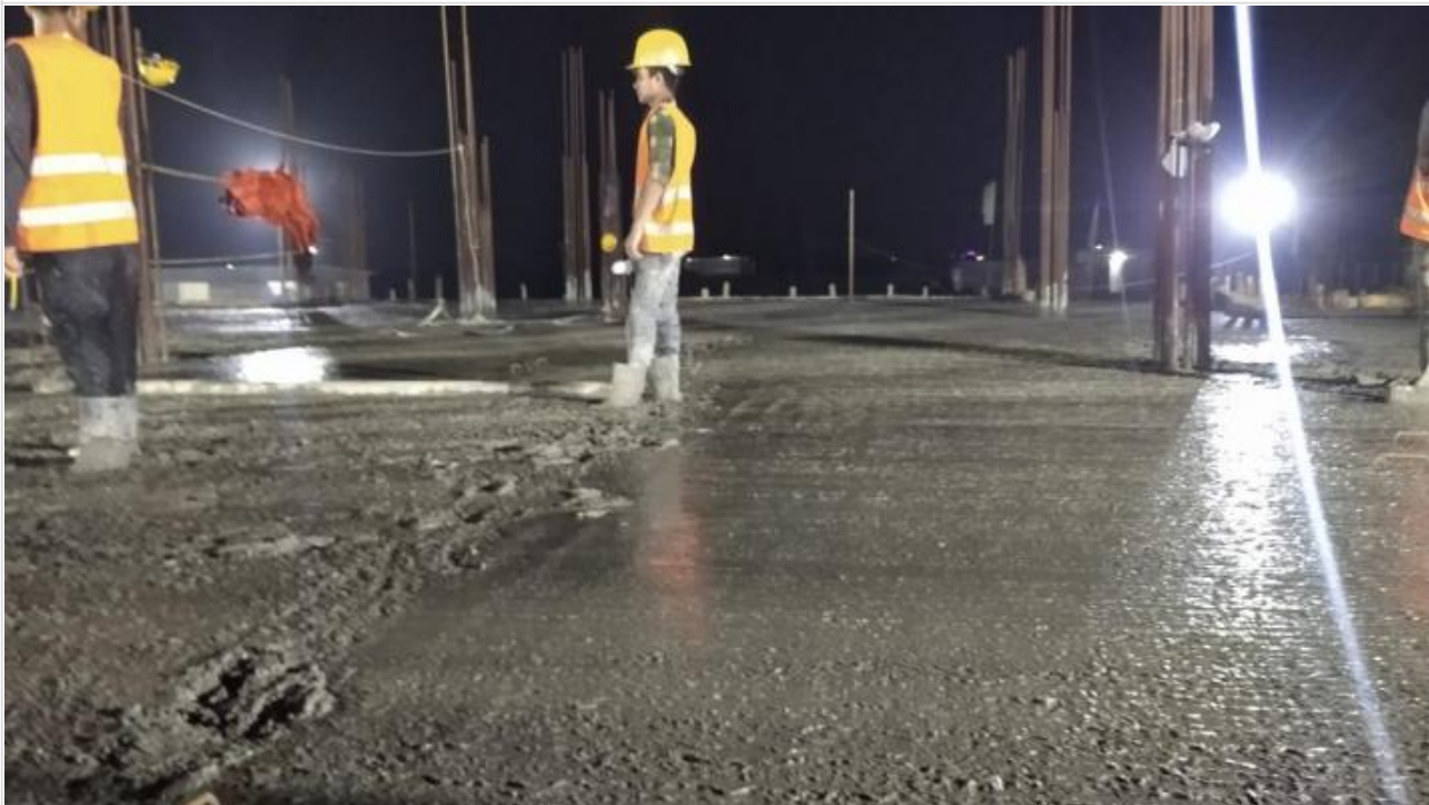
GF Slab Concreting complete at night on 15-03-21
