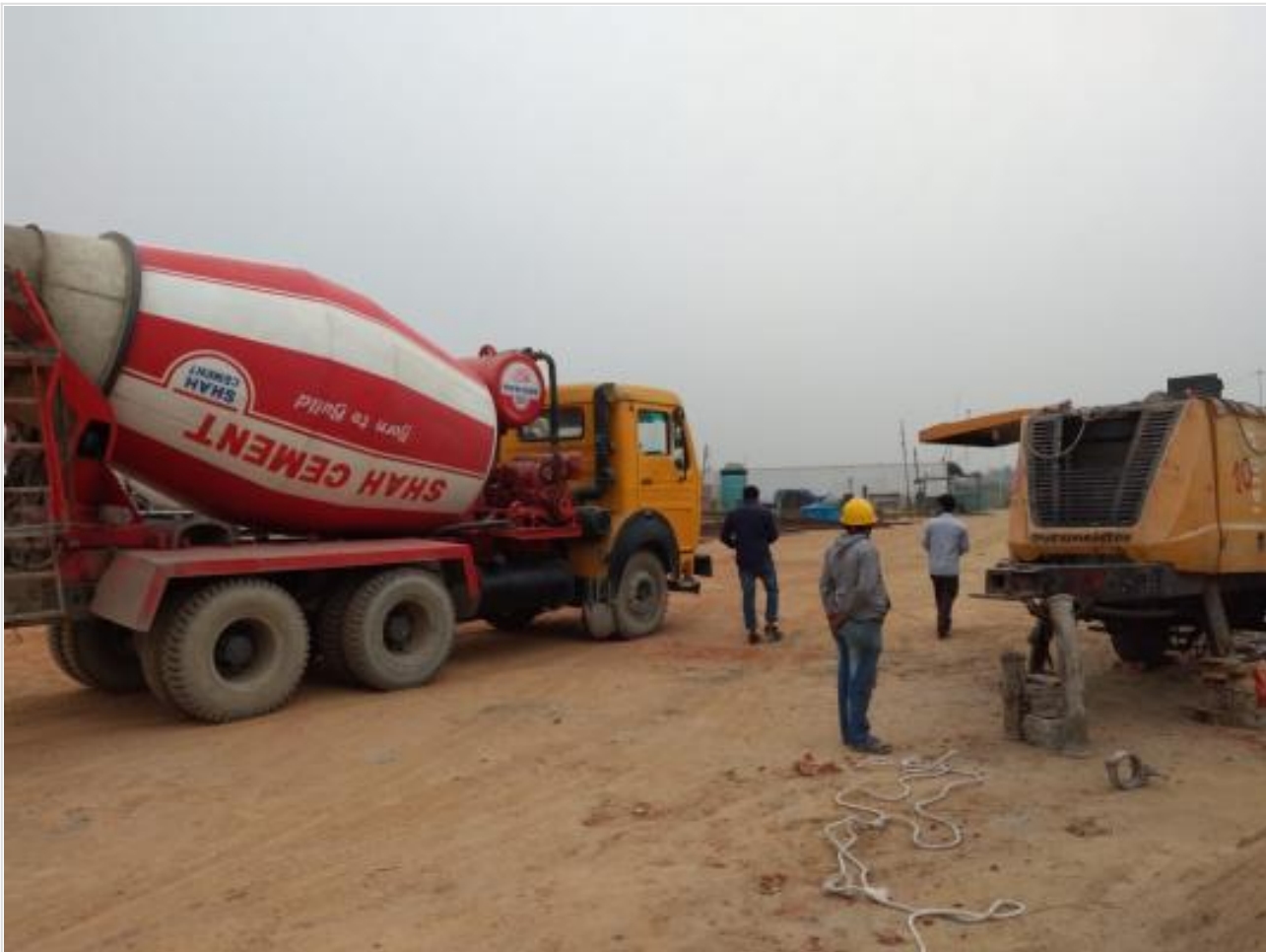
Retaining Wall Concreting on 20-02-21
