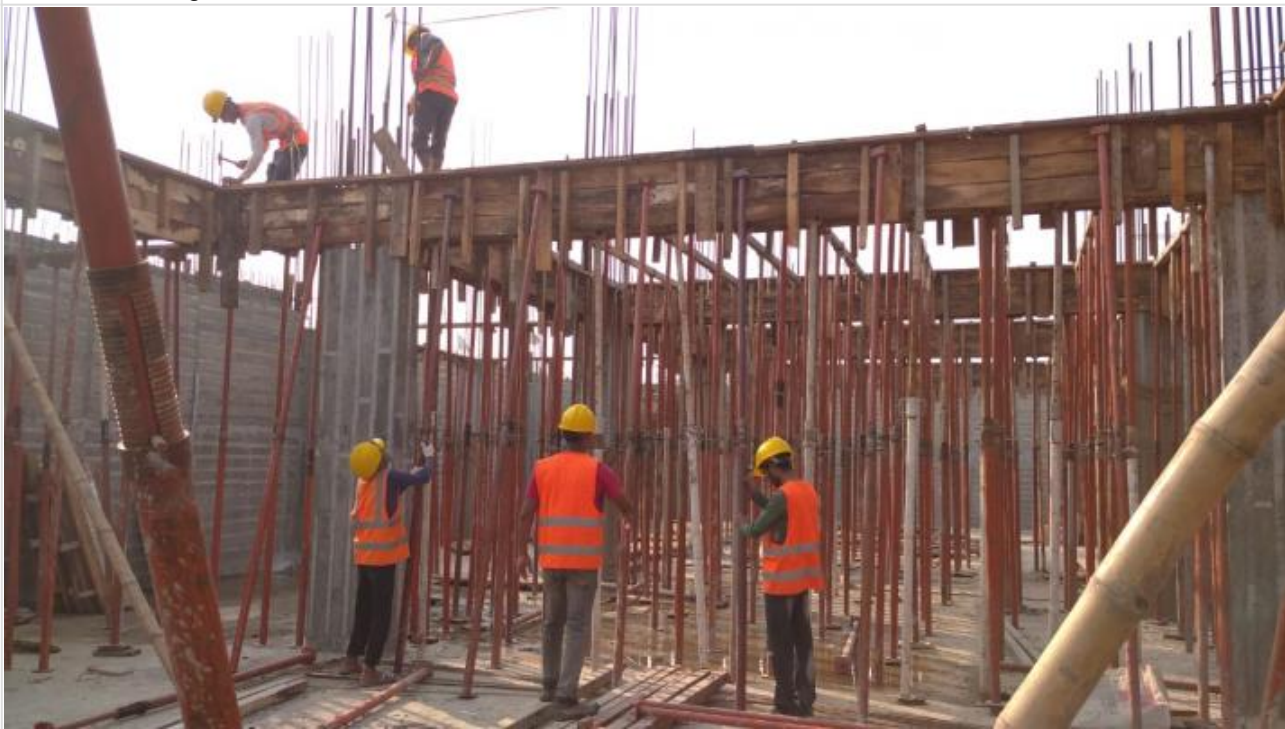
Ground Floor Slab Shuttering on 25-02-21
