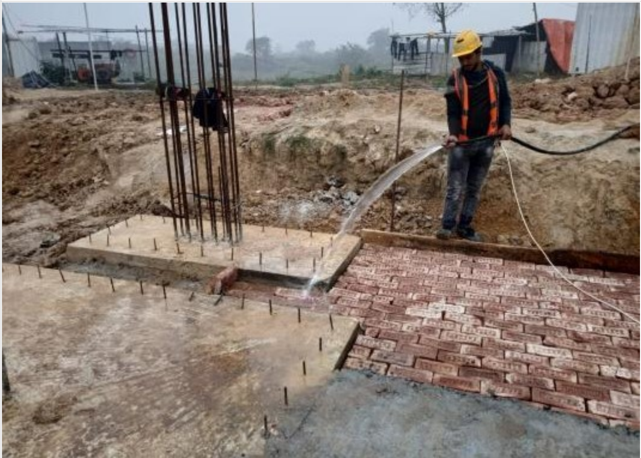
Footing Curing on 15-12-20
