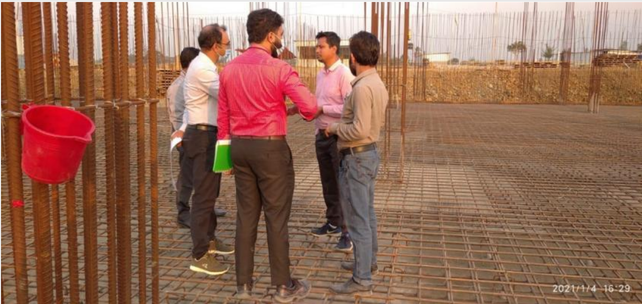
Inspection before Mat Concreting on 05-01-21
