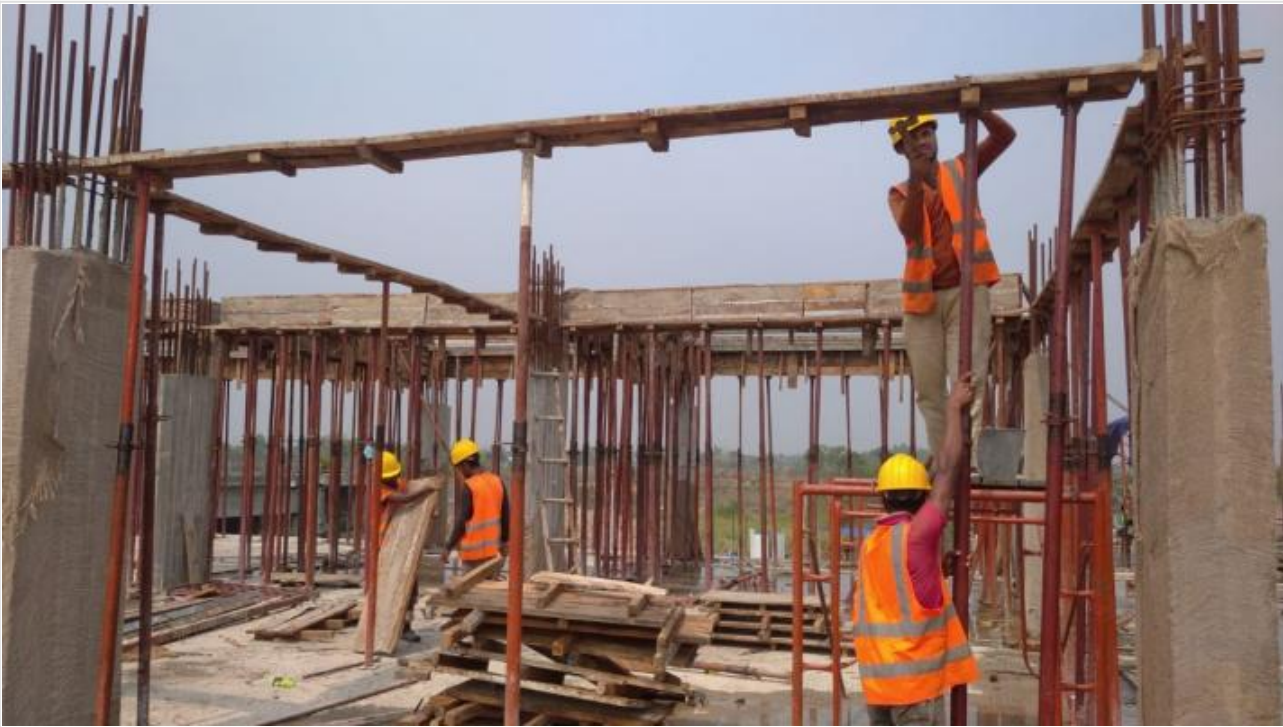
Beam Shuttering on 03-05-21
