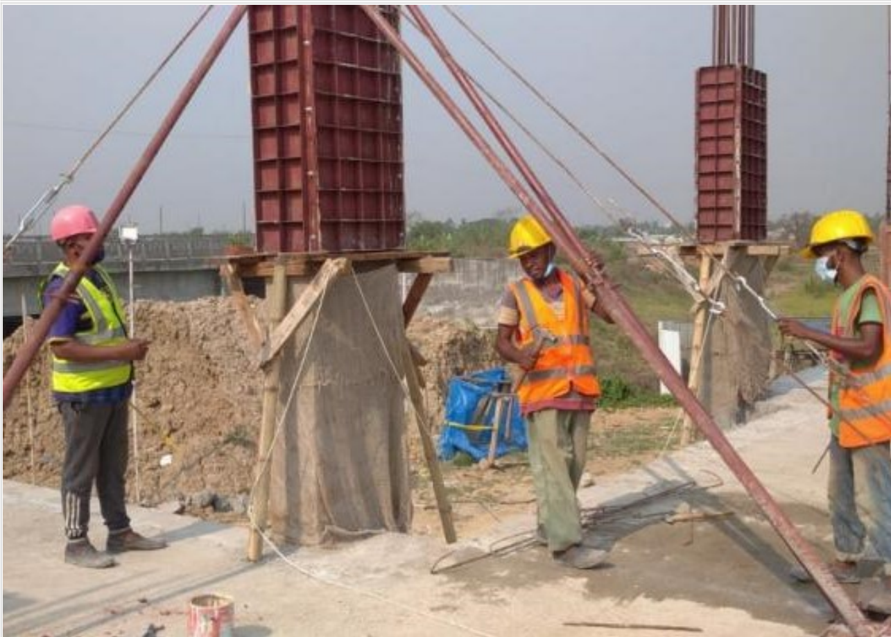
Column Shuttering on 09-05-21
