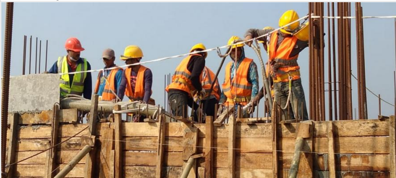
South Retaining wall 2nd Lift Concretin on 09-02-21
