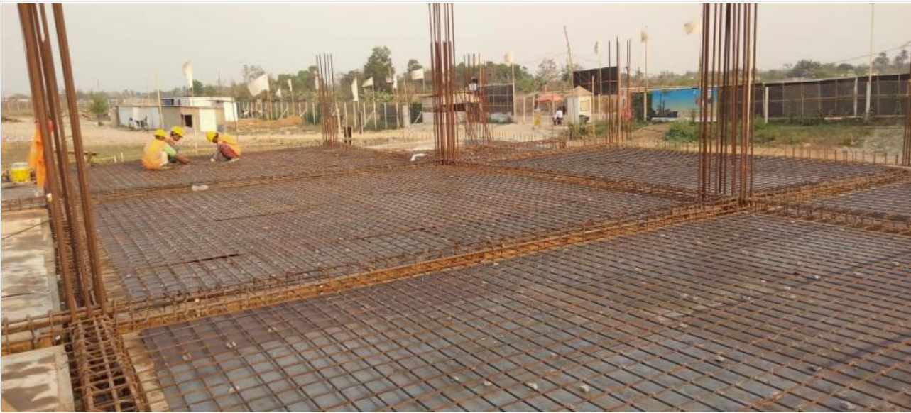
Ground Floor Slab Re-bar Work on 10-03-21
