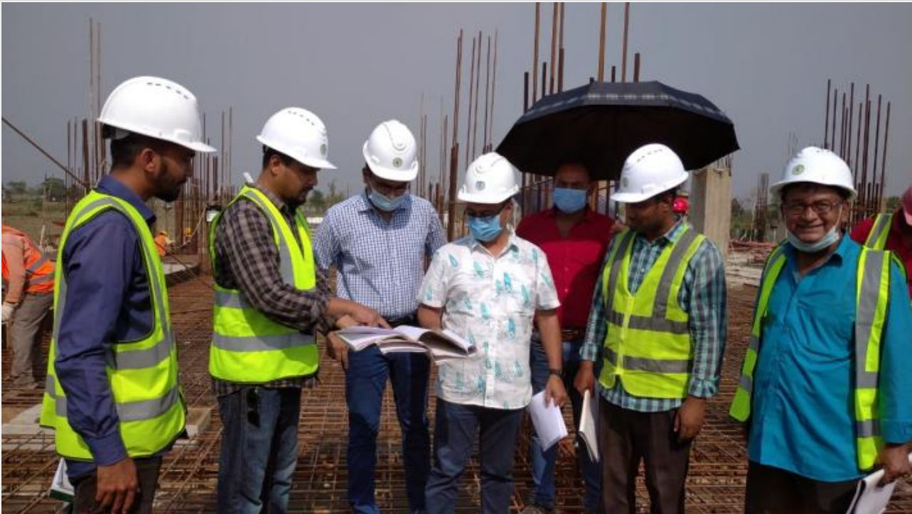
Inspection before GF Slab Concreting on 25-04-21
