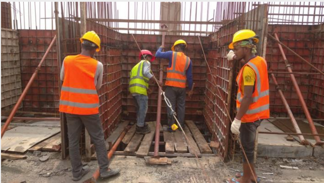
Ground floor Lift Core Shuttering on 07-06-21
