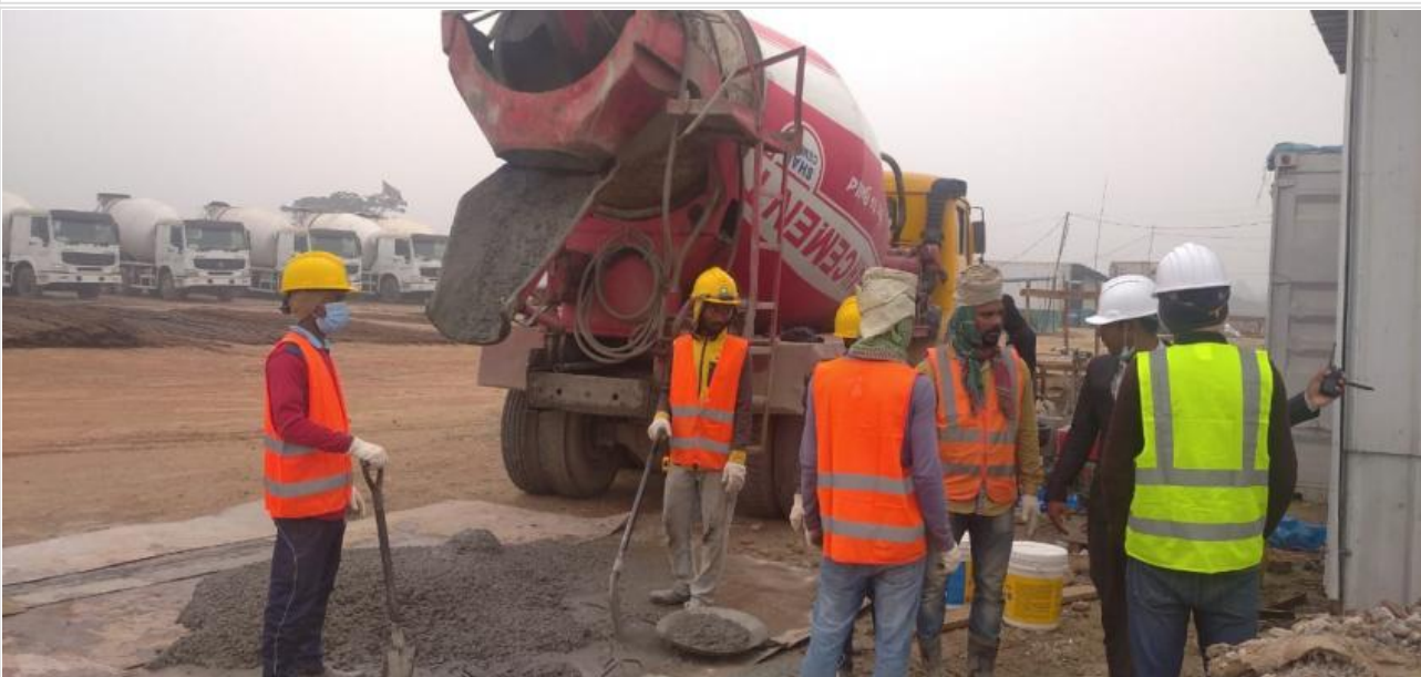
Mat Concreting on 05-01-21
