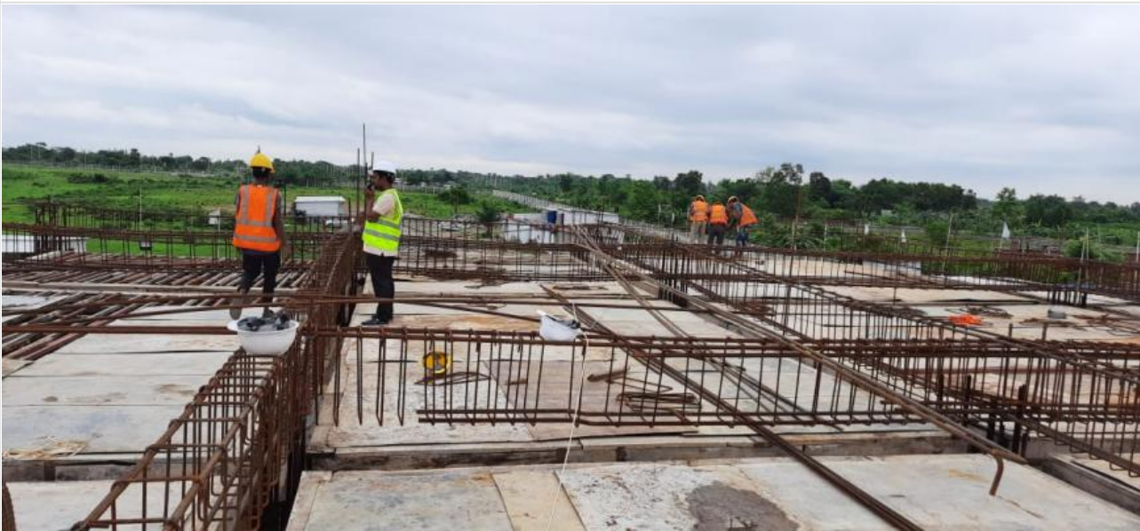
1st floor Slab Shuttering on 12-06-21
