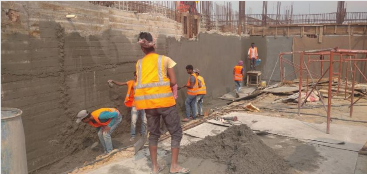
Basement West Wall Plastering on 07-03-21
