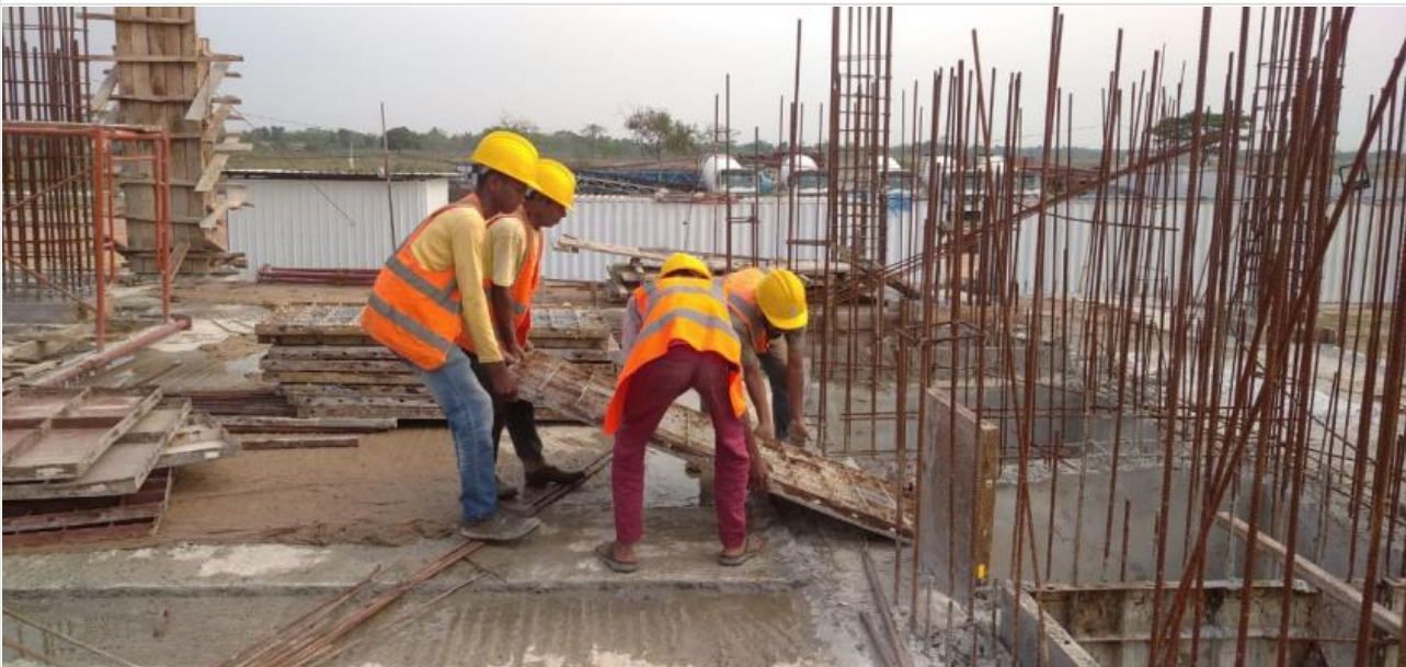
Column Re-bar Work on 08-05-21
