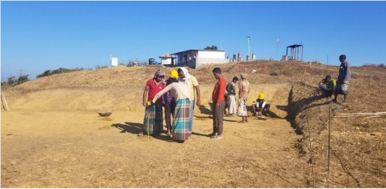
Guest House-Preparation for Layout on 05-01-21
