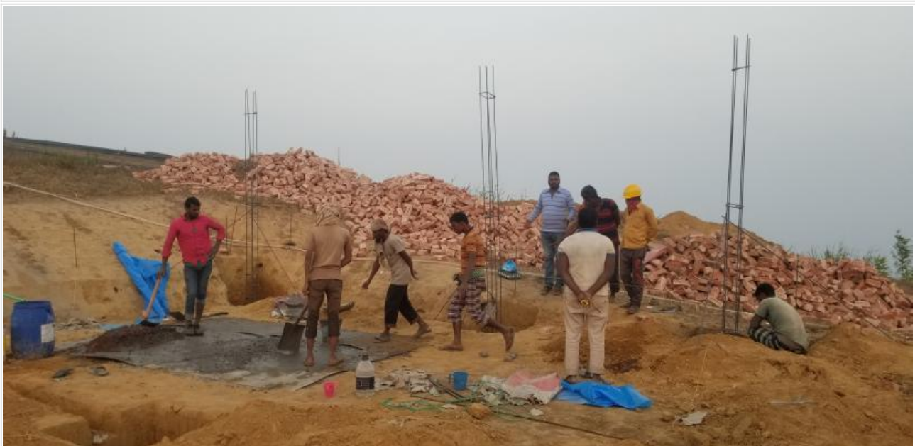
Footing & column casting work on going on 13-01-21
