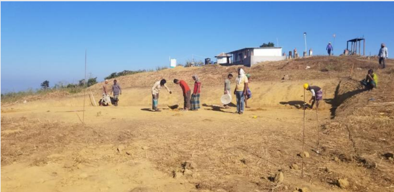
Guest House-Preparation for Layout on 06-01-21
