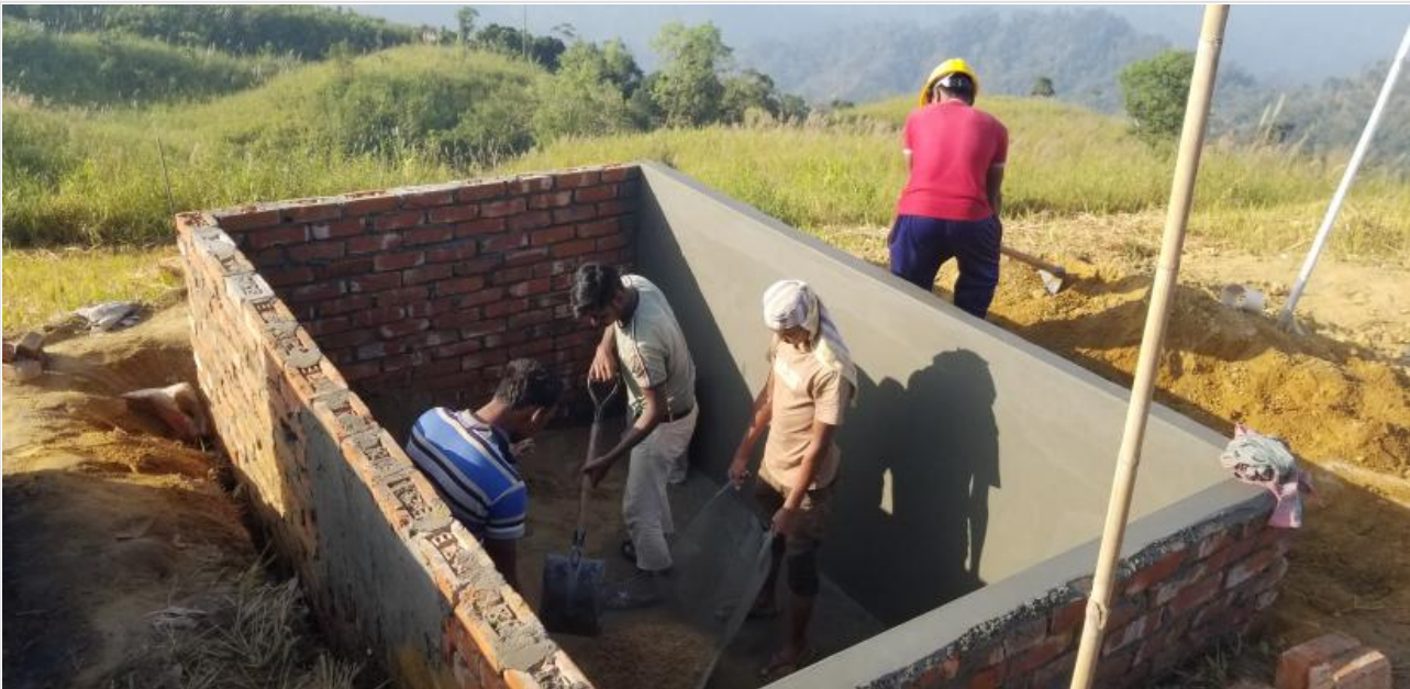
Plaster work for labour Shed on 12-01-21
