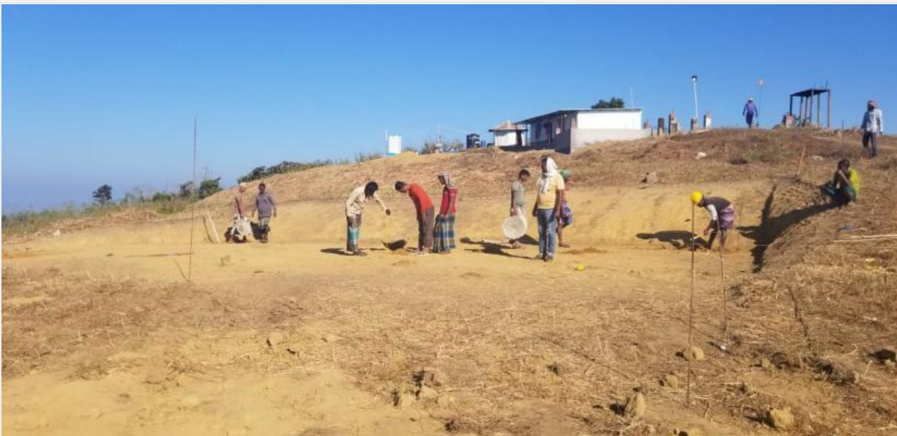
Guest House-Preparation for Layout on 07-01-21
