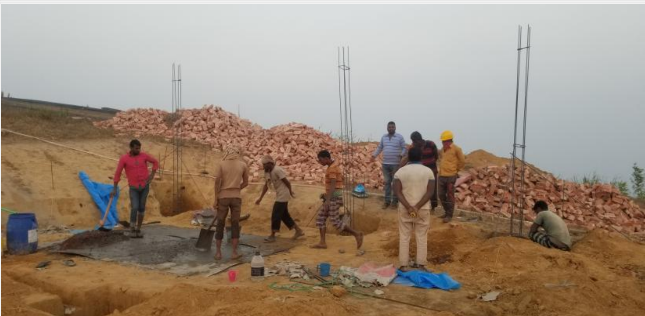
Footing & column casting work on going on 13-01-21
