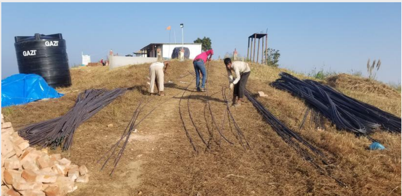
MS rod cutting & binding on 12-01-21
