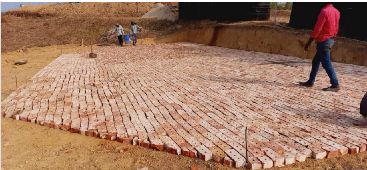
Soling for PVC Water Tank on 20-01-21
