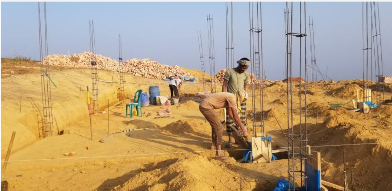
Short column casting work for guest house on 17-01-21
