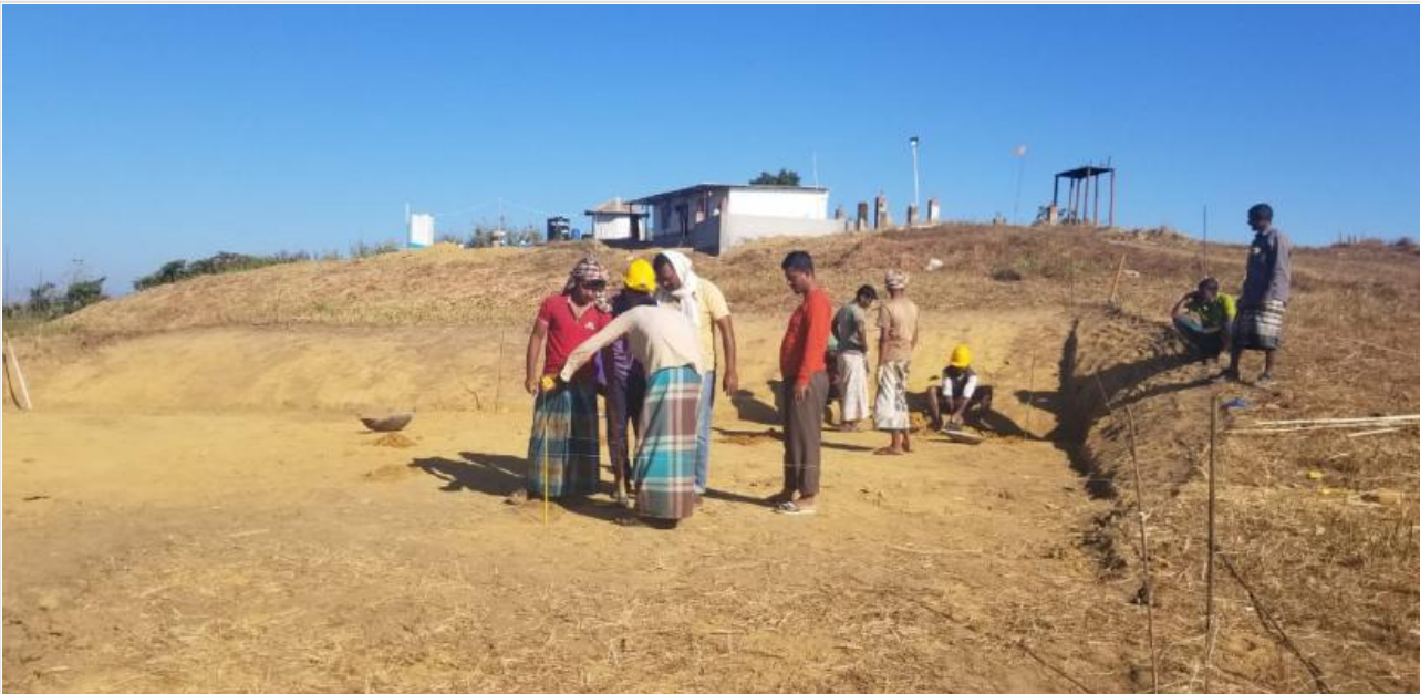
Guest House-Preparation for Layout on 07-01-21
