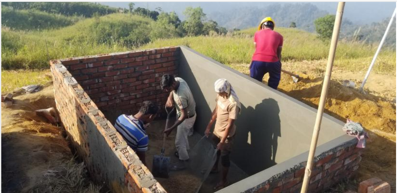
Plaster work for labour Shed on 12-01-21
