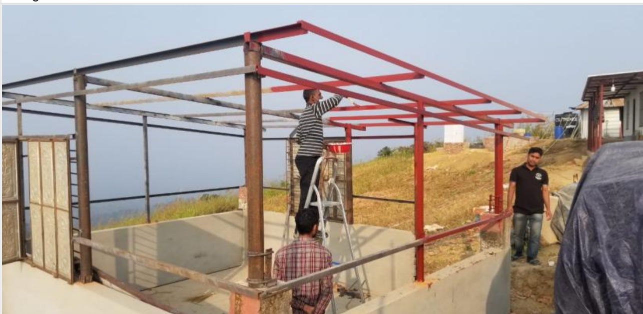
Mechanics Shed Frame Work on 20-01-21
