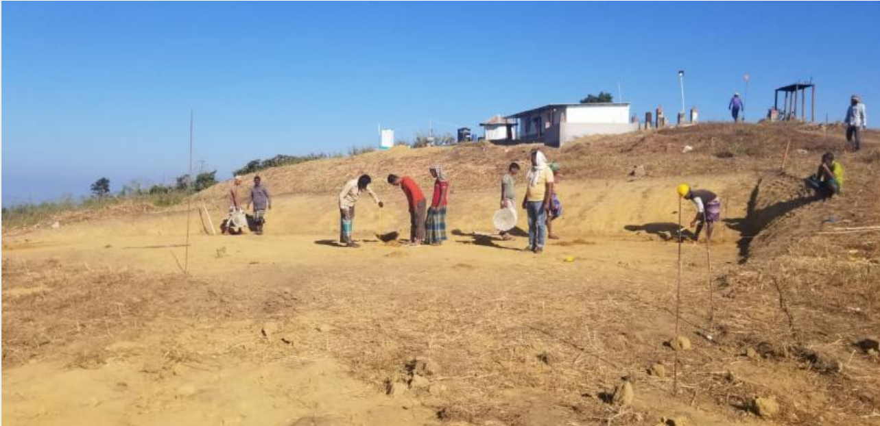
Guest House-Preparation for Layout on 05-01-21
