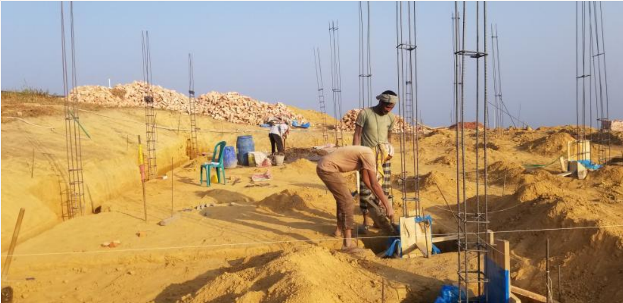
Short column casting work for guest hous on 17-01-21
