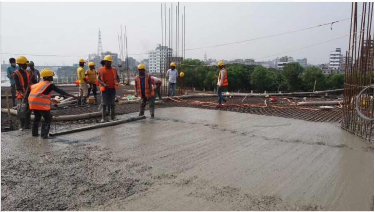
Mosque 1st Floor Slab Concreting on 06-04-21
