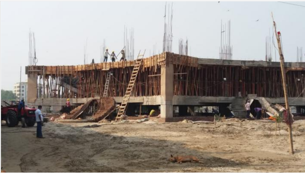
Mosque under Construction on 13-04-21
