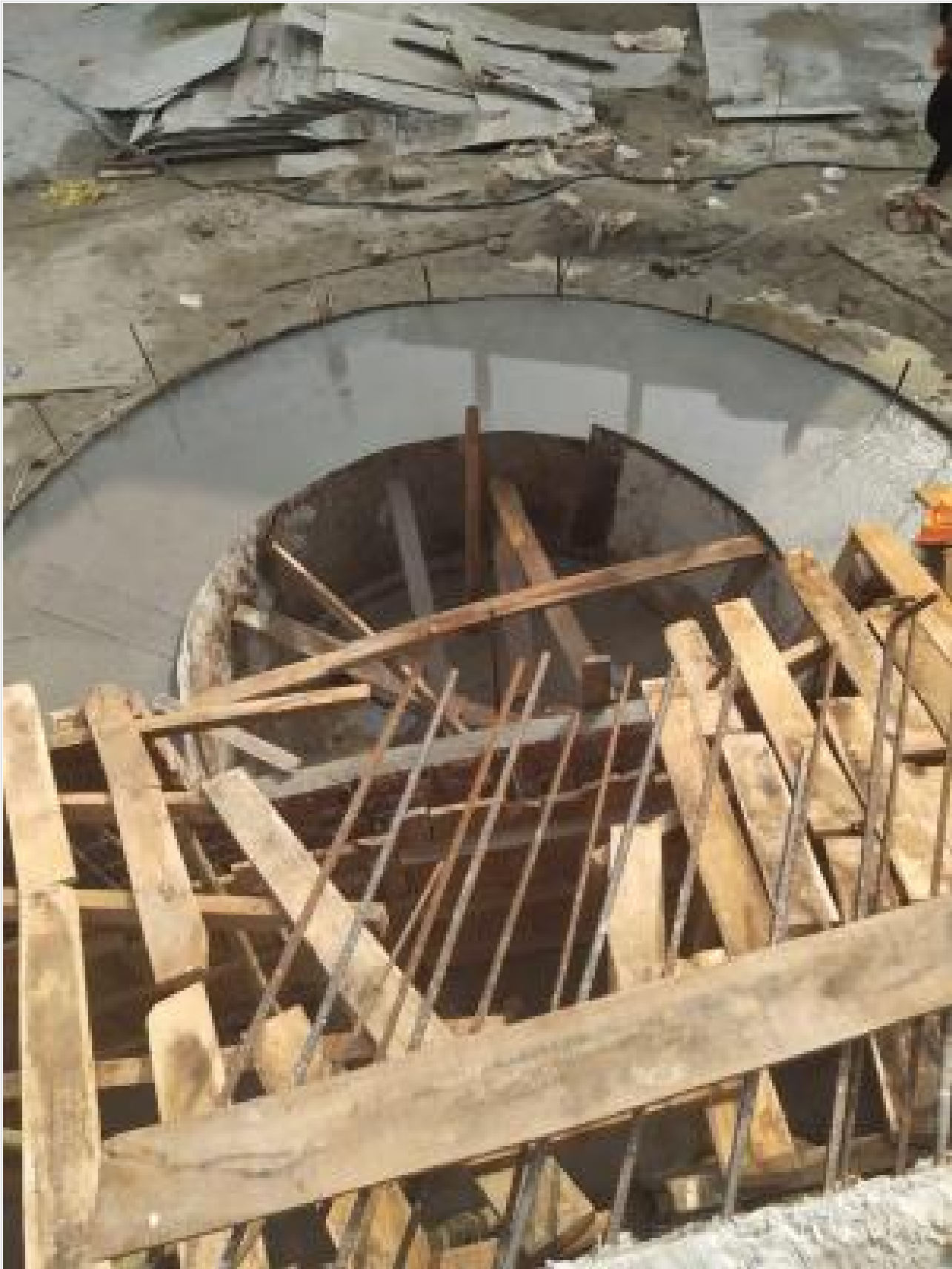
Mosque Ground Floor Stair Concreting on 27-03-21
