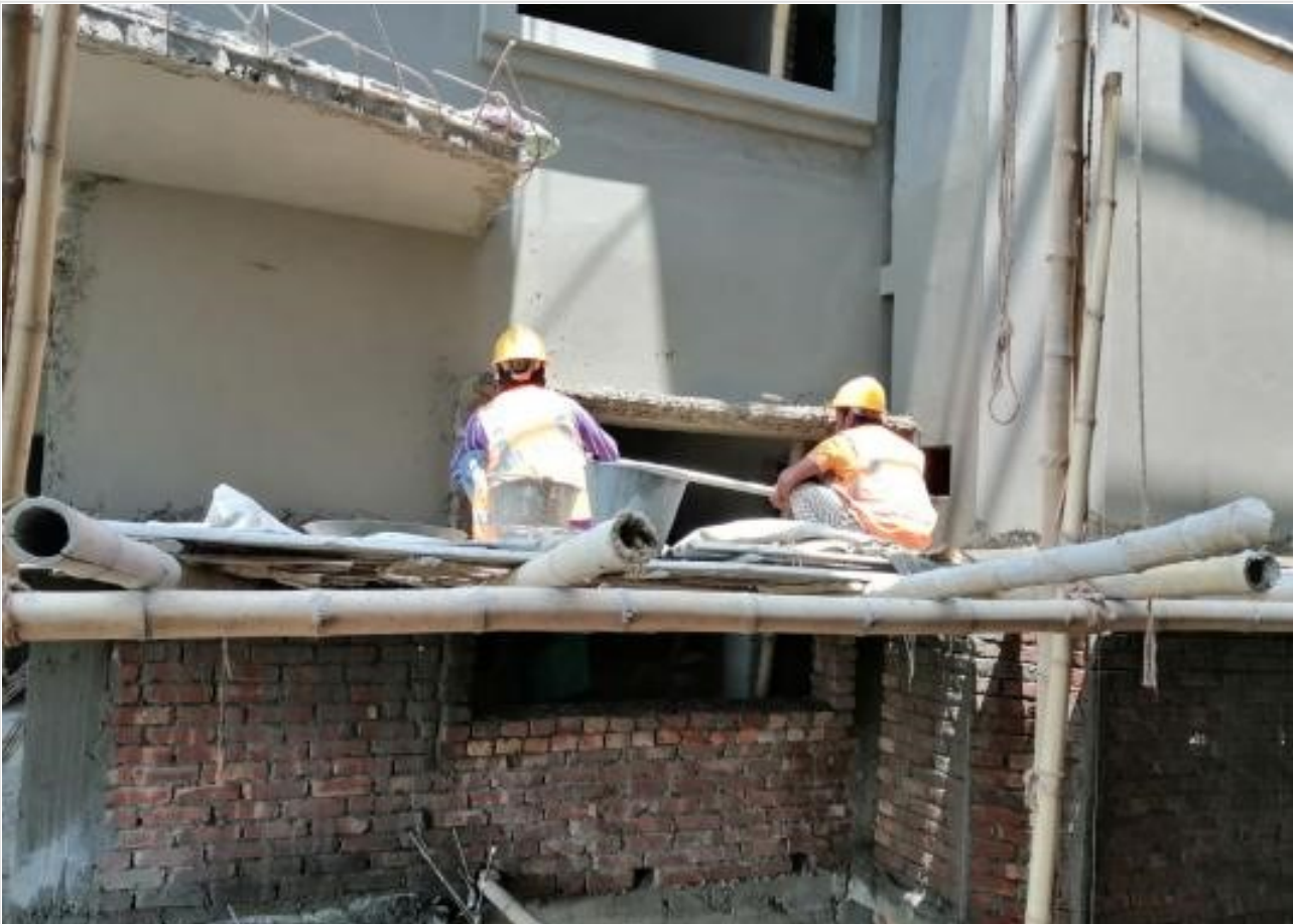
Out-side Plastering on 19-04-21
