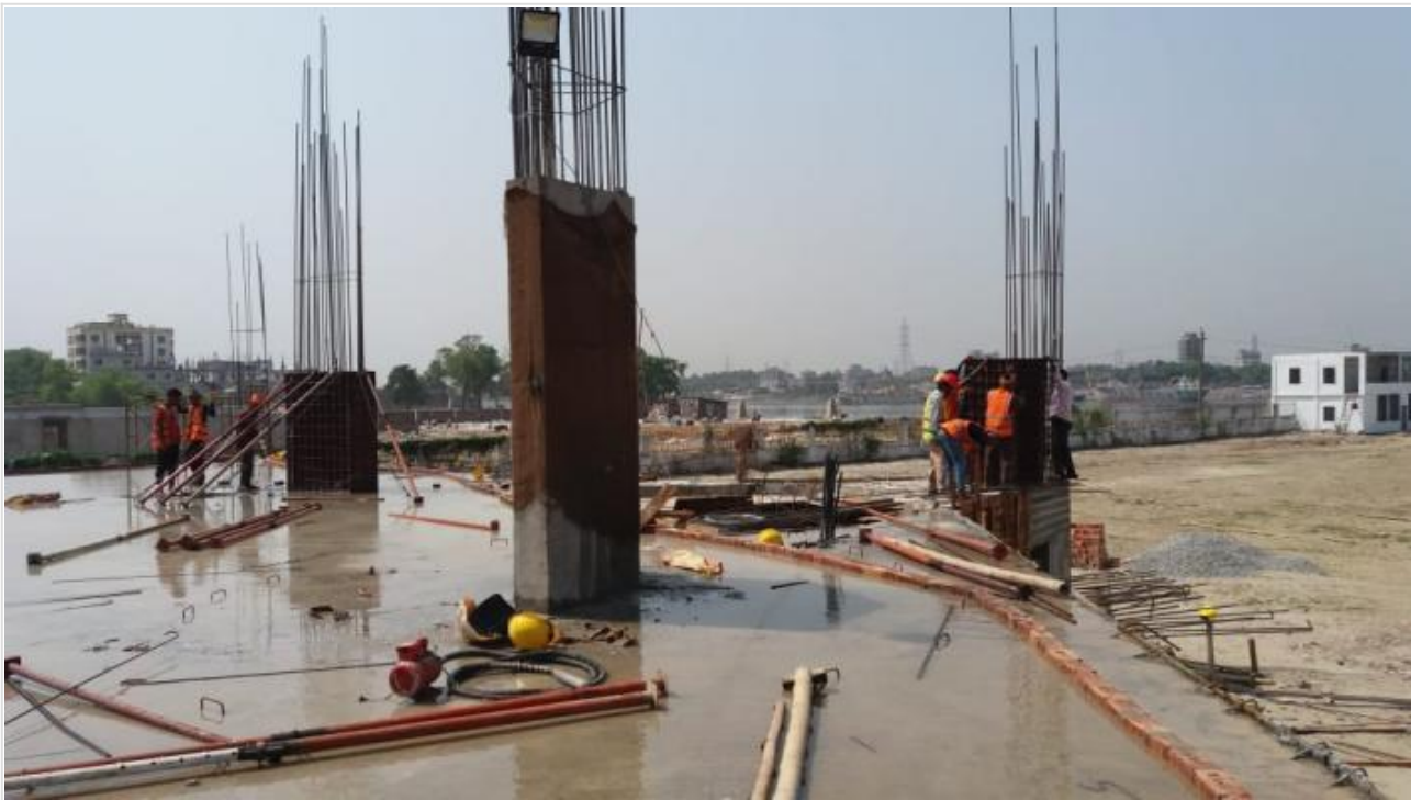
Mosque-GF Column Work on 25-03-21
