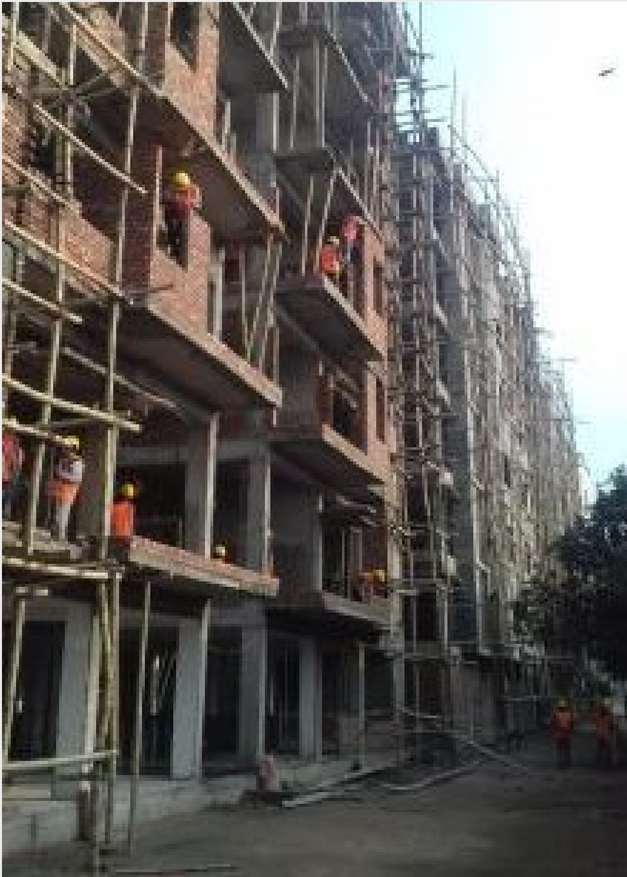
Scaffolding for outside plastering Build on 29-01-21
