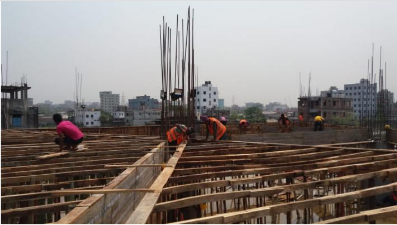
Mosque 1st Floor Slab Shuttering on 28-03-21
