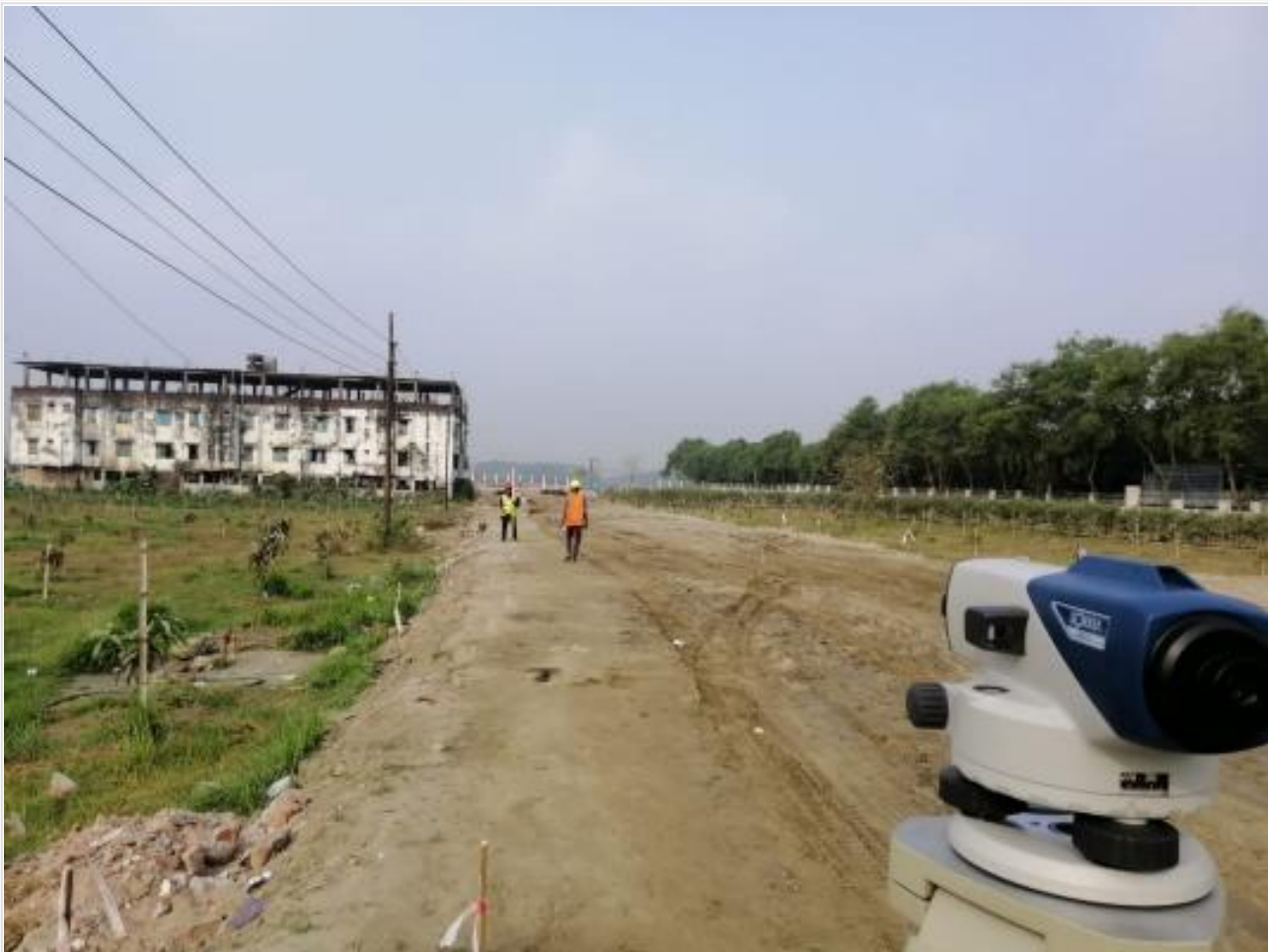
40 ft Road Dressing and Levelling on 01-03-21
