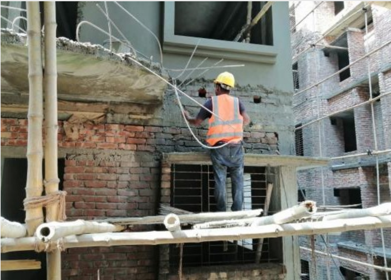
Out-side Plastering on 20-04-21
