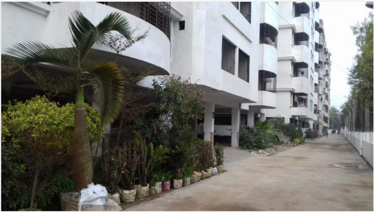
Building- outside plastering on 29-01-21
