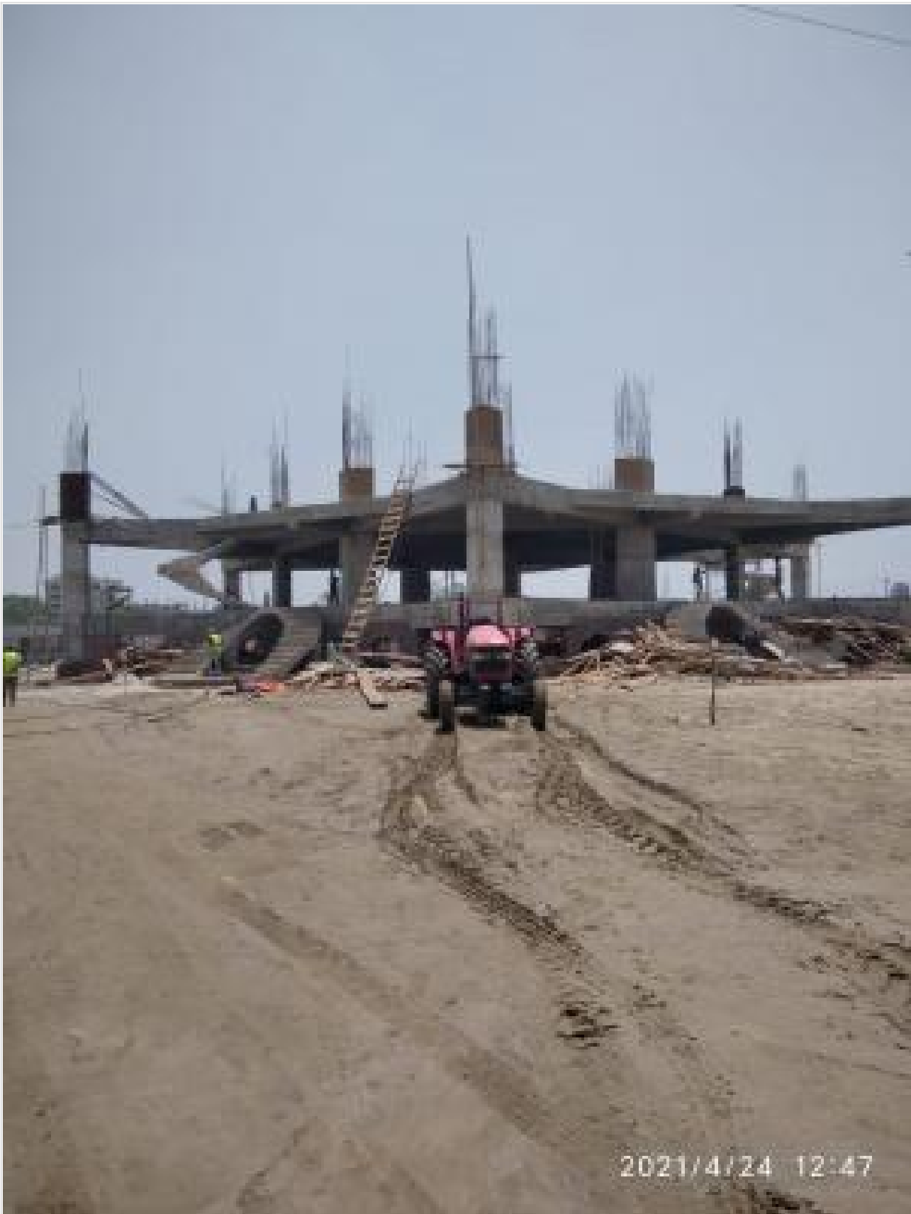
Mosque Building in Construction on 24-04-21
