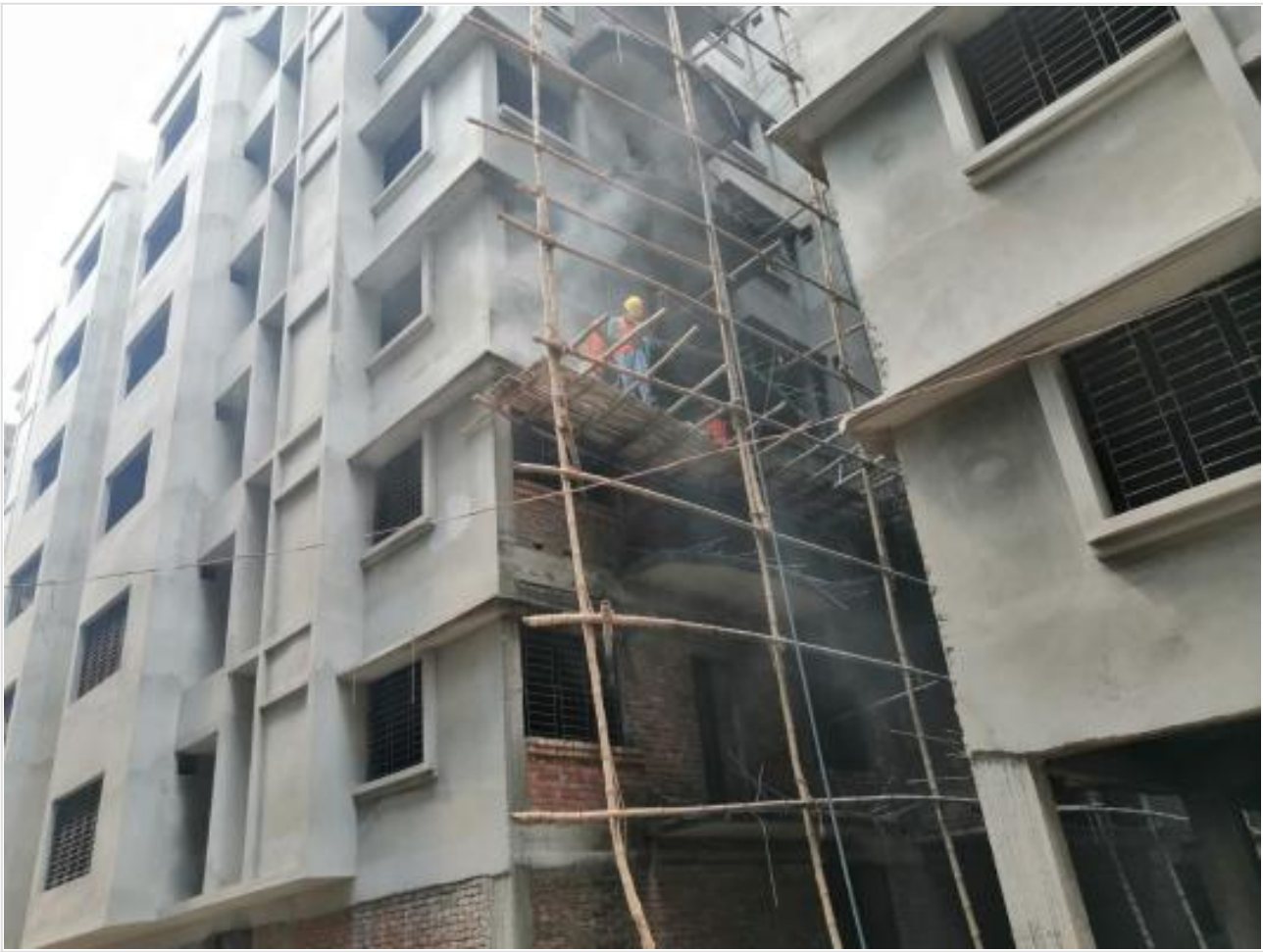
Building Outside Plastering on 08-03-21
