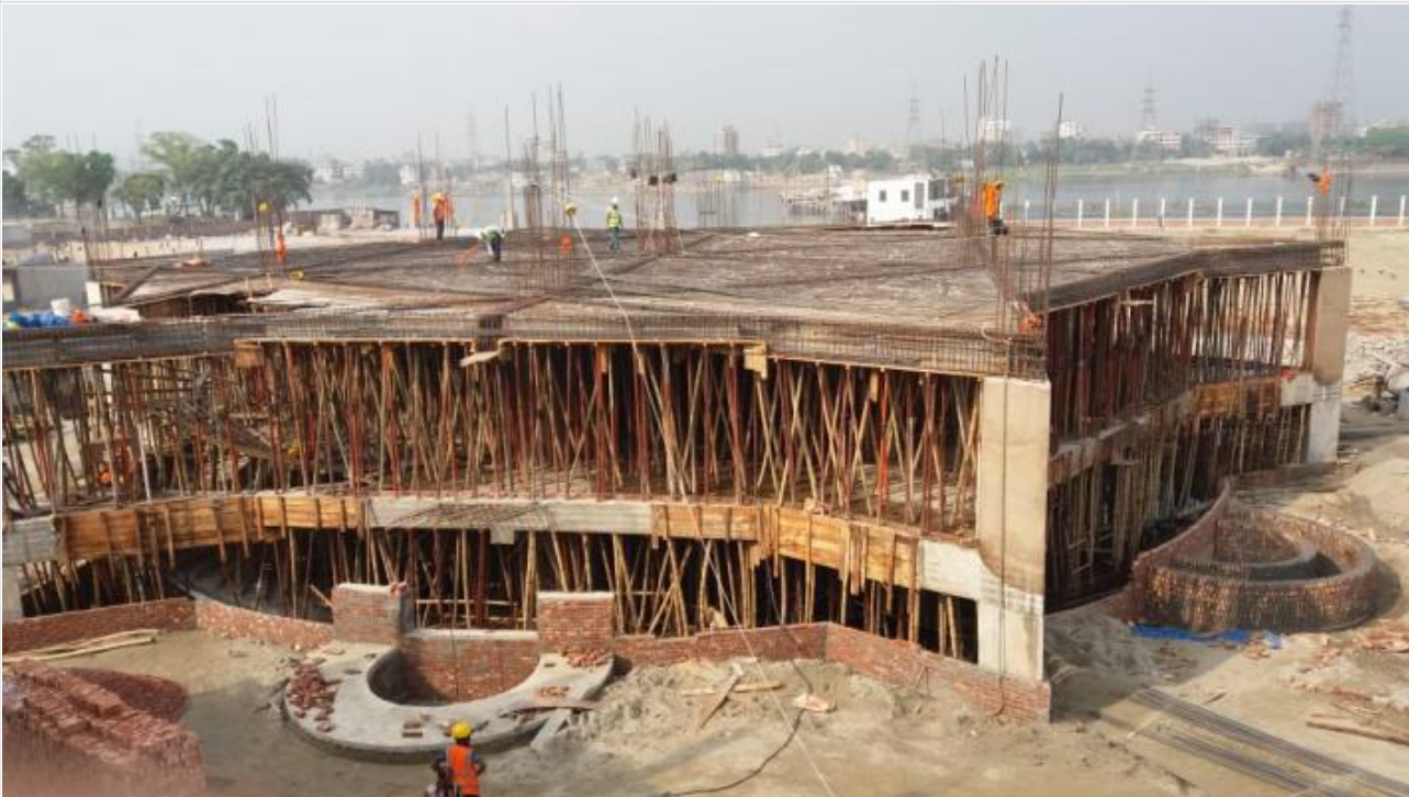
Mosque Building in Construction on 03-04-21
