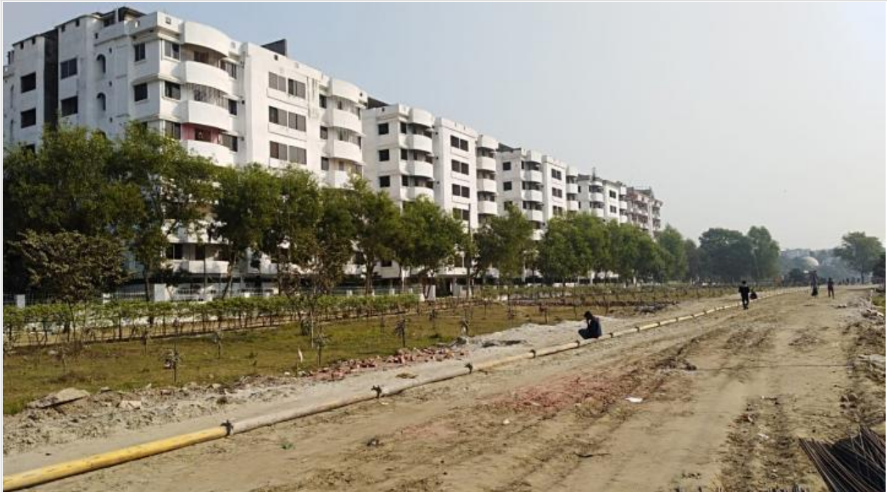
Building Outside Painting on 08-02-21
