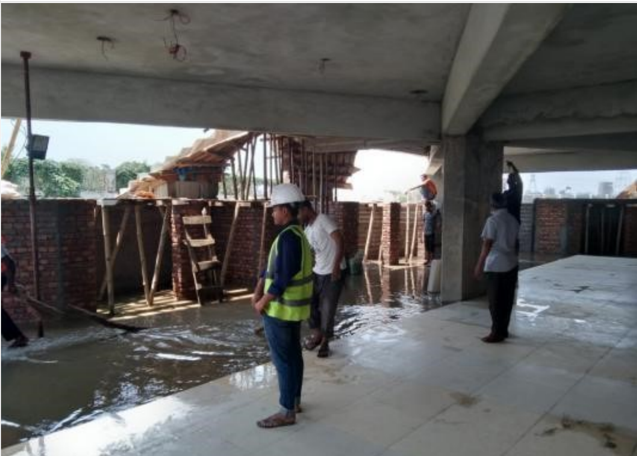
Mosque-Basement-Ancliary Work on 17-04-21
