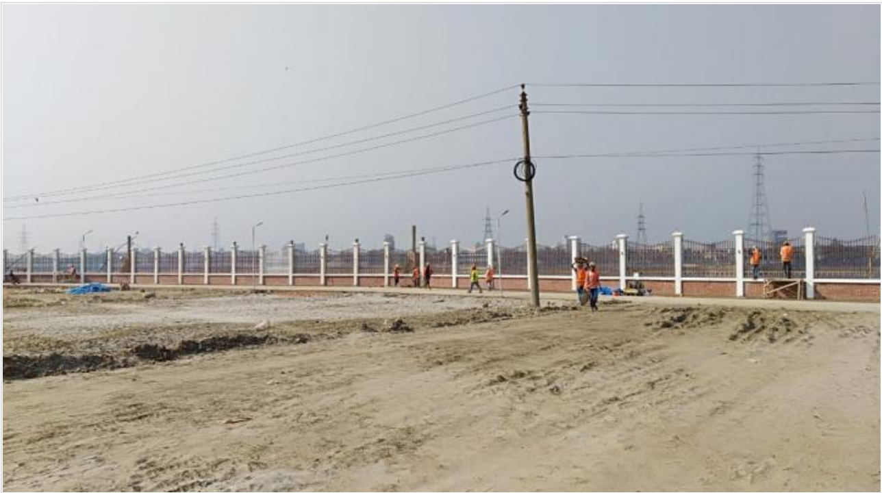
Riverside Boundary Fencing on 08-02-21
