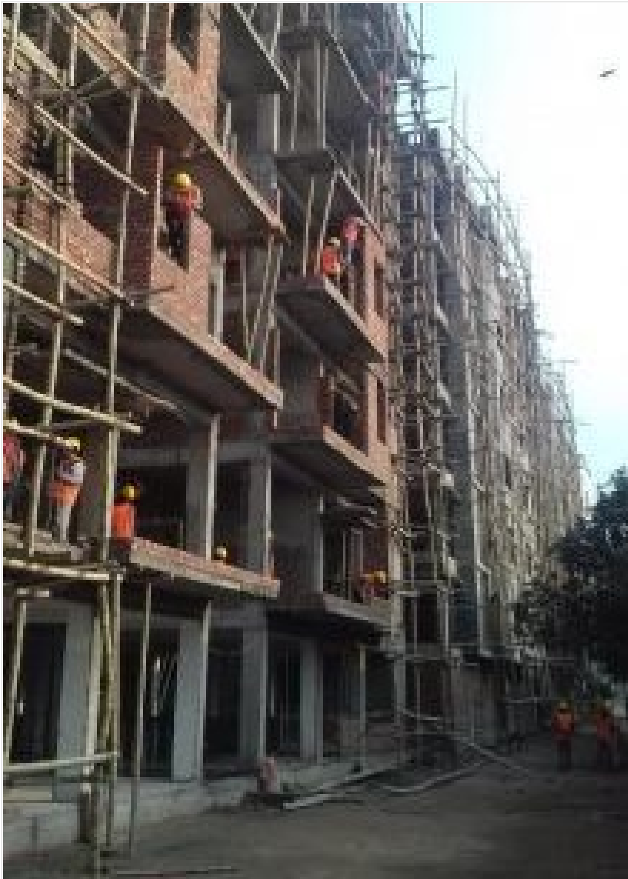
Scaffolding for outside plastering Build on 29-01-21
