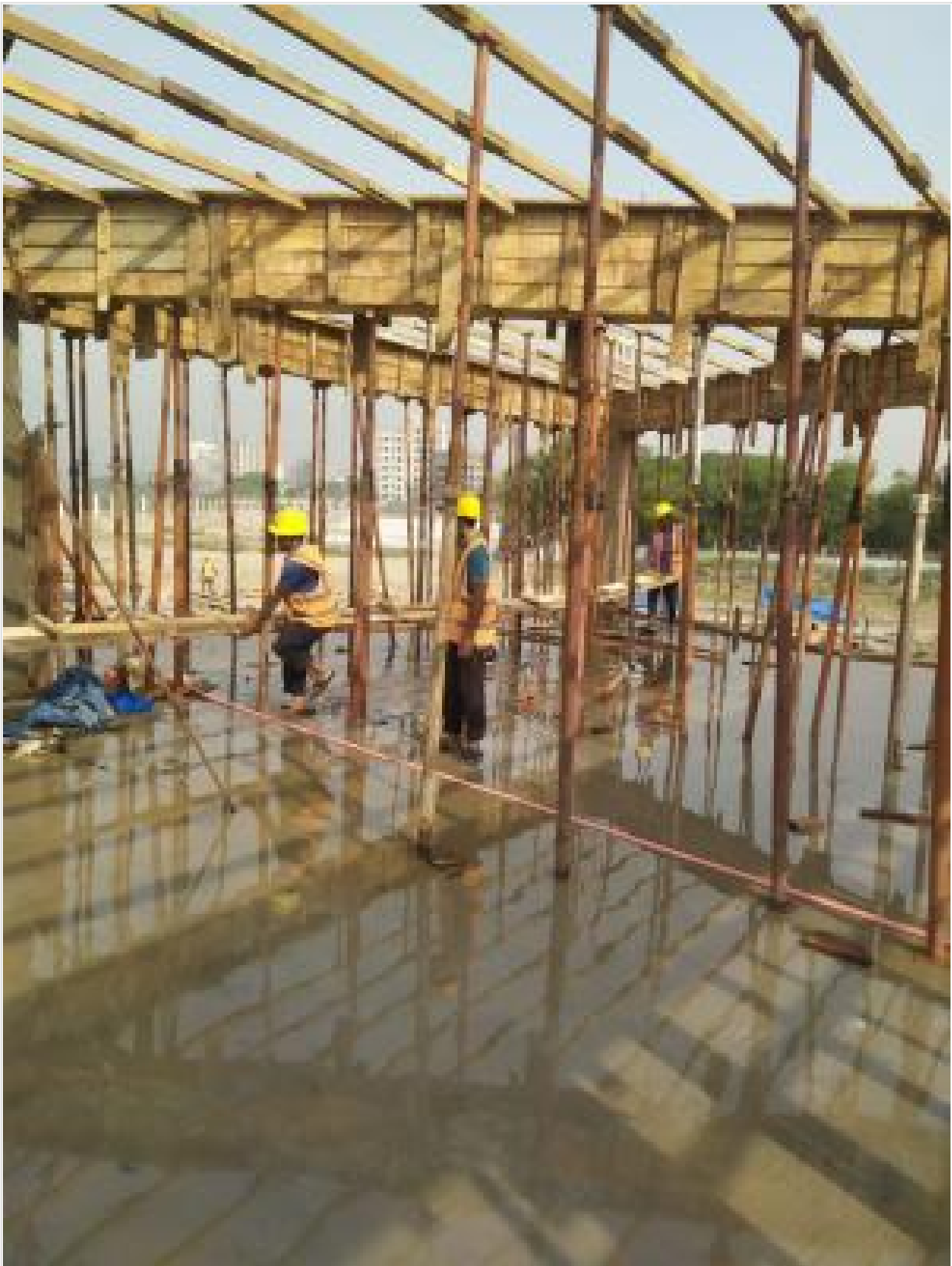
Mosque 1st Floor Slab Shuttering on 27-03-21
