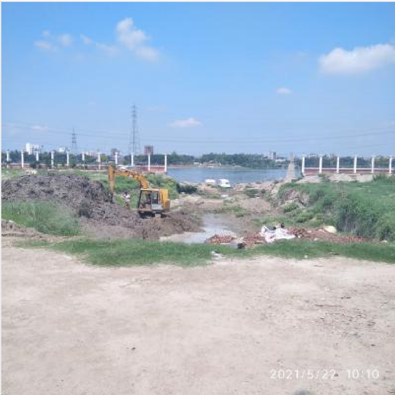
Landing Station-Excavation on 22-05-21
