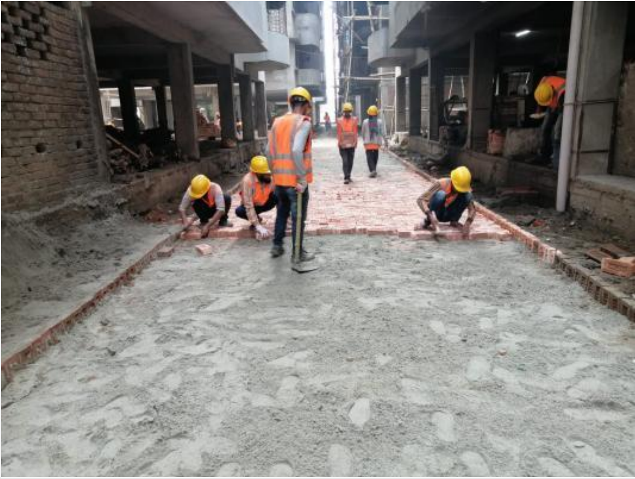
Inner Road CC Work on 27-01-21
