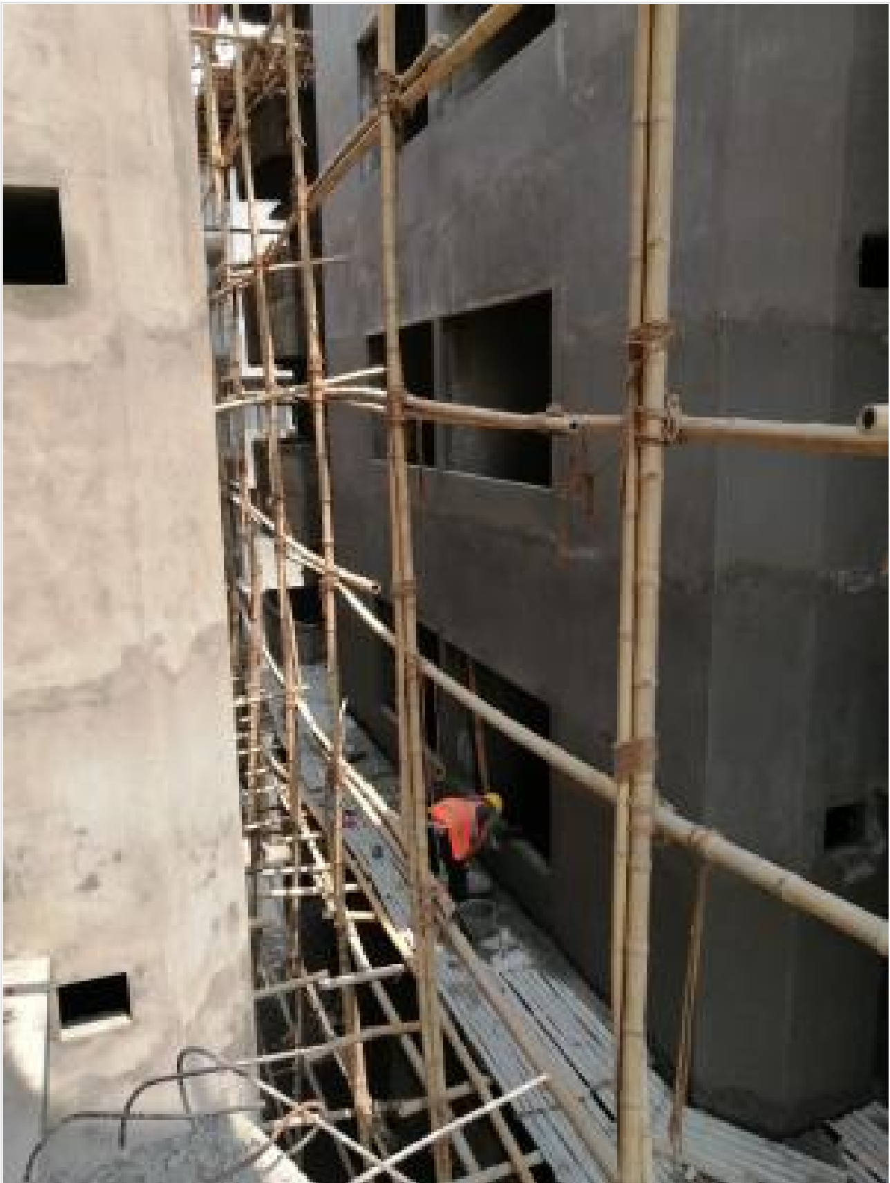
Out-side Plastering on 02-05-21
