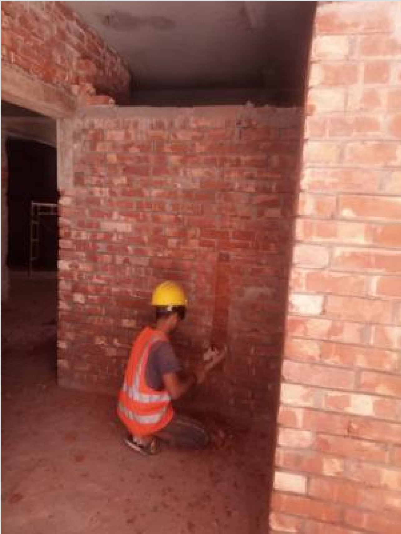
Electrical Conduit Conesealing on 25-02-21
