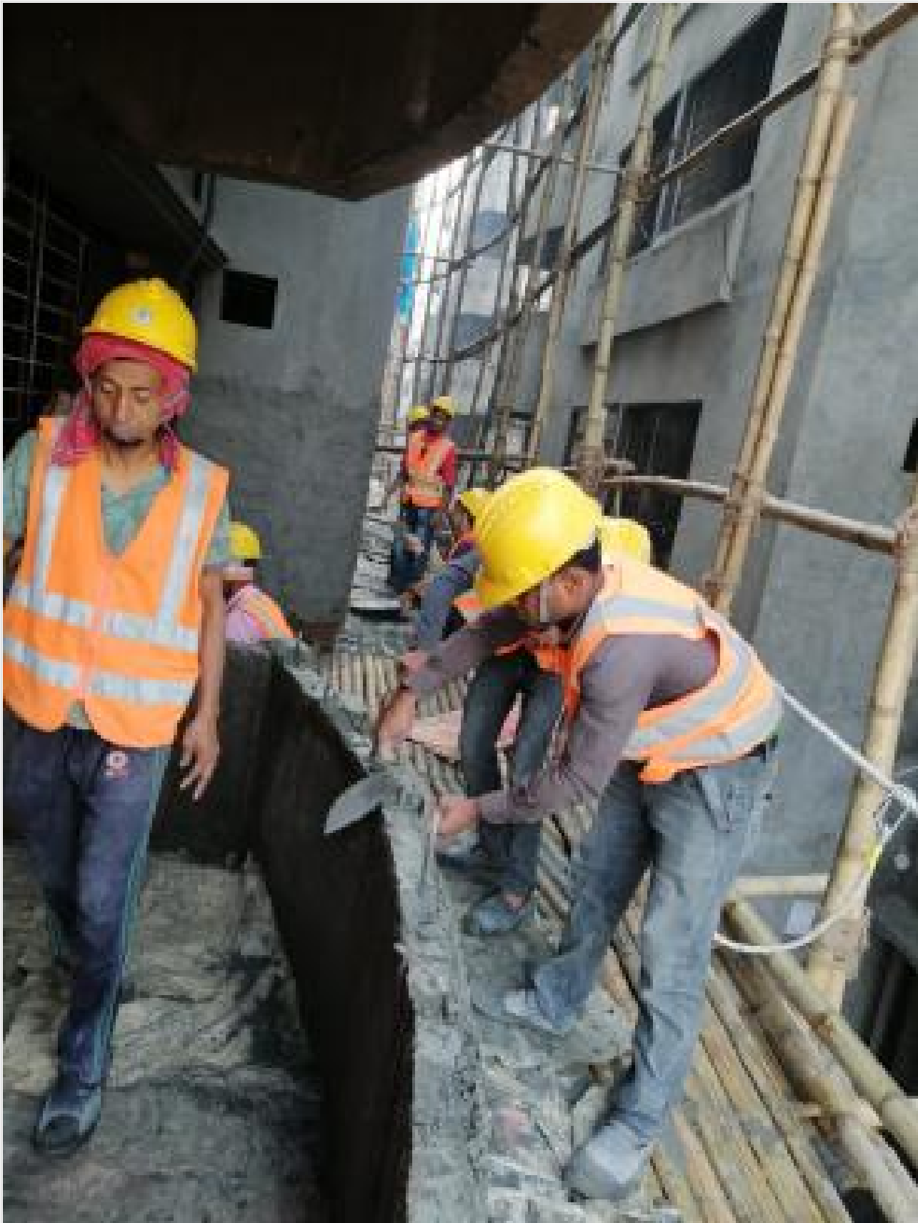
Out-side Plaster Work on 05-02-21
