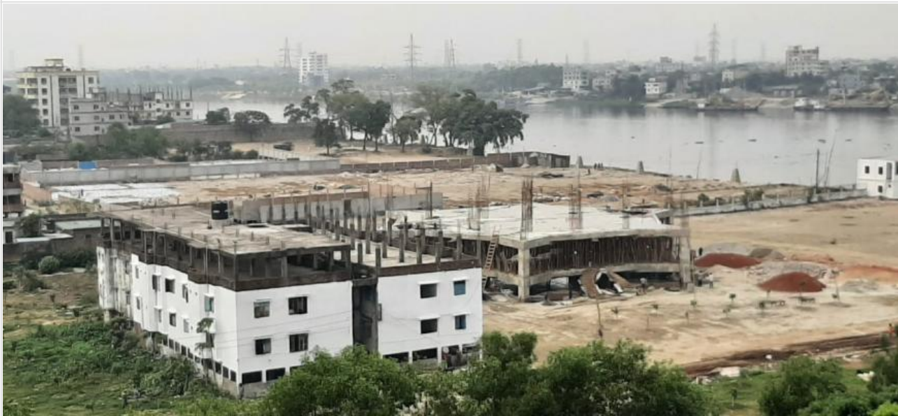
Mosque in Construction on 15-04-21
