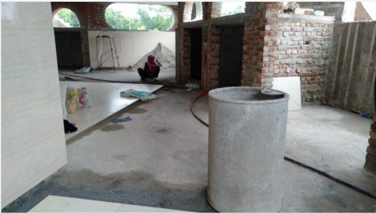
Mosque-Basement-Tile Work on 31-05-21
