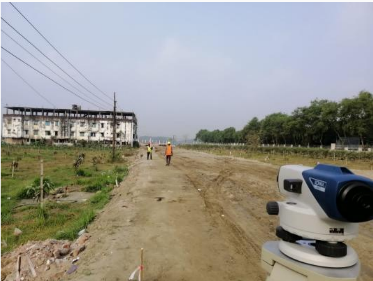
40 ft Road Dressing and Levelling on 01-03-21
