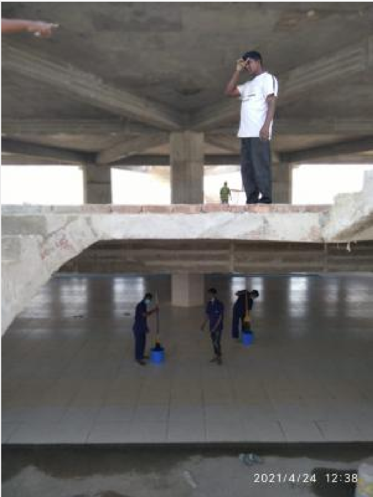
Mosque-Gr.Floor Roof De-shuttering on 24-04-21
