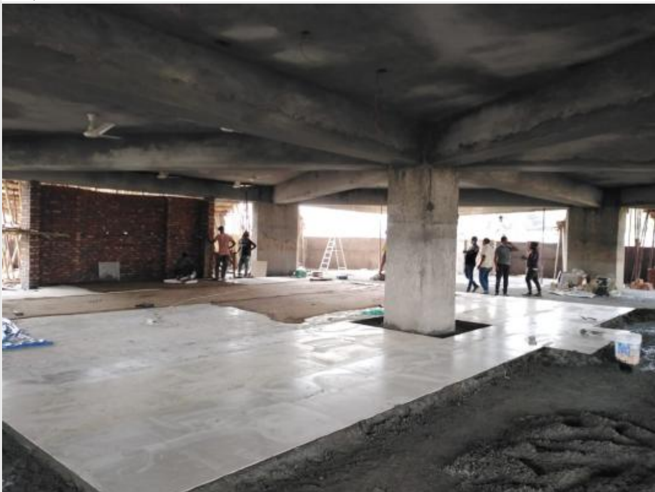
Mosque-Basement Tiles Work on 11-04-21
