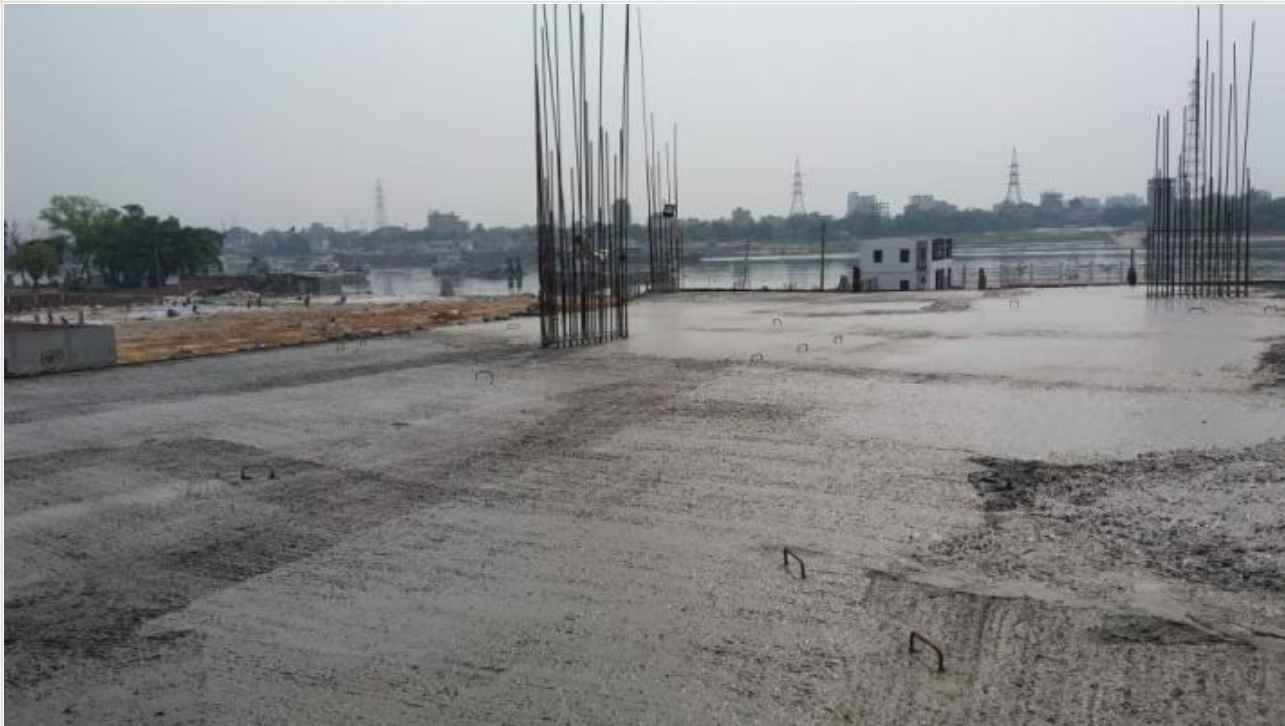
Mosque 1st Floor Slab Concreting on 06-04-21
