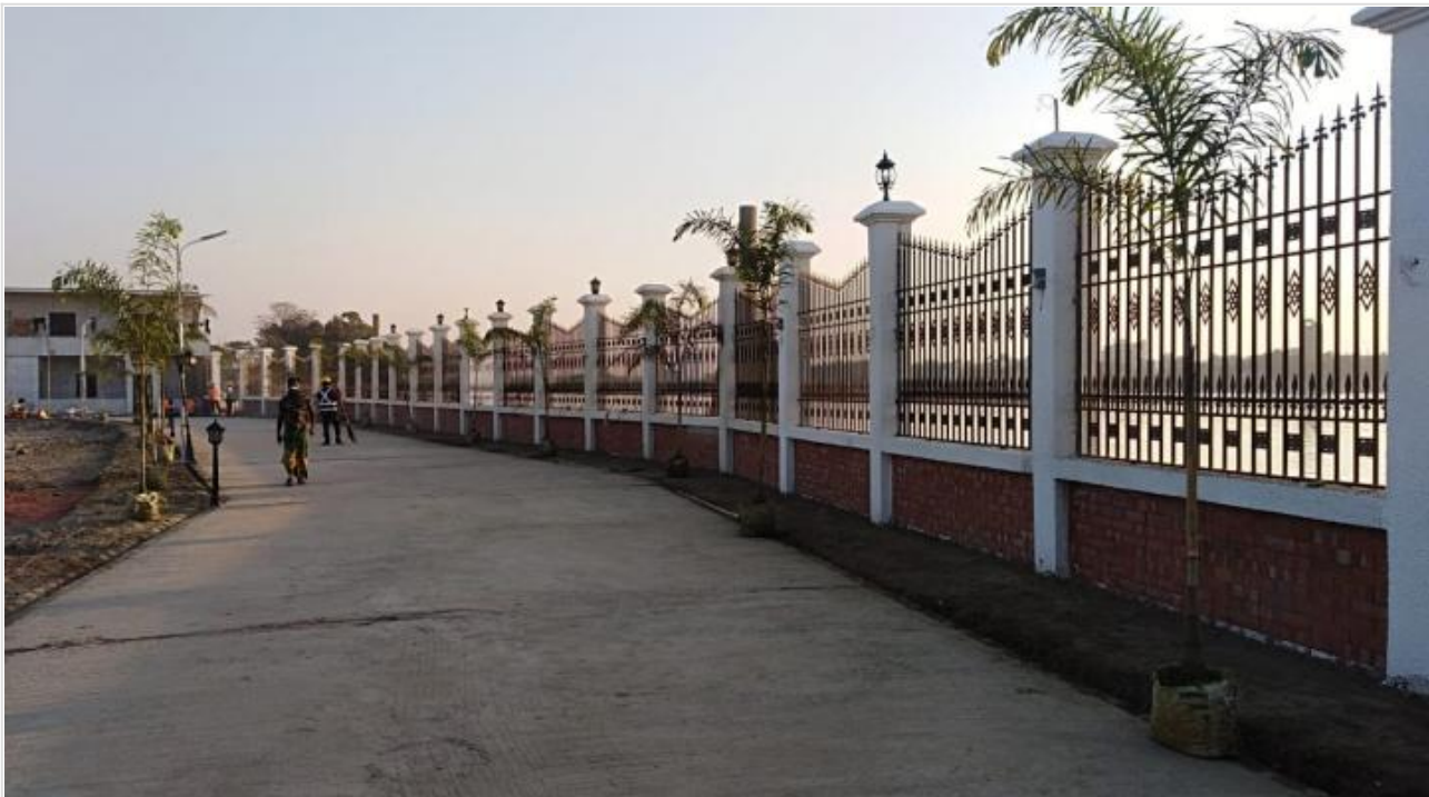
River Side Boundary Fencing on 10-02-21
