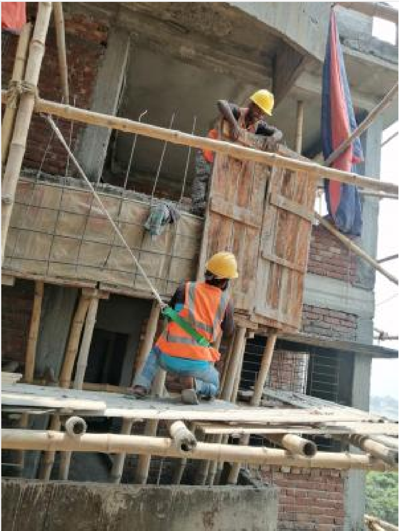
Drop Wall Shuttering on 01-05-21
