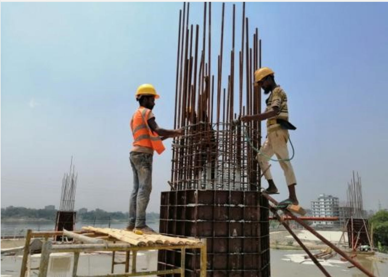
Mosque-1st Floor Column Re-bar Work on 19-04-21
