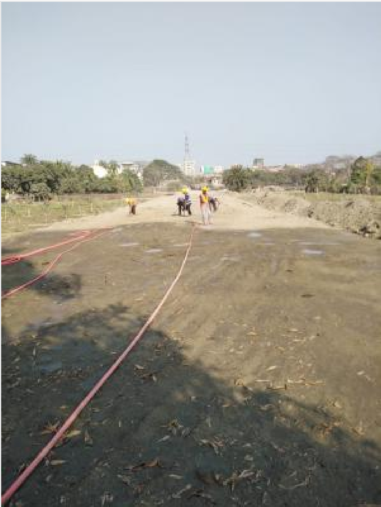
40 ft Road Dressing and Levelling on 28-02-21
