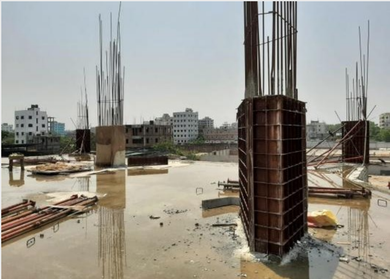
Mosque-1st Floor-Column Shuttering on 26-04-21
