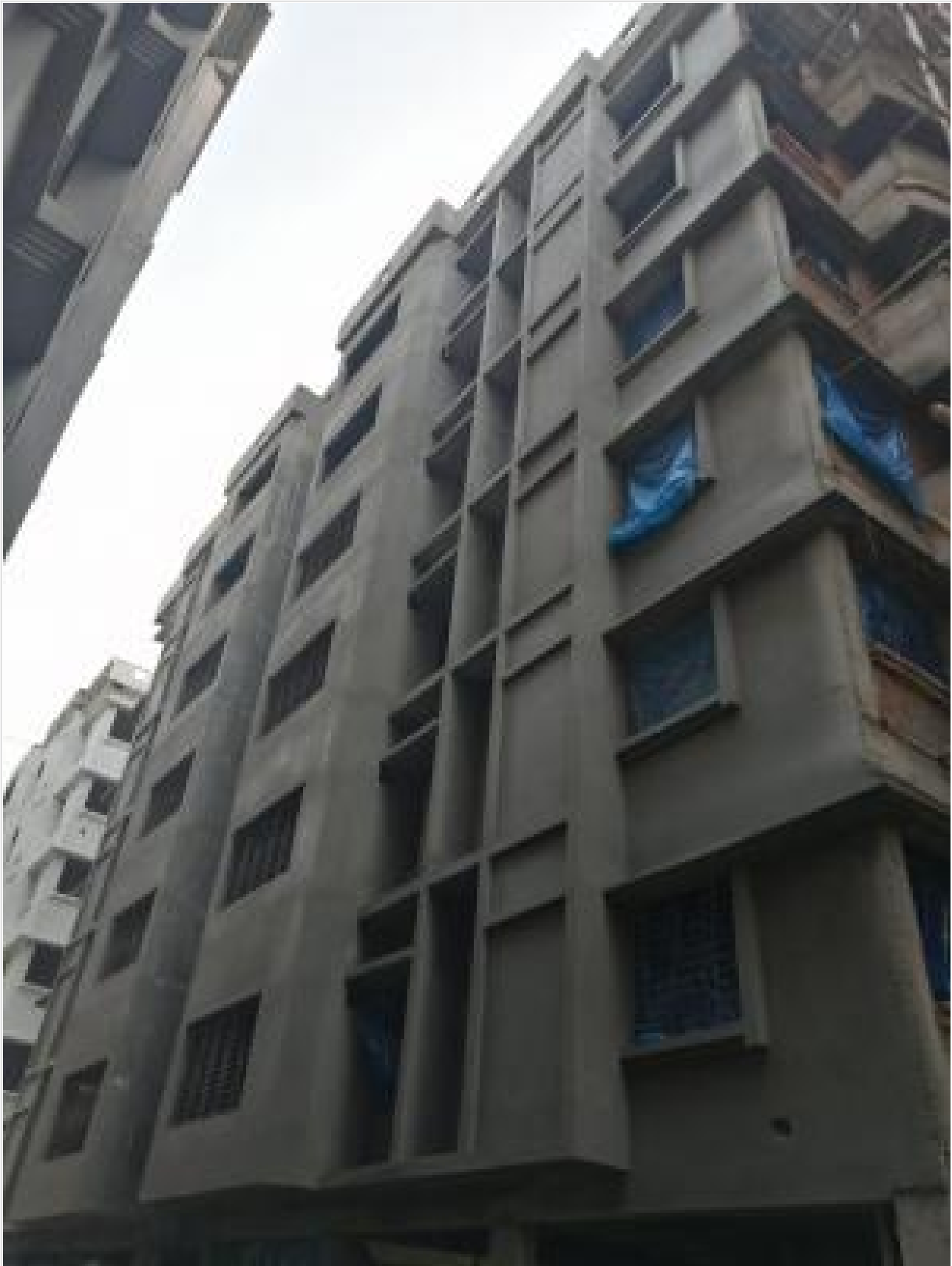
Building-J outside plastering on 28-01-21
