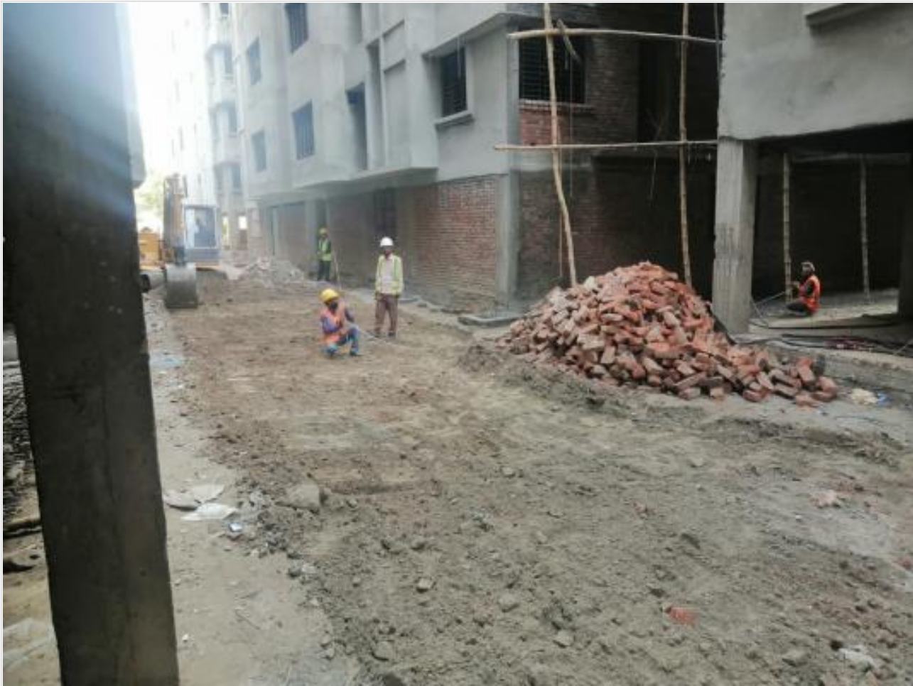
12 ft Road Filling on 28-02-21
