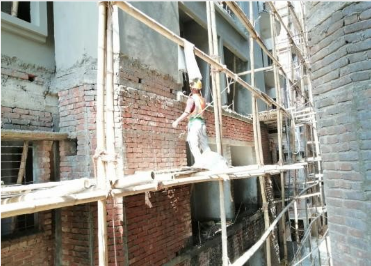
Out-side Plaster Work on 20-04-21
