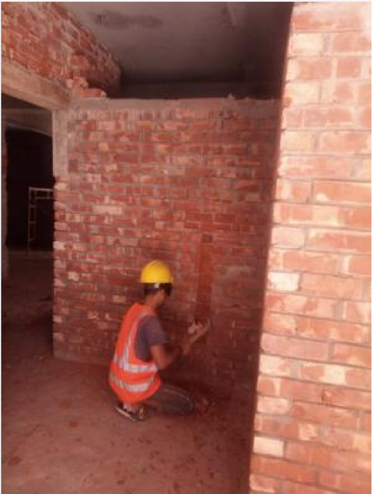
Electrical Conduit Consealing on 25-02-21
