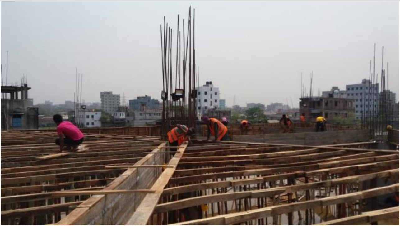
Mosque 1st Floor Slab Shuttering on 28-03-21
