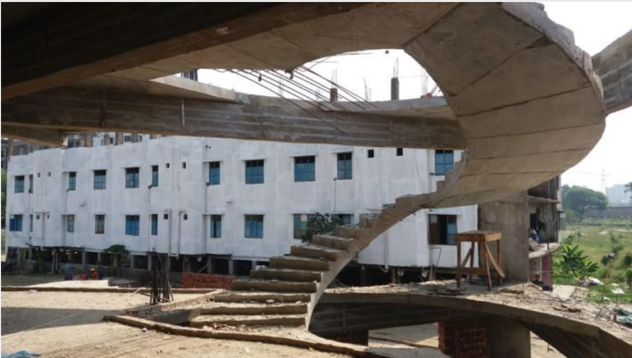
Mosque-Stair Case on 25-04-21
