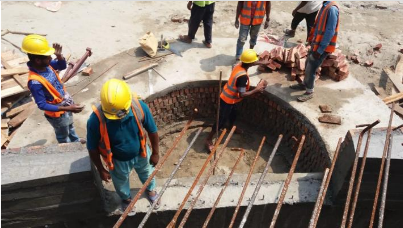
Mosque Ground Floor Stair Concreting on 28-03-21
