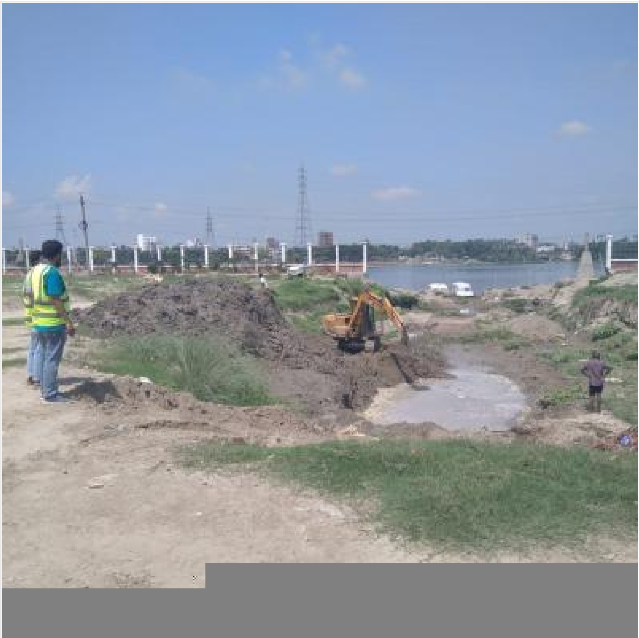
Landing Station-Excavation on 22-05-21
