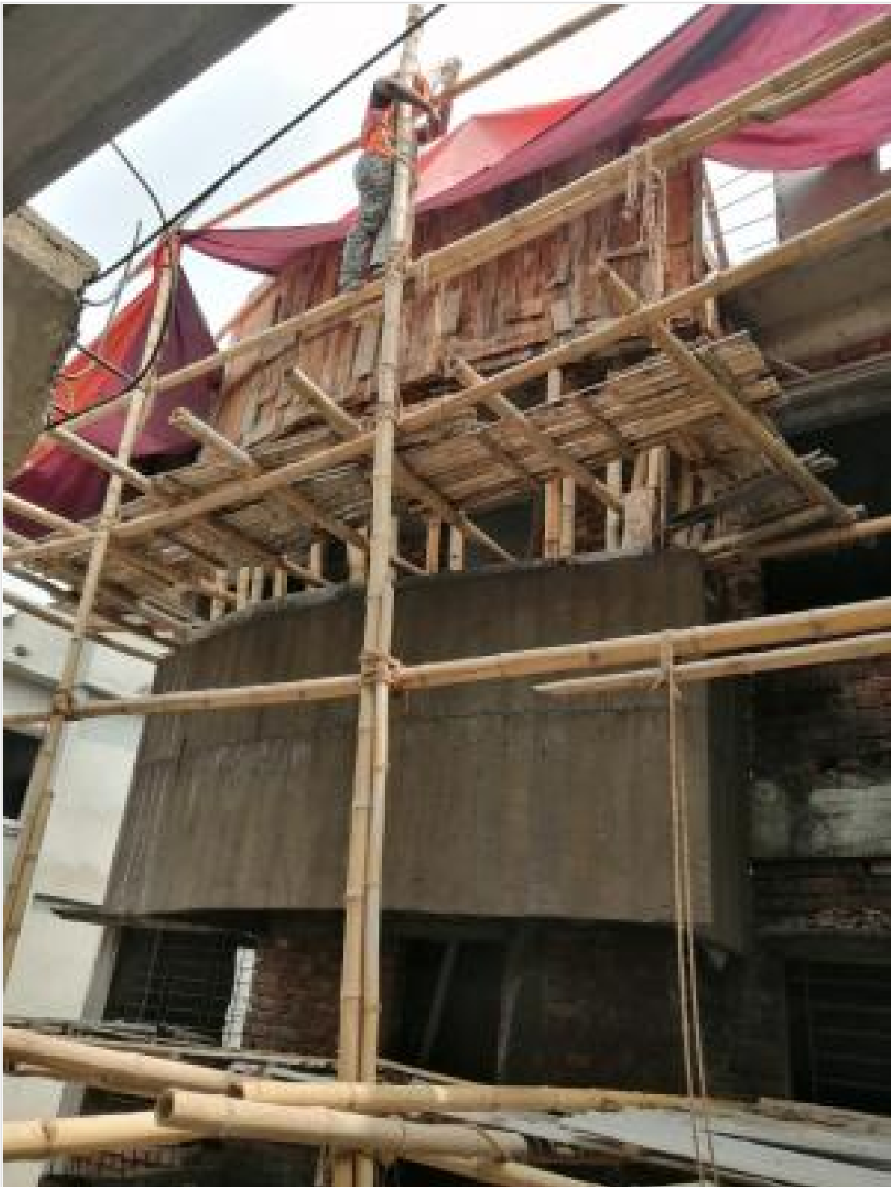
Drop Wall Shuttering on 28-04-21
