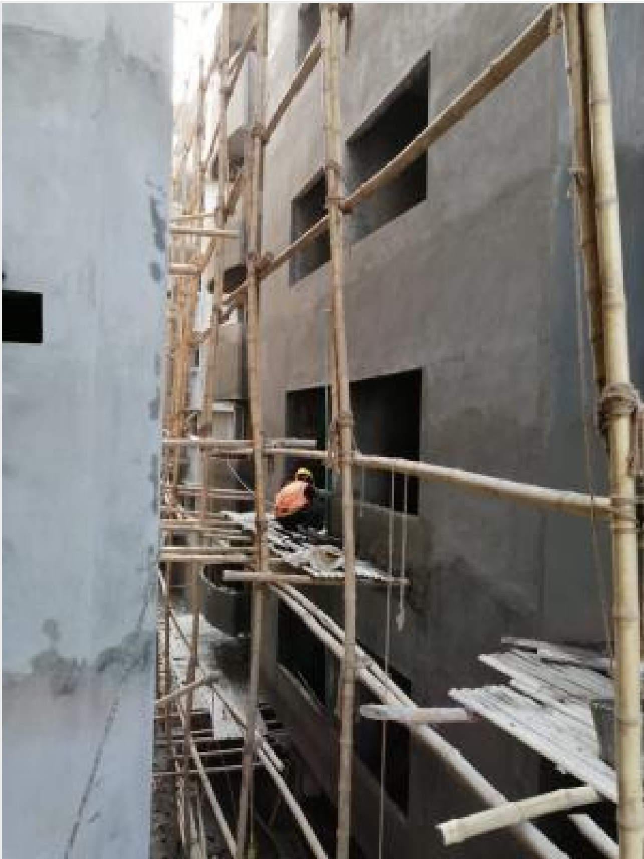
Bulding-Q-Out-side Plastering on 09-05-21
