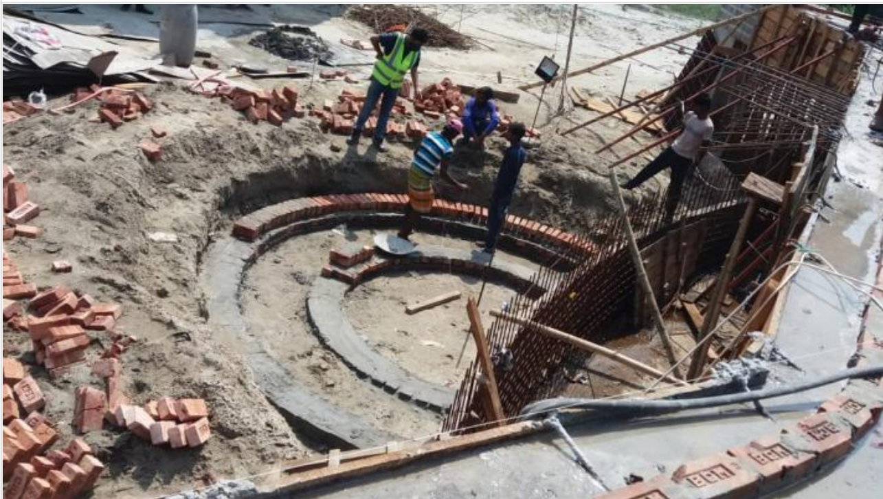
Mosque-GF-Stair Case Foundation Work on 25-03-21
