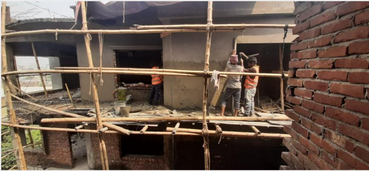
Out-side Plastering on 15-04-21
