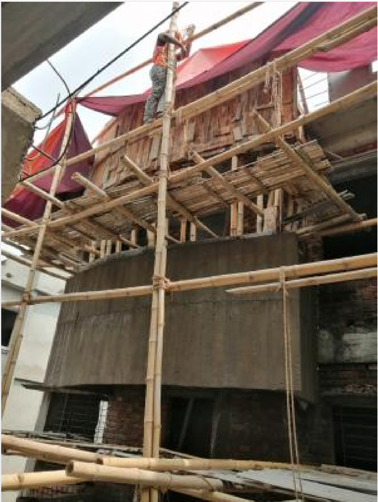
Drop Wall Shuttering on 28-04-21
