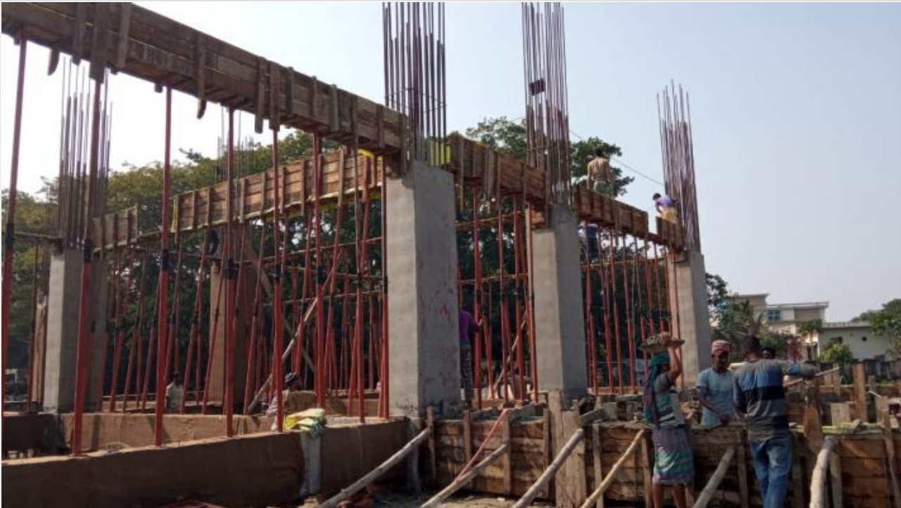
Tower-1-GF Beam Shuttering on 15-12-20
