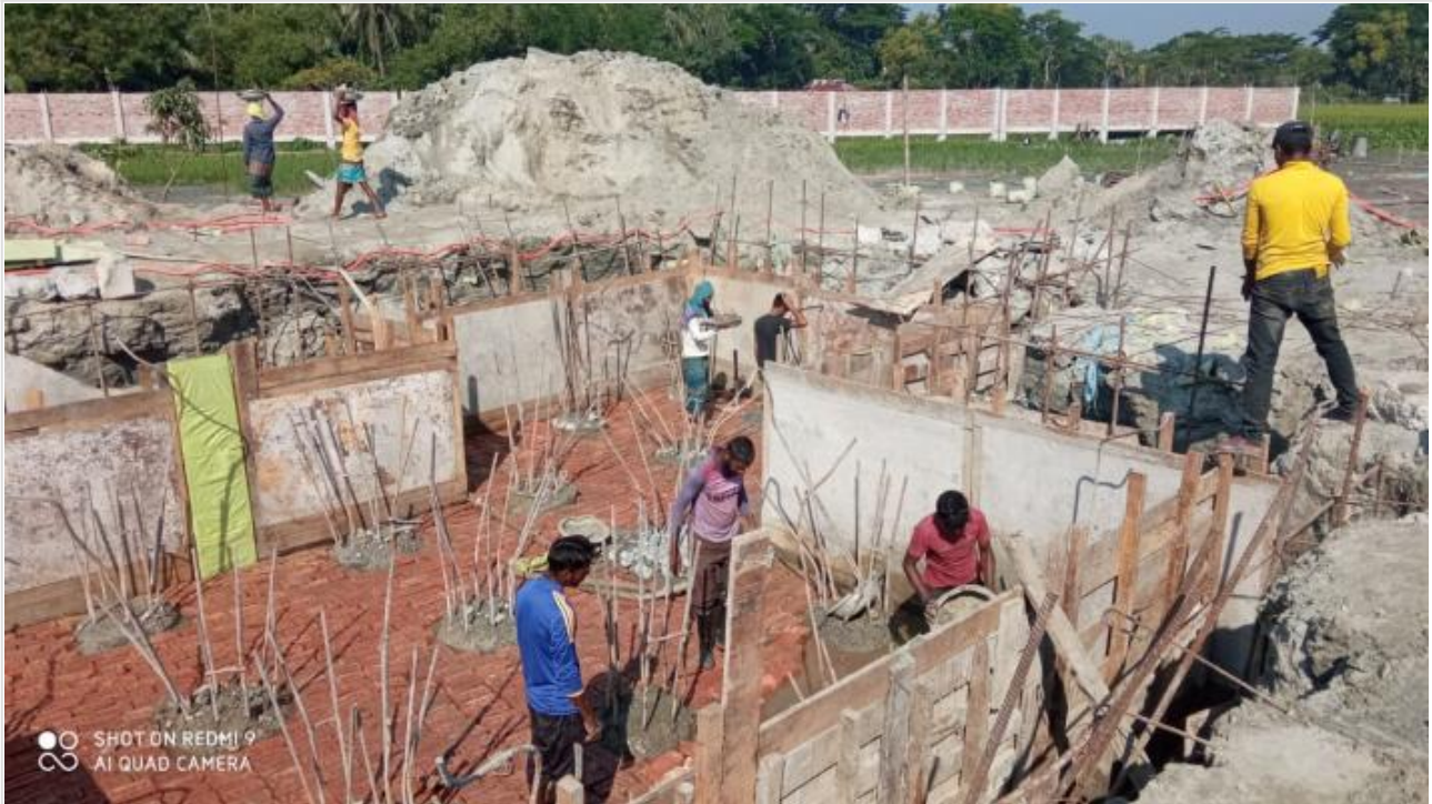
Tower-1-Pile Cap Work on 28-11-20
