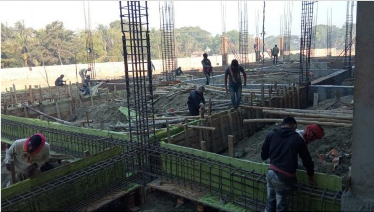
Tower-2-Grade Beam Shuttering on 10-02-21
