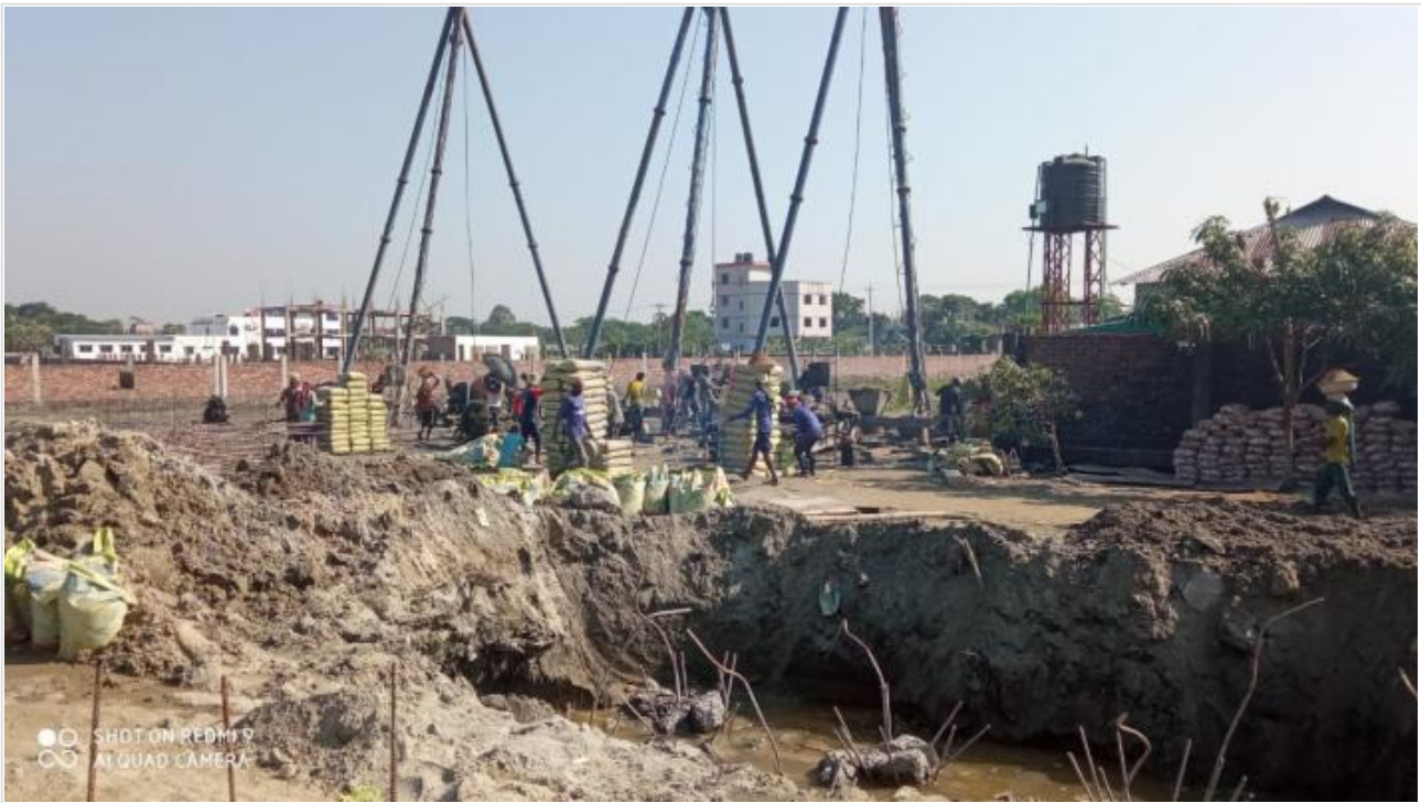
Tower-2-Piling Work on 28-11-20
