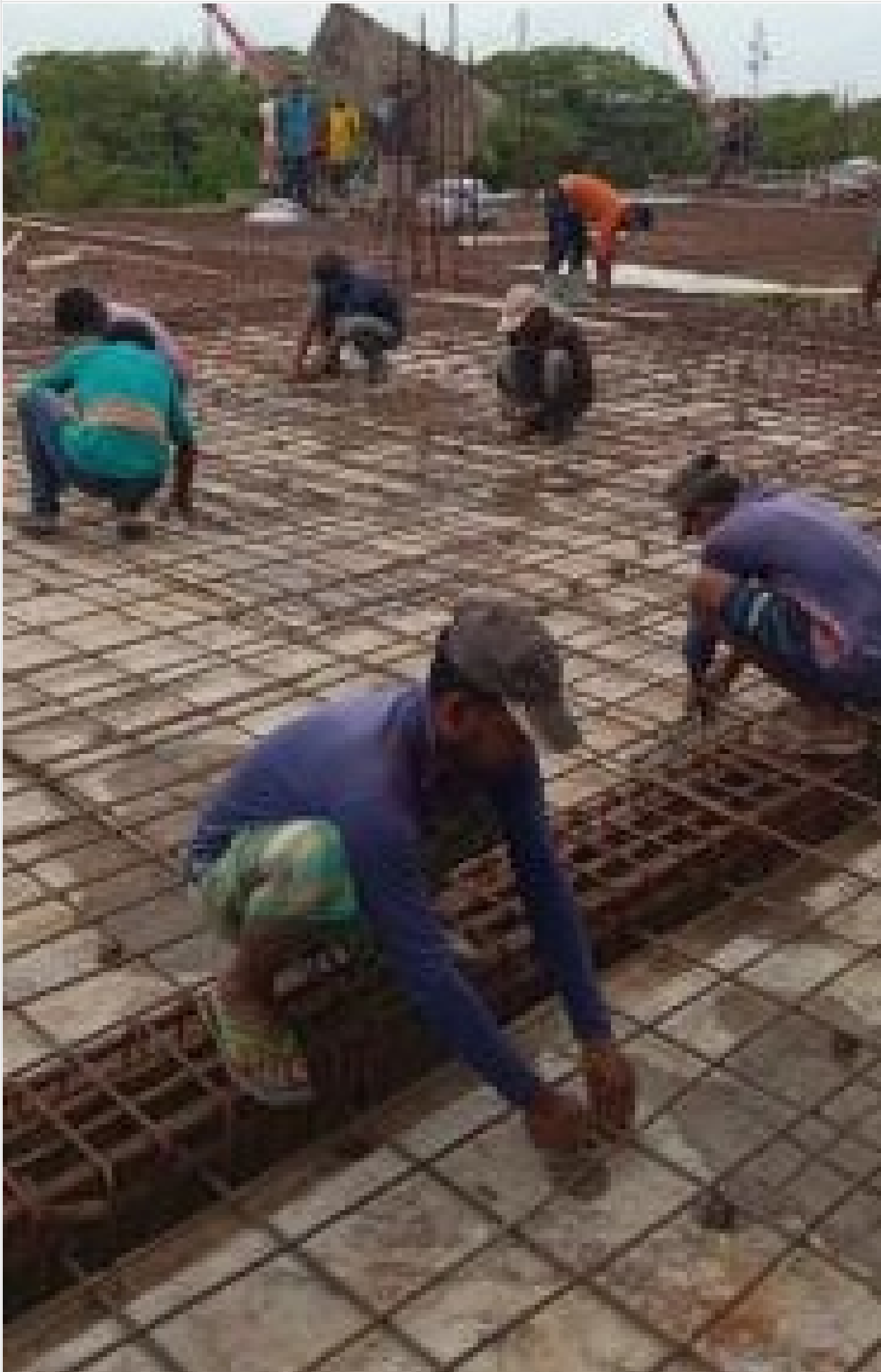
Restaurant-3rd Floor Slab Concreting on 12-06-21
