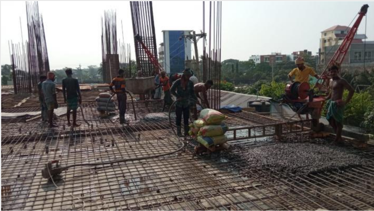
Between Tower1-2-GF Roof Slab-Concreting on 26-04-21
