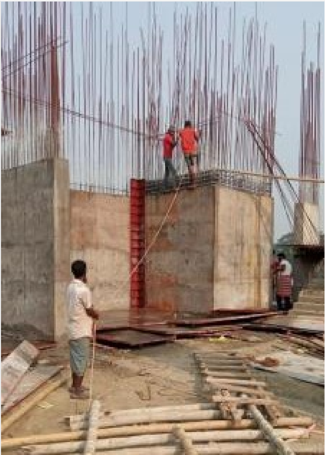
Tower-2: Lift Wall De-shuttering Work on 25-03-21
