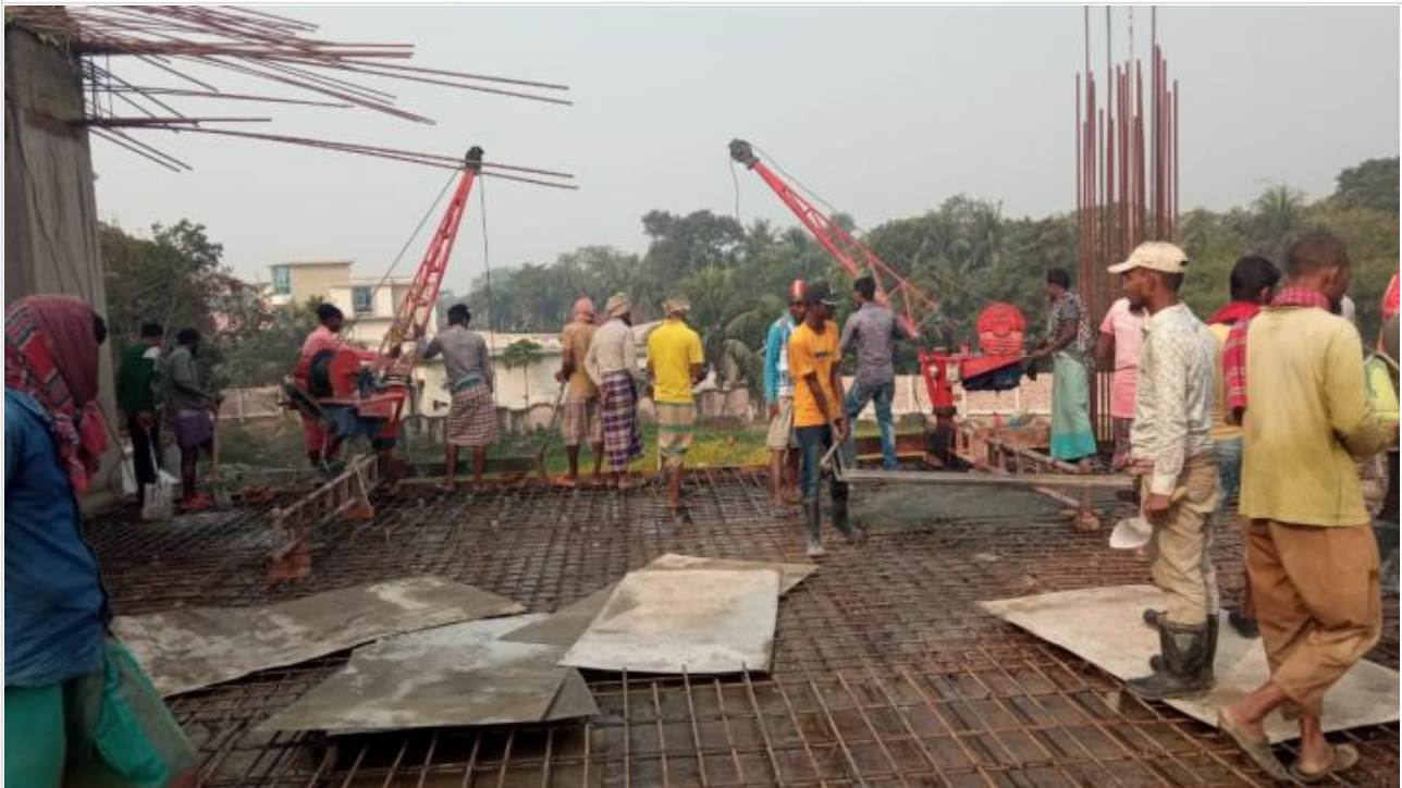
Tower-1-GF Roof Slab Concreting on 16-01-21
