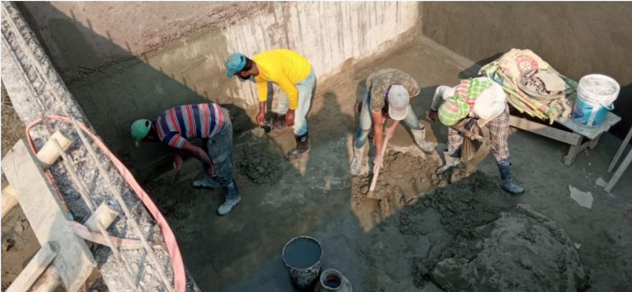
East Septic Tank Plastering on 01-02-22
