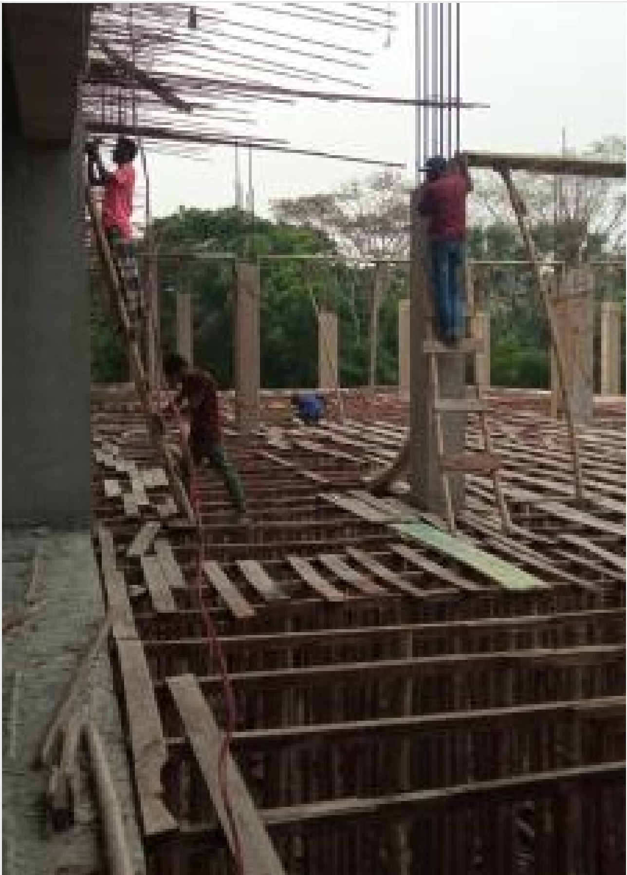
Tower-1-3rd Floor Roof Slab-Beam Shutter on 23-03-21
