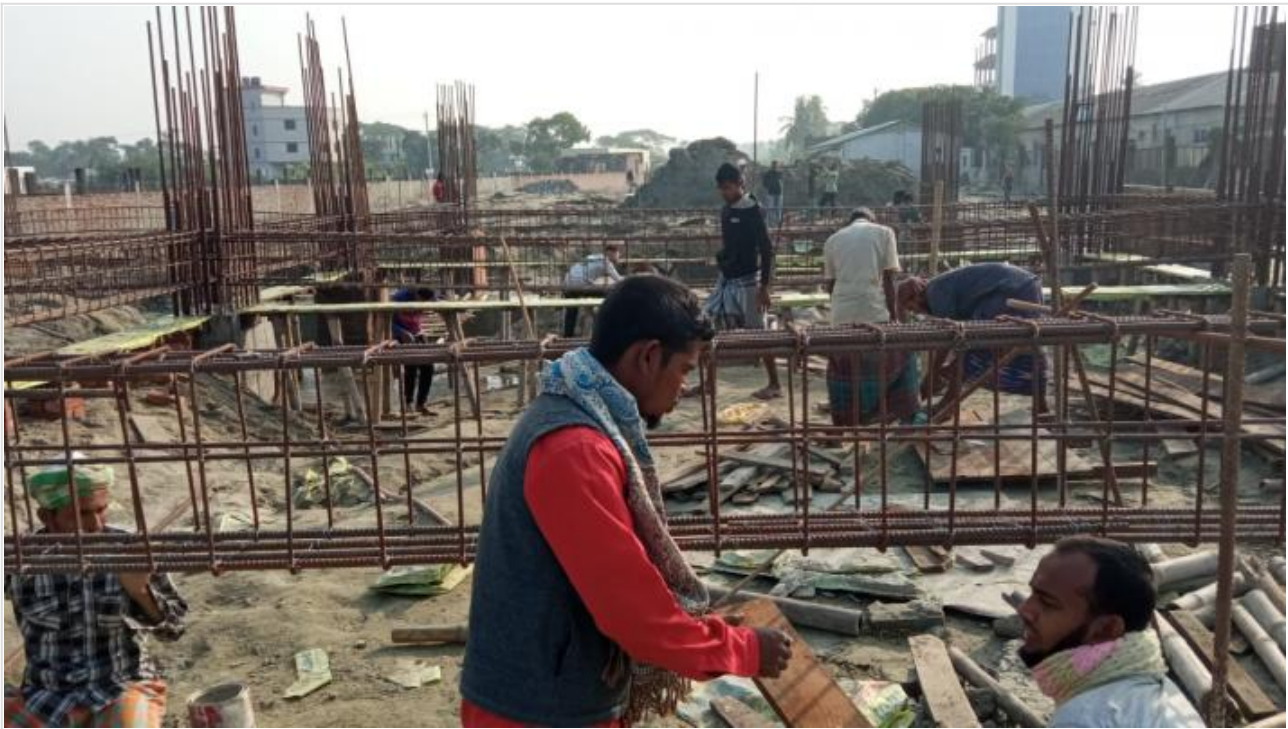
Tower-1-Grade Beam Re-bar Fabrication on 18-12-20
