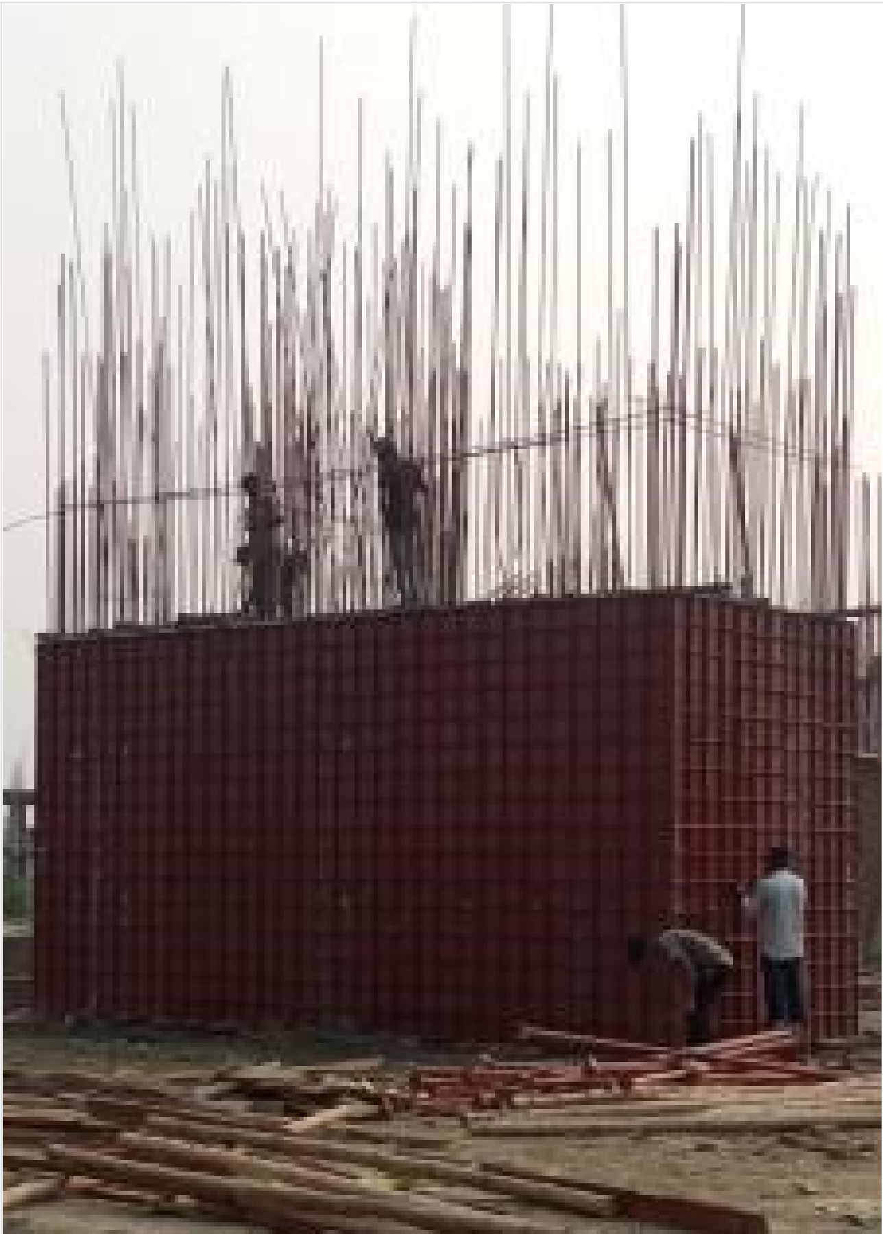
Lift Core Wall Shuttering on 24-03-21
