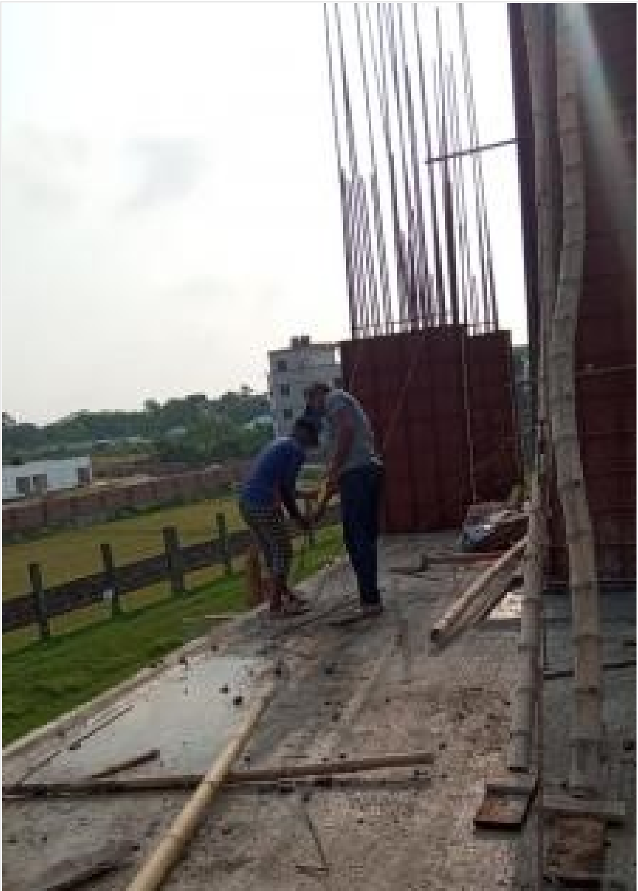
Column Shuttering Work on 30-04-21
