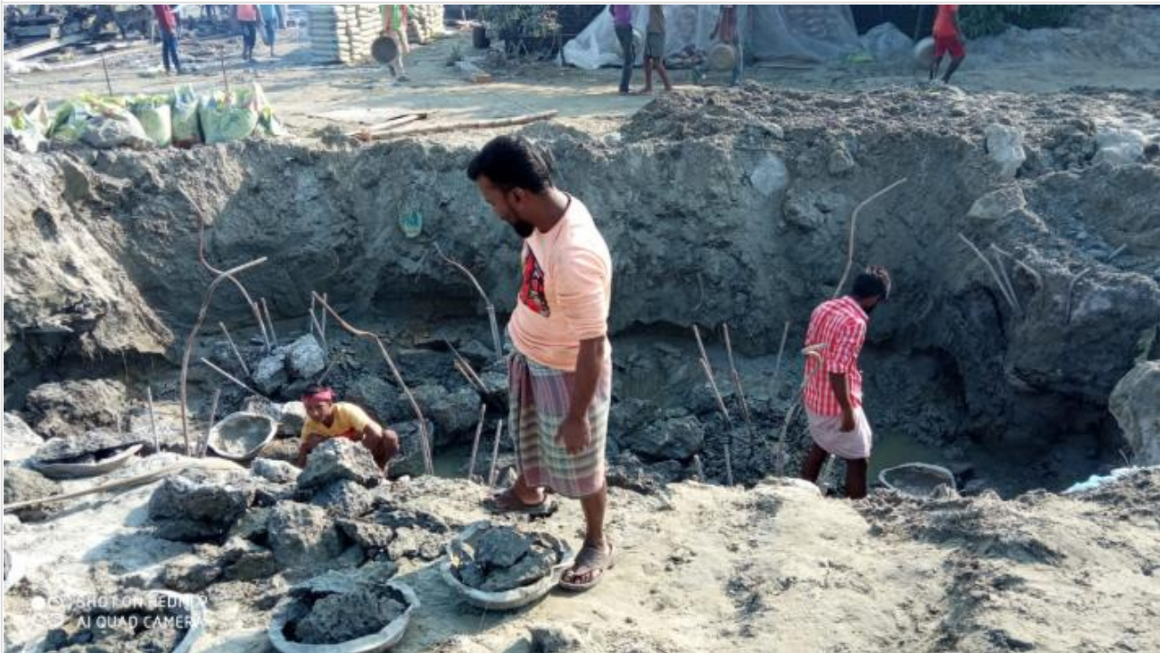
Tower-1-Pilehead breaking on 30-11-20
