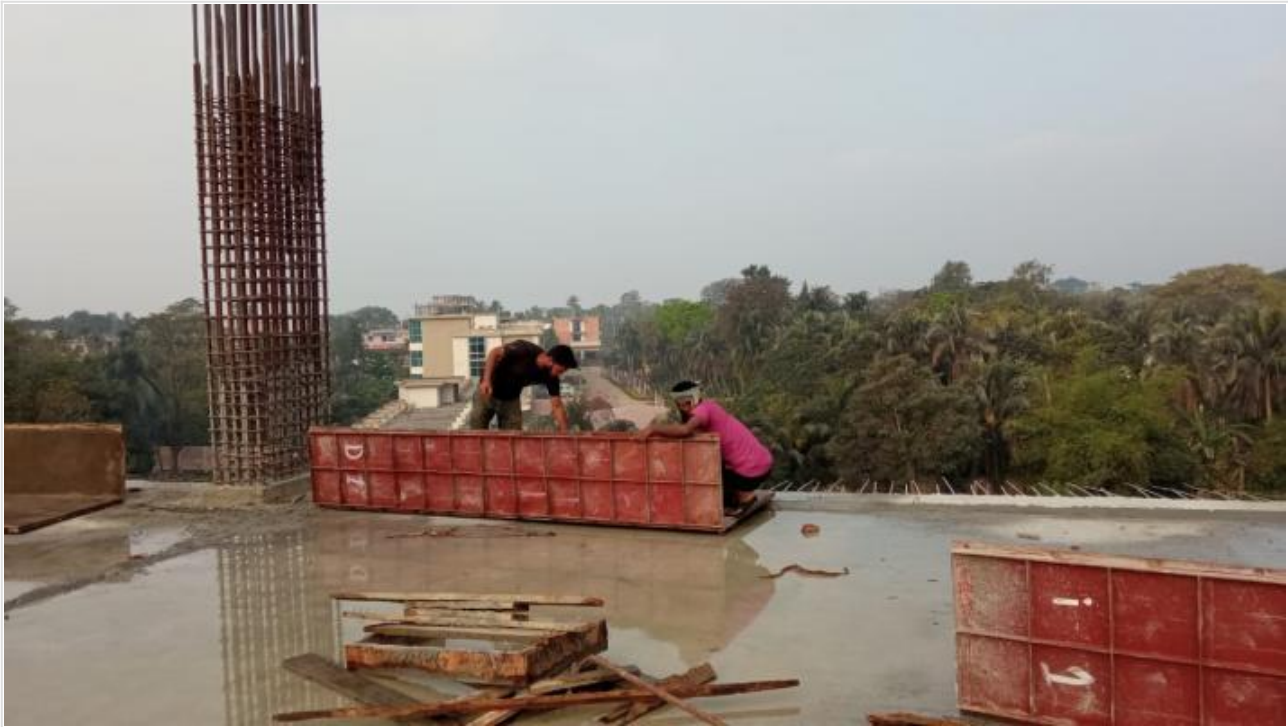
Tower-1-3rd Floor Column Shuttering on 28-02-21
