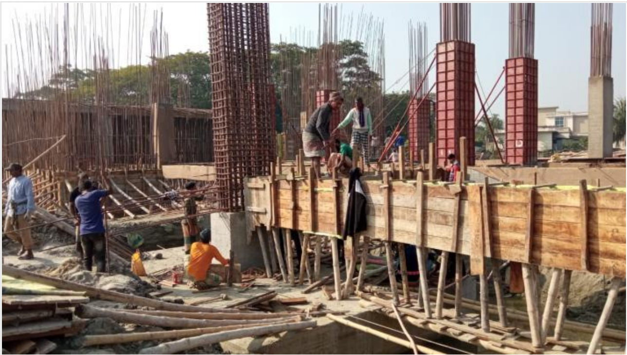
Tower-1-Grade Beam Shuttering on 24-12-20
