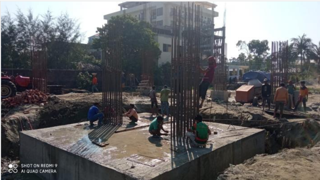
Tower-1 Pile Cap on 30-11-20
