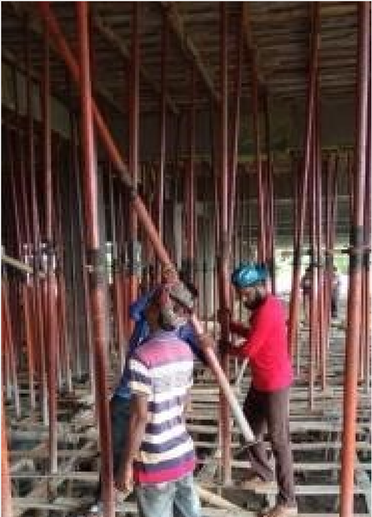
Roof Slab De-shuttering on 24-05-21
