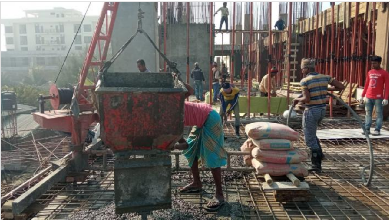
Tower-1-GF Roof Slab-4250sft Concreting on 27-01-21
