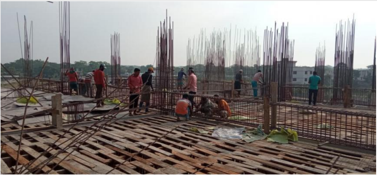
Roof Slab Shuttering on 04-05-21
