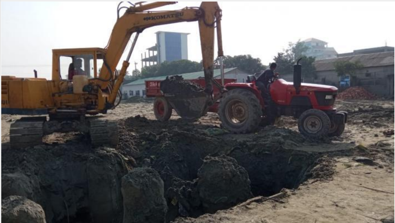
Tower-2-Excavation for Pile Head Breakin on 24-12-20
