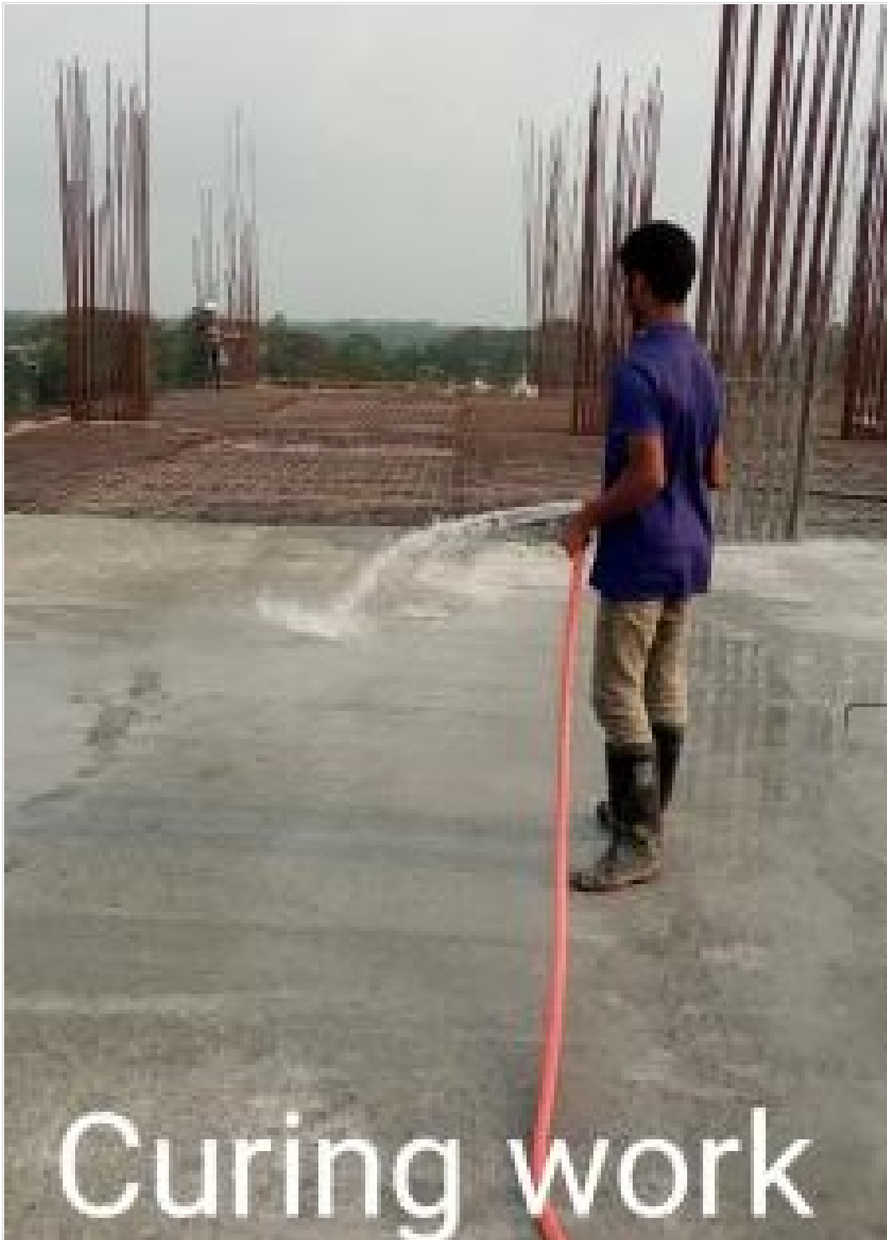
Tower-1-3rd Floor Roof Slab Curing on 31-03-21
