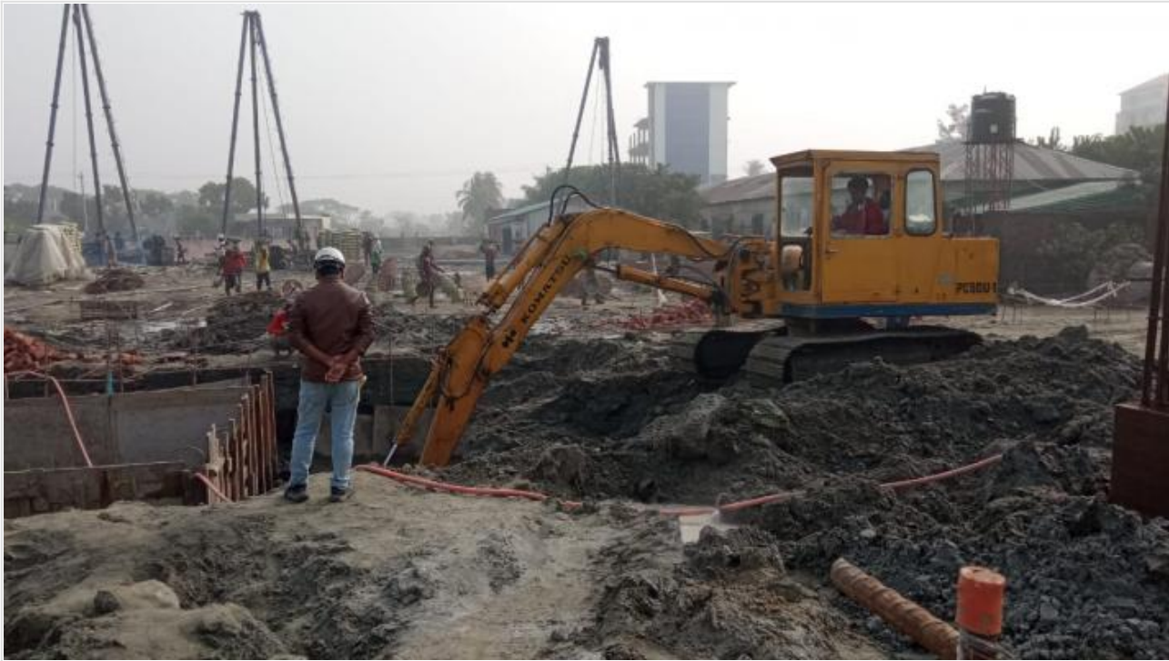
Tower-1-Excavation for Pile Cap on 09-12-20
