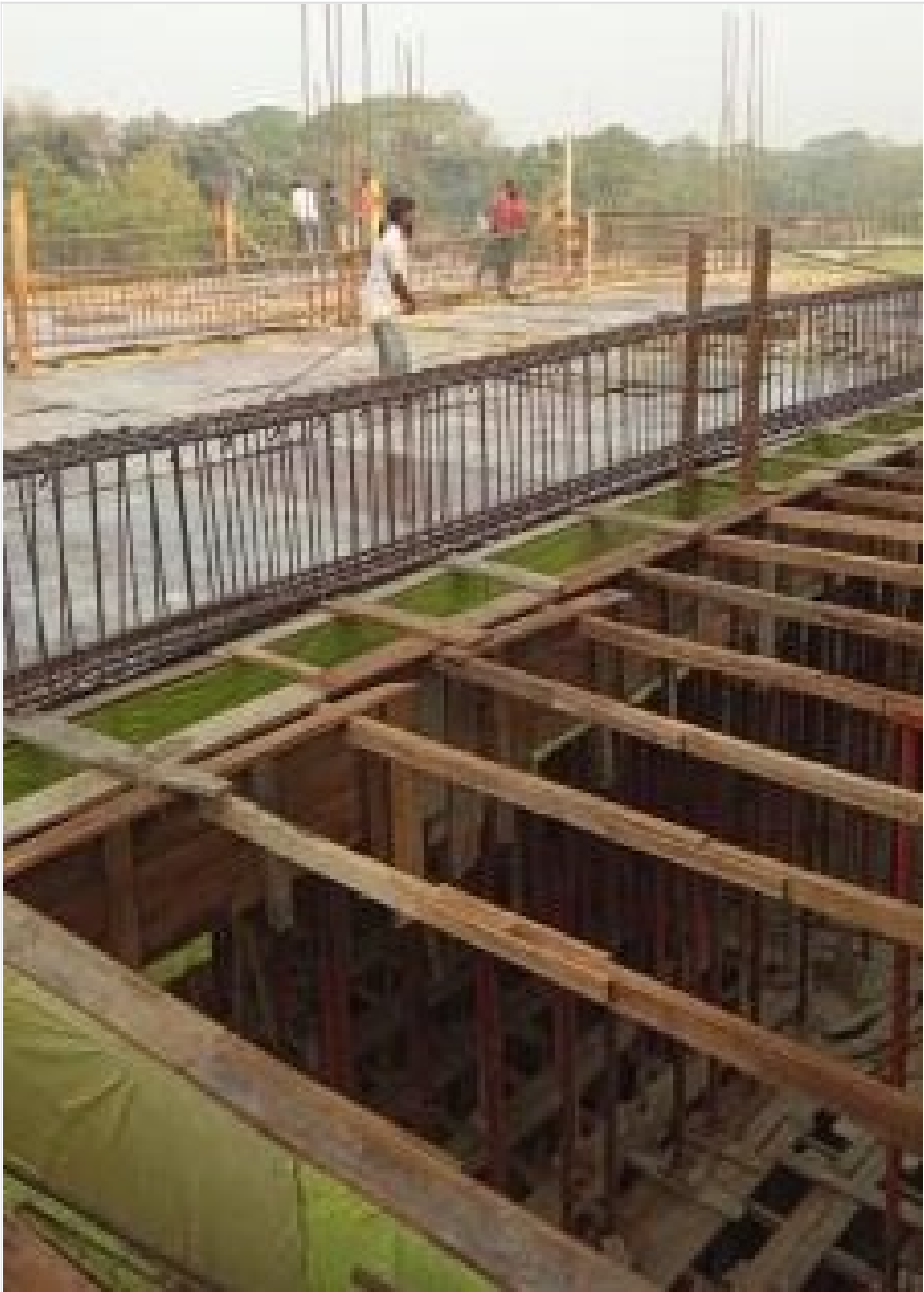
Tower-1-3rd Floor Roof Slab Shuttering on 13-03-21
