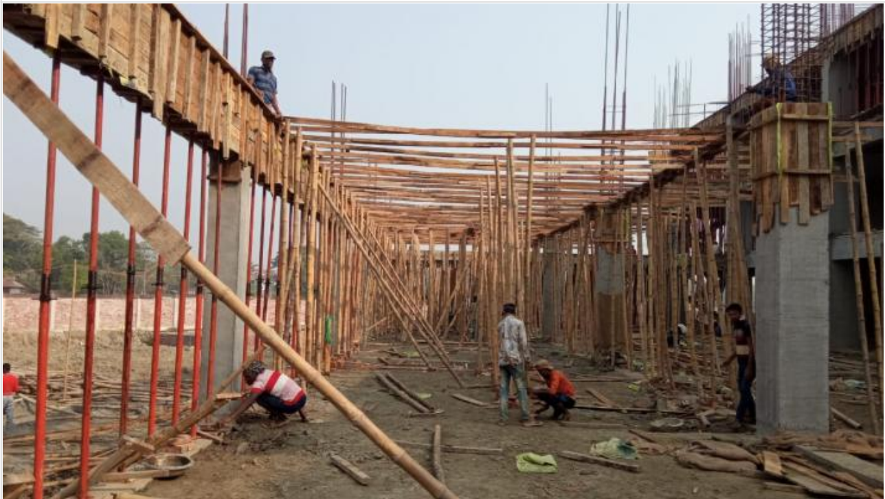
Restaurant Area Slab Shuttering on 23-02-21
