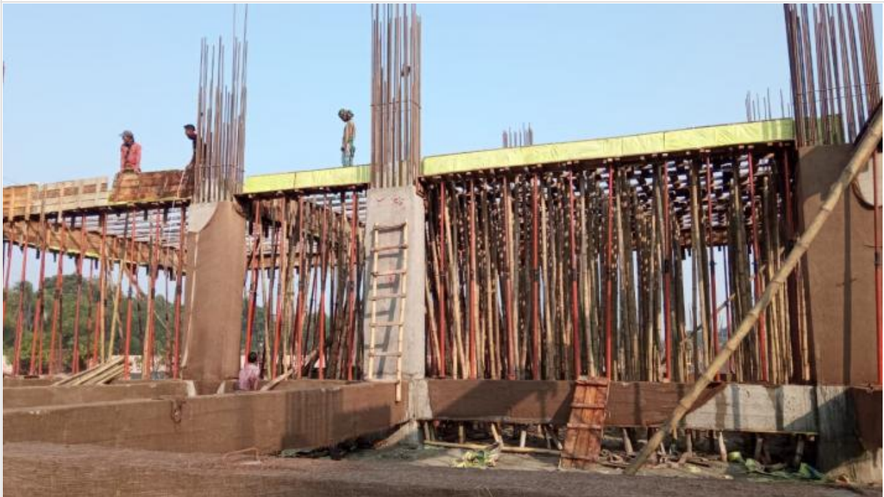
Tower-1-GF Beam Shuttering on 18-12-20
