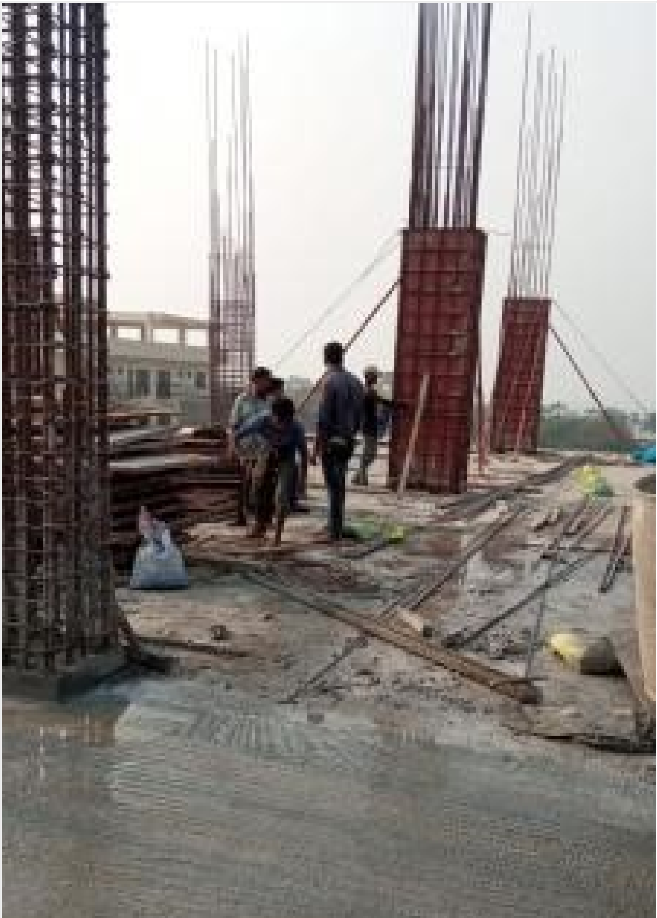
Column Shuttering Work on 25-03-21
