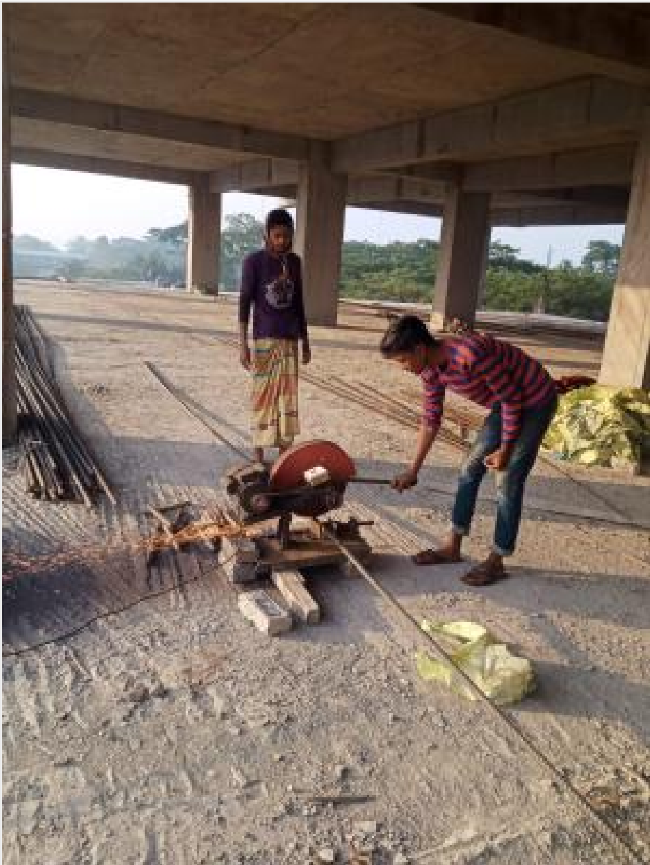
Re-bar Cutting on 08-01-22
