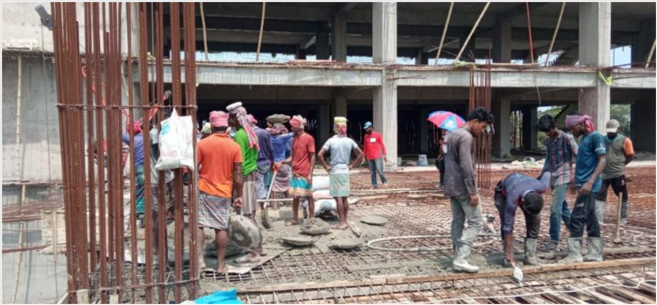
Between Tower1-2-1st Flr Roof Slab-Concr on 05-06-21
