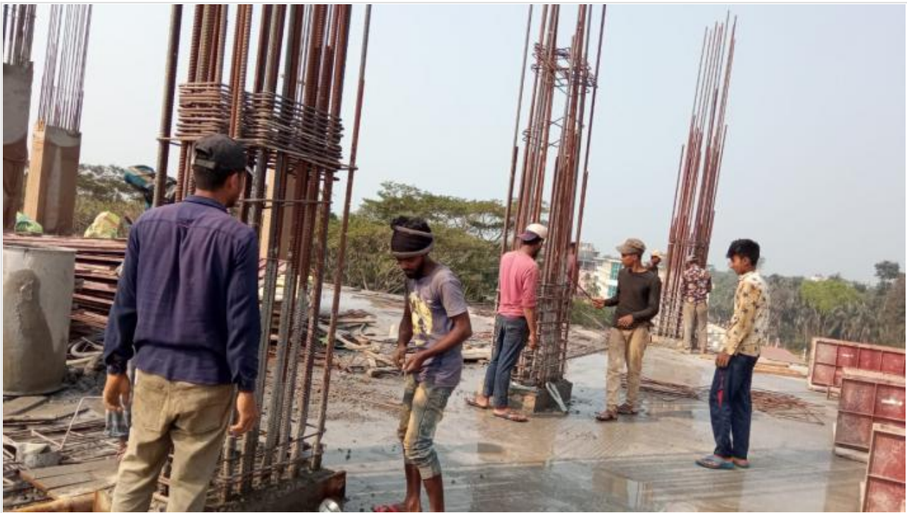
Tower-1-3rd Floor Column Re-bar Work on 23-02-21
