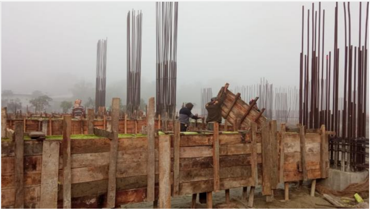
Tower-1-Grade Beam on 04-12-20
