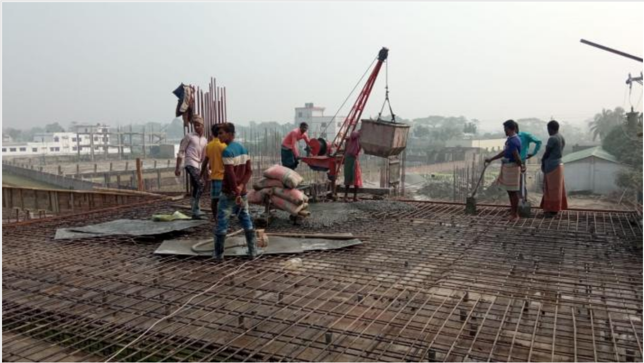
Tower-1-GF Roof Slab 1800 sft Concreting on 18-01-21
