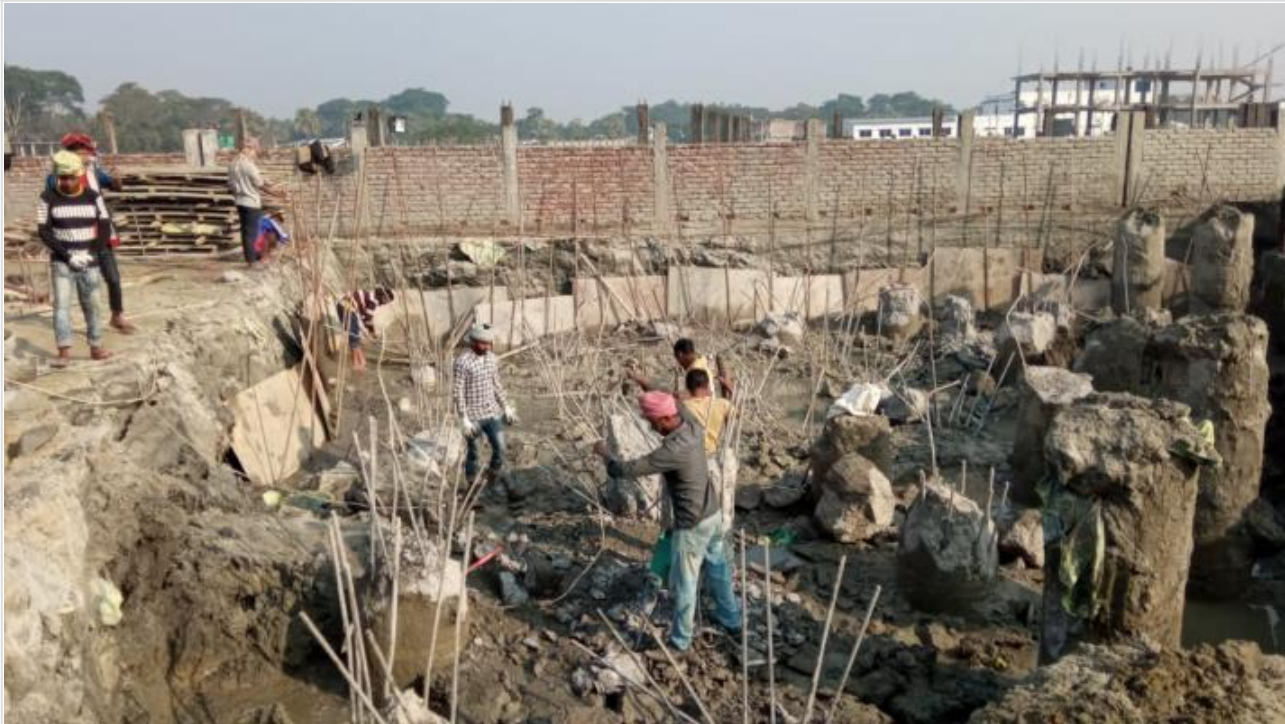
Tower-2-Pile Head Breaking on 27-12-20
