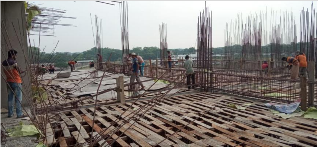
Roof Slab Shuttering on 04-05-21
