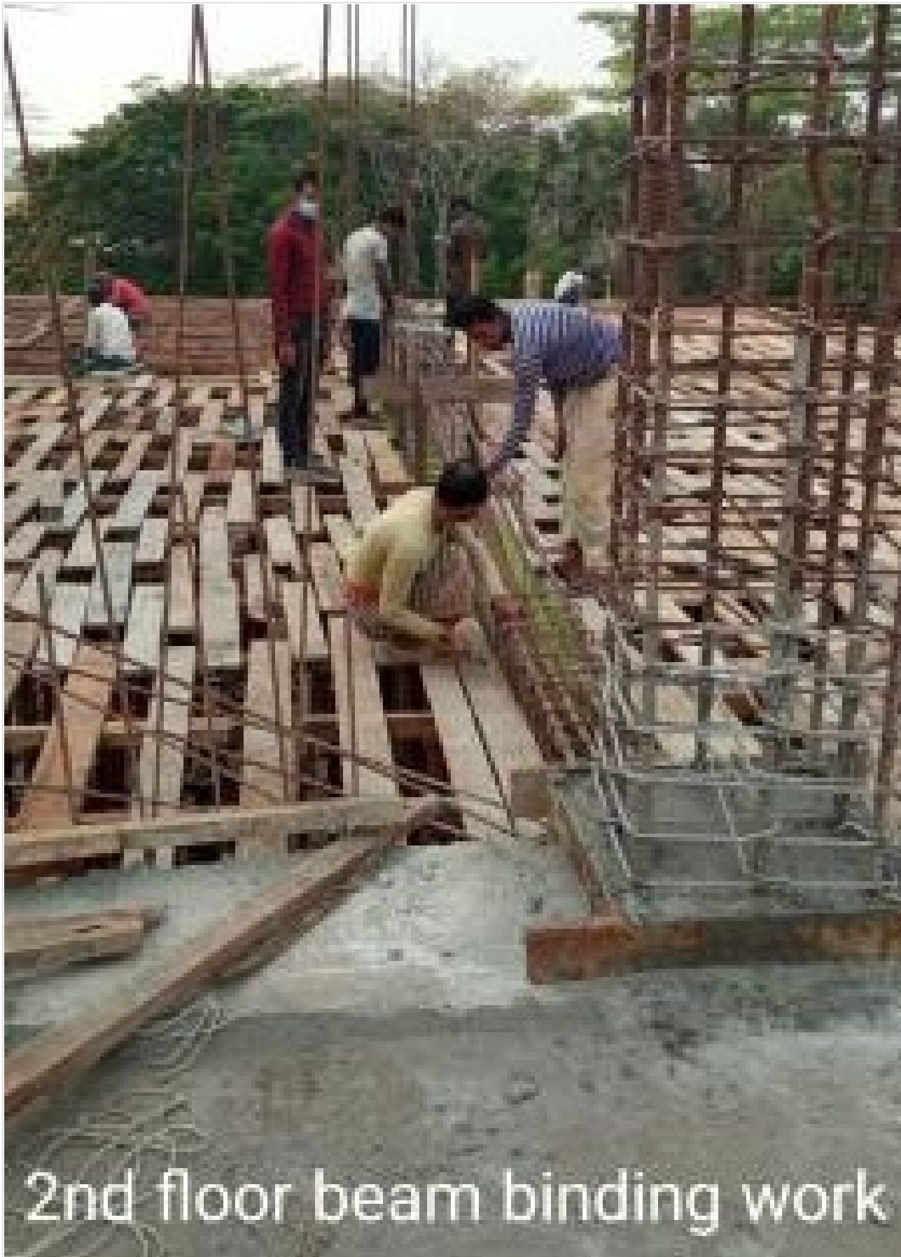
Restaurant-GF Double Ht Roof Slab-Re-bar on 30-03-21
