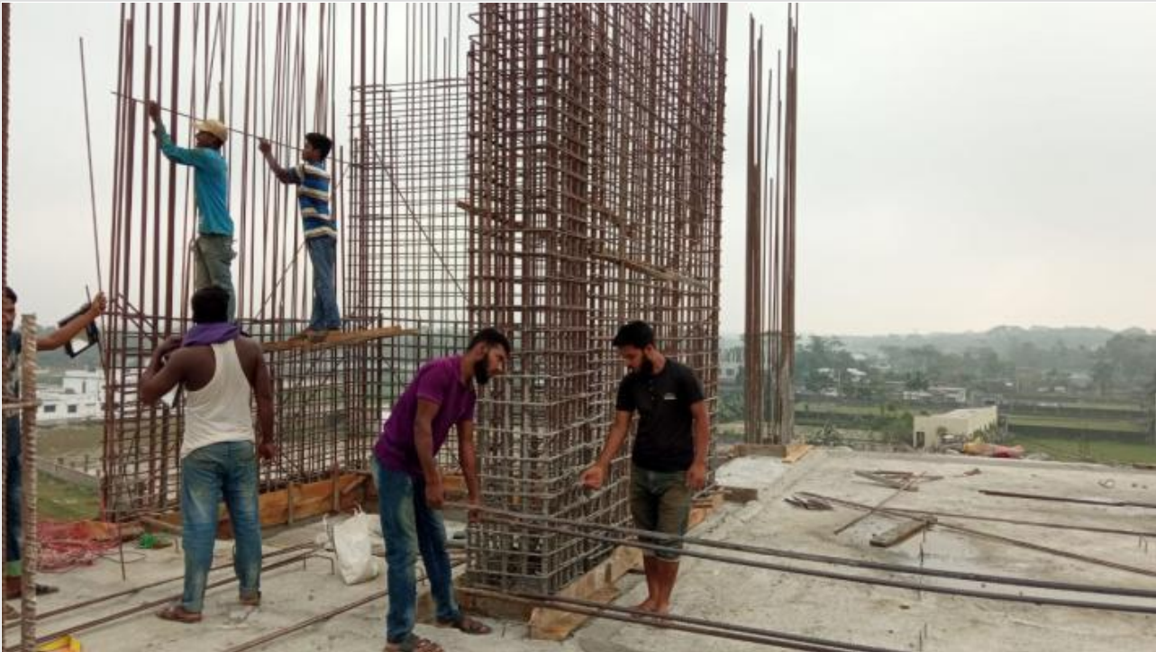
Tower-1-3rd Floor Lift Core Re-bar Work on 02-03-21
