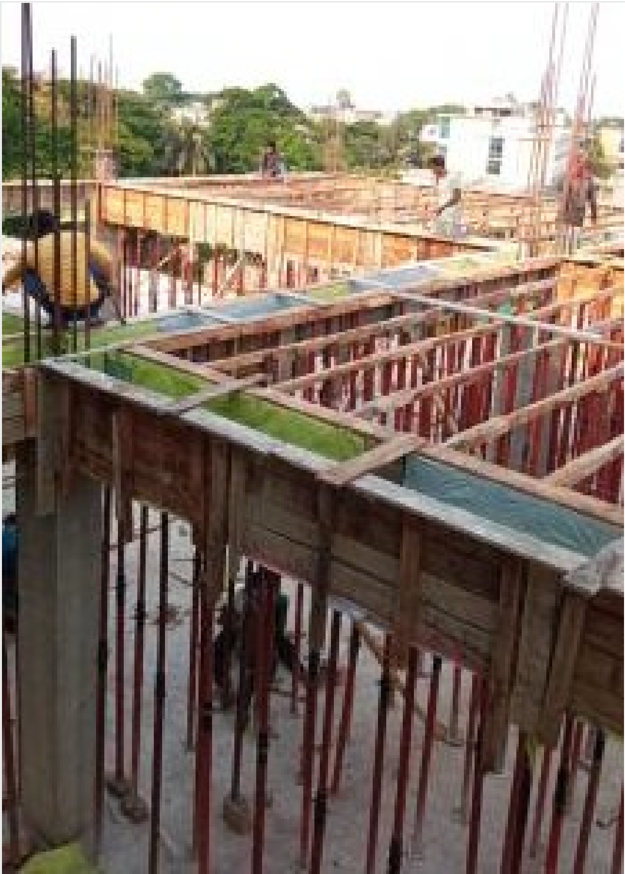
Beam Shuttering on 29-04-21
