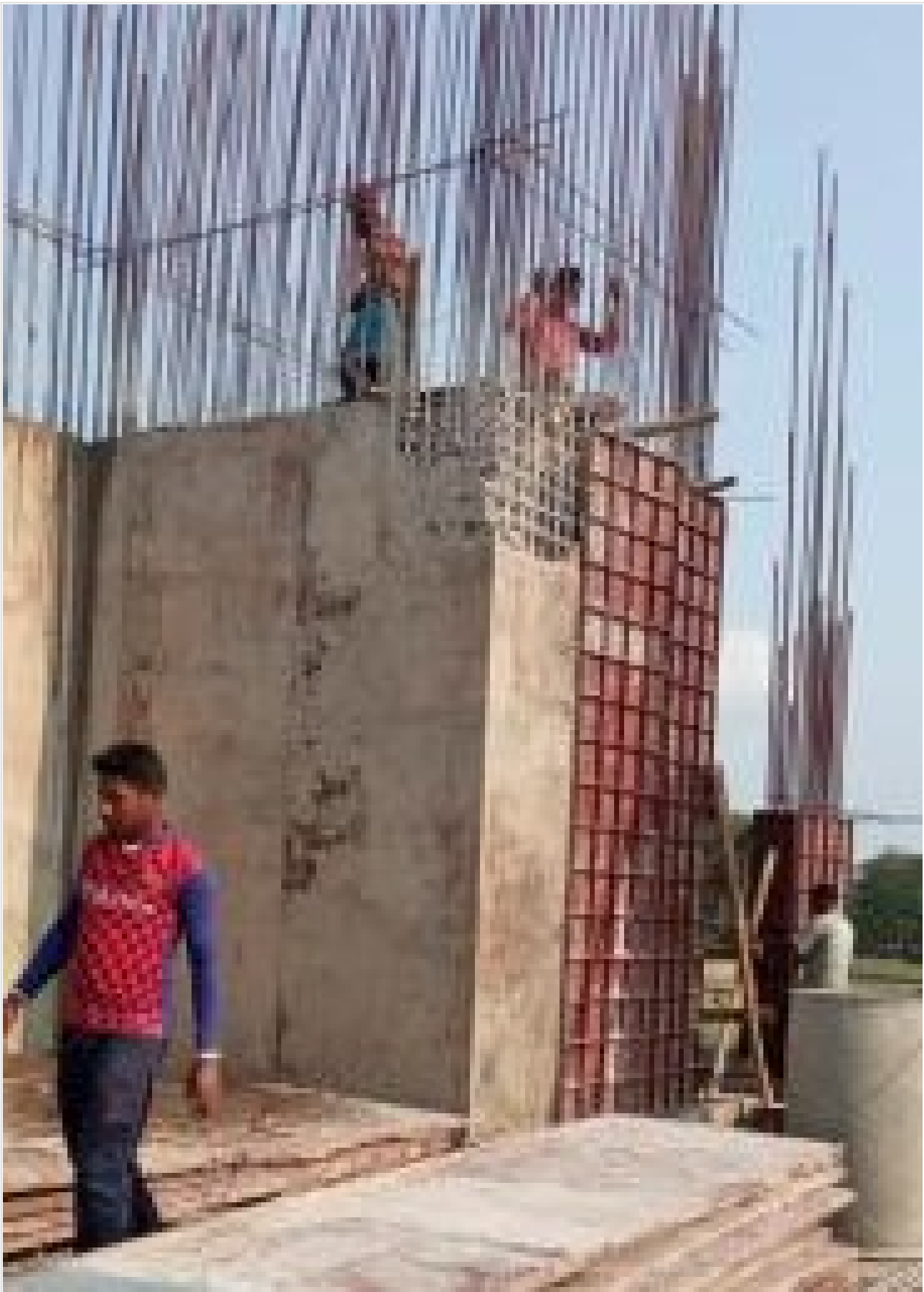
Tower-2-Lift Core Deshuttering on 02-05-21
