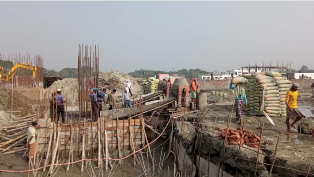
Tower-1-Pilecap Concreting on 12-12-20
