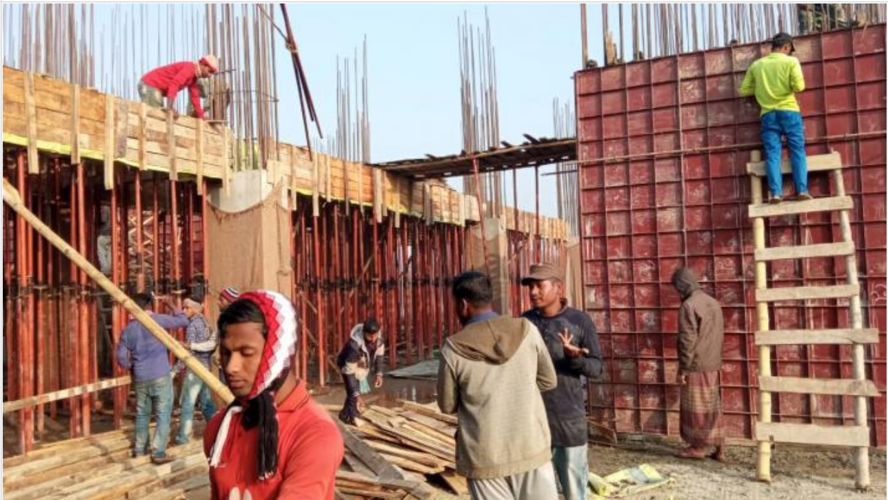
Tower-1-Lift Core and Slab Shuttering on 27-01-21
