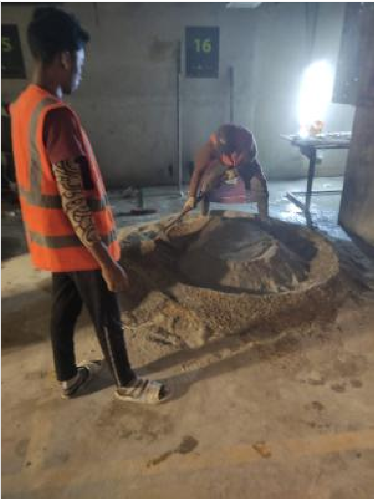
Retrofit-B2-Column Concrete on 27-02-23
