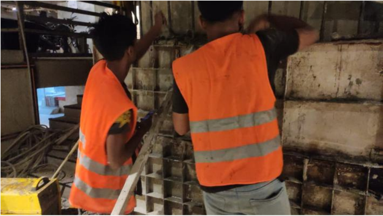
B-2-Column Retrofit shutter removing on 27-03-23
