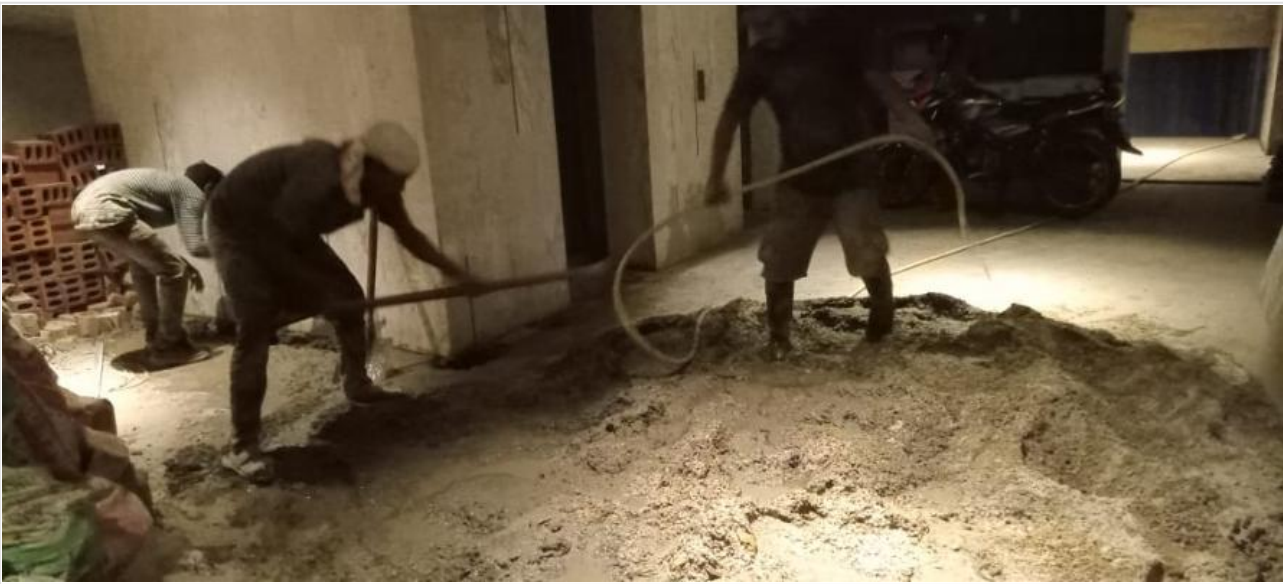
Basement-3 Lift-wall Concreting on 09-01-23
