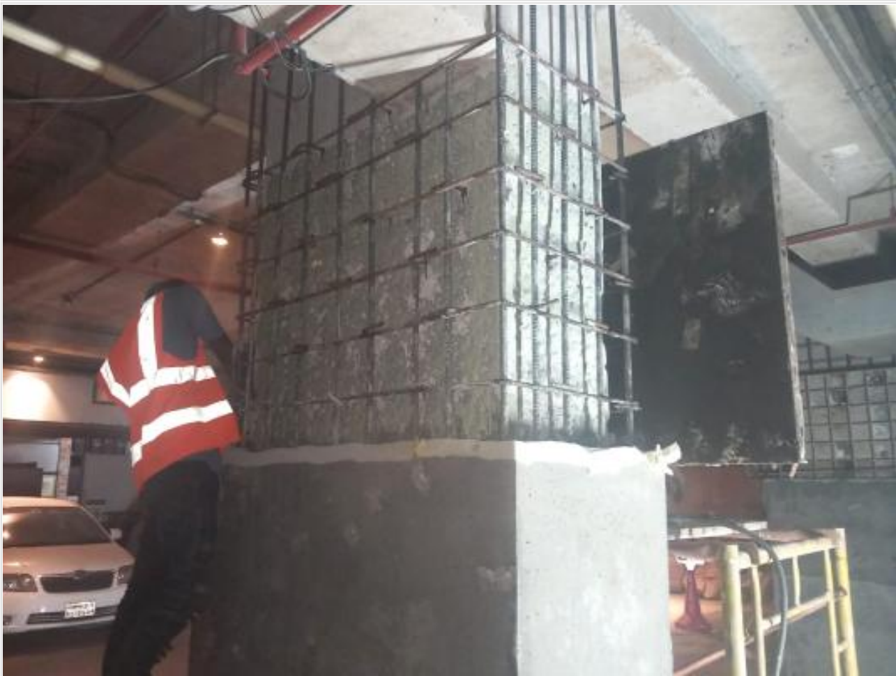
B-1-Column retrofit re-bar work on 09-03-23
