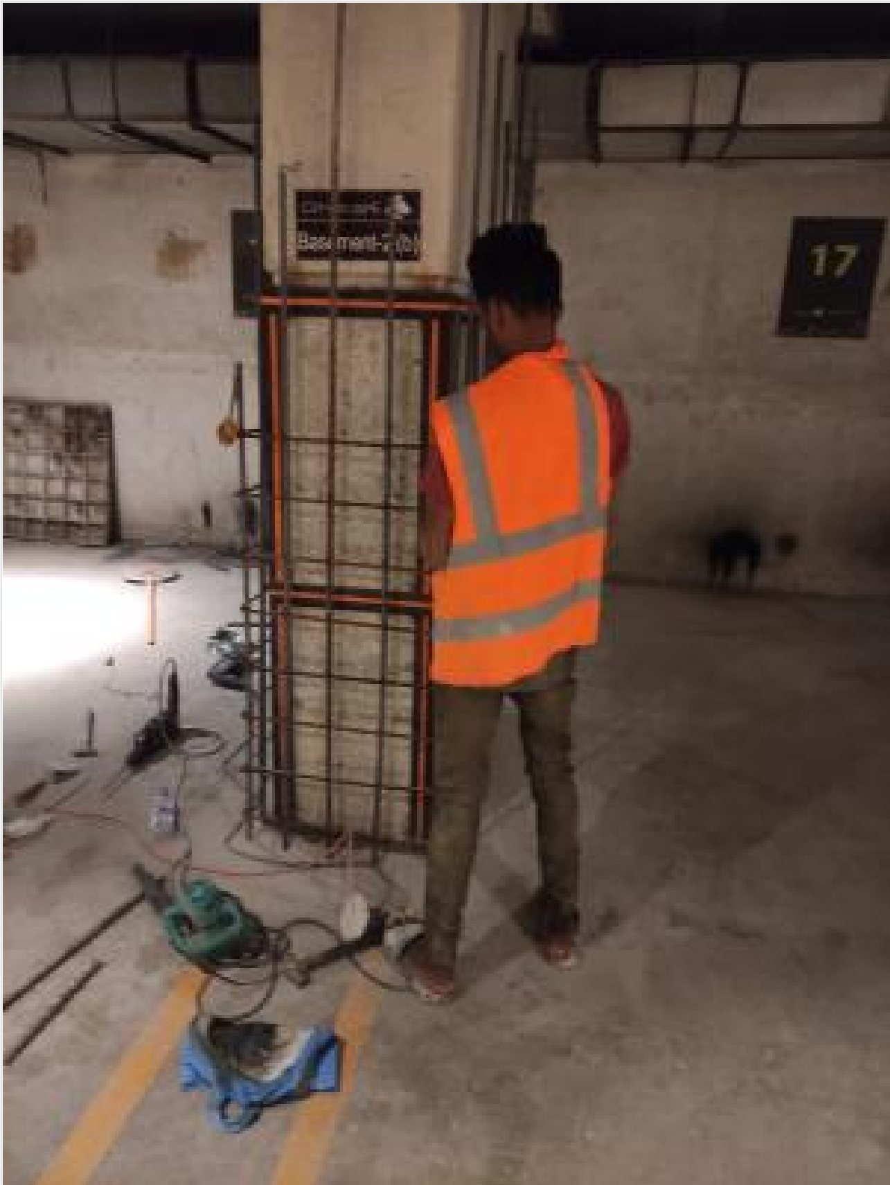
B-2 Col retrofit re-bar work on 15-02-23
