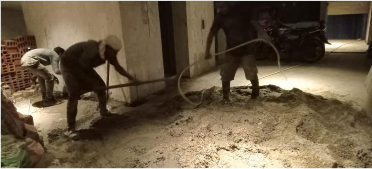
Basement-3 Lift-wall Concreting on 09-01-23
