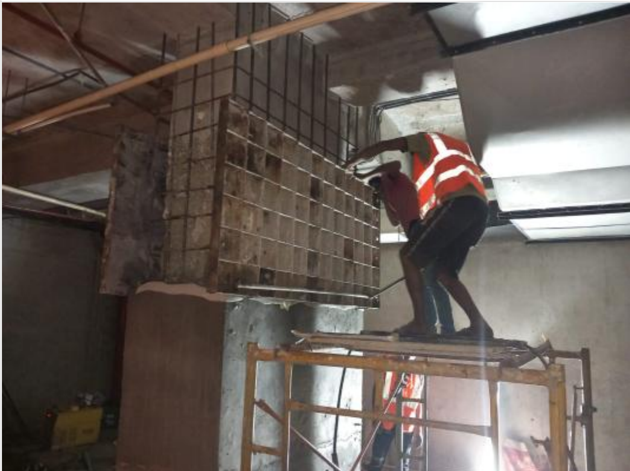
B-1-Column retrofit re-bar work on 09-03-23
