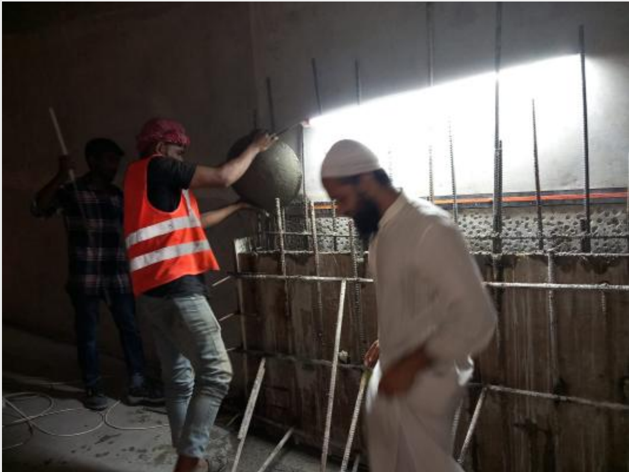
B-2-Column retrofit concreting on 29-03-23
