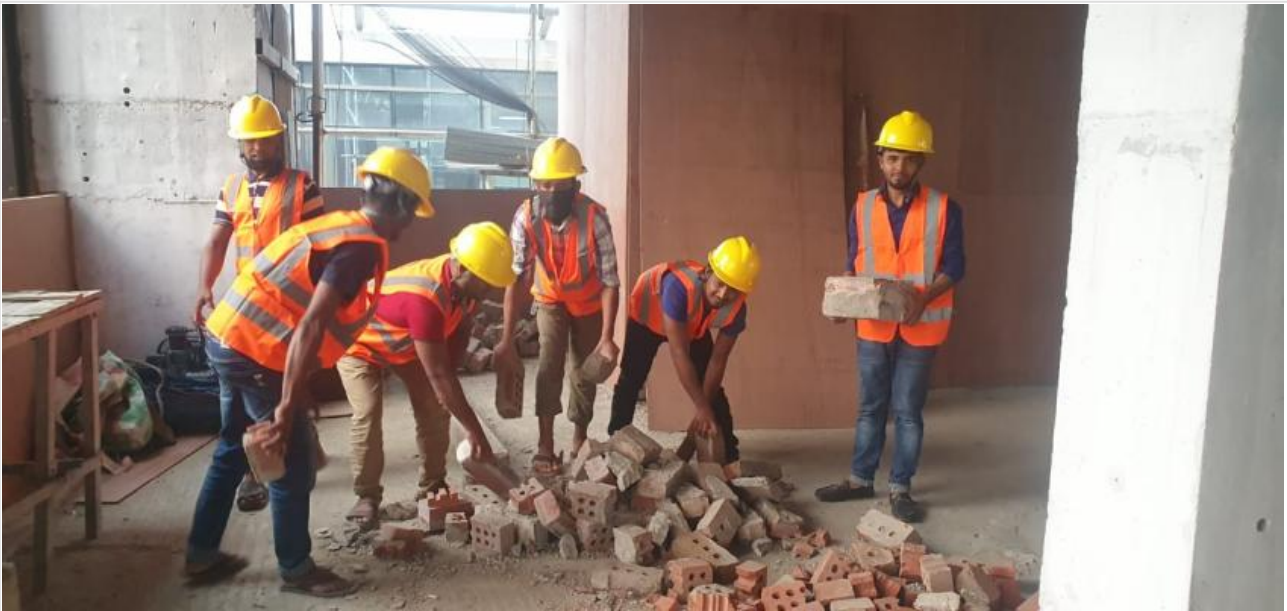
Brick work demolition on 22-12-22
