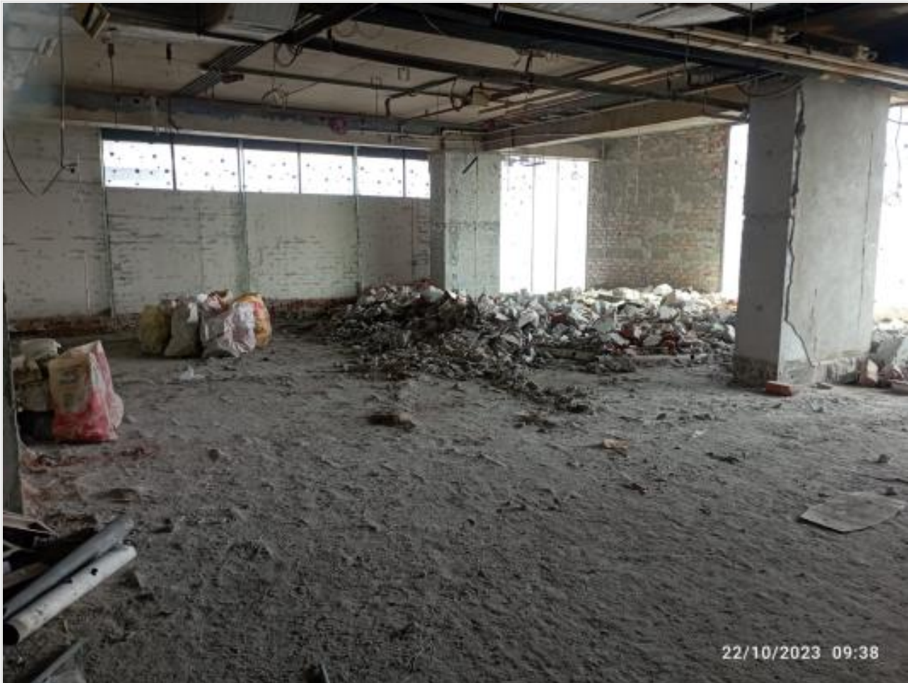
L-14-Kitchen Area on 23-10-23
