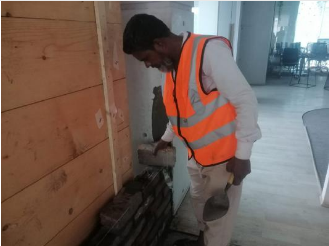
L-11-Steam n Suana-Brickwork on 29-11-23
