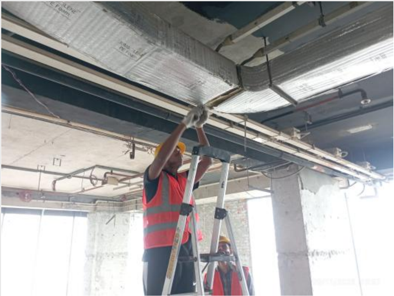
L-14-Old AC duct removing on 09-11-23
