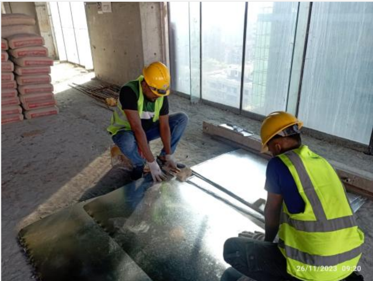
L-14-AC Duct fabrication on 26-11-23
