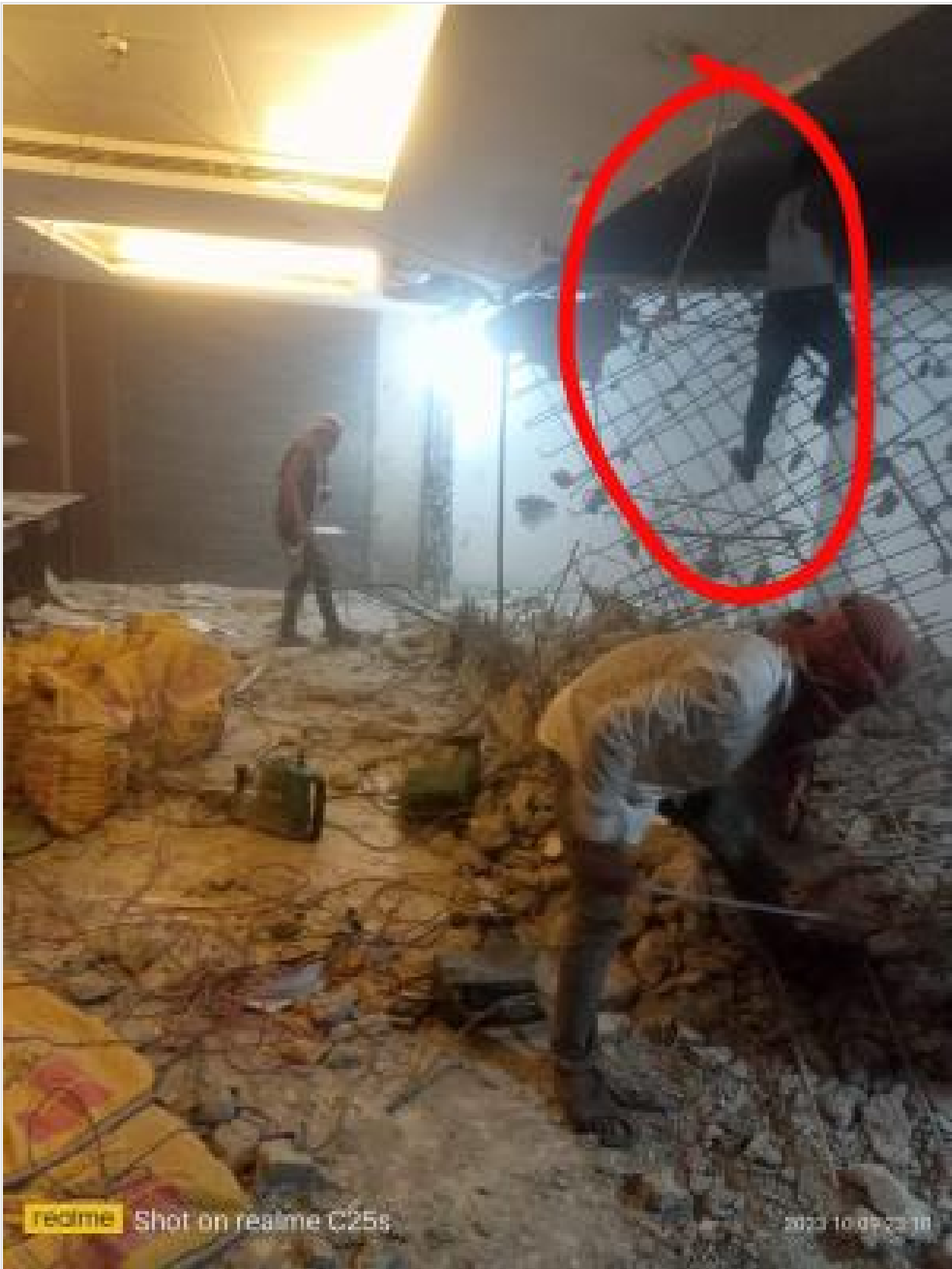
L-4-North Vault dismantling on 09-10-23
