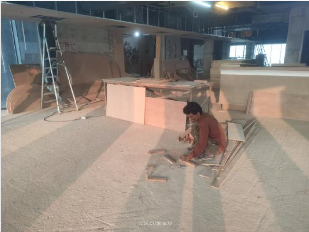
L-14-False Ceiling Work on 08-01-24
