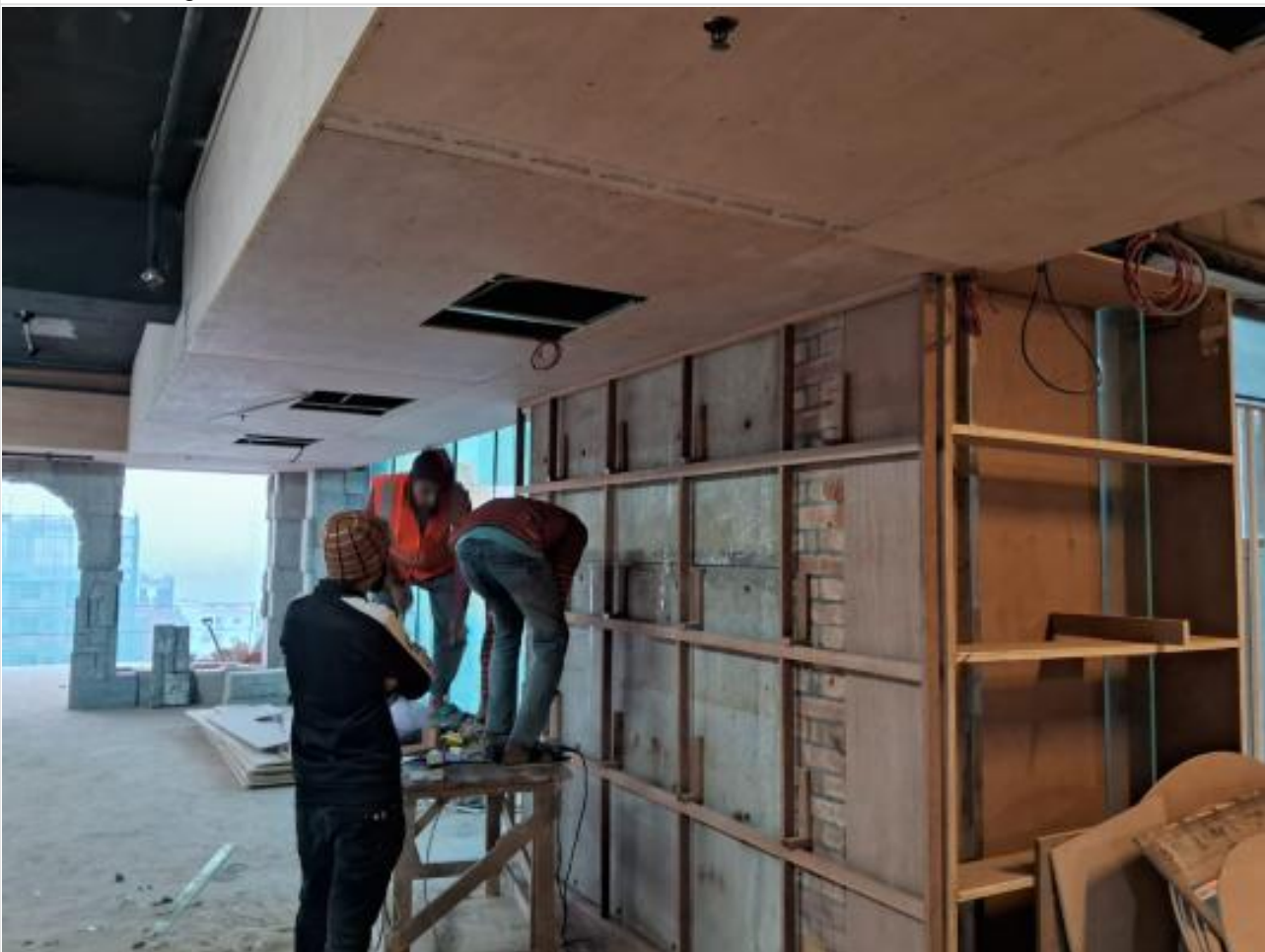
L-14-False Ceiling Work on 17-01-24
