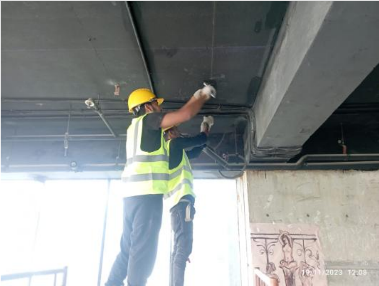
L-14-AC Installation on 19-11-23
