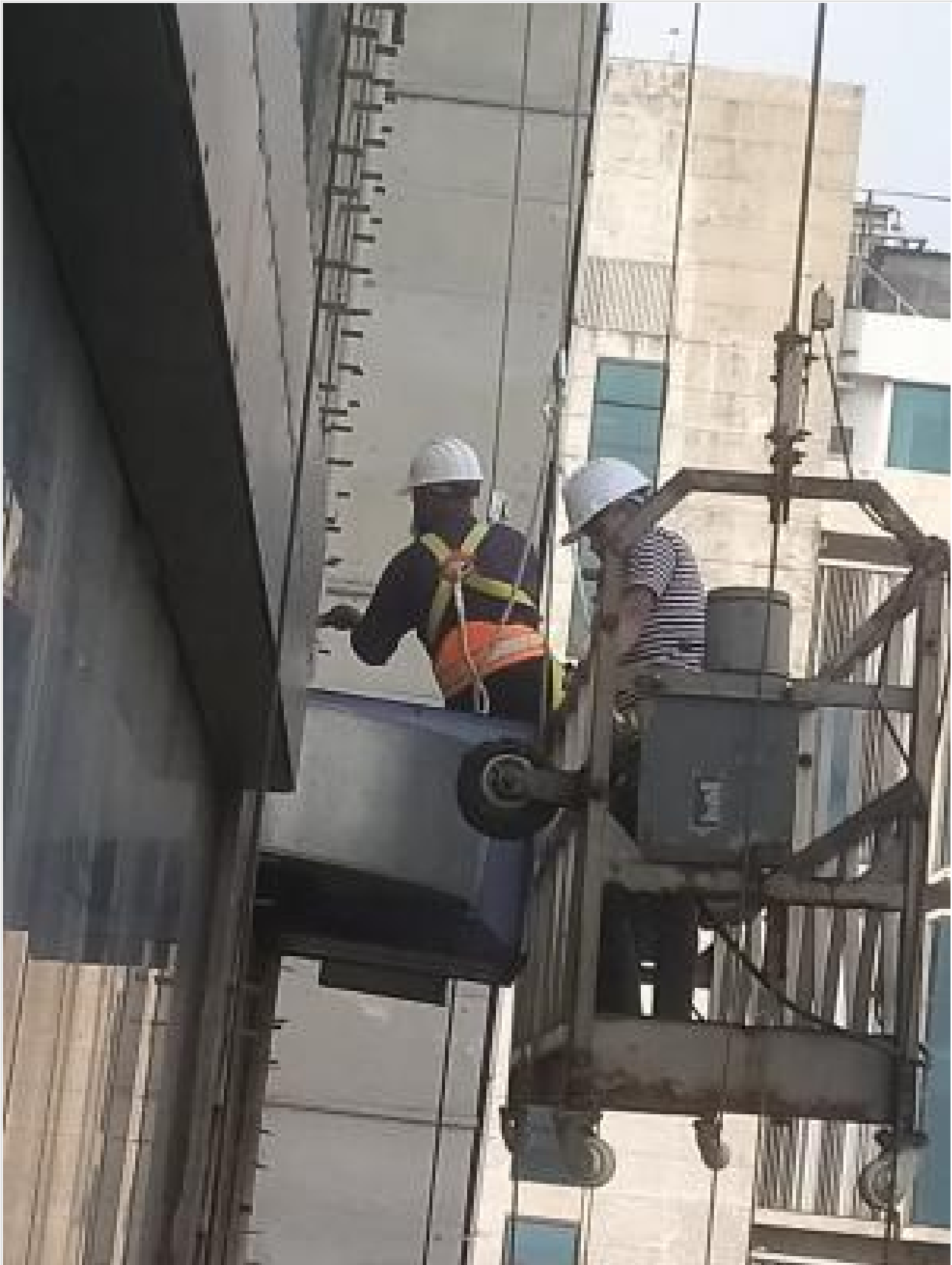
L-11-Steam-Suana-Plumbing work on 10-12-23
