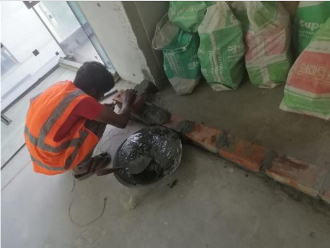
L-11-Steam n Suana-Brickwork on 28-11-23
