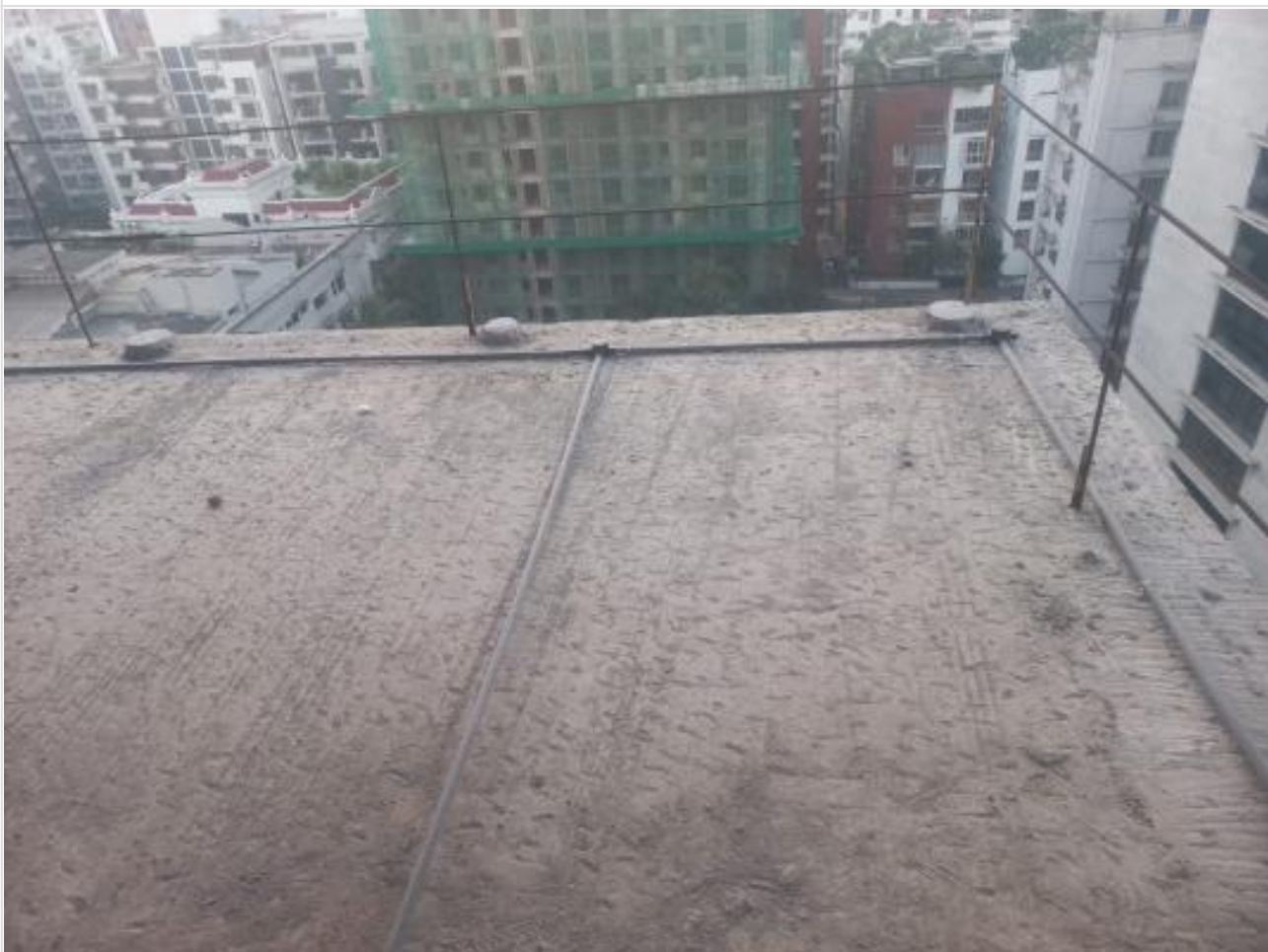
L-14-Electrical Pipe Laying on 26-11-23
