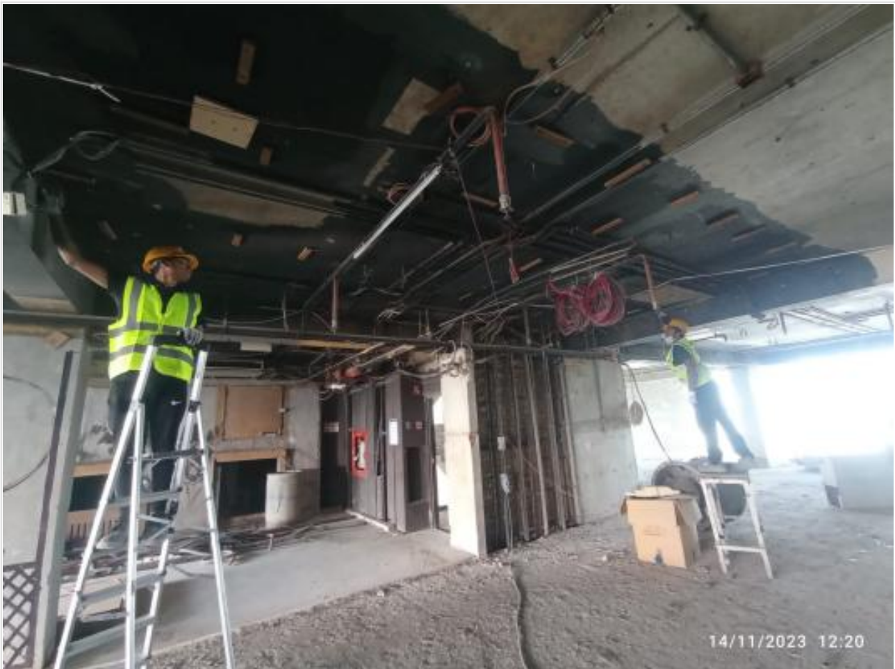
L-14-AC installation on 14-11-23
