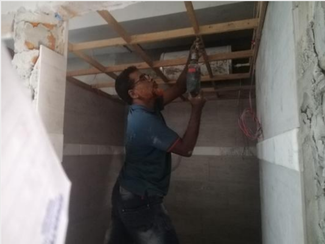
L-11-Steam-Suana-False Ceiling on 28-12-23
