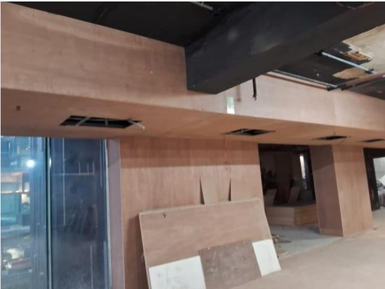
L-14-False Ceiling and Interior on 22-01-24
