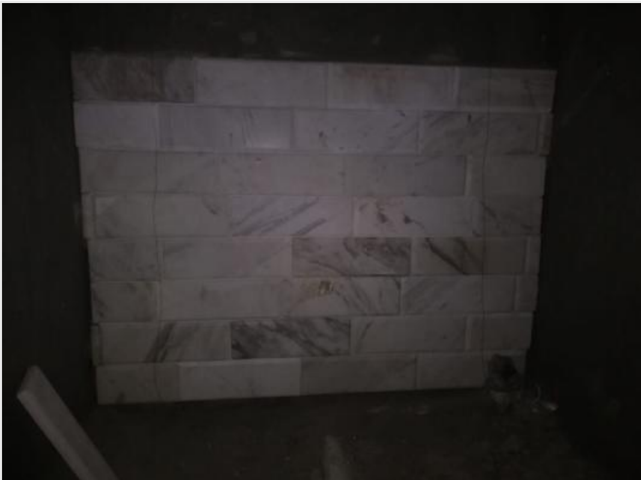
L-11-Steam-Tile Work on 17-12-23
