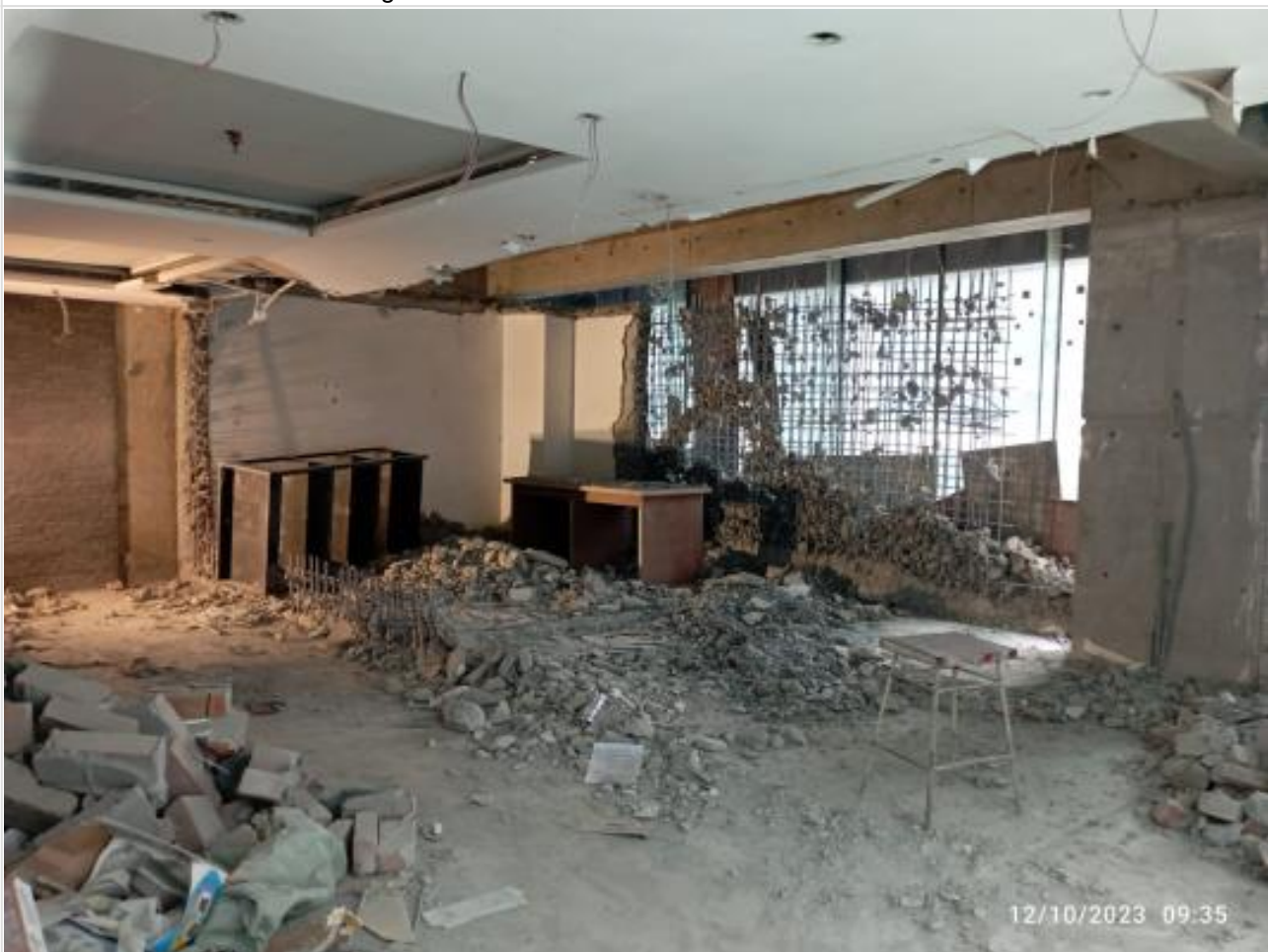
L-4-North Vault dismantling on 11-10-23
