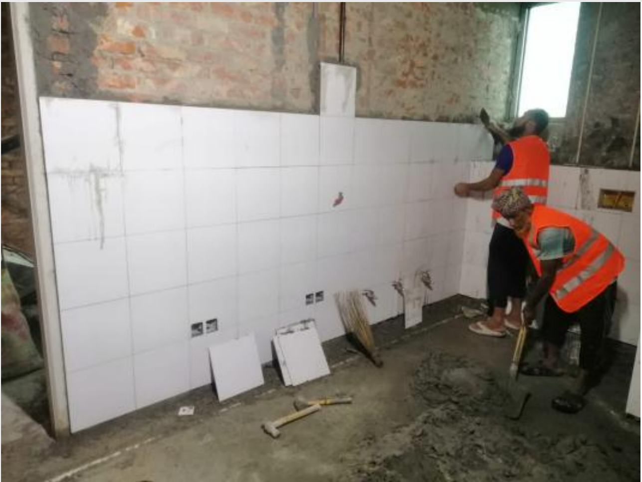
14th Floor-Kitchen Tile Fixing on 30-06-24
