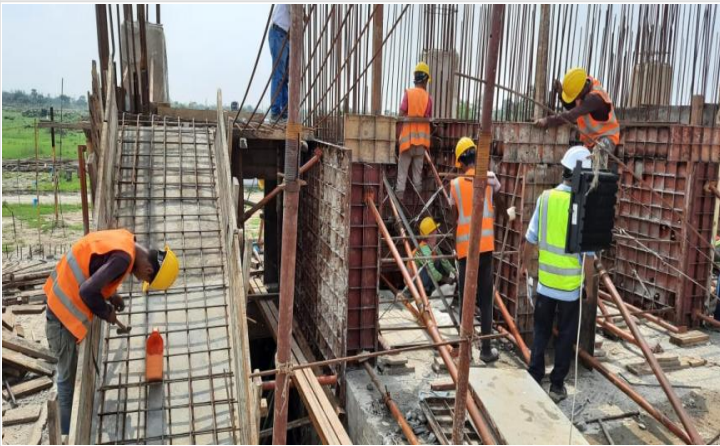
Ground Floor Stair Re-bar work on 09-06-21
