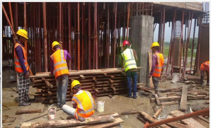
1st floor Slab Shuttering on 15-06-21
