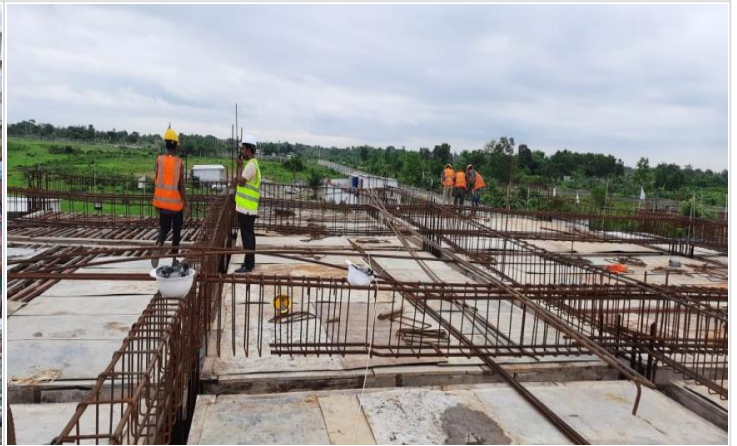
1st floor Slab Shuttering on 12-06-21
