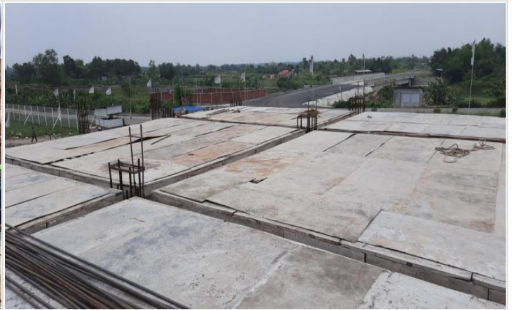
1st floor Slab Shuttering on 09-06-21
