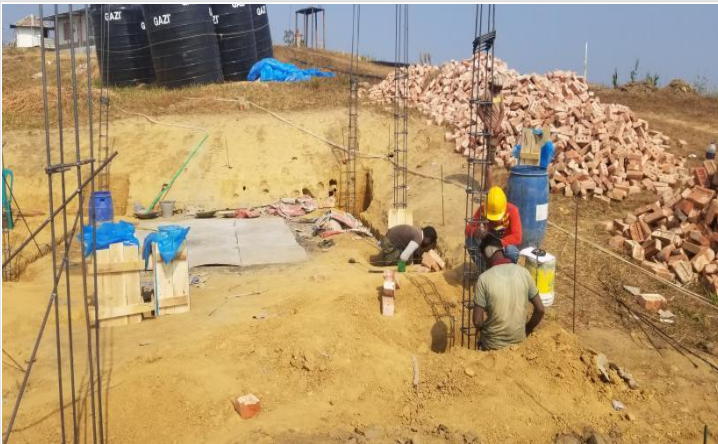
Shuttering fitting work for short column on 16-01-21
