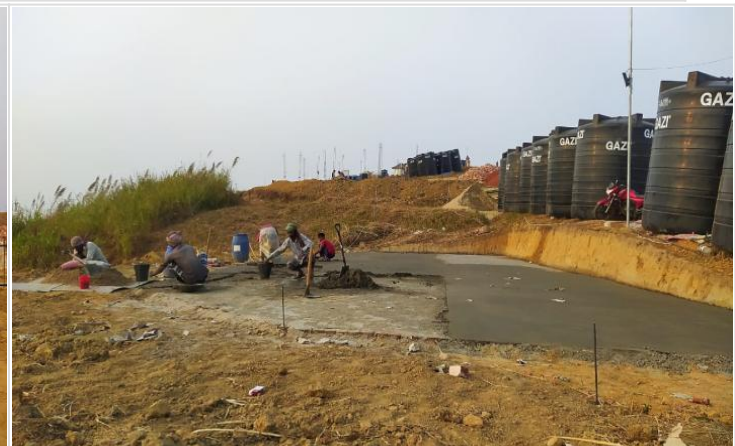
Solling joint fillup & plaster work at w on 21-01-21
