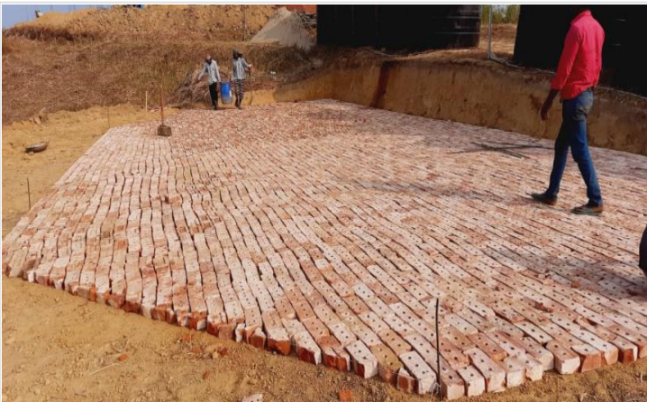
Soling for PVC Water Tank on 20-01-21
