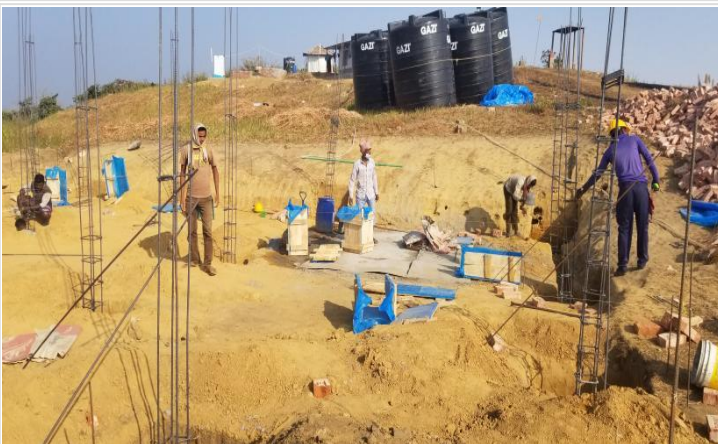
Shuttering fitting work for short column on 17-01-21
