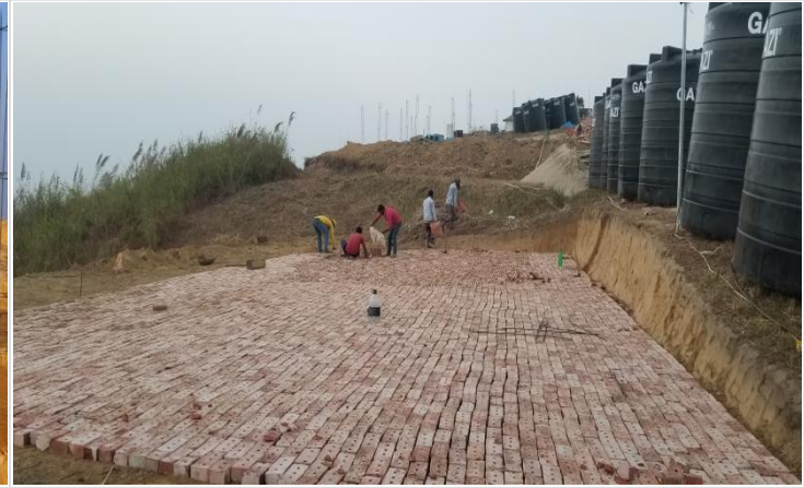
Brick solling work for water tank placei on 19-01-21
