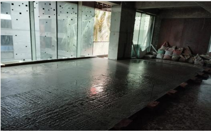
4th Flr-Floor Raining Concreting Complet on 10-07-24
