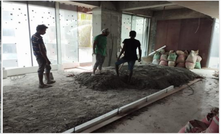
4th Flr-Floor Raising Concreting on 09-07-24
