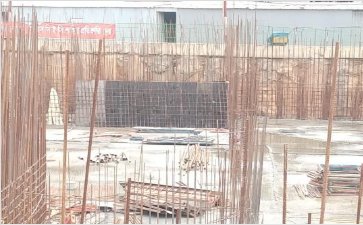
South stair shutter on 03-02-22
