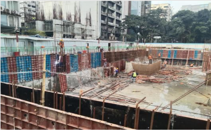
Retaining wall shuttering on 20-02-22
