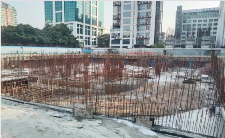
Basement-1-south retaining wall-Re-bar on 16-02-22
