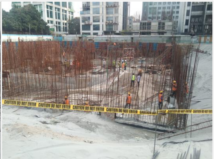
Basement-1-North Retaining wall-1st Lift
