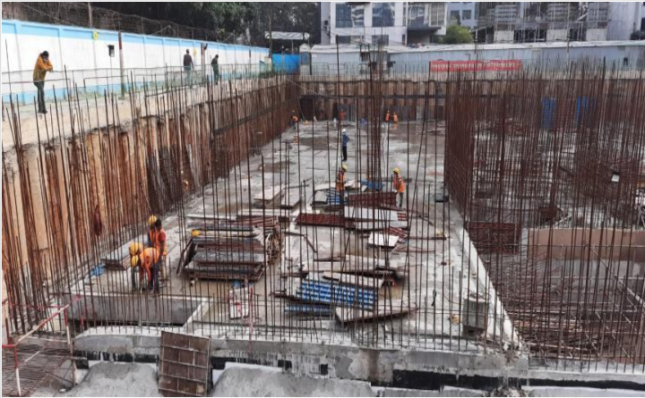
South Retaining wall on 09-02-22
