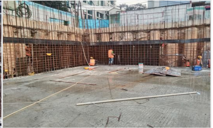
South Retaining wall shuttering on 09-02-22
