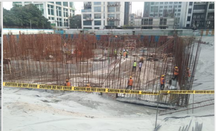
Basement-1-North Retaining wall-1st Lift on 28-02-22
