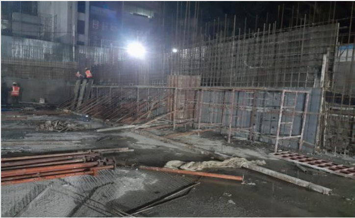
Shuttering work on 18-02-22
