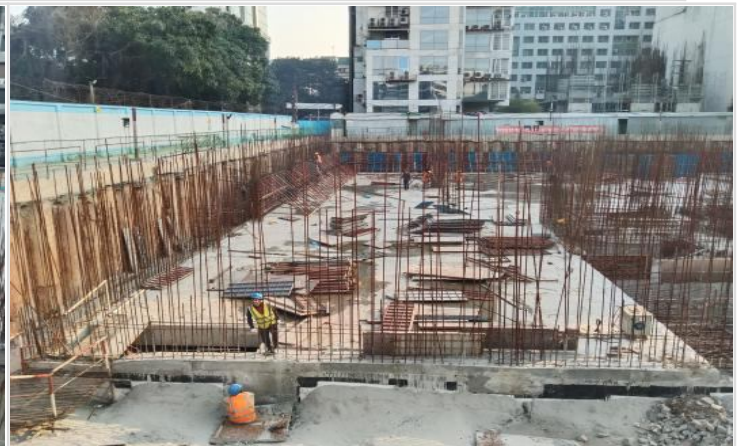
Basement-1-South Retaining Wall-Shutteri on 12-02-22
