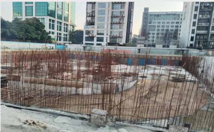
Basement-1-South Retaining wall on 12-02-22
