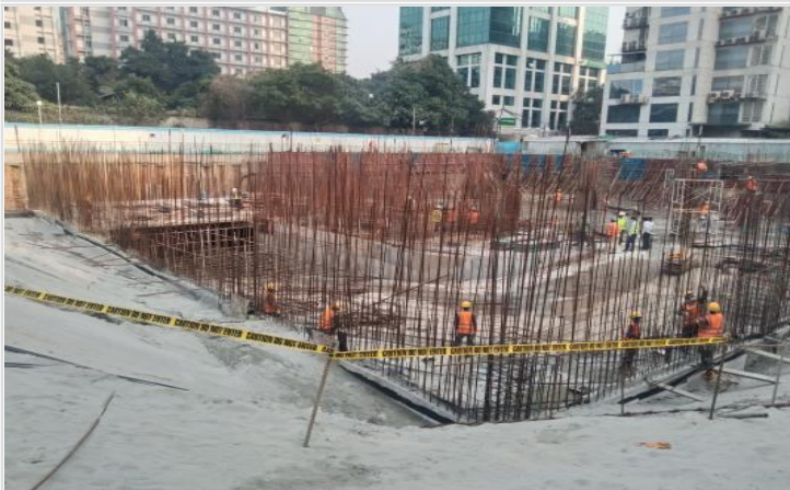
B-1-North retaining wall rebar work on 28-02-22
