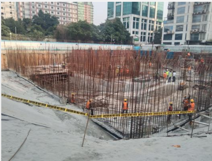
B-1-North retaining wall rebar work
