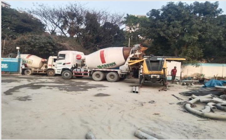
Ready-mix Concrete Truck and Pump on 26-02-22
