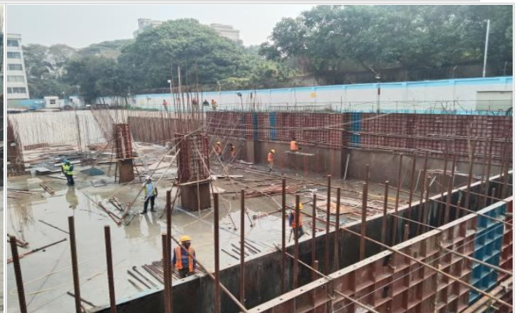
Basement-1-South Column shuttering on 23-02-22
