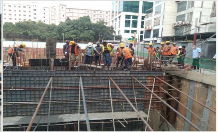
B-1-South 2nd Retaining wall concreting on 26-02-22
