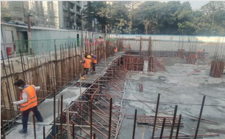
Basement-1-South retaining wall 2nd lift on 16-02-22
